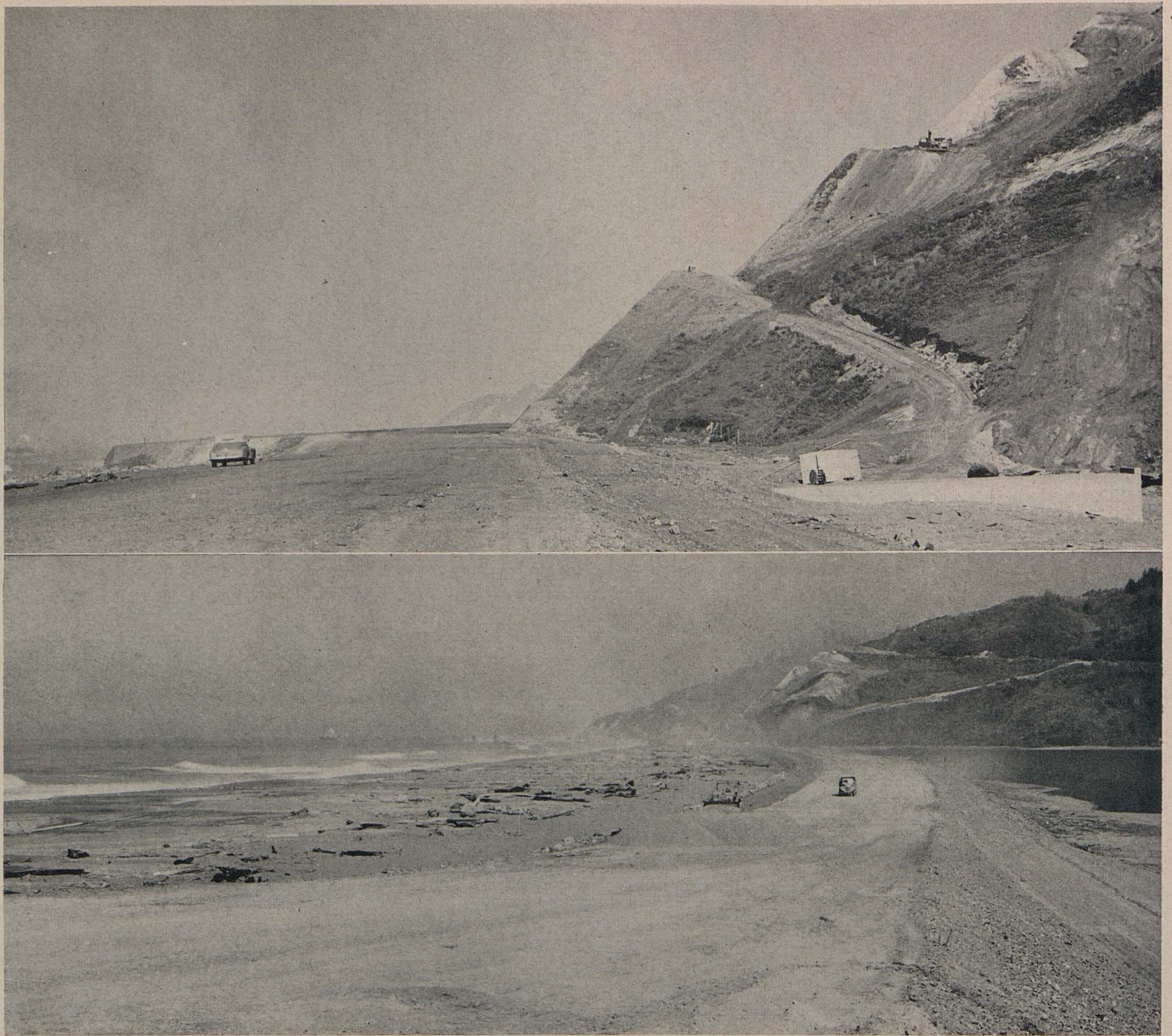
UPPER—View of completed 220-foot-high cut at Lookout Point near the north end of the project. This point was the location of the ancient Indian burial ground unearthed during construction operations. In the foreground is the equalizer culvert to control the water elevation in Freshwater Lagoon to the right. LOWER—View of new location along the sand spit with Freshwater Lagoon on right and Pacific Ocean on left. In the far distance is Lookout Point. The old highway can be seen at upper right
