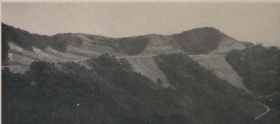
Extensive cut and fill area exposed to erosive forces by construction of this high-standard mountain road. Compare with old road at lower right. (Near San Marcos Pass above Santa Barbara)
