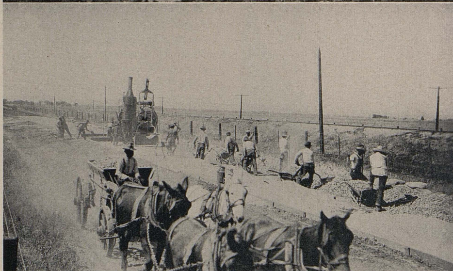
UPPER—This is U. S. 101 in Ventura County in 1916. Mr. Gibson is again stalled in the mud. LOWER—Pick and shovel crews and mule drawn equipment built highways for Mr. Gibson in 1916. This photo was taken on U. S. 99 in Butte County
