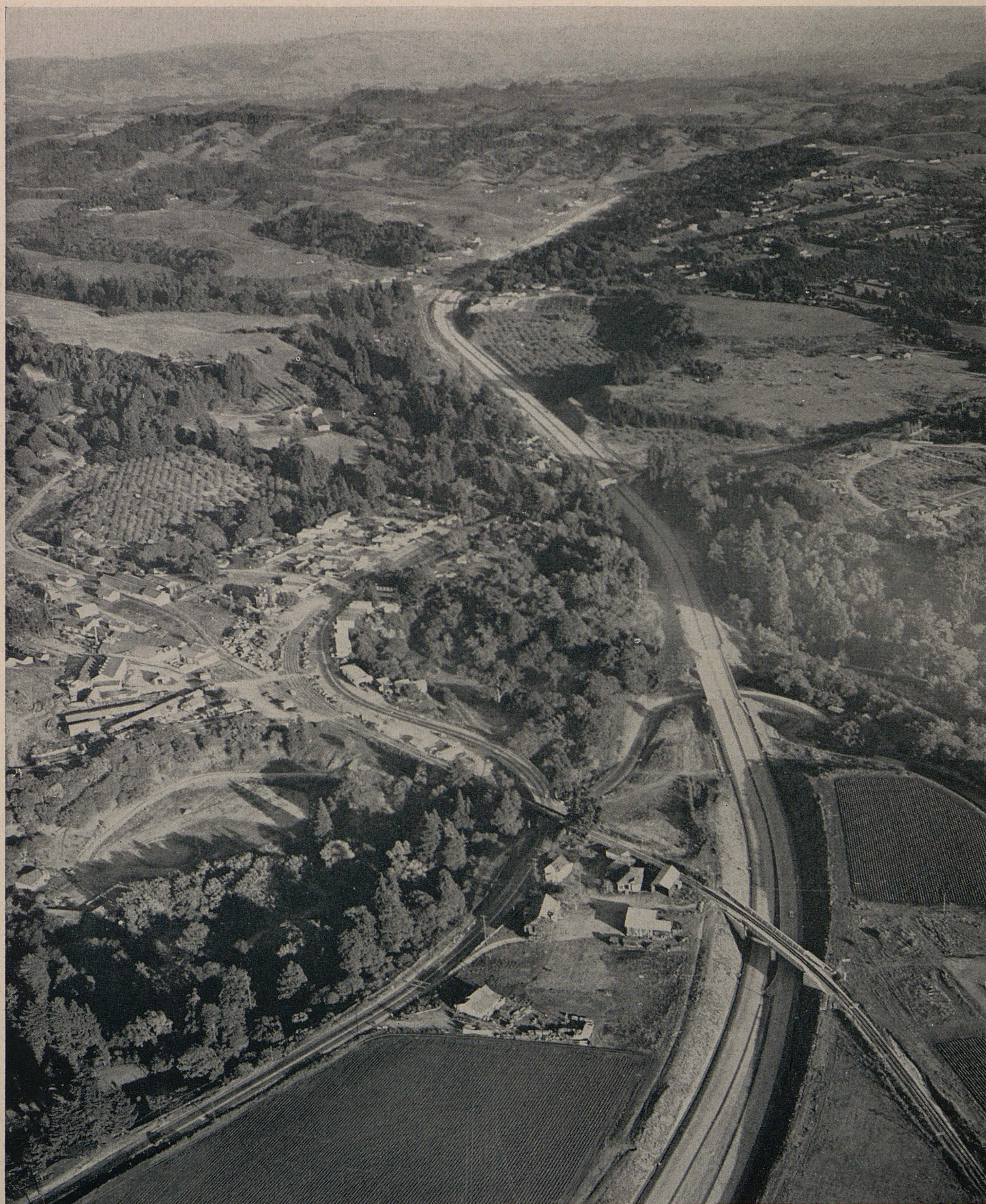
Aptos Creek Bridge looking toward South Aptos Railroad Underpass with North Aptos Underpass in the foreground. Town of Aptos in left center and Public Works
