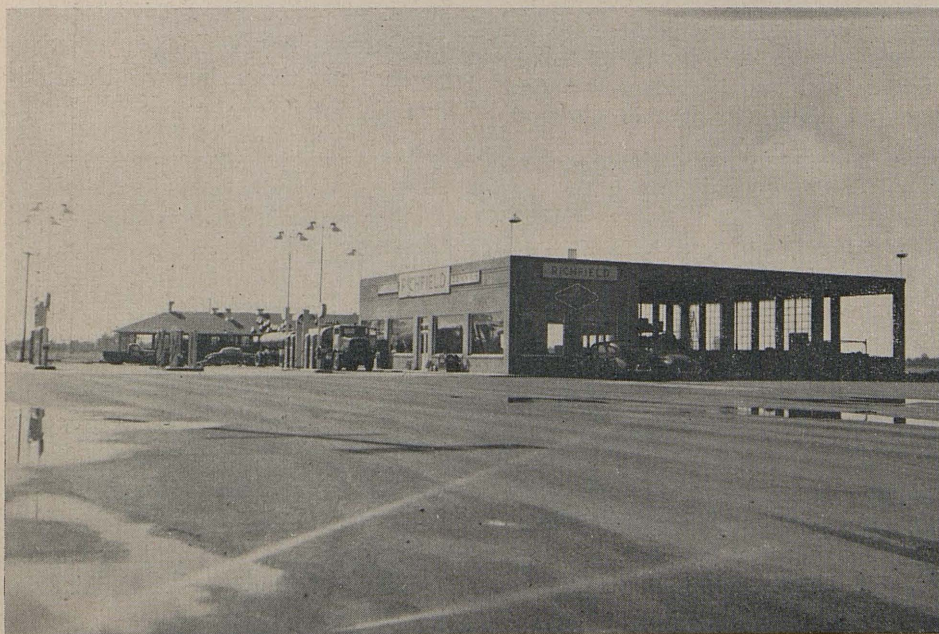
This large truck-service station was constructed upon one of the investigated properties subsequent to the freeway development. This station is located on the outer highway
