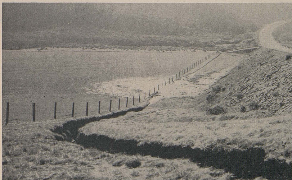
Adjacent property affected by debris from eroded highway drainage ditch. (On Coast Route, south of Half Moon Bay, San Mateo County)
