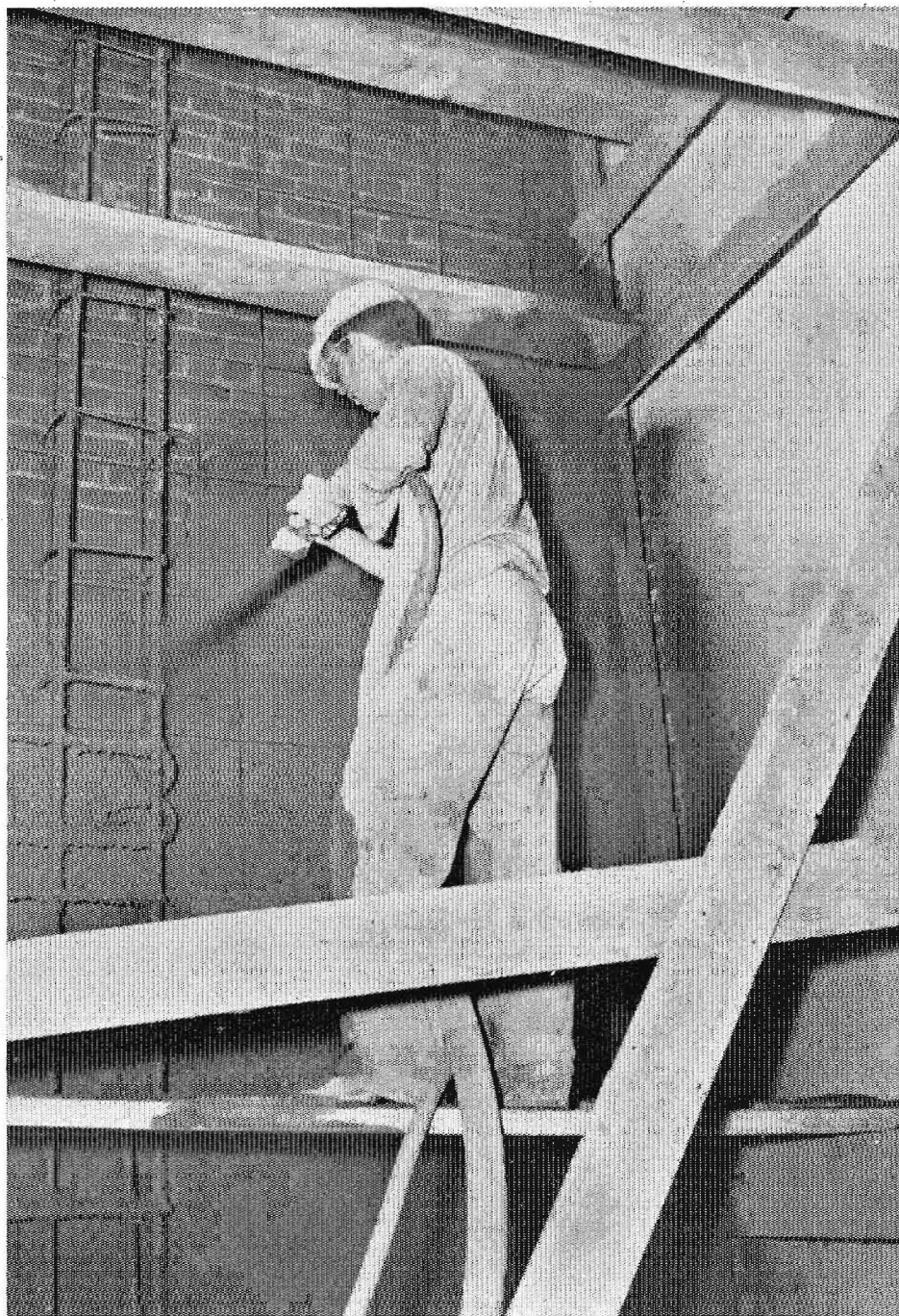
Strengthening center brick wall below second floor with gunite
