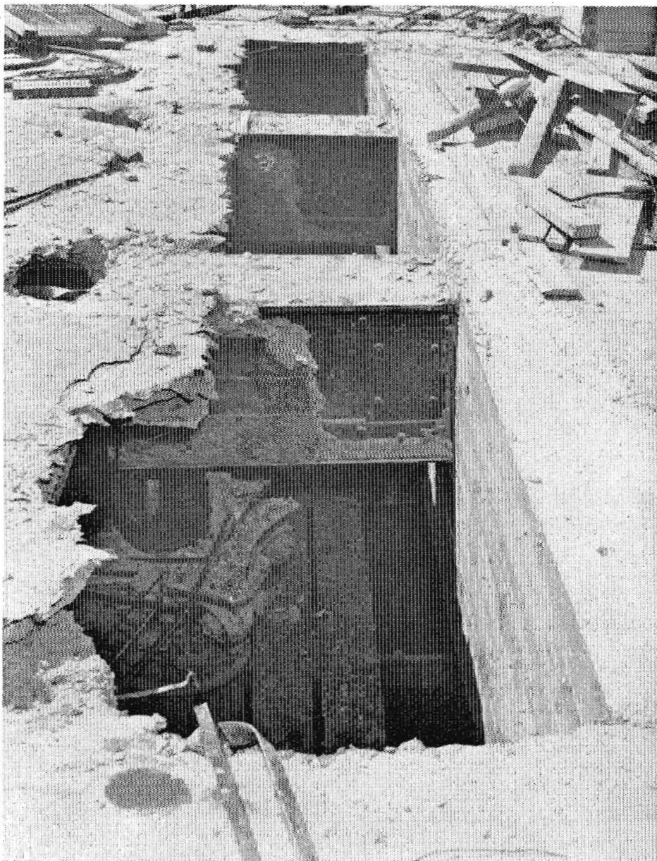
View of fourth floor level, showing box girders at cut line
