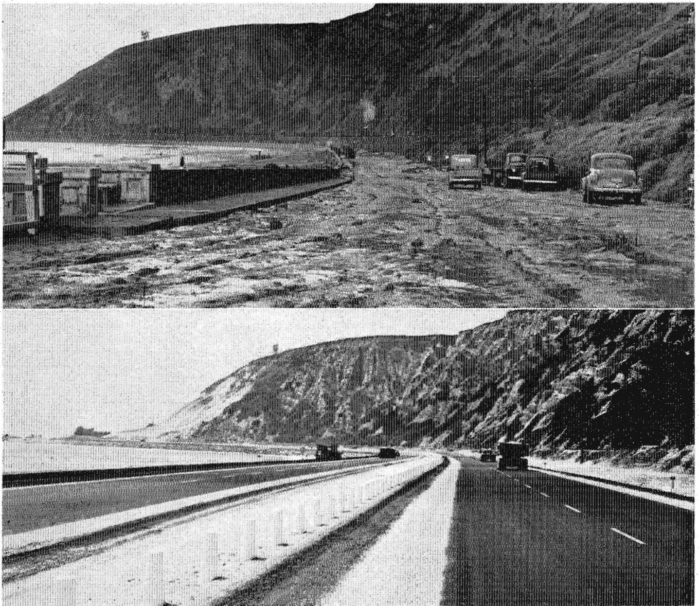
UPPER—View looking northwesterly from Seacliff, showing storm damage of October 18, 1934. LOWER—View looking northwesterly from approximately same location, taken August, 1949, showing completed four-lane divided highway
