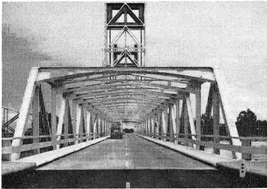
Looking southerly along bridge. The new bridge roadway is 26 feet in width with two 3-foot 6-inch sidewalks
