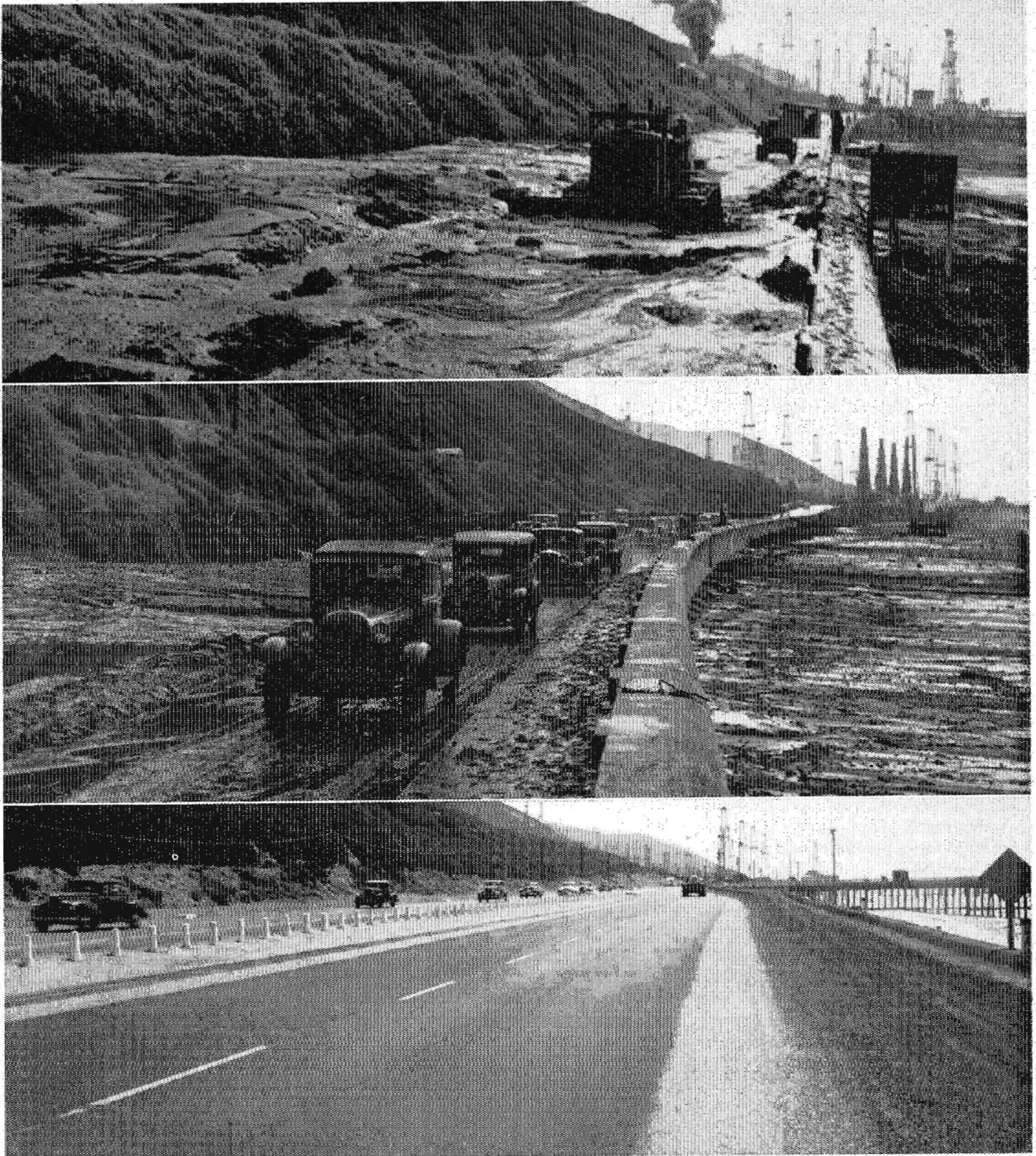
UPPER—View southeasterly looking toward Seacliff oil wells, showing storm damage March 1, 1941. CENTER—Looking southeasterly toward Seacliff oil wells, showing storm damage of October 18, 1934. LOWER—View from approximately same location, taken August, 1949, showing completed four-lane divided highway
