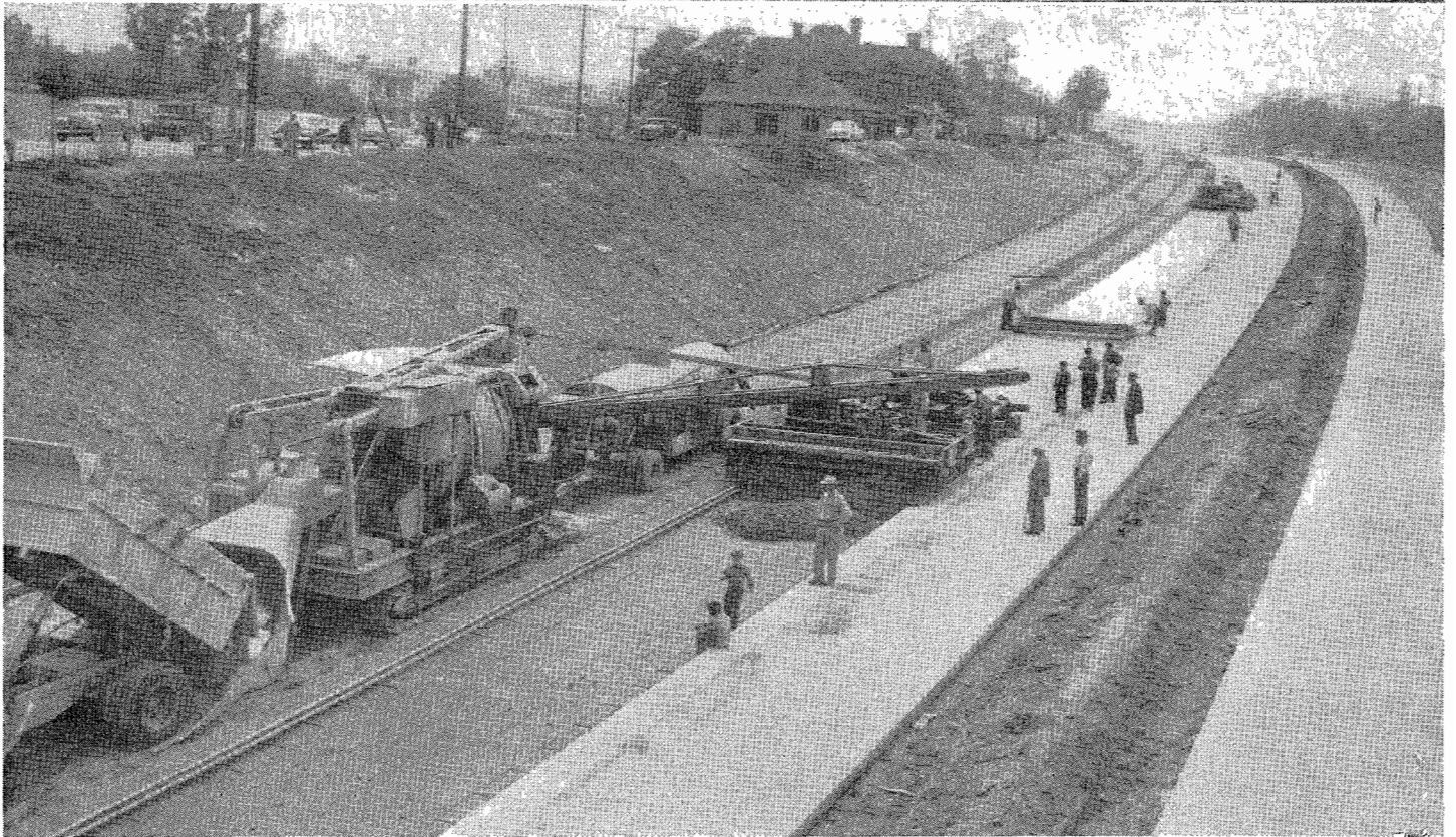
UPPER—Portland cement concrete paving operations at Edgware Road Overcrossing. Looking east with fire station on left. LOWER—Portland cement concrete paving operations as viewed looking west from the Edgware Road Overcrossing
