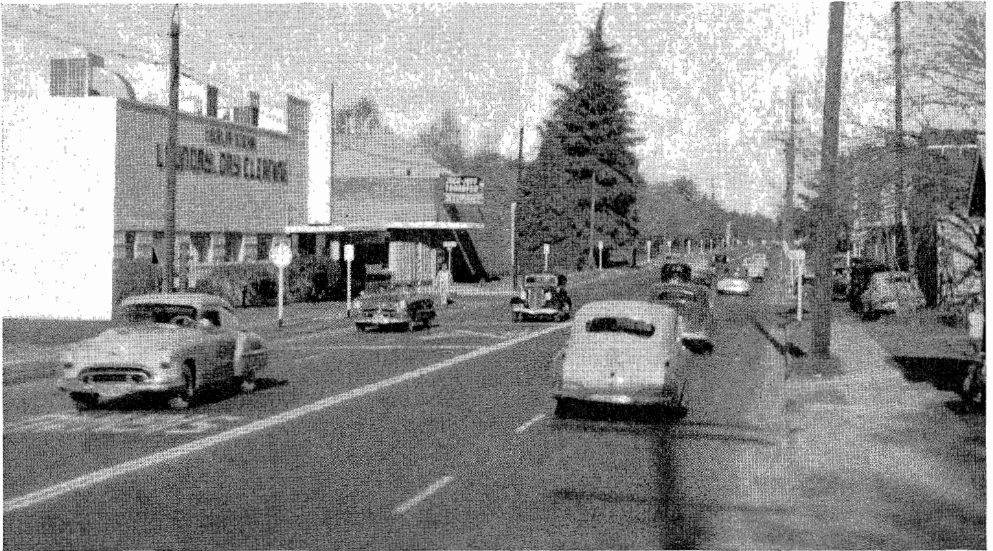
Mineral King Avenue in Visalia now is handling a heavy flow of traffic without congestion due to elimination of parking
