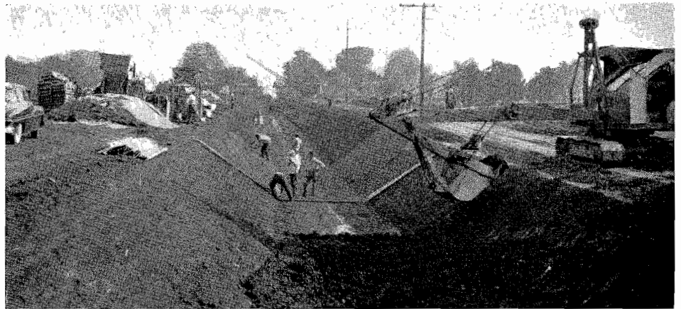
Irrigation canal under construction
