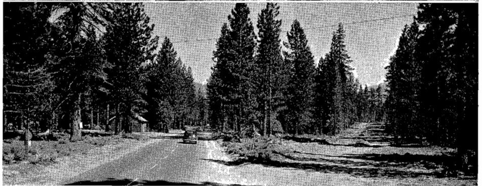
Construction is under way for the improvement of U. S. 50 from the foot of Meyers Grade to Mays, a cooperative project of the U. S. Forest Service, U. S. Bureau of Public Roads, and State Division of Highways. Lower photo shows existing highway on left, realignment on right
