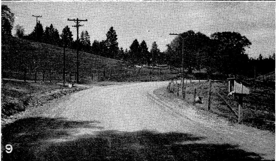
7—New six-inch base material with penetration oil treatment. Placed November, 1948. Appearance in April, 1949. 8—Closeup of same section as above. 9—New six-inch base material which went through winter without oil treatment. Appearance in April, 1949
