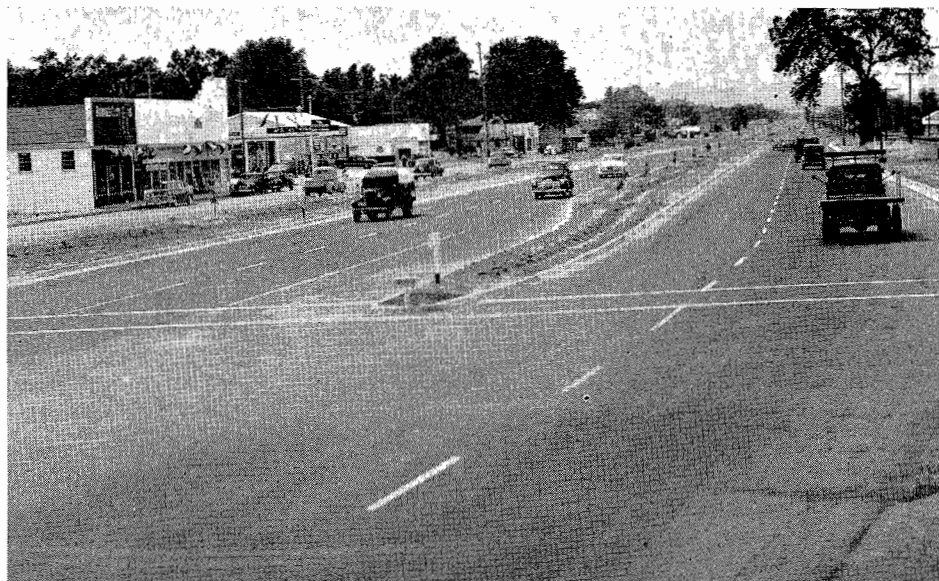
Completed section of new freeway in Anderson. Frontage road on left
