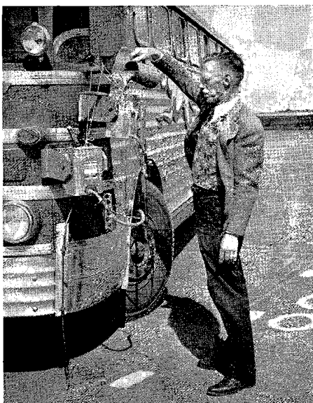
Apparatus used for making trace on pavement (Front overhang of bus)
