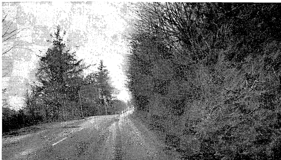
The foreground shows result of mowing brush on slope. Brush in background is typical before-mowing scene
