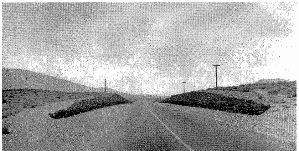
UPPER—Wind erosion affects both the sandy cut slope and the traveled way. (Near Carmel, Monterey County.) LOWER—Rock placed by hand on sandy cut slope face, controls wind erosion in desert areas. (Near Little Lake, Inyo County)
