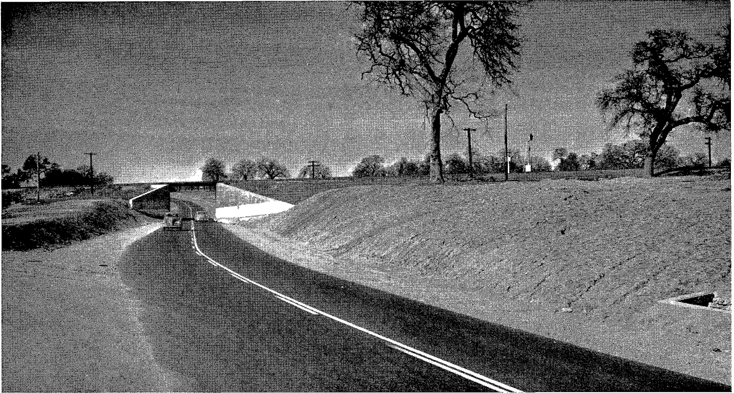
Widening of U. S. 99E gives sight distance at Andora subway one mile north of Roseville, previously a traffic hazard
