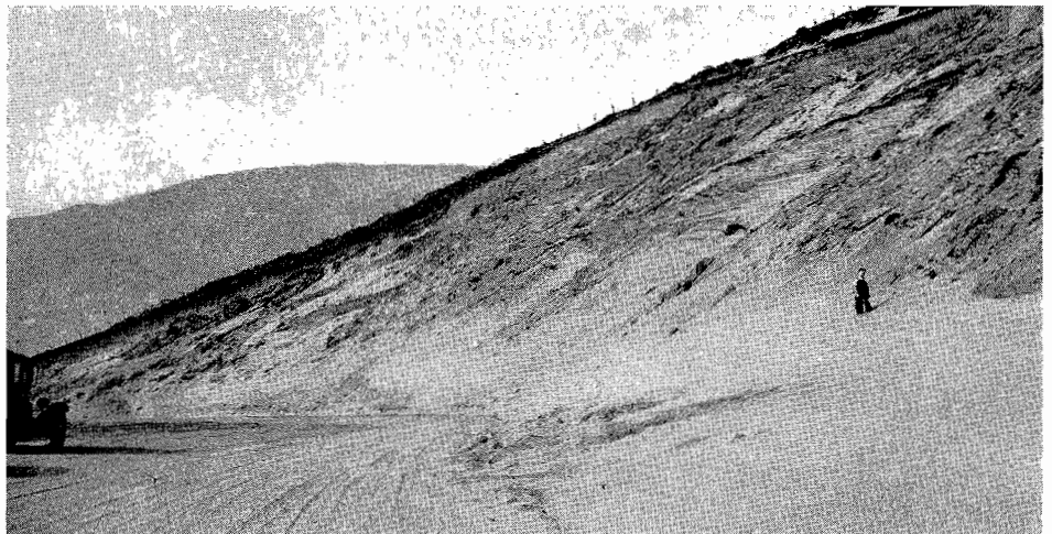
UPPER—Wind erosion affects both the sandy cut slope and the traveled way. (Near Carmel, Monterey County.) LOWER—Rock placed by hand on sandy cut slope face, controls wind erosion in desert areas. (Near Little Lake, Inyo County)
