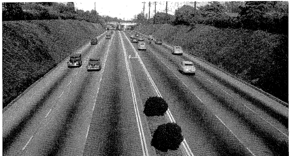
UPPER—Type A stabilization during construction. Topsoil is cast on by dragline. (Seventh Street Interchange, Santa Ana Freeway, Los Angeles.) LOWER—Established ground cover planting on Type A Stabilized 1:1 cut slopes. (Arroyo Seco Parkway, Los Angeles to Pasadena)
