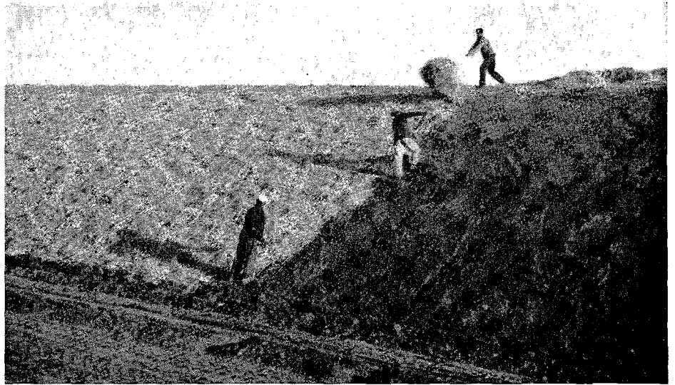
Spreading straw on newly topsoiled slope
