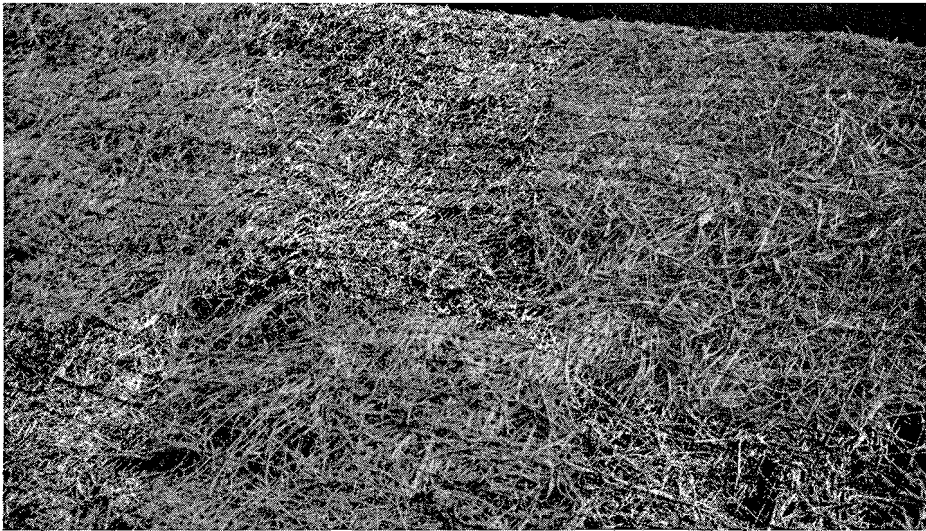
Type B stabilization treatment ready for ground cover planting
