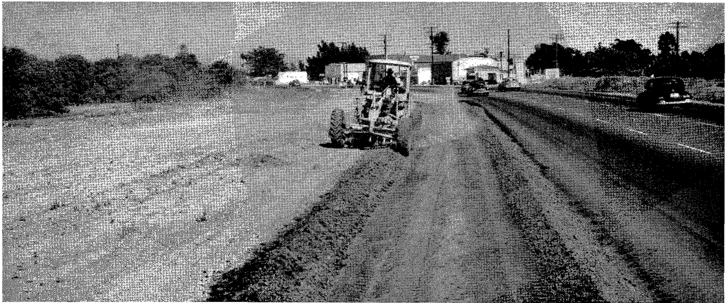
Looking southeasterly showing construction under way near the City of Anaheim
