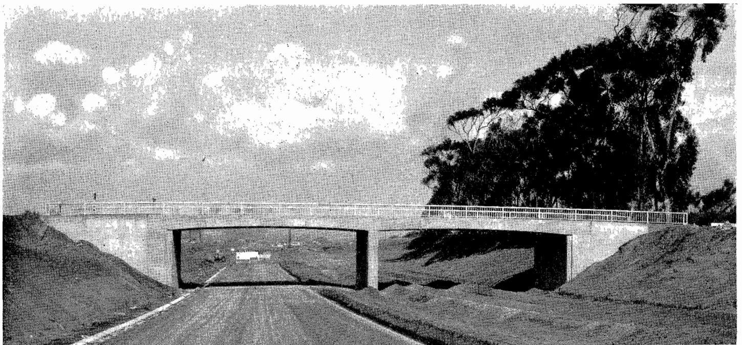
This is the E Street freeway overcrossing in Chula Vista
