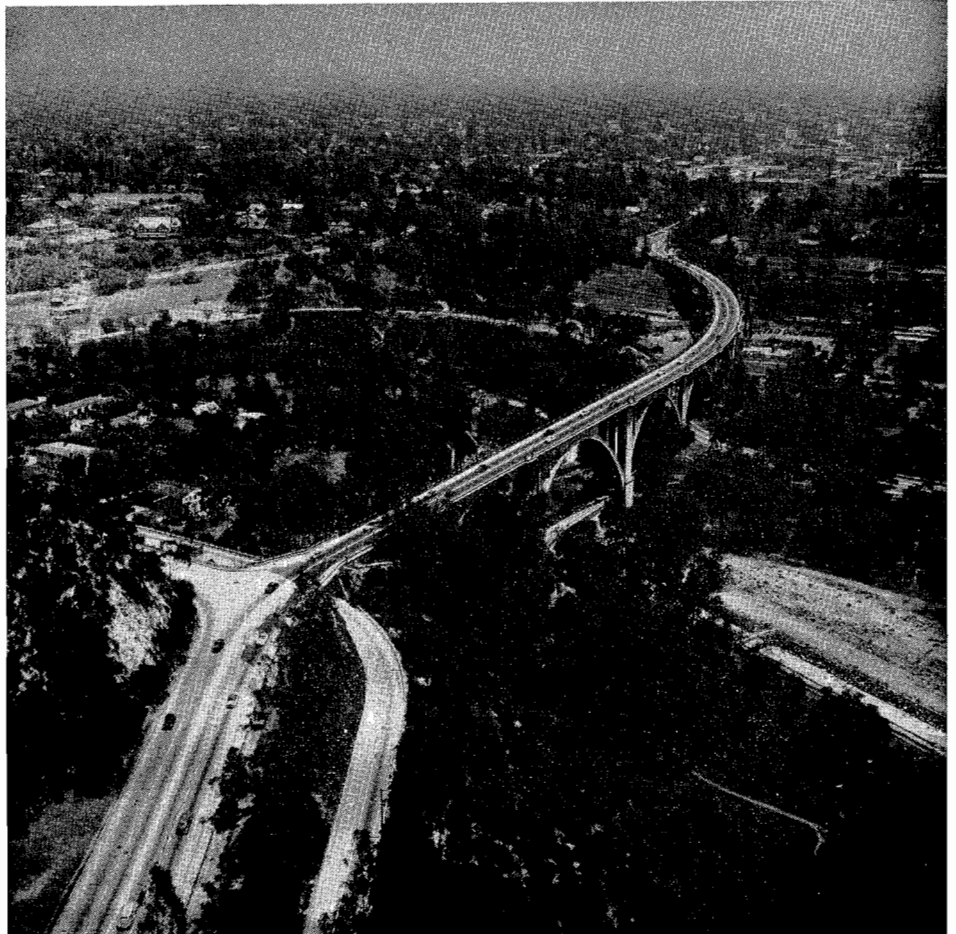
PHOTO 1—Old Colorado Bridge looking east toward Pasadena, showing main topographic features of the site of the new bridge
