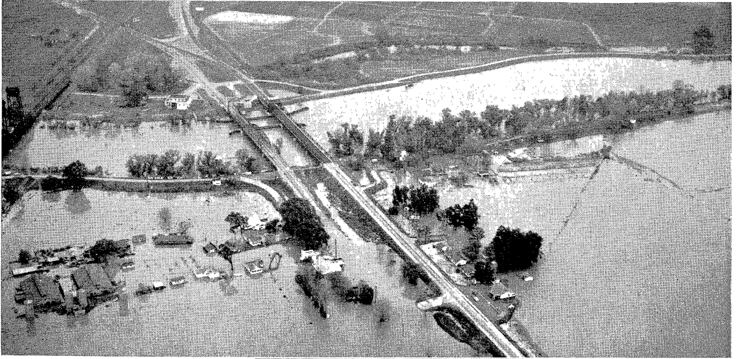
UPPER—Floodwaters destroyed the Paradise Cut overflow bridge on U. S. 50 west of Mossdale. LOWER—Aerial closeup of the bridge which was undermined and collapsed. Westbound traffic lanes are under water
