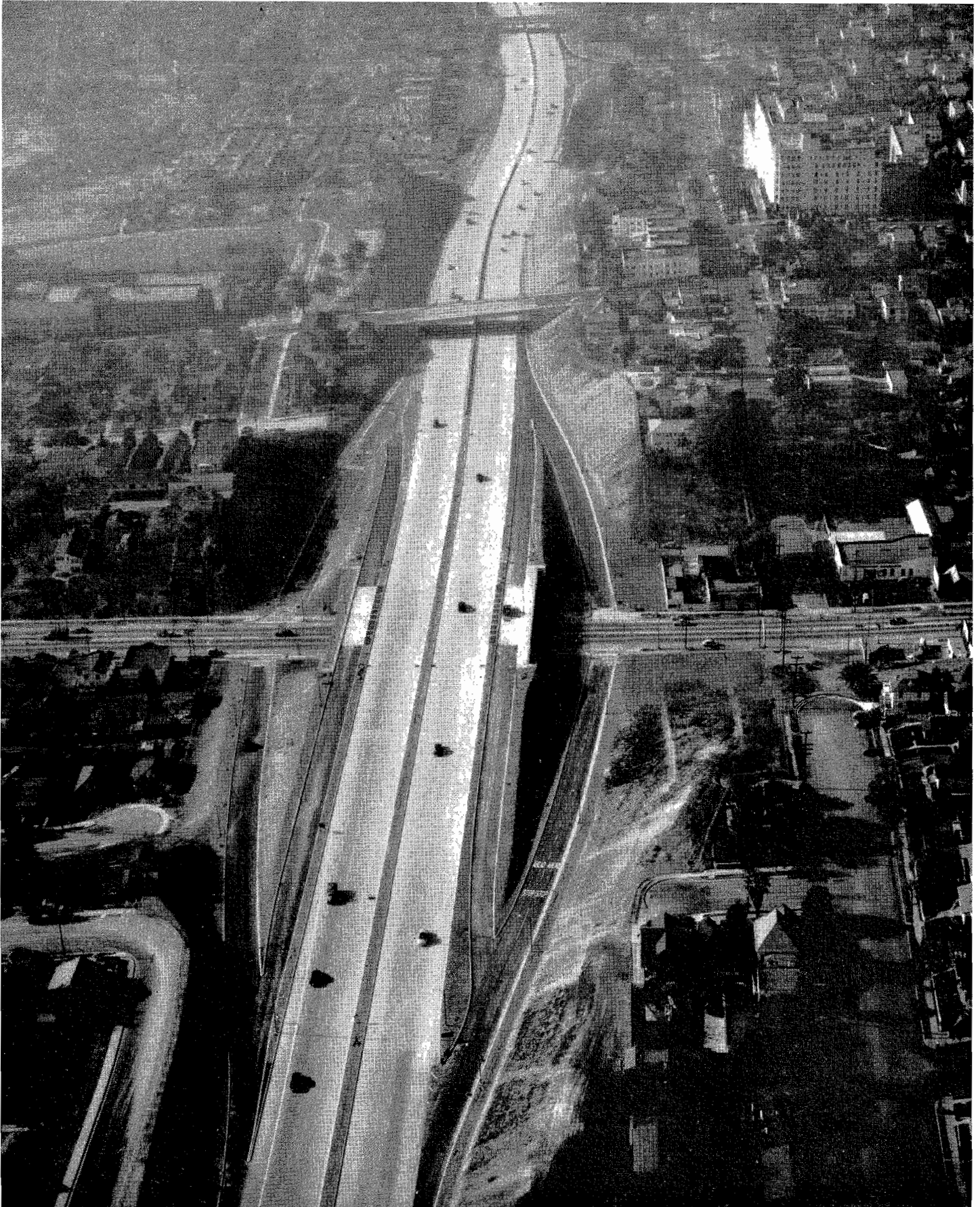
Looking westerly over Alvarado Street interchange structure. In center is Rosemont Avenue bridge crossing with Benton Way bridge crossing in extreme background
