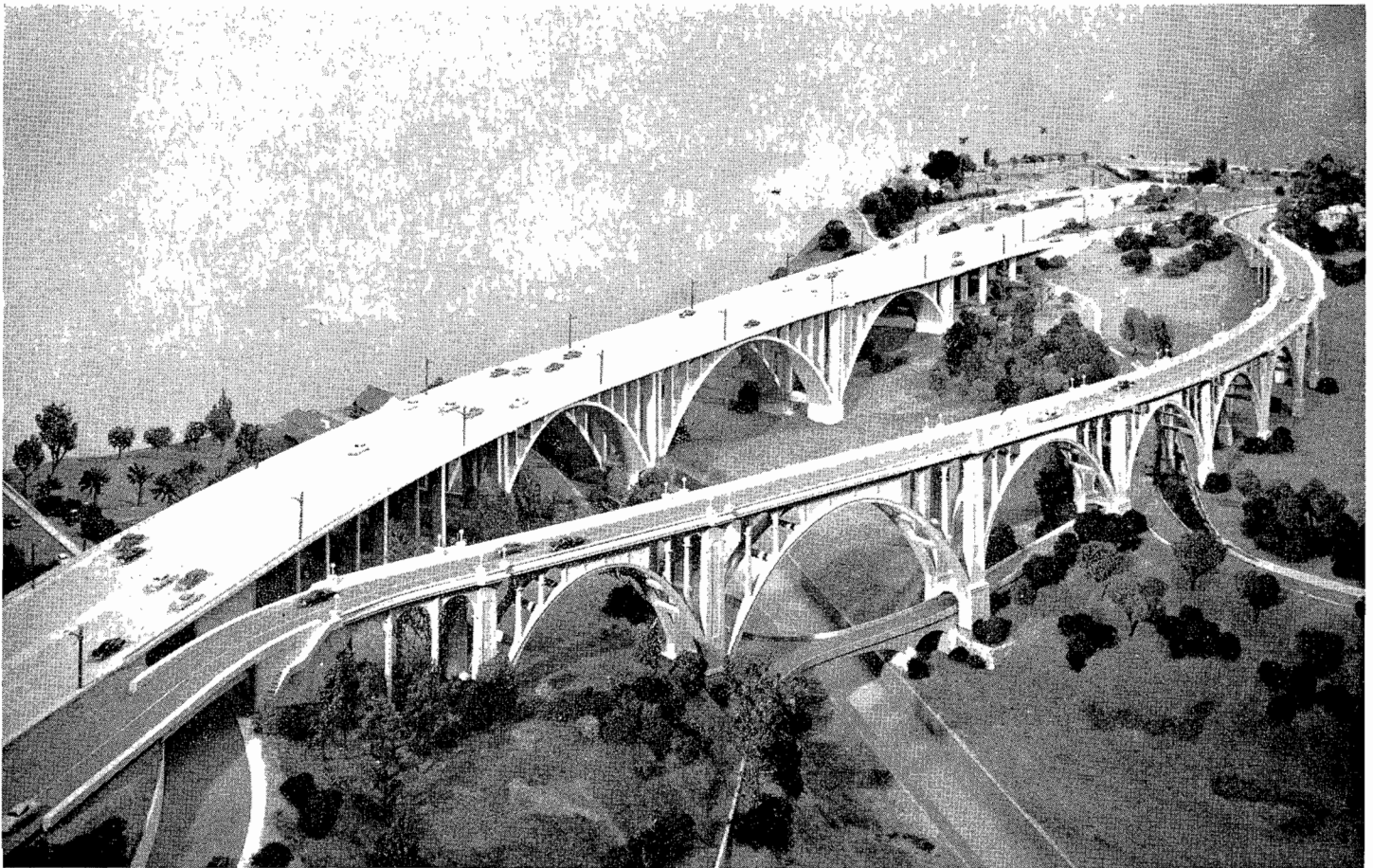
PHOTO 3—This is a photograph of a model of the new Colorado Street Bridge, showing the existing bridge on the right
