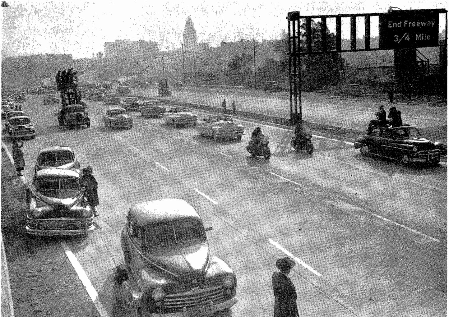
Official cars leading traffic over newly completed Hollywood Freeway following dedicatory ceremonies
