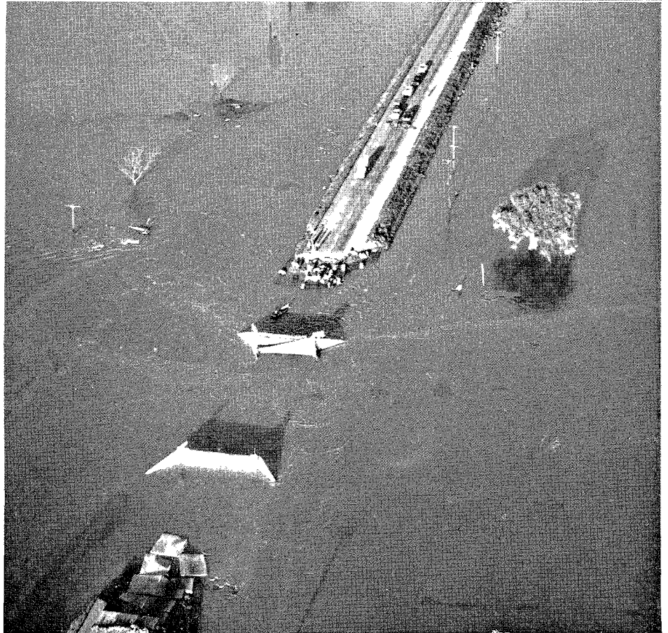
UPPER—Floodwaters destroyed the Paradise Cut overflow bridge on U. S. 50 west of Mossdale. LOWER—Aerial closeup of the bridge which was undermined and collapsed. Westbound traffic lanes are under water
