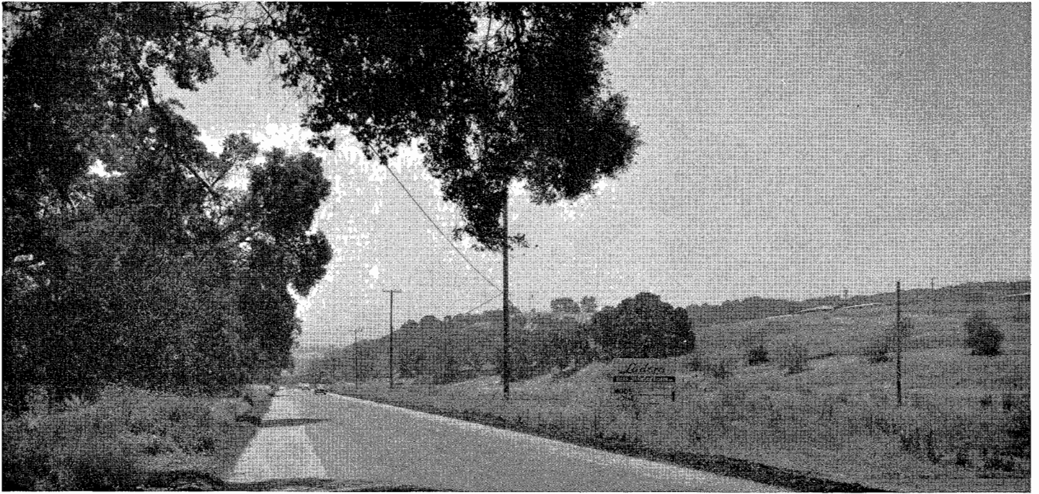
Another view of new Alpine Road in San Mateo County looking west
