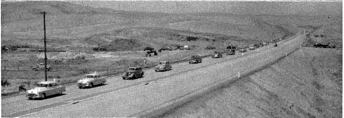
UPPER—Scene at dedication at Port Chicago end of freeway showing separation structure. Eastbound traffic uses lanes on left, westbound traffic elevated lanes on right. CENTER—Caravan goes over new highway. BOTTOM—New highway looking west.
