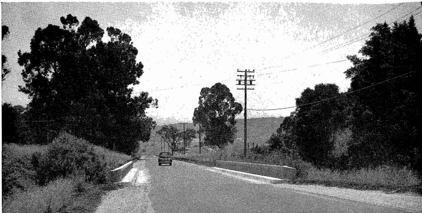
Alpine Road looking west across new bridge
