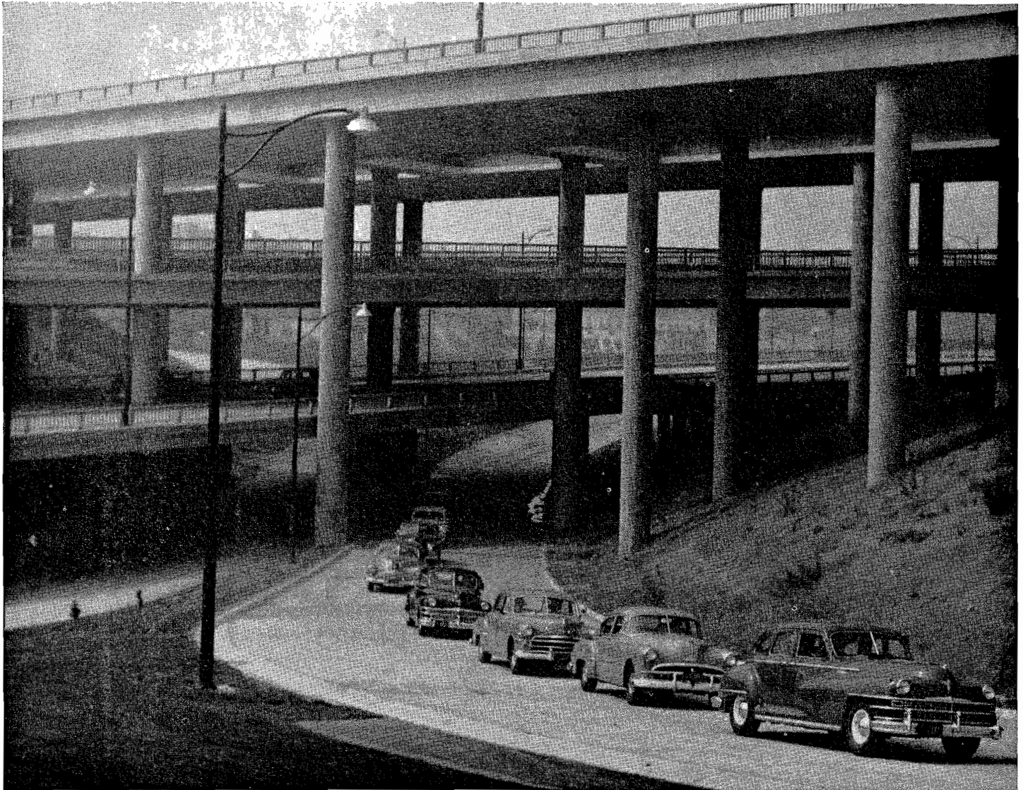
Autos passing under four-level grade separation structure using the lowest level for first time
