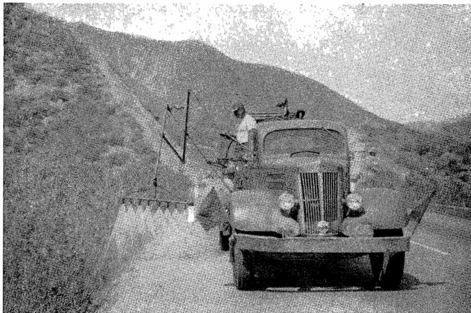
City Creek highway. Second seasonal application at top of fill slope.
