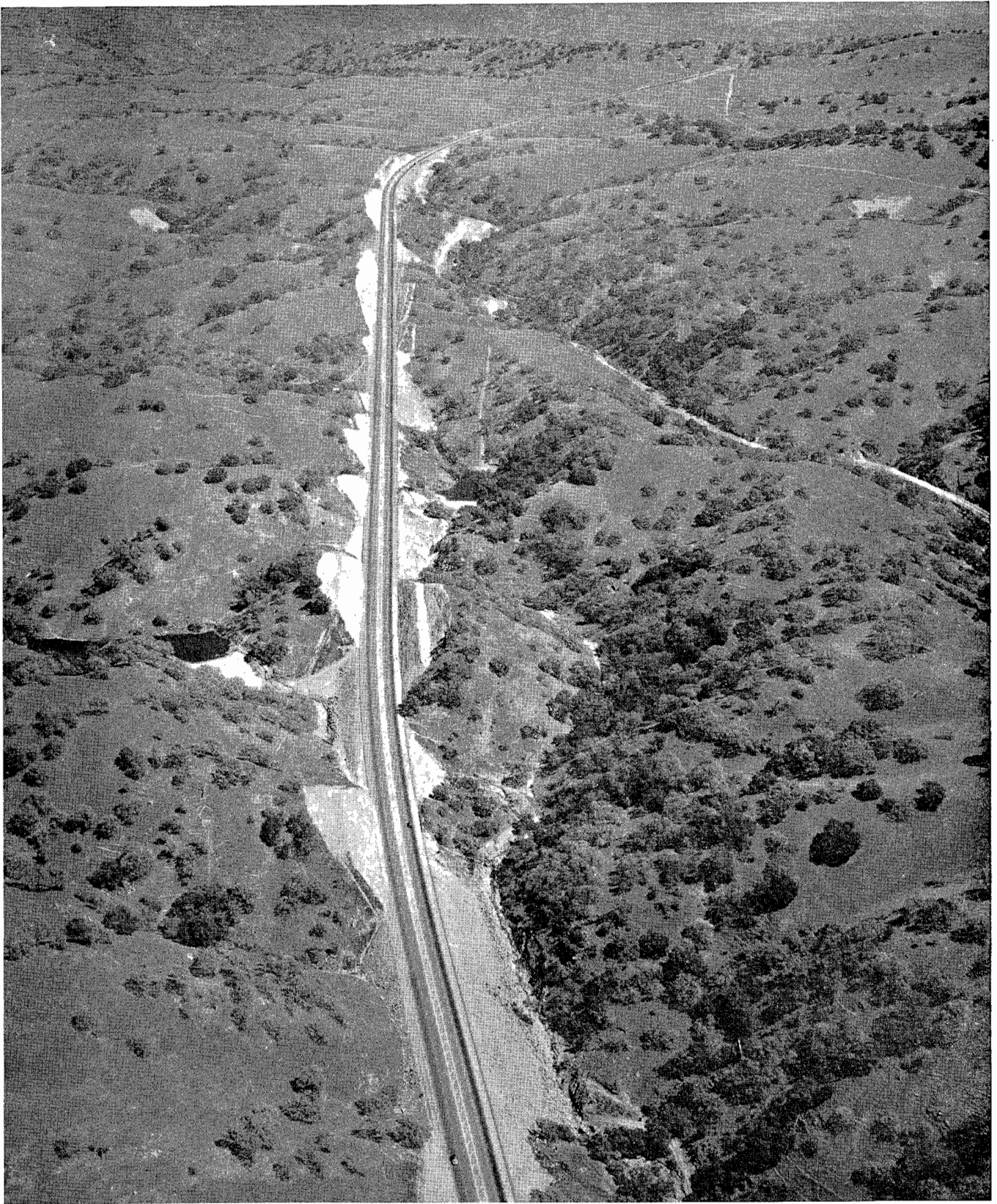
This aerial photograph shows benching of cuts and embankment toe protection on new highway
