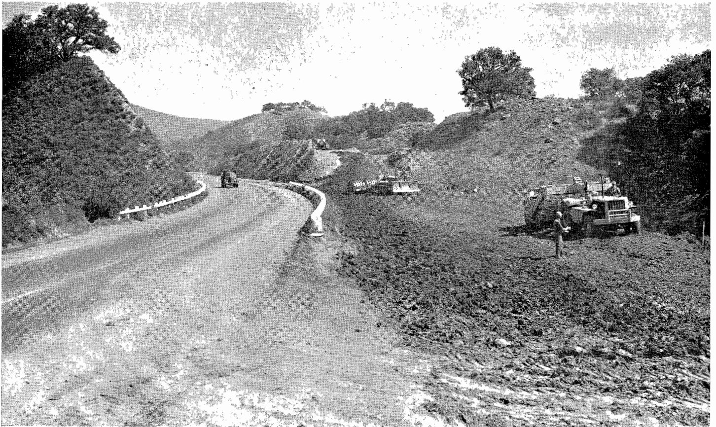
UPPER—Nojoqui Grade showing inadequacy of existing roadway. The new four-lane highway which will be developed from existing two-lane highway will eliminate hazardous conditions on this grade. LOWER—Construction operations in progress on Nojoqui Grade just south of the summit.
