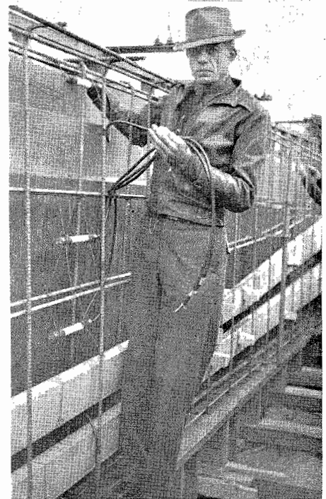
ABOVE—Interior of girder form, showing sheet metal cable enclosures, before sides of form brought together. RIGHT—Resident Engineer Jack Sylvester holding leads to Carlson electrical resistance strain gages. Note sheet metal enclosures built around wire cable groups in lower part of beam to form tunnel-like cavities.
