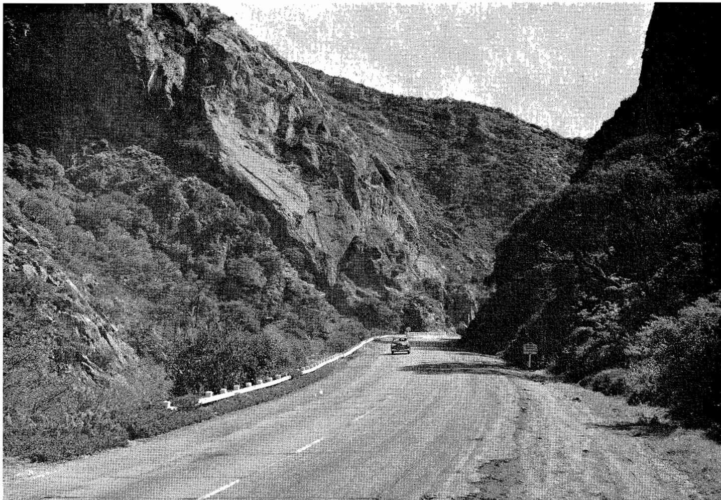
View of Gaviota Gorge looking south. The natural beauty will be maintained by boring through the massive sandstone ledge and minimizing the removal of surface rock.
