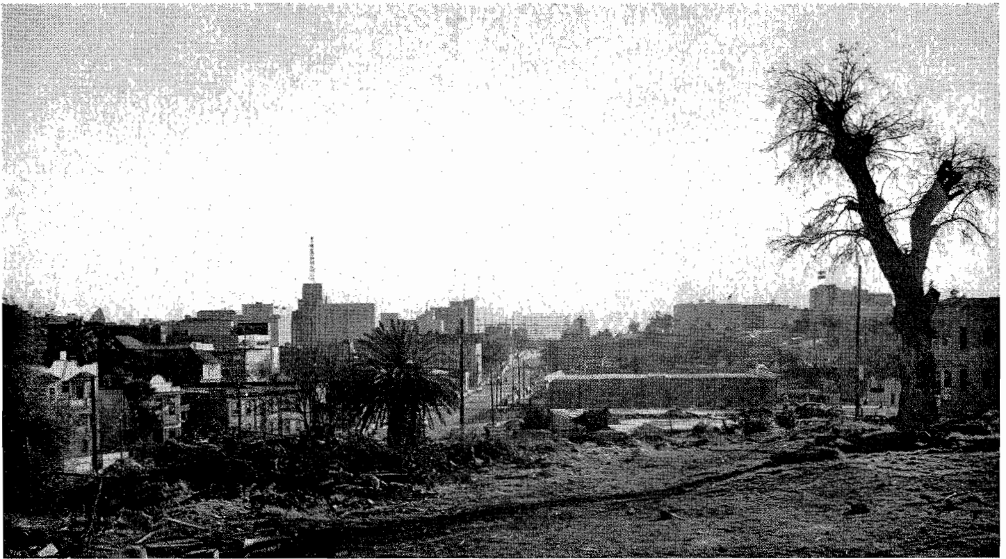
View from Temple Street looking southerly along cleared right of way for Harbor Freeway showing in middle foreground completed First Street and Second Street underpass grade separation bridges. The city street to the left is Fremont Avenue and in the background is the steel framework of the Statler Center Hotel.
