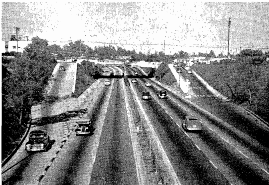
Example of ascending outlet on Arroyo Seco Parkway between Los Angeles and Pasadena
