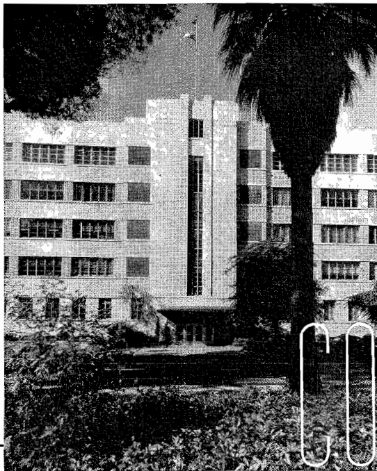
Public Works Building Twelfth and N Streets Sacramento
