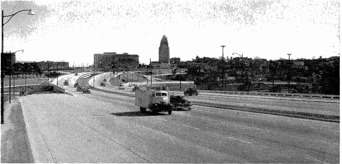
Portland cement concrete pavement on the Hollywood Freeway in Los Angeles
