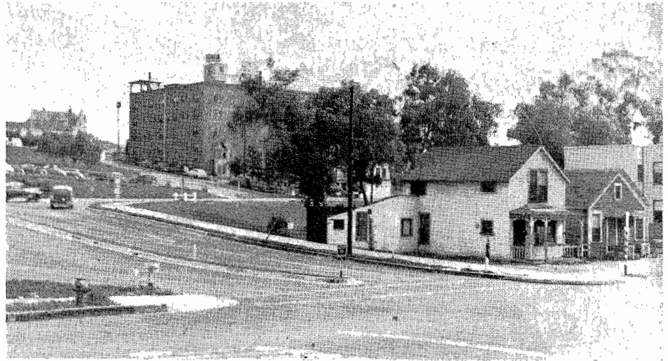
Southeast corner of 10th and Ash Streets in San Diego before construction. Stucco apartment building visible at extreme right. Ash Street approach to Cabrillo Freeway in left foreground.
