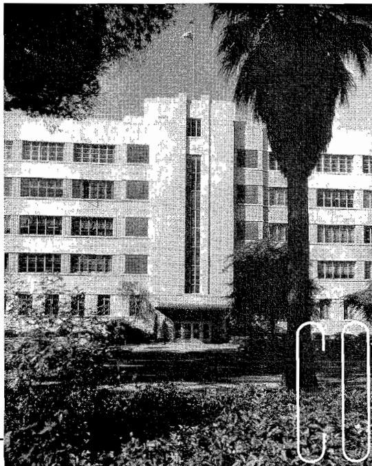
Public Works Building Twelfth and N Streets Sacramento
