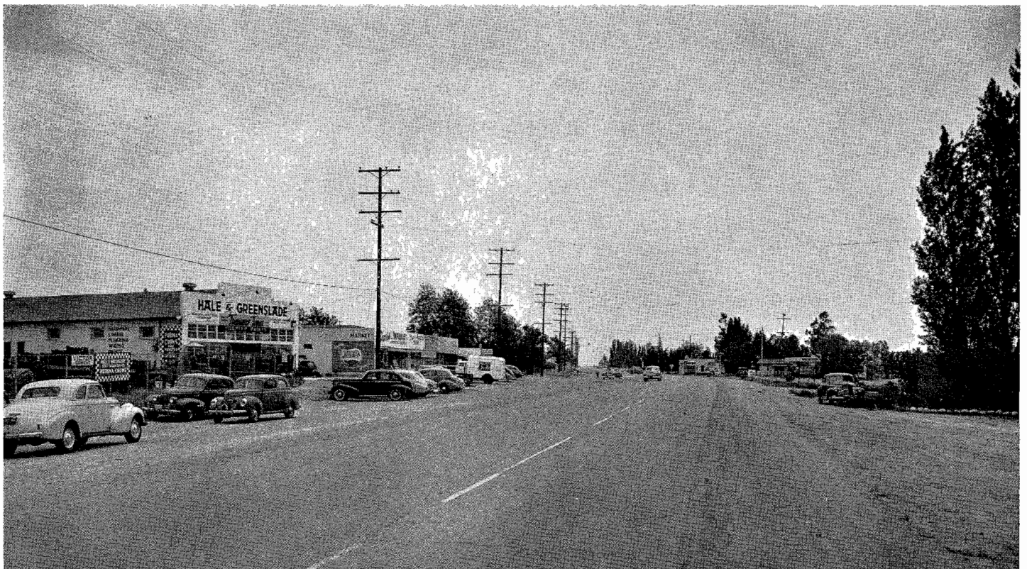
This view is looking east through Calimesa after highway modernization
