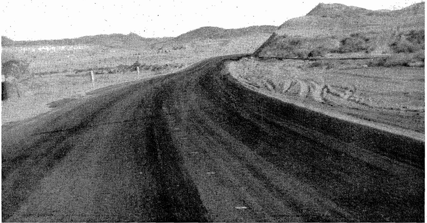
Roadmixed surfacing near Salt Wells in San Bernardino County
