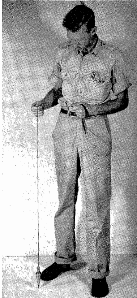
Chainman using plumb bob to transfer measurement from tape to point on ground
