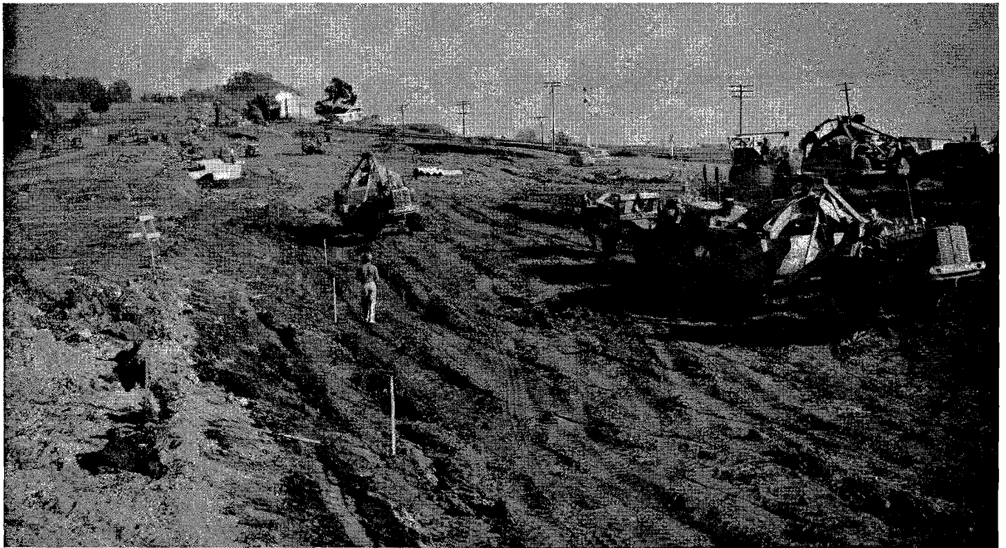
Heavy equipment engaged in construction at Summerland
