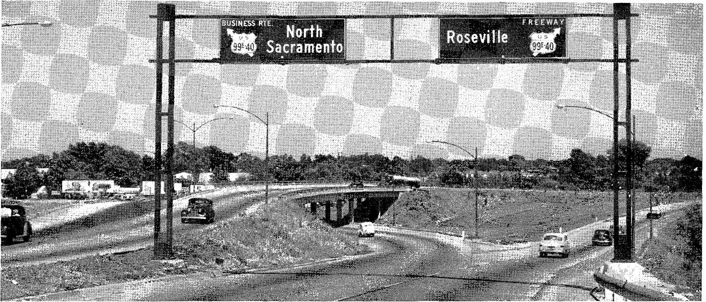
Overhead sign bridge on North Sacramento Freeway
