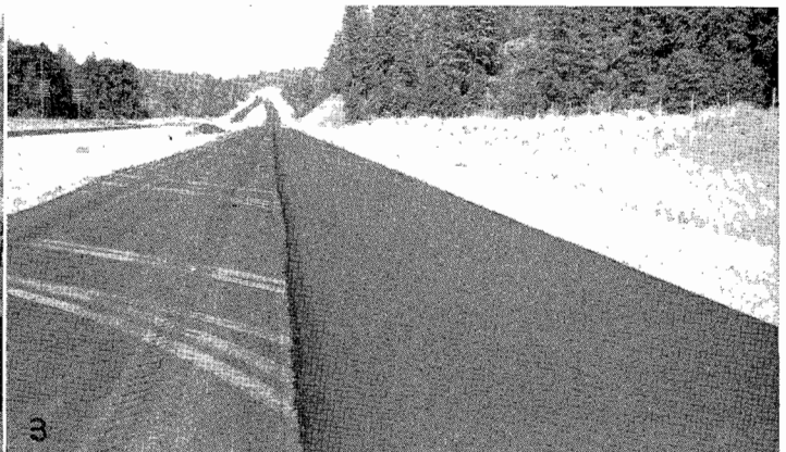
PHOTO 2—General view of plant (rubber added at top platform). PHOTO 3—Experimental section on right after rolling (leveling course at left). PHOTO 4—Placing surface with Barber-Greene. PHOTO 5—Close-up of bituminous surface with rubber added. (Pictures taken August 21, 1950.)
