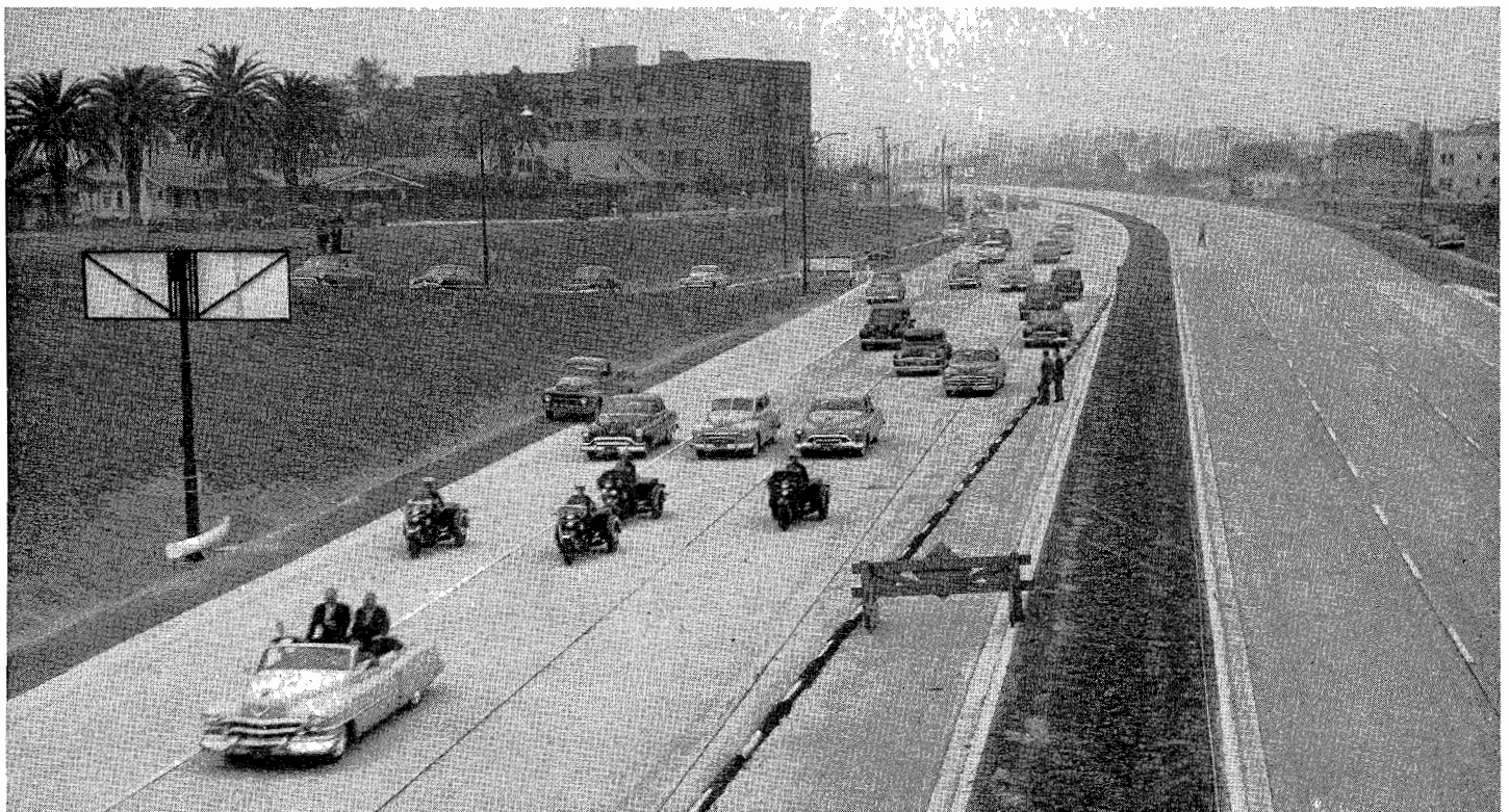
View of completed Hollywood Freeway looking southerly from Santa Monica Boulevard, showing caravan using northbound roadway
