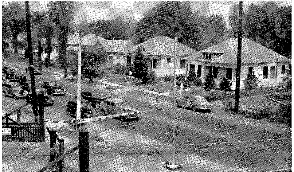
Eastbound Fifth Street traffic blocked. Surveys showed these gates were down almost one-third of the time before overhead was built.
