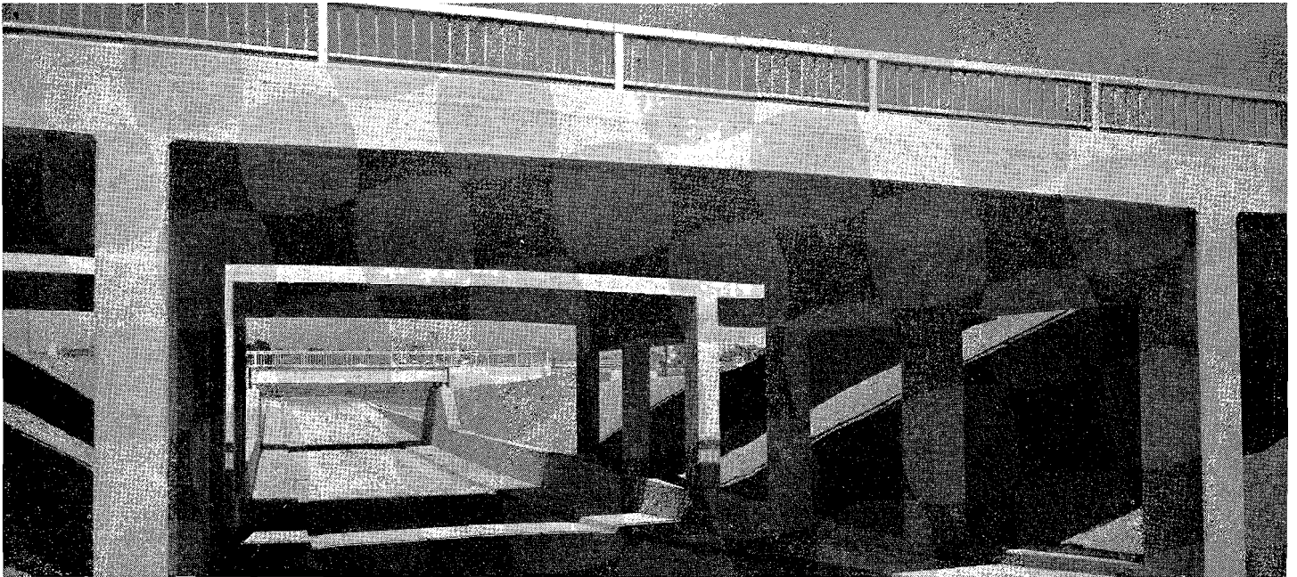
This is the completed 24th Street bridge
