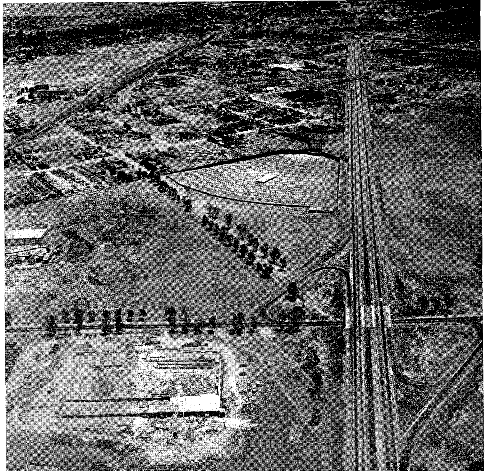
Aerial photograph looking northeasterly along the North Sacramento Freeway, shows the $1,600,000 Continental Baking Plant under construction in the left foreground
