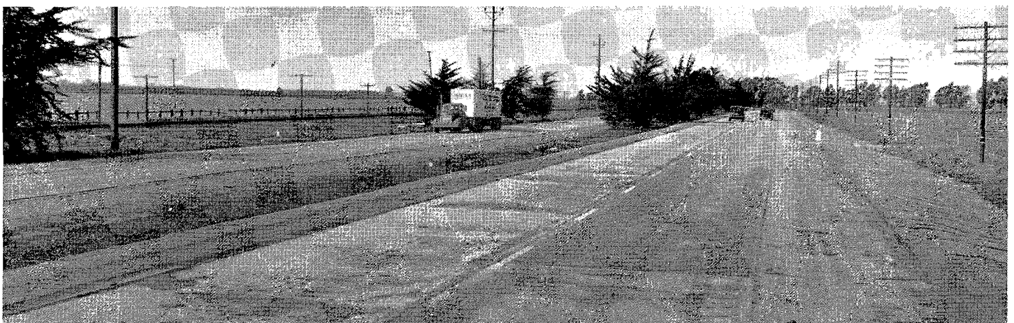
Completed section of U. S. 101 between Chualar and Spence Underpass
