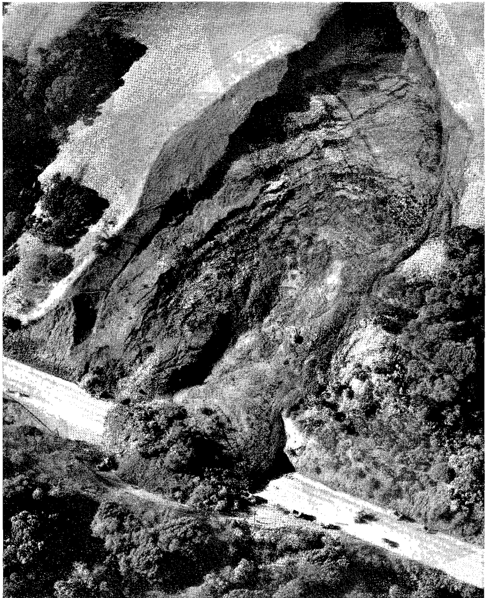
Aerial photograph of Orinda Slide graphically shows its size. San Francisco Examiner photo.
