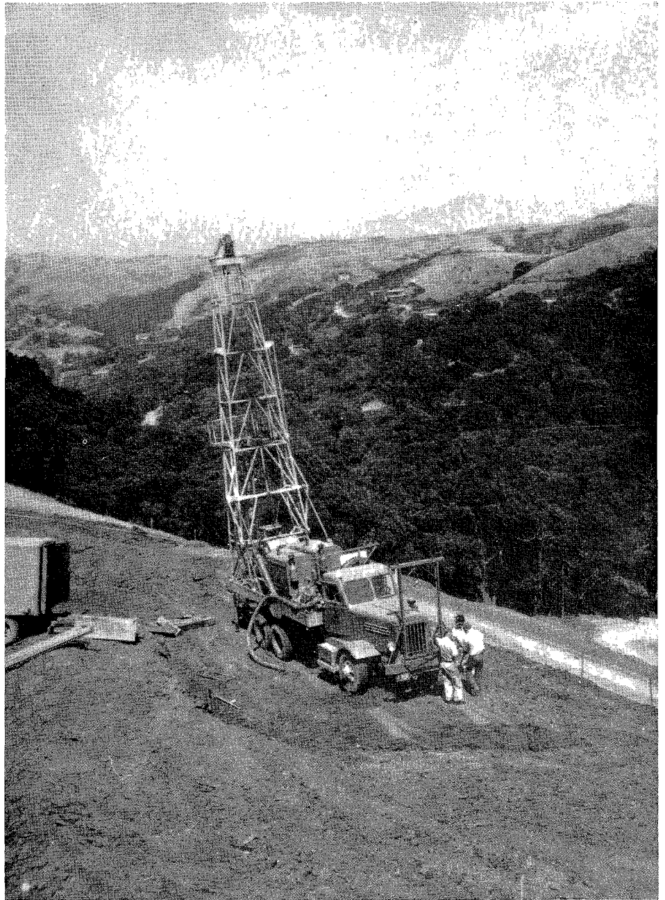
Vertical drilling equipment of Materials and Research Department
