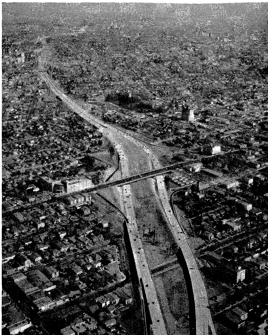
Looking easterly along Hollywood Freeway, taken from above Melrose Avenue, showing in foreground the split between roadways to accommodate future connections with proposed Santa Monica Freeway
