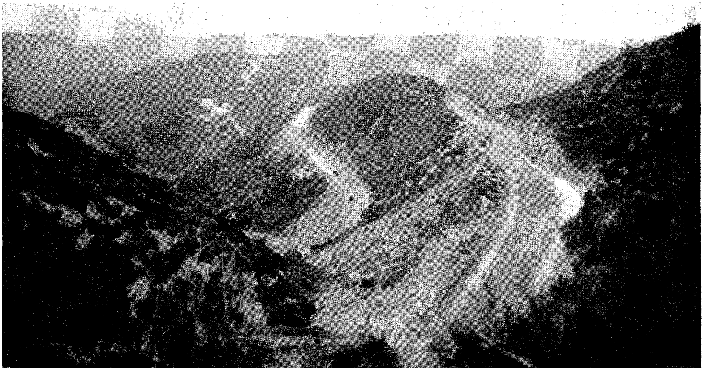
Fremont Pass, a slot through the mountains, 15 feet wide and 60 feet deep, constructed in stages by hand methods during pioneer days, was in service until 1910, at that time the most direct route from Los Angeles to the north
