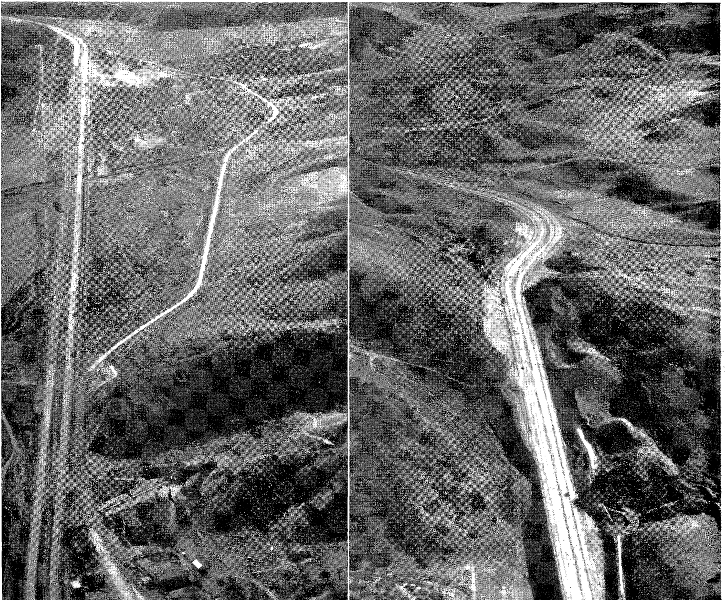
LEFT—Looking southerly along completed section of Ridge Route. Lebec is shown in foreground. Tejon Summit is just off upper left corner of photograph. RIGHT—Looking southerly along completed section of Ridge Route southerly of Gorman.
