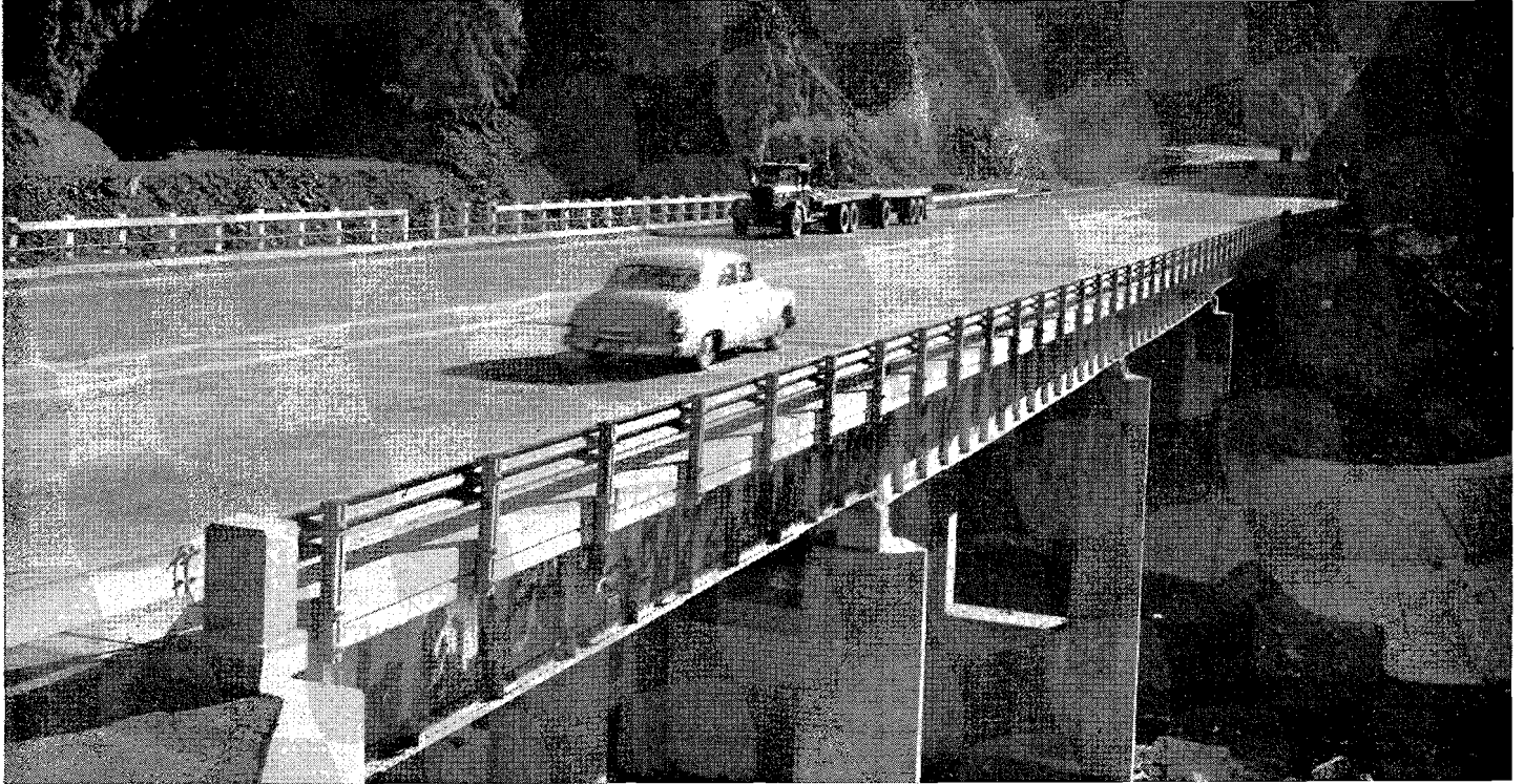
UPPER—Aerial view, looking northerly, showing completed Ridge Route in Piru Gorge with Pyramid Cut in left foreground. LOWER—Looking southerly, showing completed Ridge Route with Piru Creek Bridge in the foreground.
