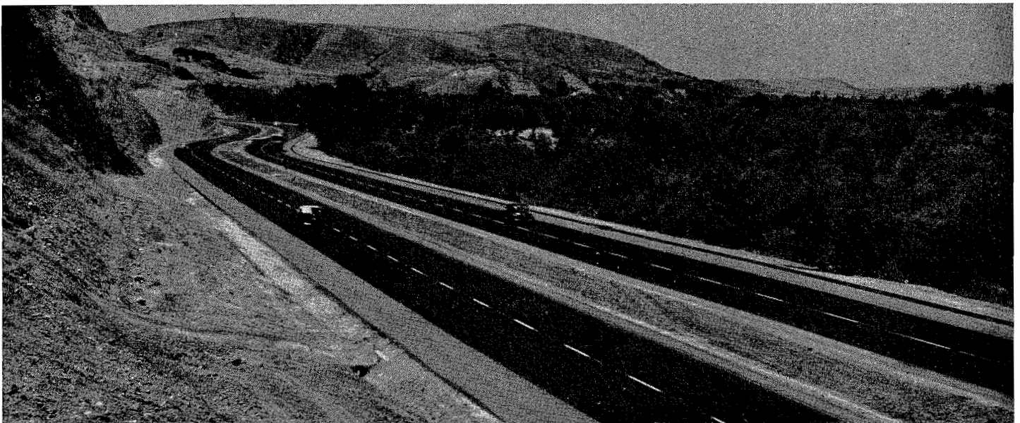
Completed construction of four-lane, limited access freeway on Santa Ana Canyon Road in Orange County
