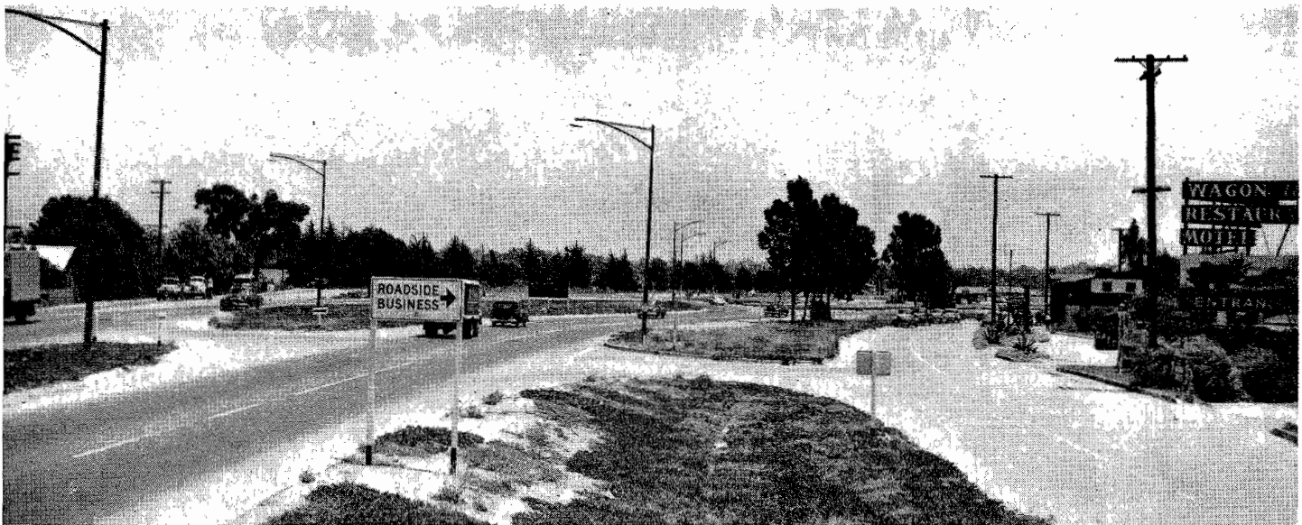
Looking southeasterly at El Rio channelized intersection between U. S. 101 and U. S. 101 Alt.
