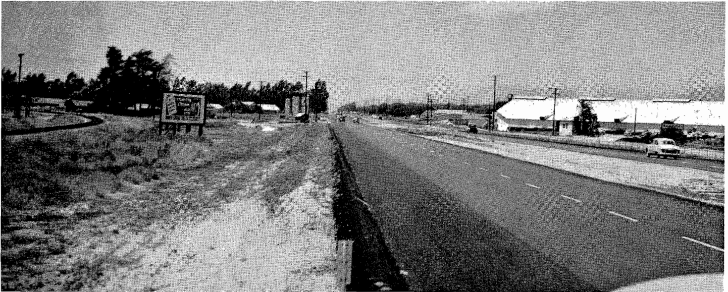
Looking northwesterly toward Ventura along completed freeway. Main line track of Southern Pacific in relocated position at extreme left.
