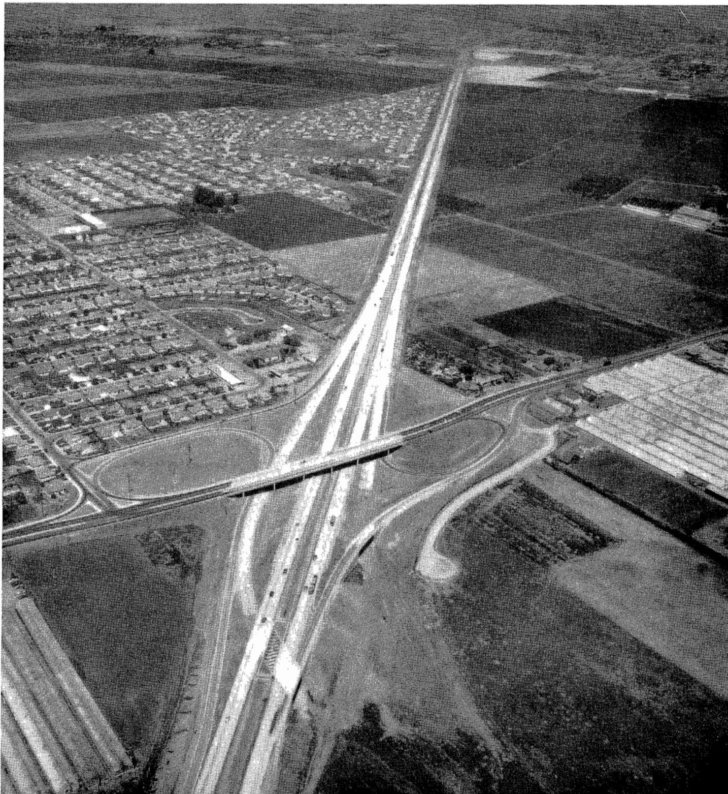
Eastshore Freeway, looking north, showing Washington Avenue interchange. Recent housing development shown in left background. Underpass in foreground is future on-ramp from State Route 228. Frontage road in foreground provides for access to future residential area.
