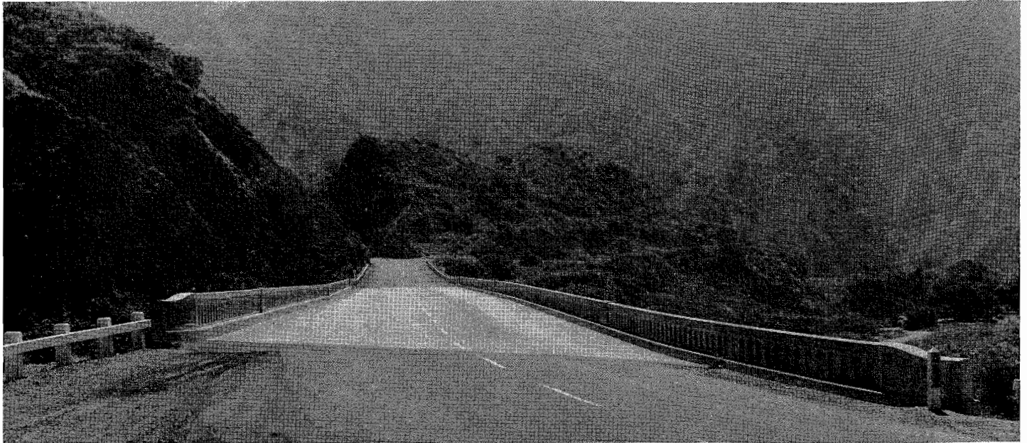
Bridge 3—Bridge on San Gabriel Canyon Road (F. A. S. Route 825) over North Fork of San Gabriel River
