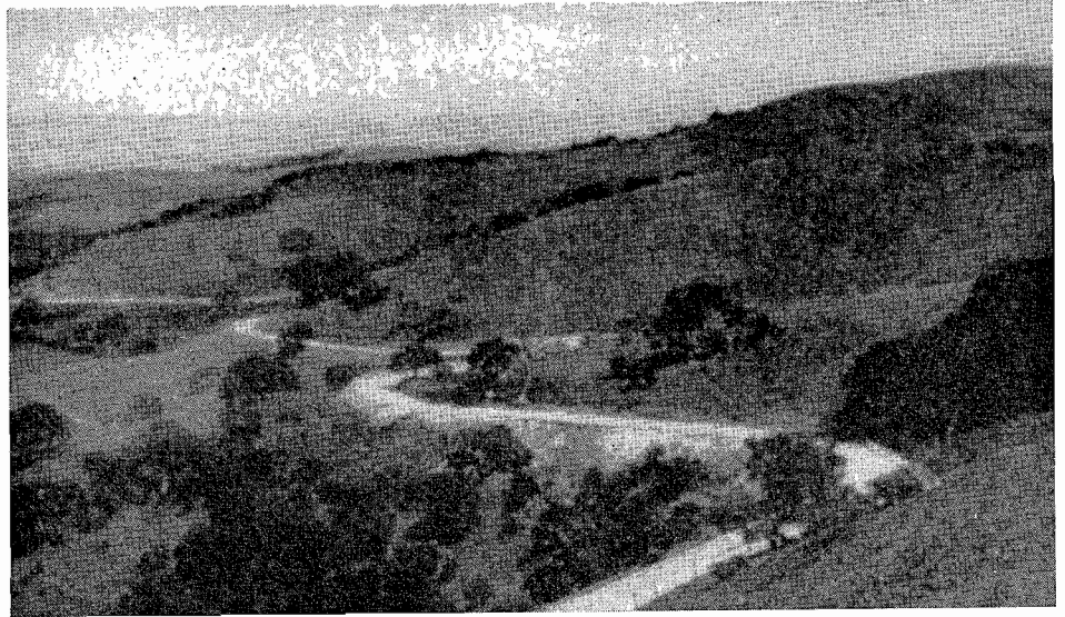
State highway in San Benito County, typical of early highways made possible by first bond issue
