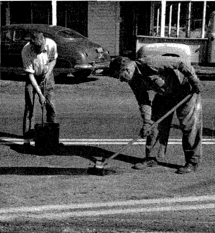
UPPER LEFT—John Perry explains the features of the casting carriage, operated by Ed Pirro, to the author, on right. UPPER RIGHT—Proportioning and mixing machine mounted on truck. Hose to casting carriage comes out from below truck frame directly below mixing chamber. LOWER LEFT—Applying cementing agent to pavement immediately ahead of casting. LOWER RIGHT—Casting carriage in operation. Yoke handle raises nozzle when pump is stopped.
