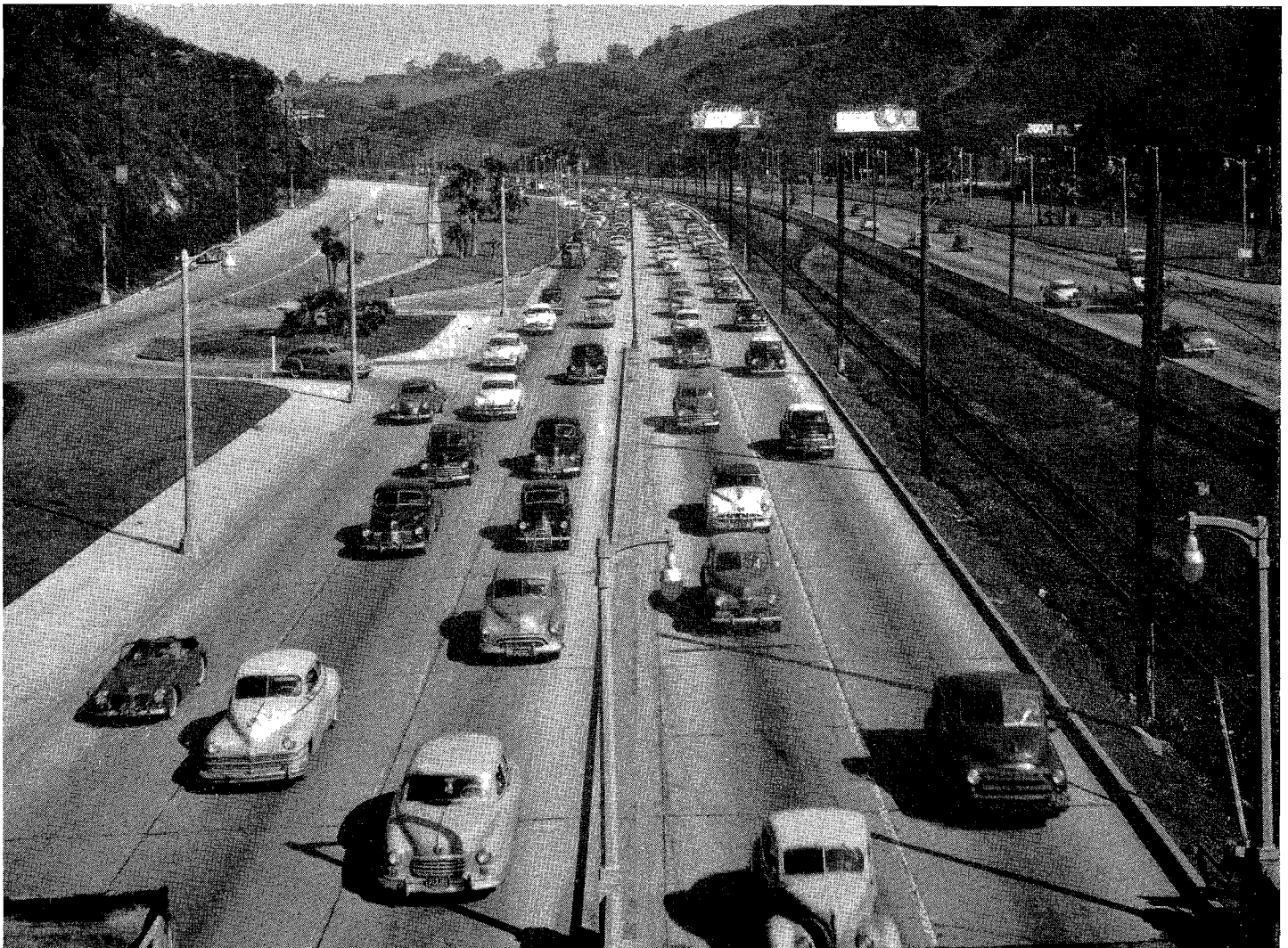
Looking northwesterly along portion of Hollywood Freeway through Cahuenga Pass from Pilgrimage Bridge. The oncoming traffic is inbound, with the two lanes to right headed for Cahuenga Boulevard and the two lanes to left headed for Highland Avenue. Traffic is over 105,000 vehicles per 24 hours.
