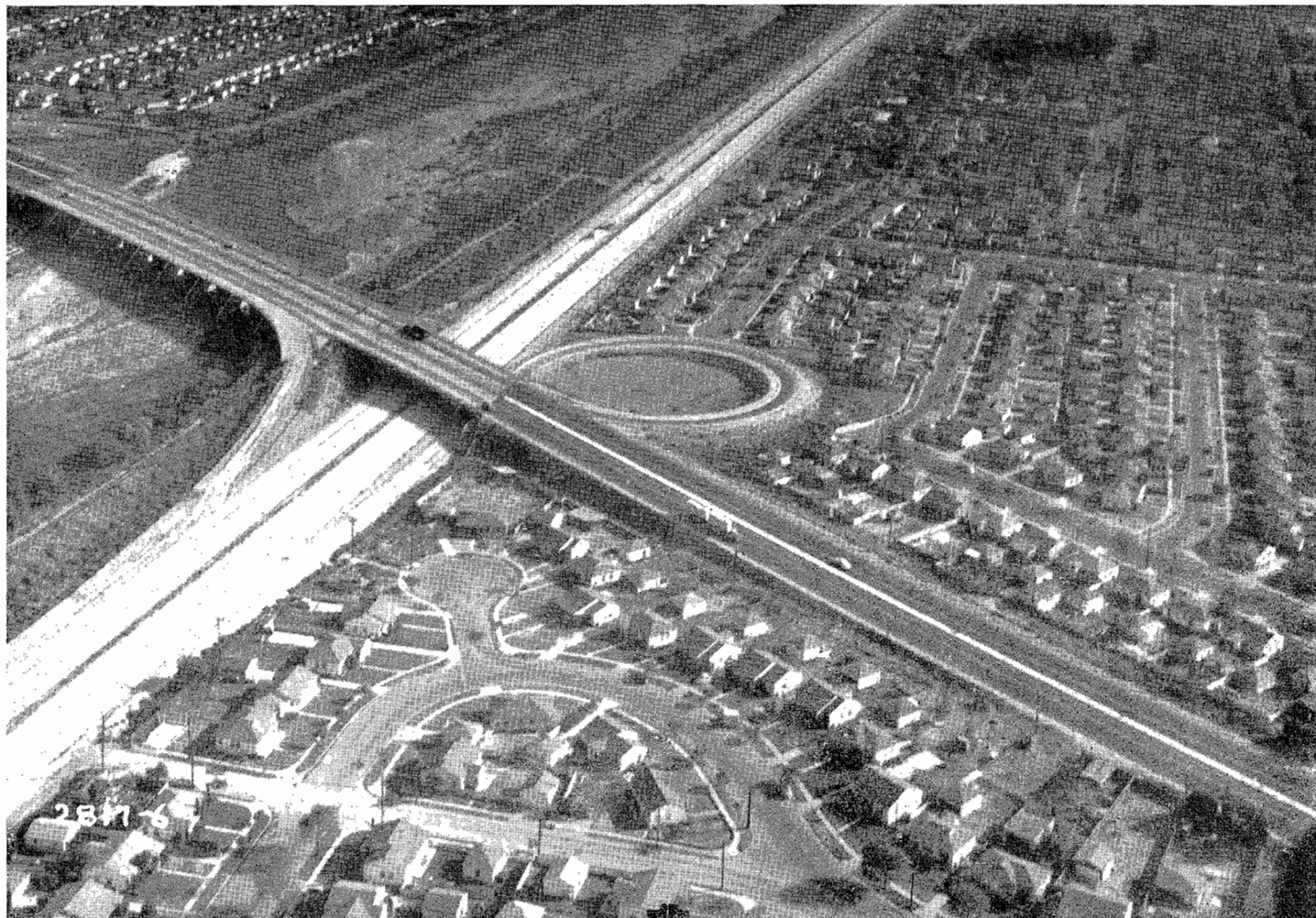
Looking southeasterly along Long Beach Freeway, showing grade separation and traffic interchange facilities at Belhart Avenue Crossing
