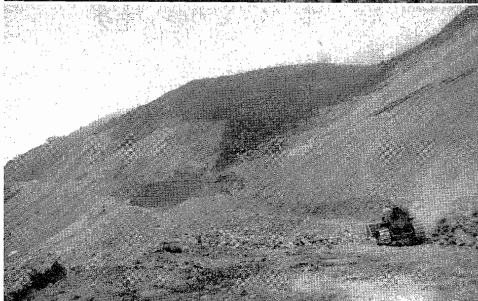
UPPER—General view of slide area during unloading operations. LOWER—Bulldozers re-establishing road at base of slide.
