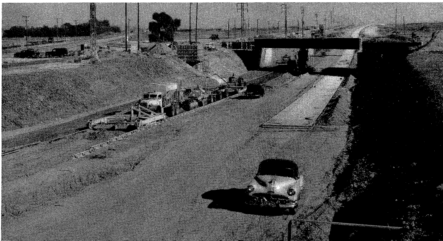
Southern Pacific spur track overcrossing, showing freeway paving operations in progress
