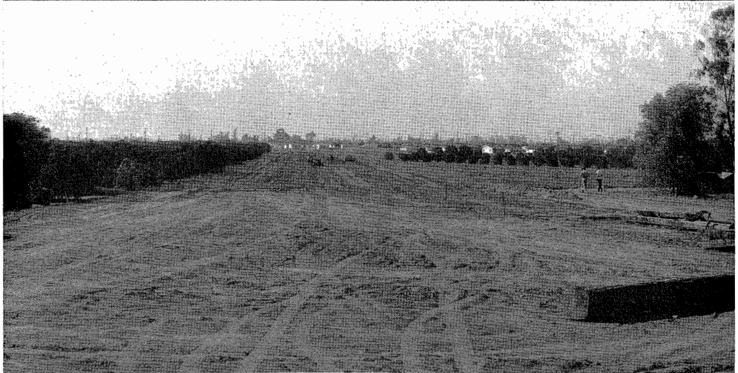
UPPER—Looking northwesterly along "Norwalk Diagonal" section of Santa Ana Freeway which will follow just to right of line of electric power poles. The channelized and signalized intersection in foreground of Firestone Boulevard with Rosecrans Avenue will be replaced, creating grade separation and traffic interchange system as indicated in lower right hand corner of perspective drawing on opposite page. LOWER—Grading operations on "Norwalk Diagonal" northwesterly from crossing with San Gabriel River.
