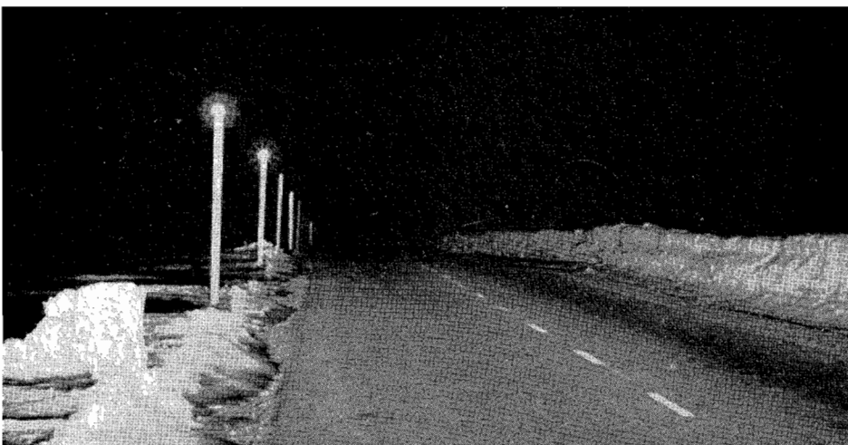
Standard three-inch reflectors attached to snow poles
