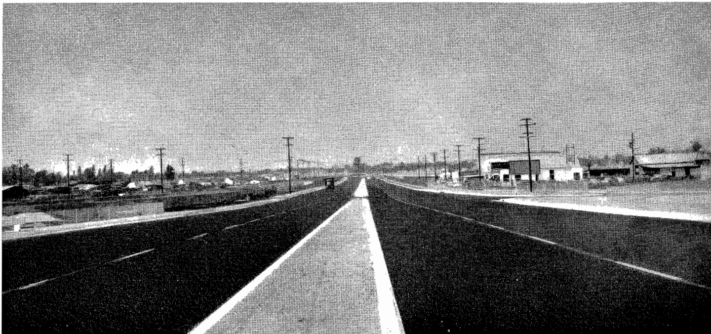
This section of four-lane divided highway has a bituminous plant-mixed surfacing over a cement-treated base. Recent construction on Rosemead Boulevard in Los Angeles.
