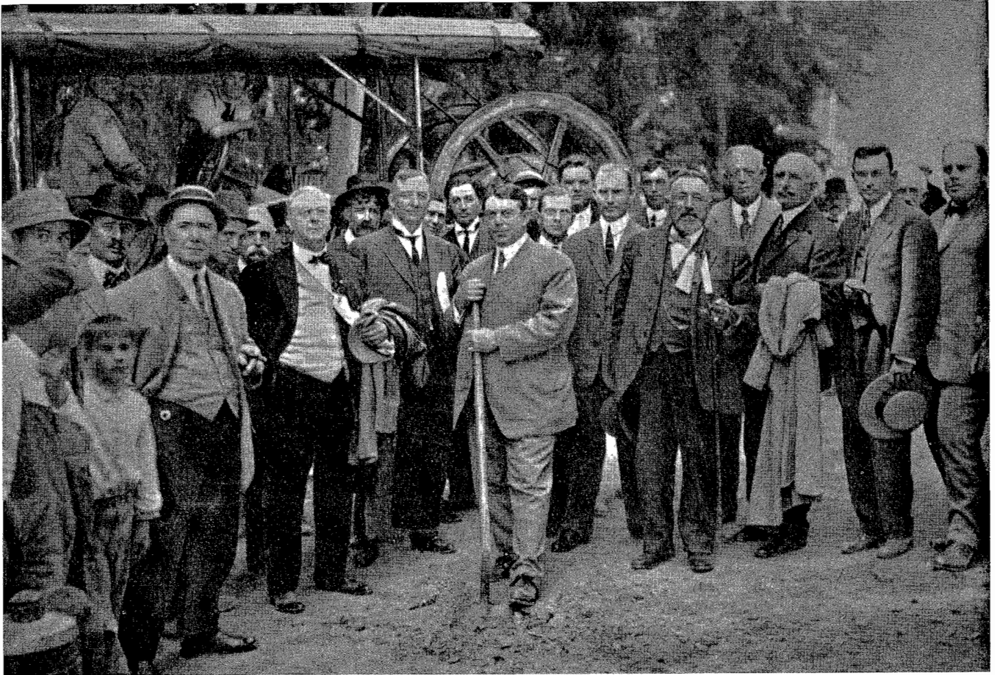
Start of actual construction on State Highway Contract No. 1 was made in San Mateo County on August 7, 1912. In the group are Chairman Towne of the Highway Commission with shovel; W. J. Martin, South San Francisco; L. E. Aubury, Ex-State Mineralogist; Judge P. E. Lamb, Burlingame; Ex-County Recorder of San Mateo County, H. O. Heiner; Dr. F. C. McGovern; A. E. Ritchie, Fred Cunningham and Supervisor W. H. Brown, San Mateo County.
