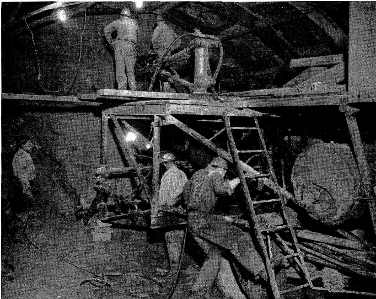
Jumbo in operation showing general position of drills at face
