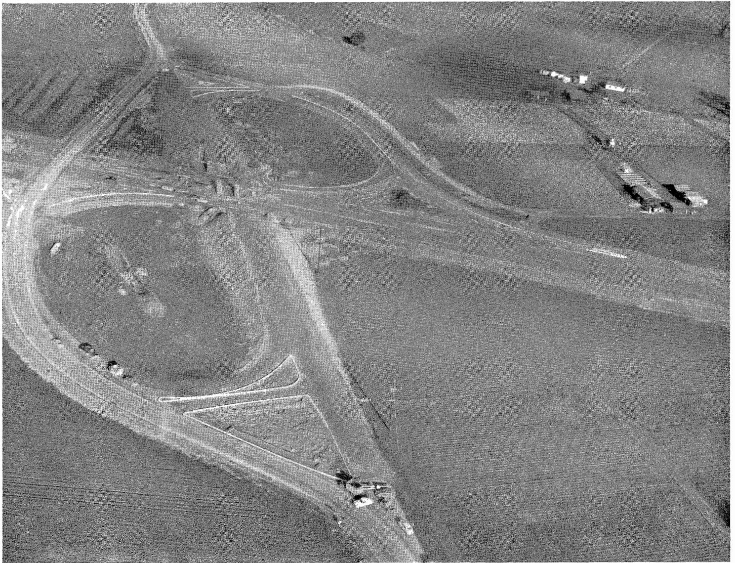
This photograph shows construction at Trimble Road overcrossing
