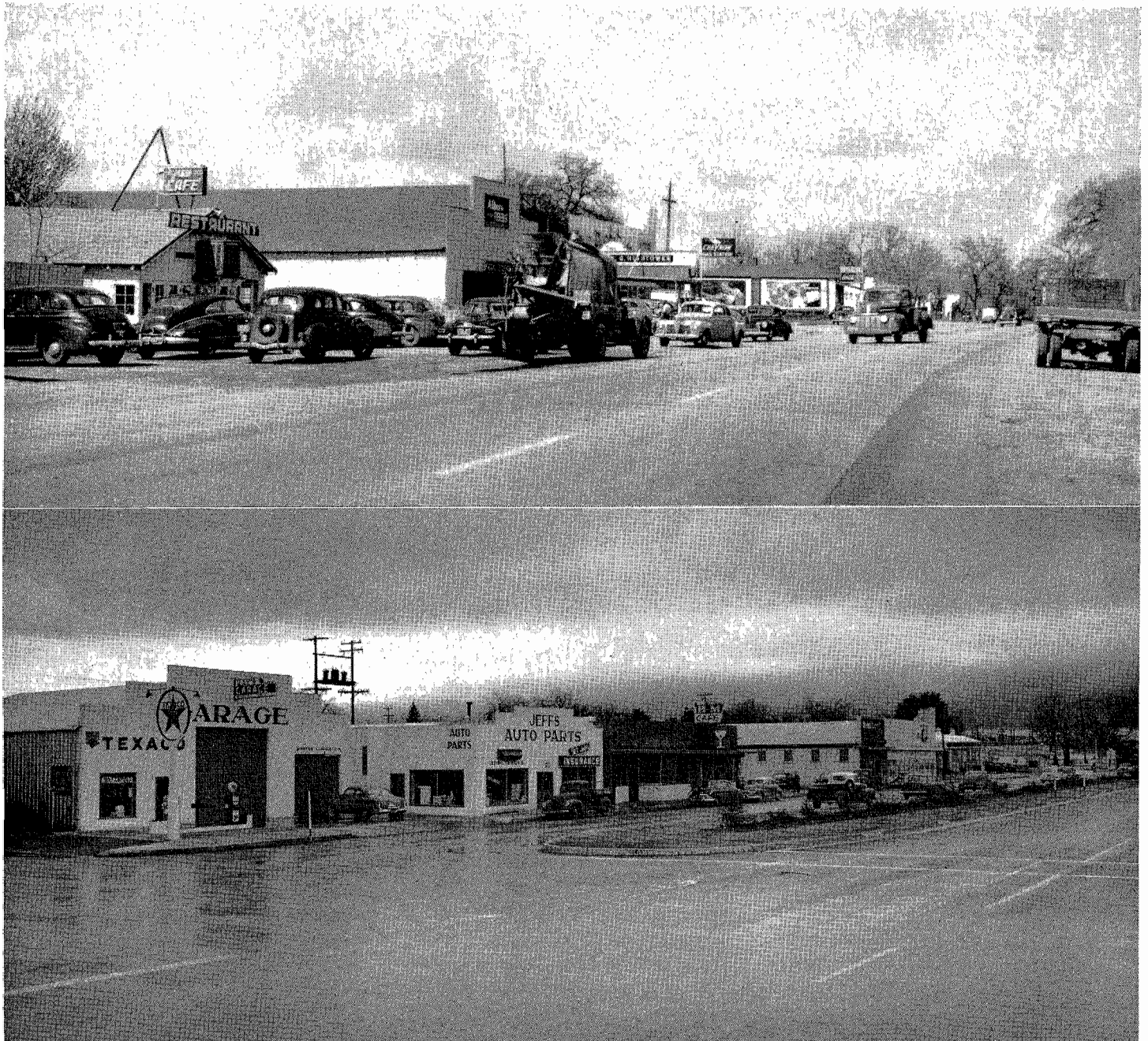
UPPER—East Center Street in Anderson before new highway construction. LOWER—Same thoroughfare after completion of freeway.
