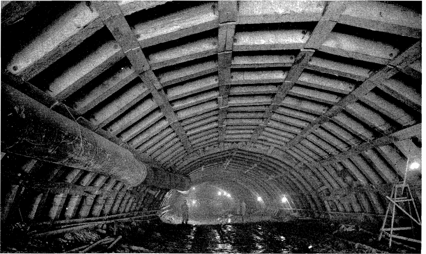
UPPER—Transition from timber to steel tunnel supports. The frill jumbo is shown in the background. LOWER—Photo showing the nine-segment timber tunnel support in the heading section. Steel supports are shown in the background. Note that the steel supports require less excavation and therefore less concrete lining thickness than the timber supports. Thirty-inch blower line is shown at left center.
