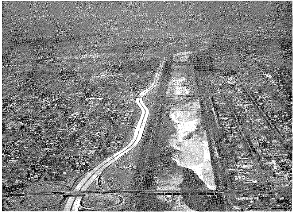
Airplane view looking northerly along completed Long Beach Freeway from Pacific Coast Highway in foreground to 223d Street in background. Beyond is shown construction now in progress along the Los Angeles River.
