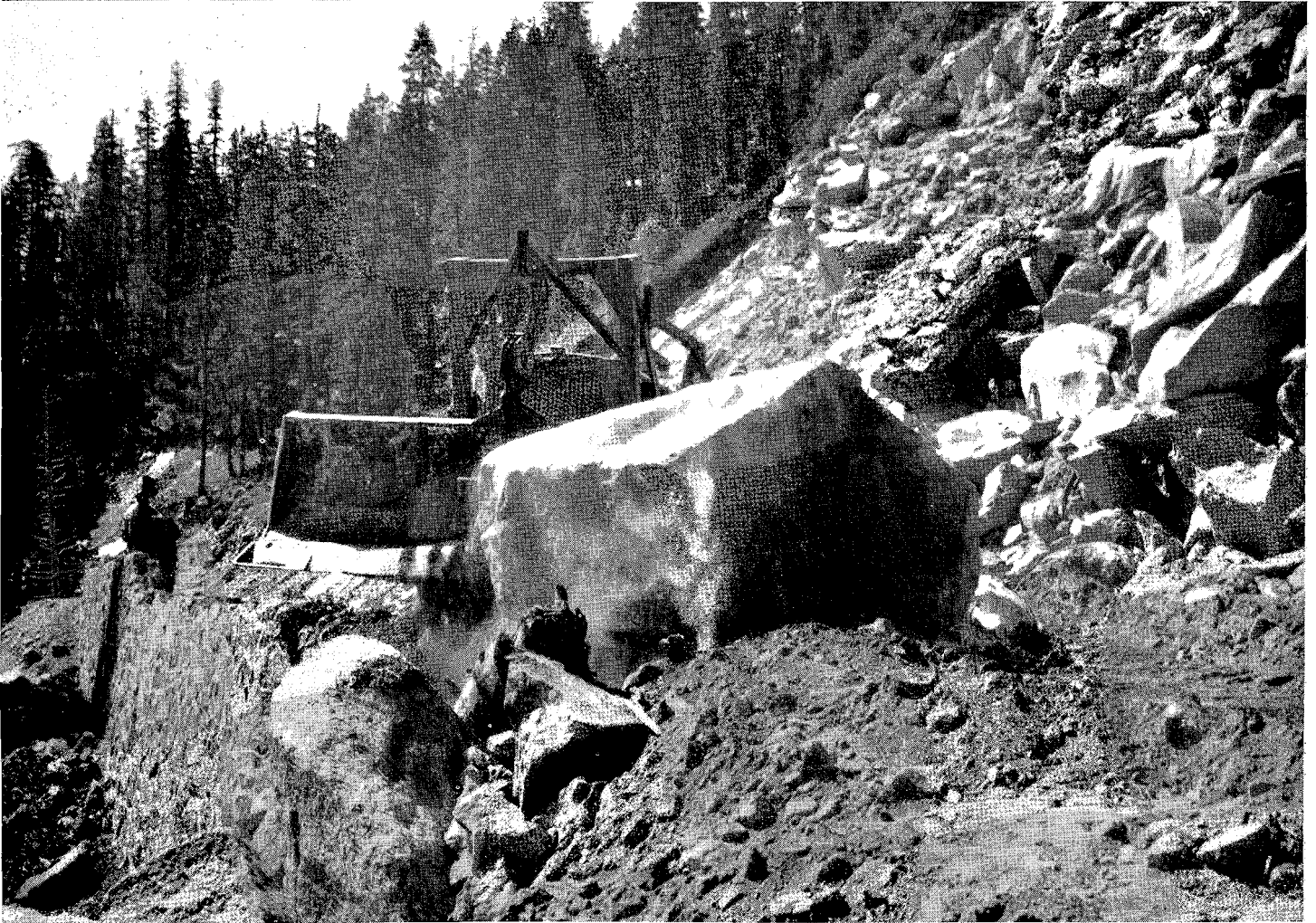
UPPER—Aerial view of slide area near Emerald Bay. LOWER—Bulldozer clearing rock slide from Sign Route 89.
