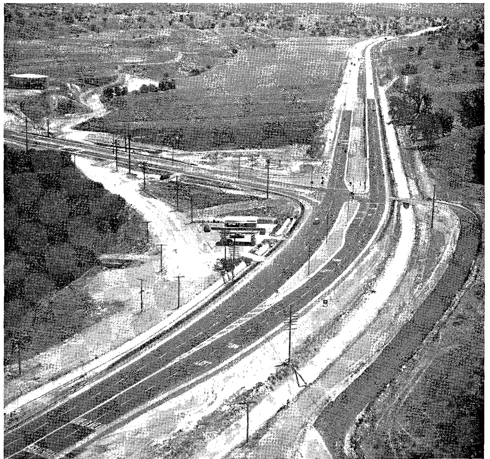
UPPER—View looking southerly through Weldon Summit, showing flattening of excavation slope on left in order to eliminate possibility of slides occurring that might obstruct highway. LOWER—Looking southerly along Ridge Route, showing junction with State Route 79 leading easterly to Saugus.
