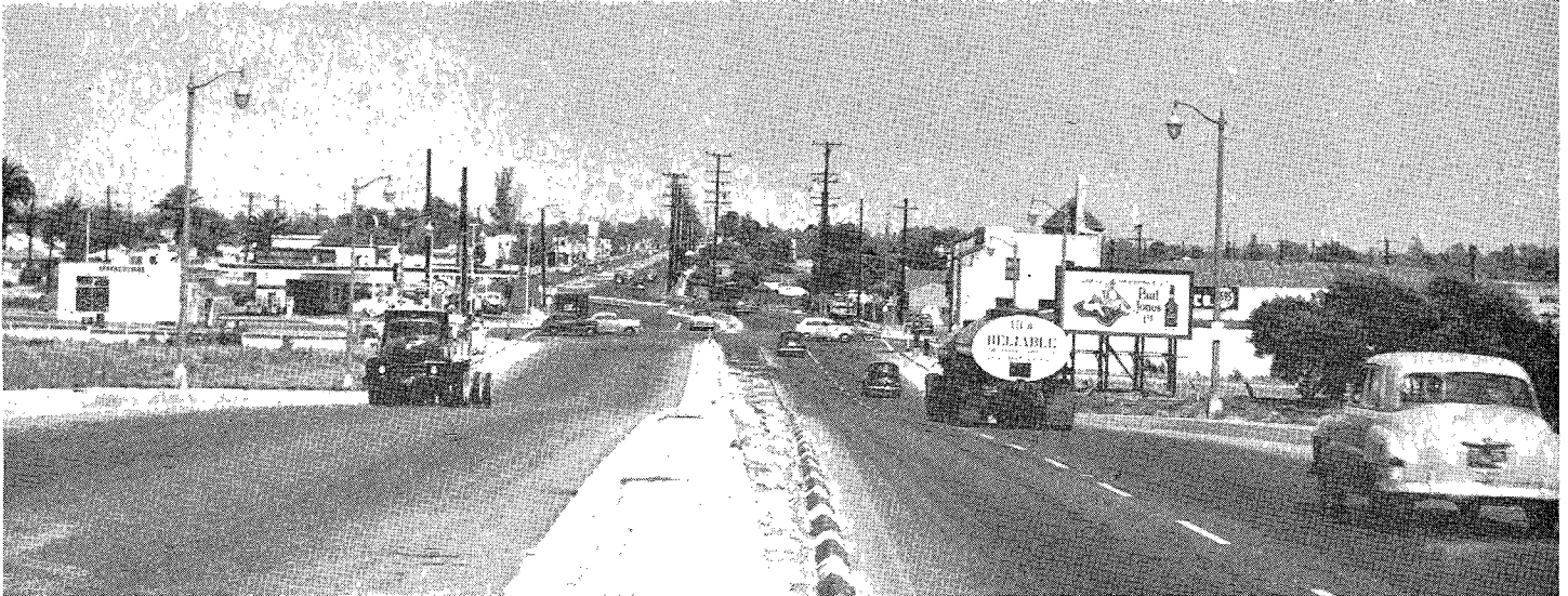
Completed Artesia Street improvement looking easterly from the Los Angeles River Bridge. The intersecting street in center of photograph is Atlantic Boulevard, State Highway Route 167.
