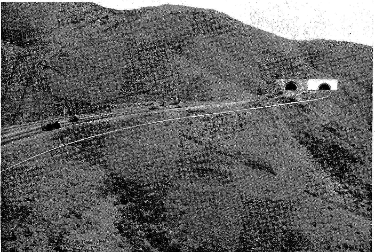
Looking north from a point above the Fort Cronkhite Tunnel portal to the site of the twin Waldo Tunnel bore. The centerline of the proposed three northbound lanes and the new northbound tunnel are shown in white.
