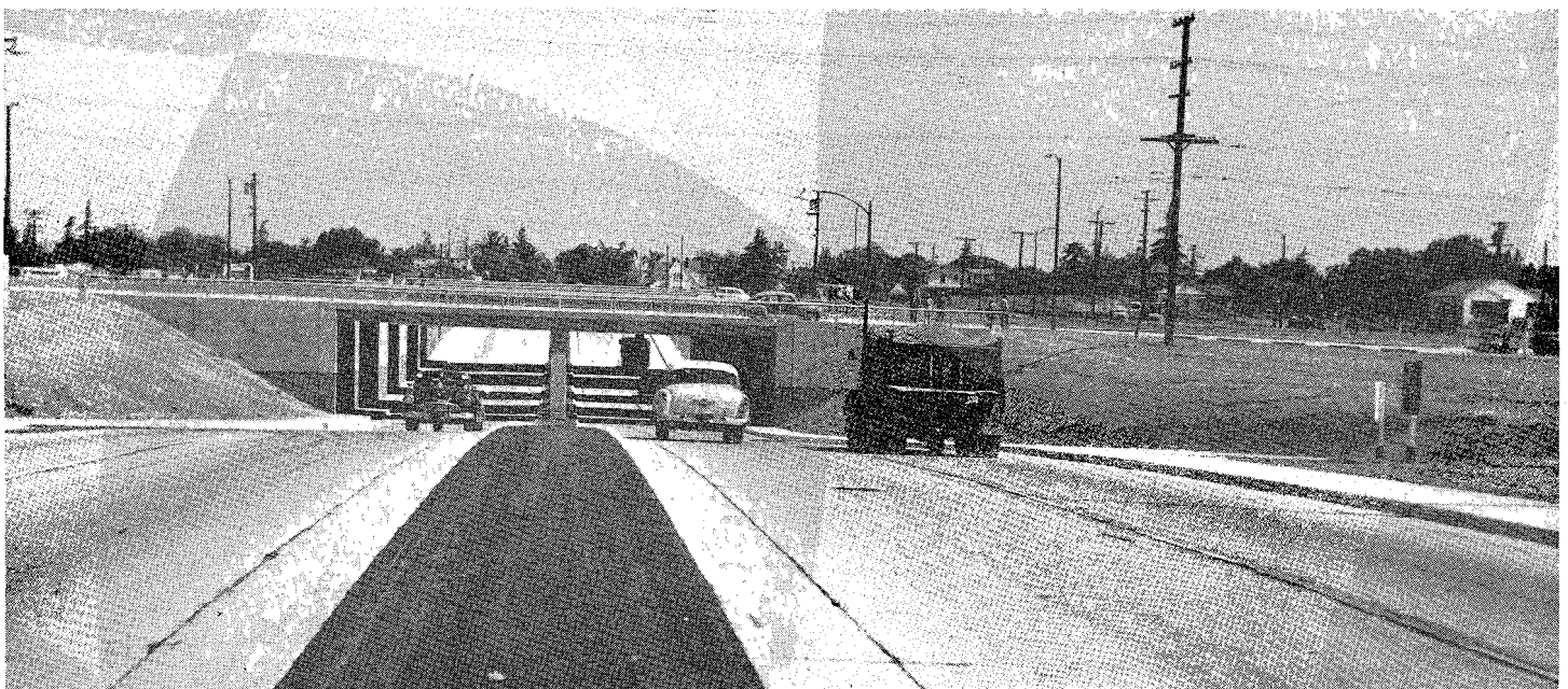
View looking northerly along Atlantic Boulevard, State Highway Route 167, showing completed bridge to carry Ramona Freeway over Atlantic Boulevard
