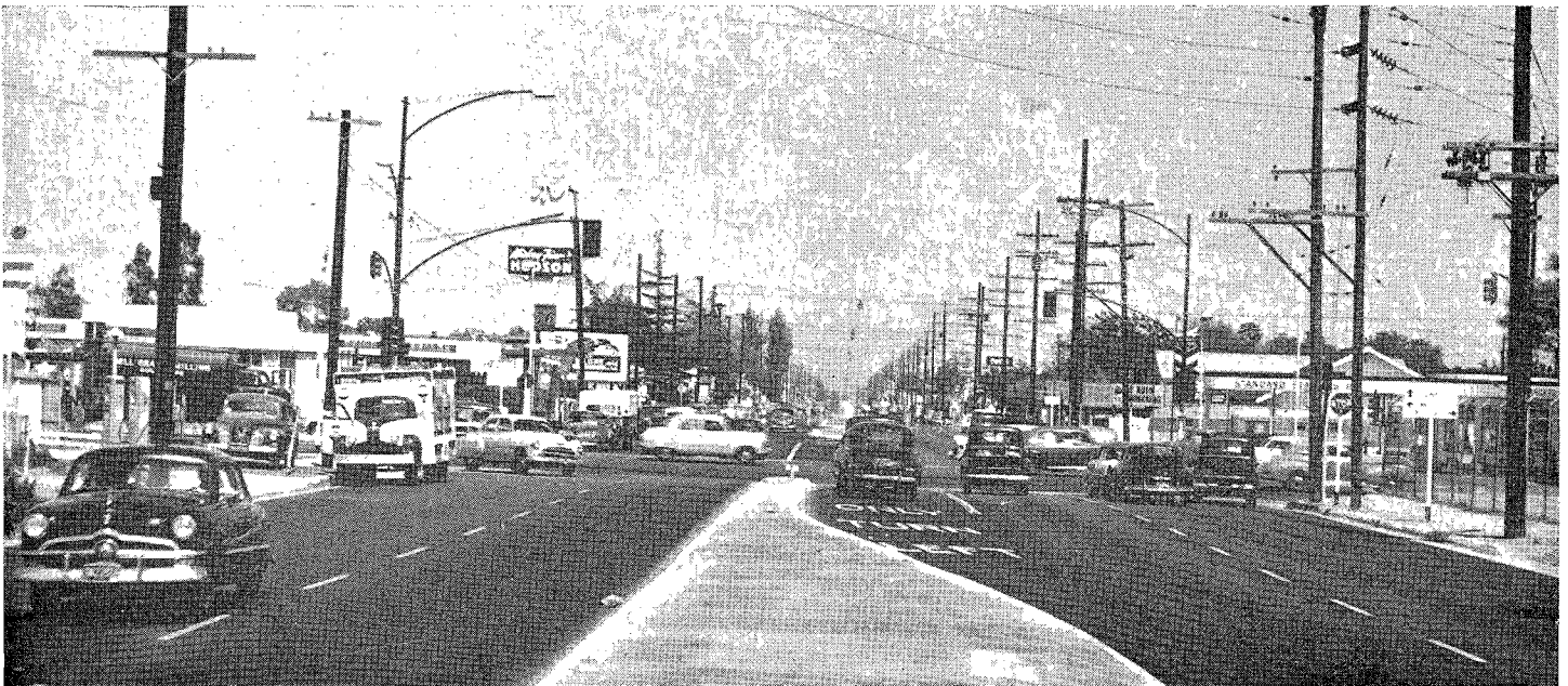
Looking easterly along completed Artesia Street improvement. The intersection in the foreground is with Lakewood Boulevard, State Highway Route 168.
