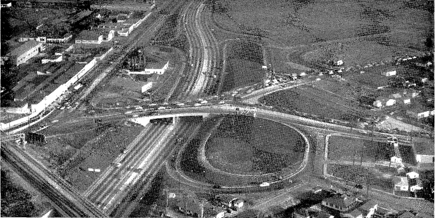
Airplane view looking southeasterly along Santa Ana Freeway showing traffic congestion on Eastern Avenue and Atlantic Boulevard where these traffic arteries come together and cross the freeway on a grade separation bridge. Union Pacific Railroad tracks are shown to the left. This traffic interchange system has become known as "The Mixmaster." Traffic congestion such as pictured here that occurs during peak hours will be relieved by construction of the Long Beach Freeway and road projects now under construction by the Los Angeles County Road Department.
