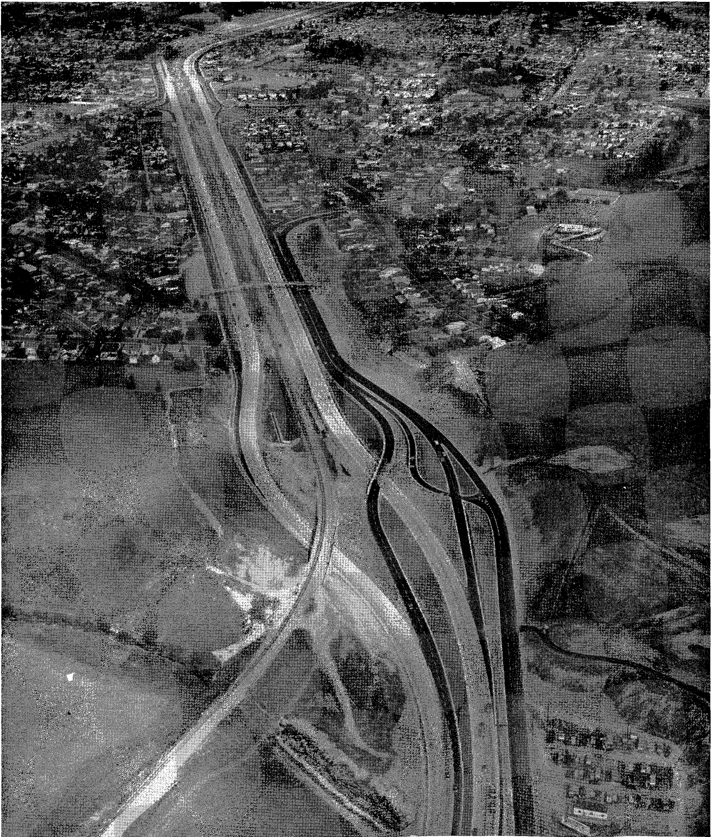
Looking easterly along completed portion of Ramona Freeway recently opened to traffic between Eastern Avenue and Fremont Avenue
