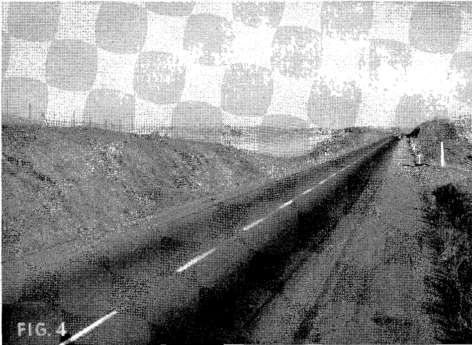
UPPER—Single line in foreground is California's Experimental Type III in background. On U. S. 50 section change just east of Folsom. LOWER—California Standard Type IV traffic stripe after eight months' service.
