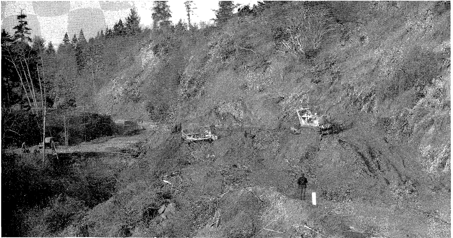
UPPER — Temporary detour under construction around washed out embankment 20 miles north of Eureka on Redwood Highway. LOWER—Washed out roadway on Redwood Highway seven miles north of Trinidad.
