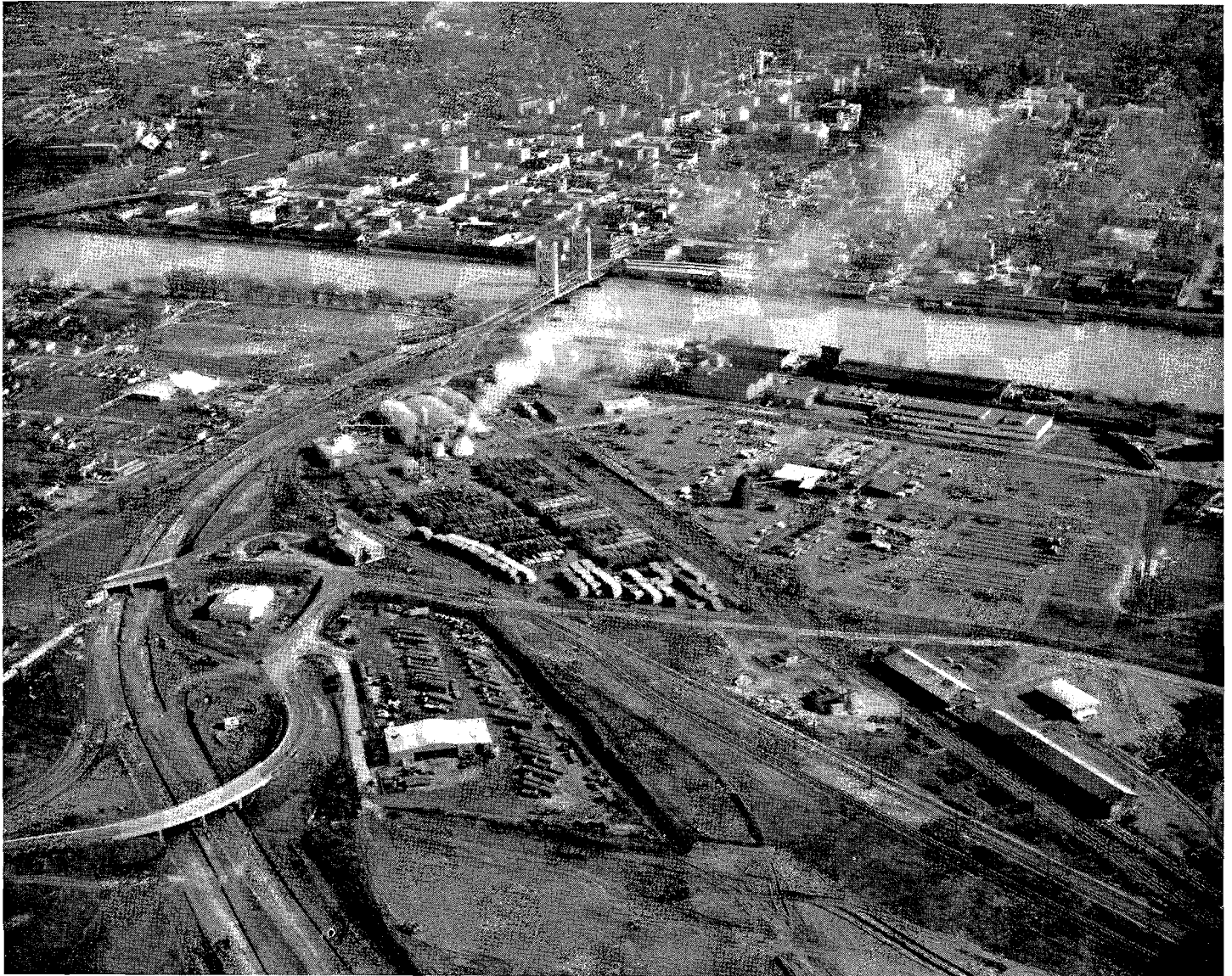
From top to bottom structures are as follows: Tower Bridge, West Sacramento Underpass and Davis Highway Ramp Overcrossing
