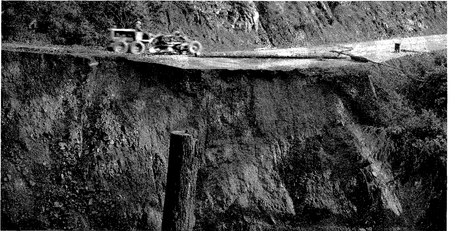
Fifteen hundred cubic yards of embankment washed out five miles east of Blue Lake on Arcata to Redding lateral, U. S. 299
