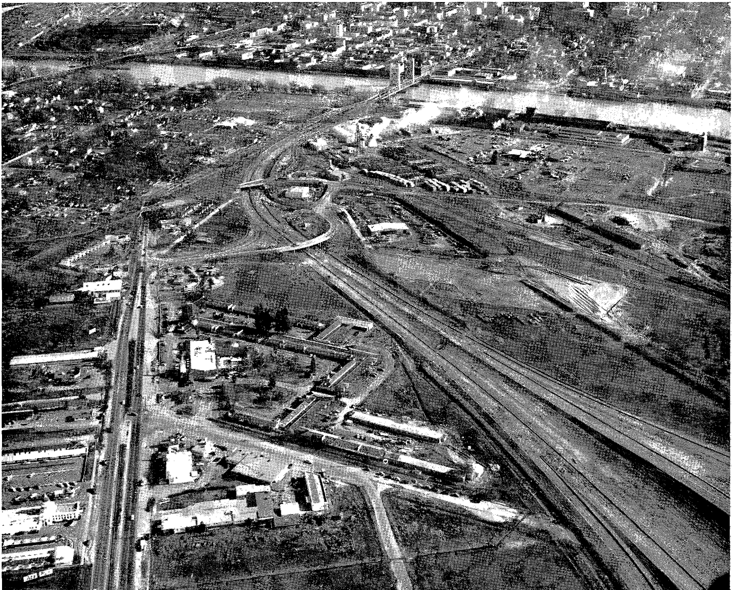
From top to bottom structures are as follows: Tower Bridge, West Sacramento Underpass and Davis Highway Ramp Overcrossing
