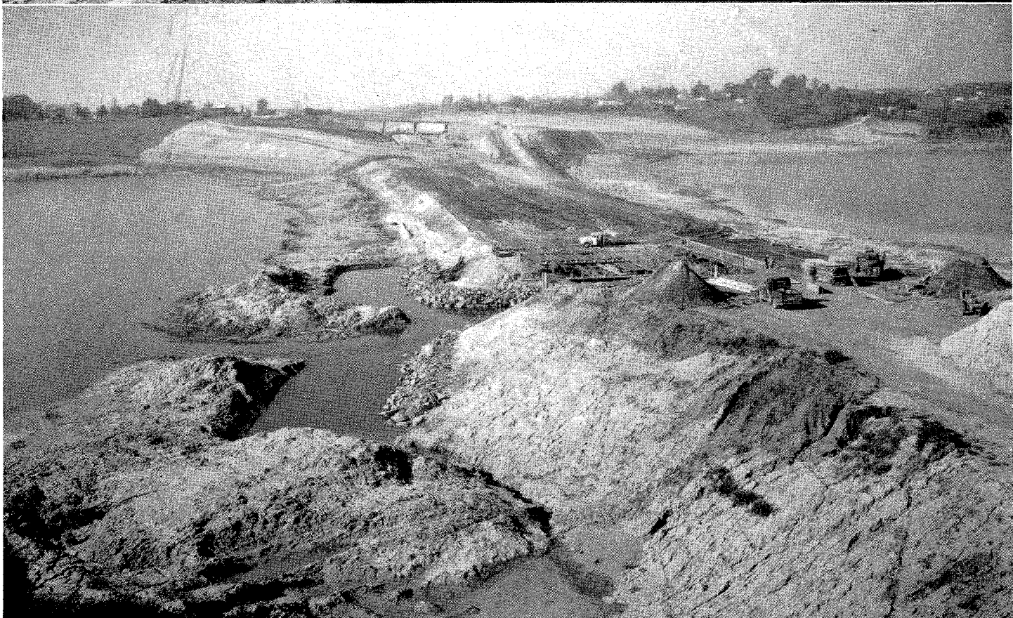
UPPER—Storm drain construction. LOWER—Fill and structures at Buena Vista.
