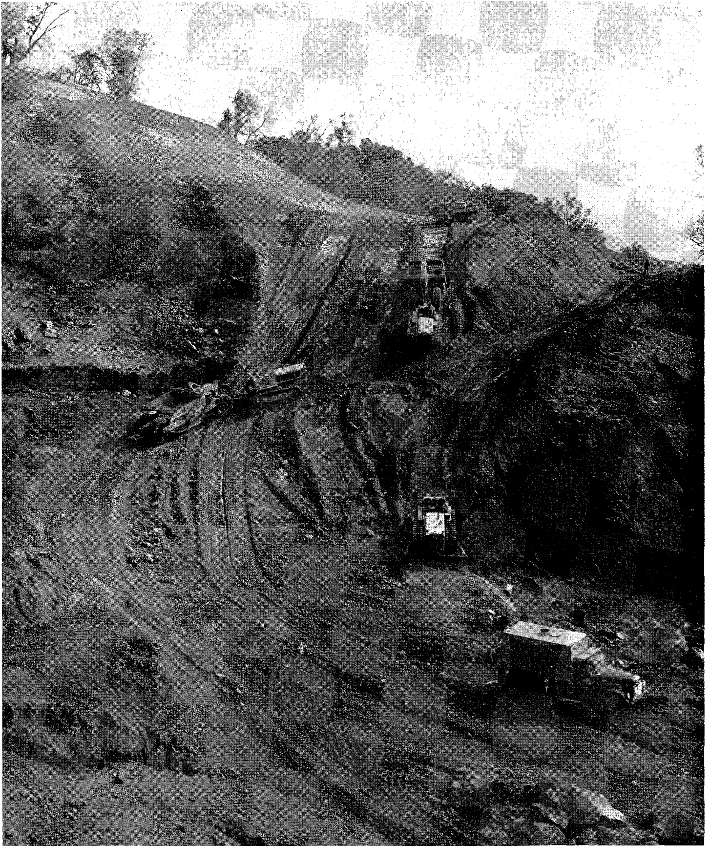
Heavy construction on section of Ridgewood grade project
