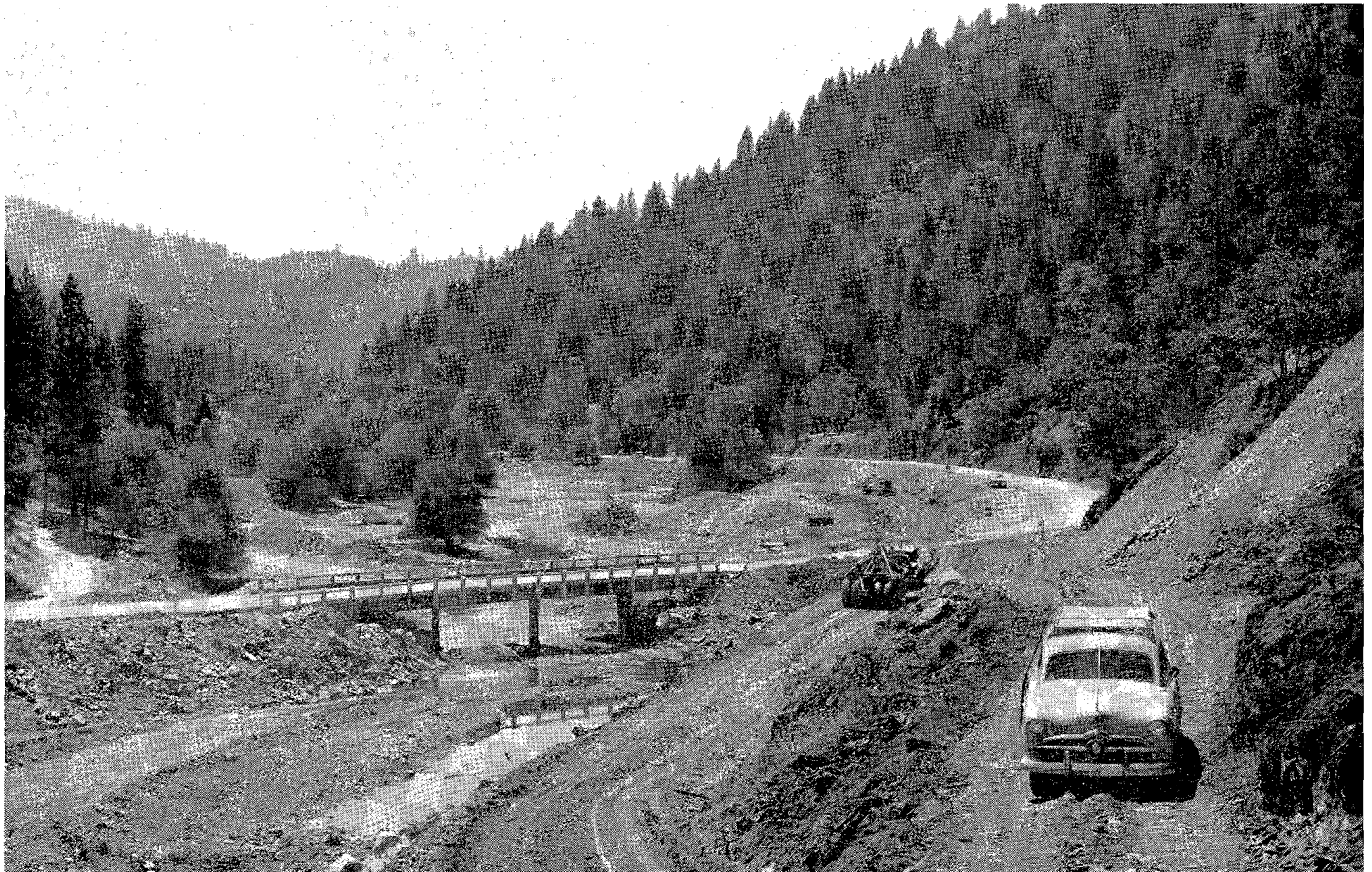
Present Weaver Creek Bridge that lost a span in last winter's flood. All the gravel in this creek channel has been mined many times.
