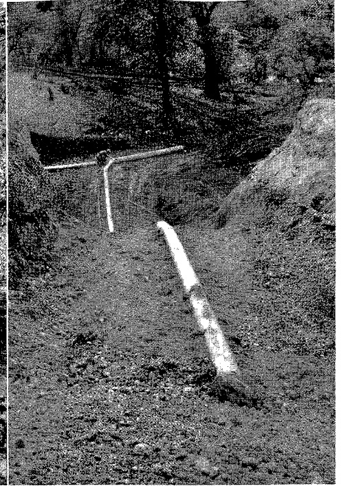
Slab trench showing pipe in place
