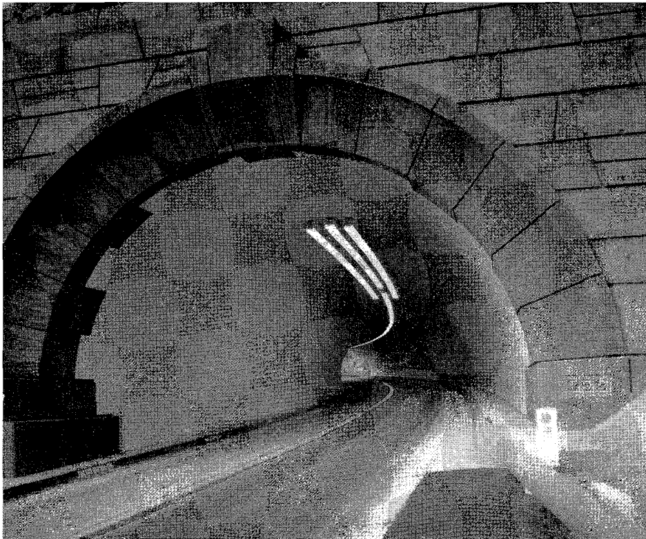
Tunnel lighting from south face of bore
