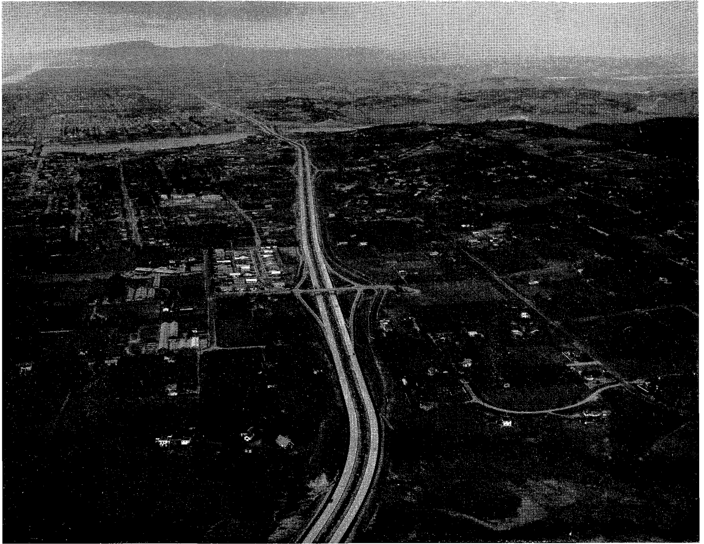
Looking north on freeway through Carlsbad. Tamarack overcrossing in center foreground.
