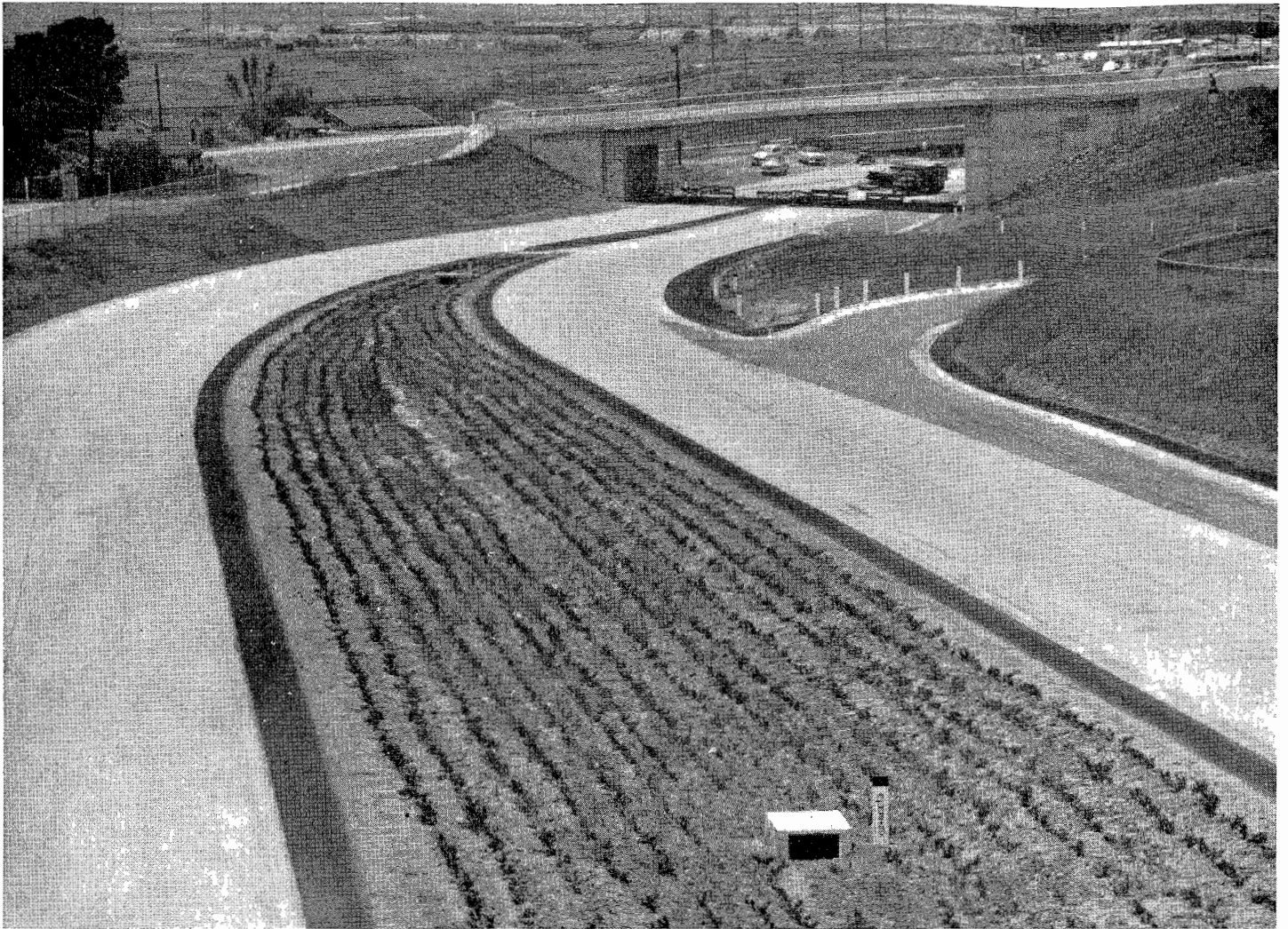
On this new section of freeway the soil will be kept in place by means of ice plant and natural grasses on the adjoining hillsides and the sloping shallow ditch which separates the northbound and southbound roadways. This is an example of planting which the Division of Highways has found necessary in enhancing traffic safety and keeping down future maintenance costs. The freeway shown here is U. S. 101 in Oceanside.
