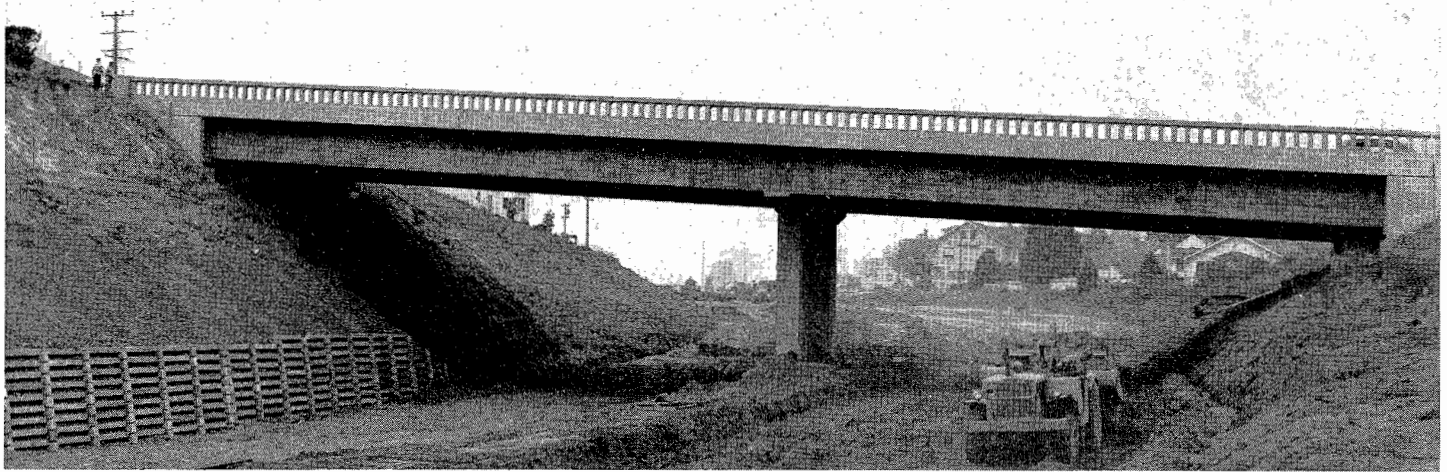
Bulldozer removing unstable material under bridge on bypass
