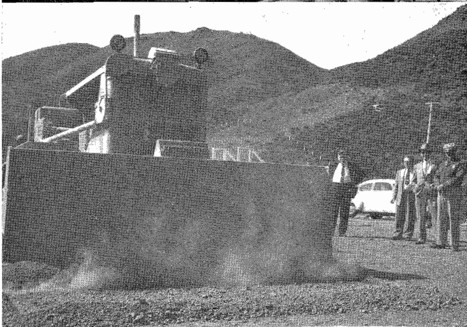
UPPER—On deck of groundbreaking bulldozer. LEFT TO RIGHT—Director of Public Works Frank B. Durkee, Joseph Diviny, President, Golden Gate Bridge and Highway District; Highway Commissioner, Walter Sandelin, State Highway Engineer, George T. McCoy, Lee H. McLeod. LOWER—Bulldozer breaks ground.
