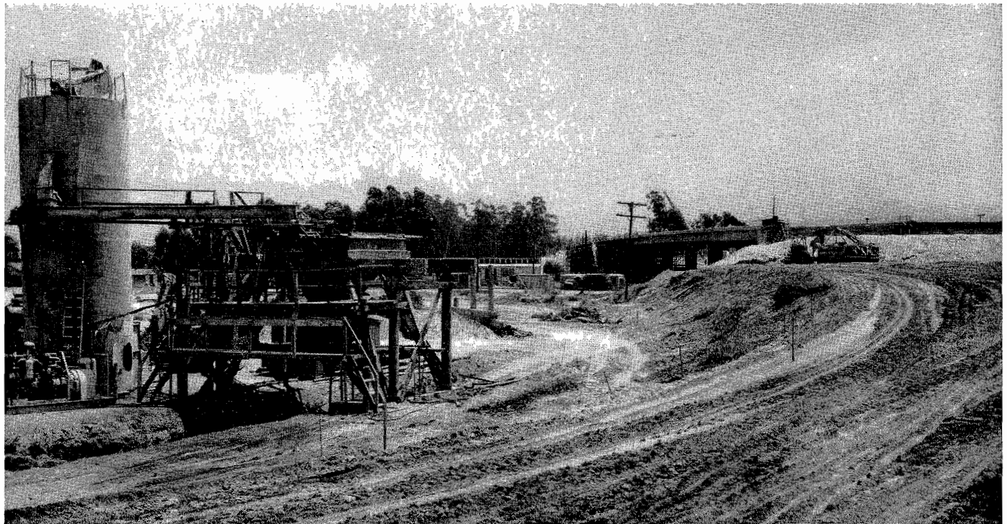
UPPER—View looking easterly along Camarillo Freeway from near Fulton Street showing grading operations in progress. In background is Camarillo Overhead. LOWER—View looking southeasterly toward Camarillo Overhead structure showing contractor's batching plant in center left of photograph.
