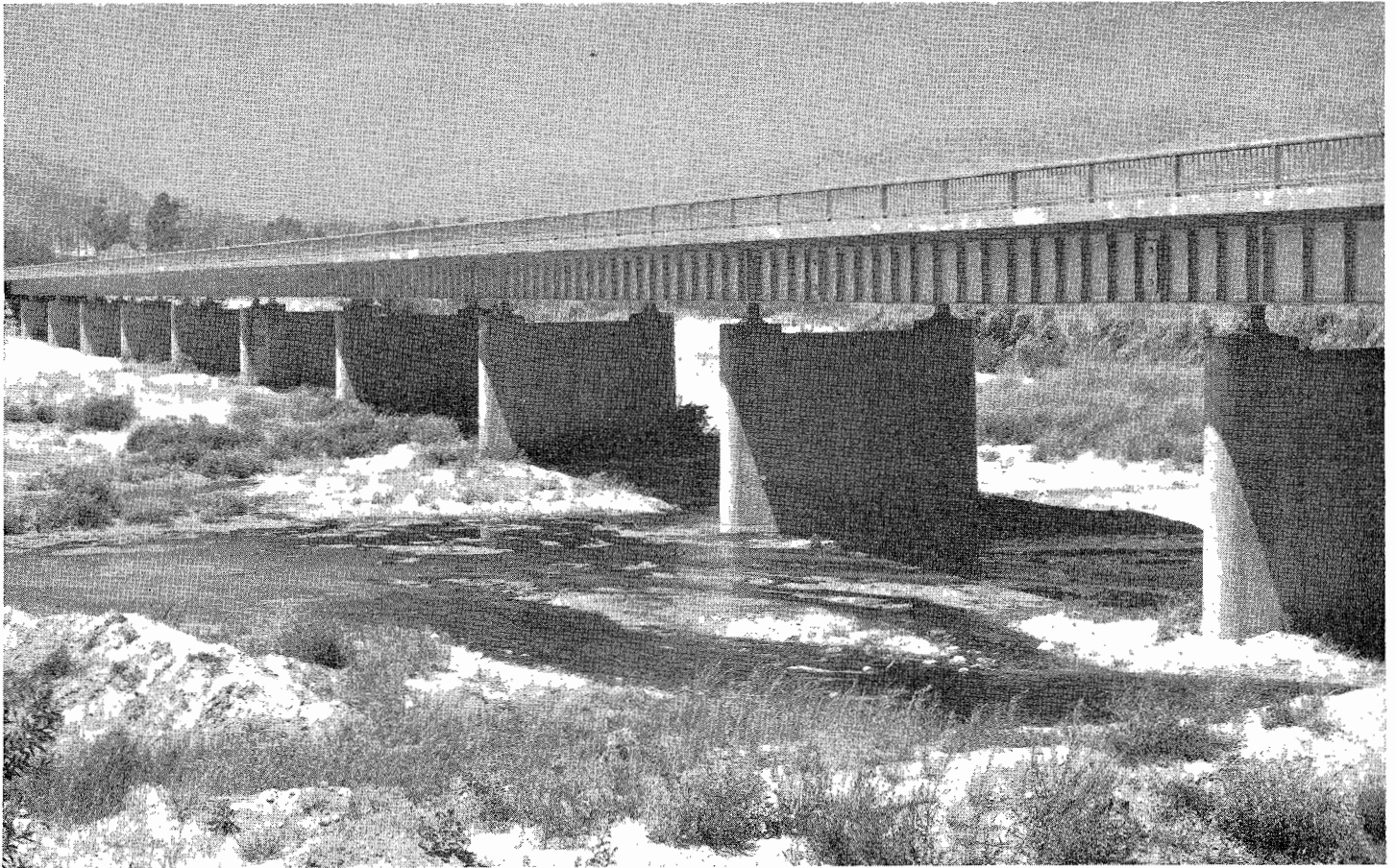
New Willard Bridge at Santa Paula over Santa Clara River. A fine example of county, state, and federal cooperation under the Federal Aid Secondary Highway Program.
