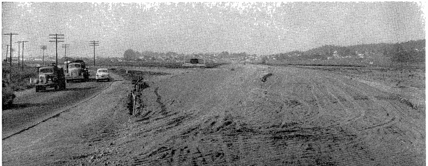
Start of construction on south end of project
