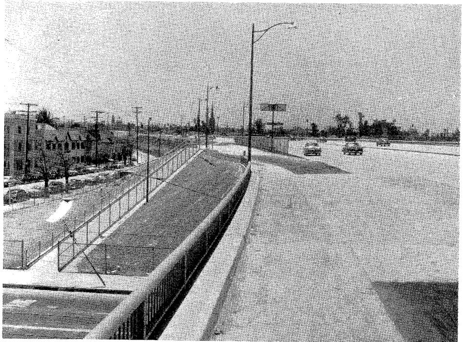
Looking southerly along completed section of Harbor Freeway from above Pico Boulevard, showing bus turnout on east side of freeway for northbound traffic. The city street shown on extreme left is Bond Street.
