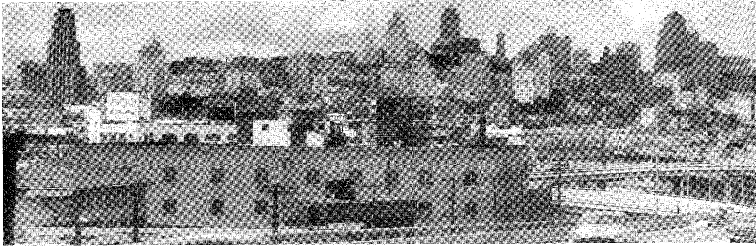
Entering the city from the south the elevated structures
