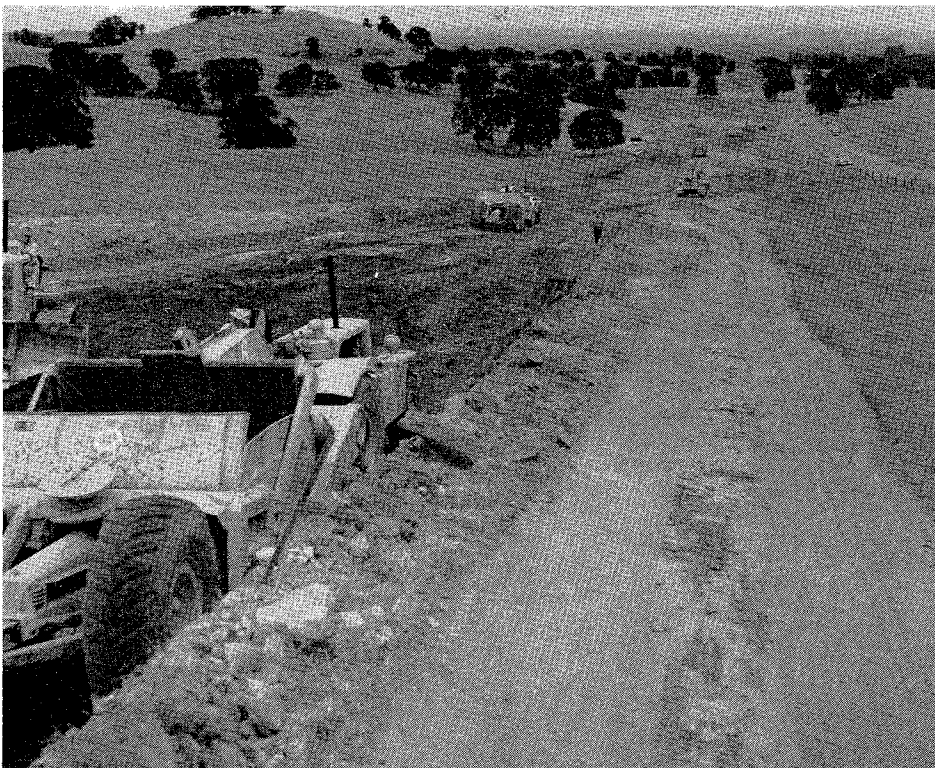
Grading between Amador County line and two miles easterly
