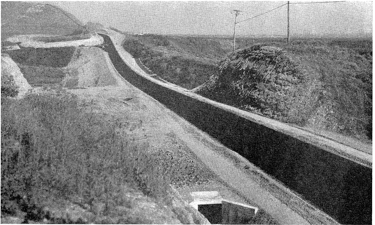
Looking south toward Laguna Creek fill
