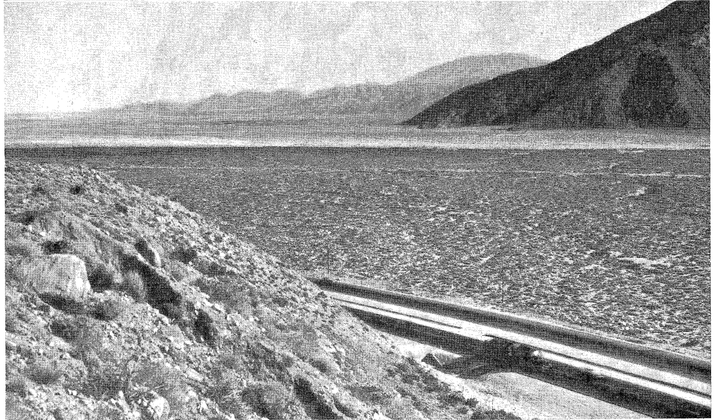
UPPER: Recently completed bridges across Whitewater River. Although the channel in this February scene is dry and dusty, a peak discharge of 42,000 cubic feet per second was recorded at this site in the March, 1938, flood. LOWER: Looking south from the vicinity of Whitewater toward Coachella Valley. Recently completed construction in foreground. Palm Springs in center background beyond Whitewater River.
