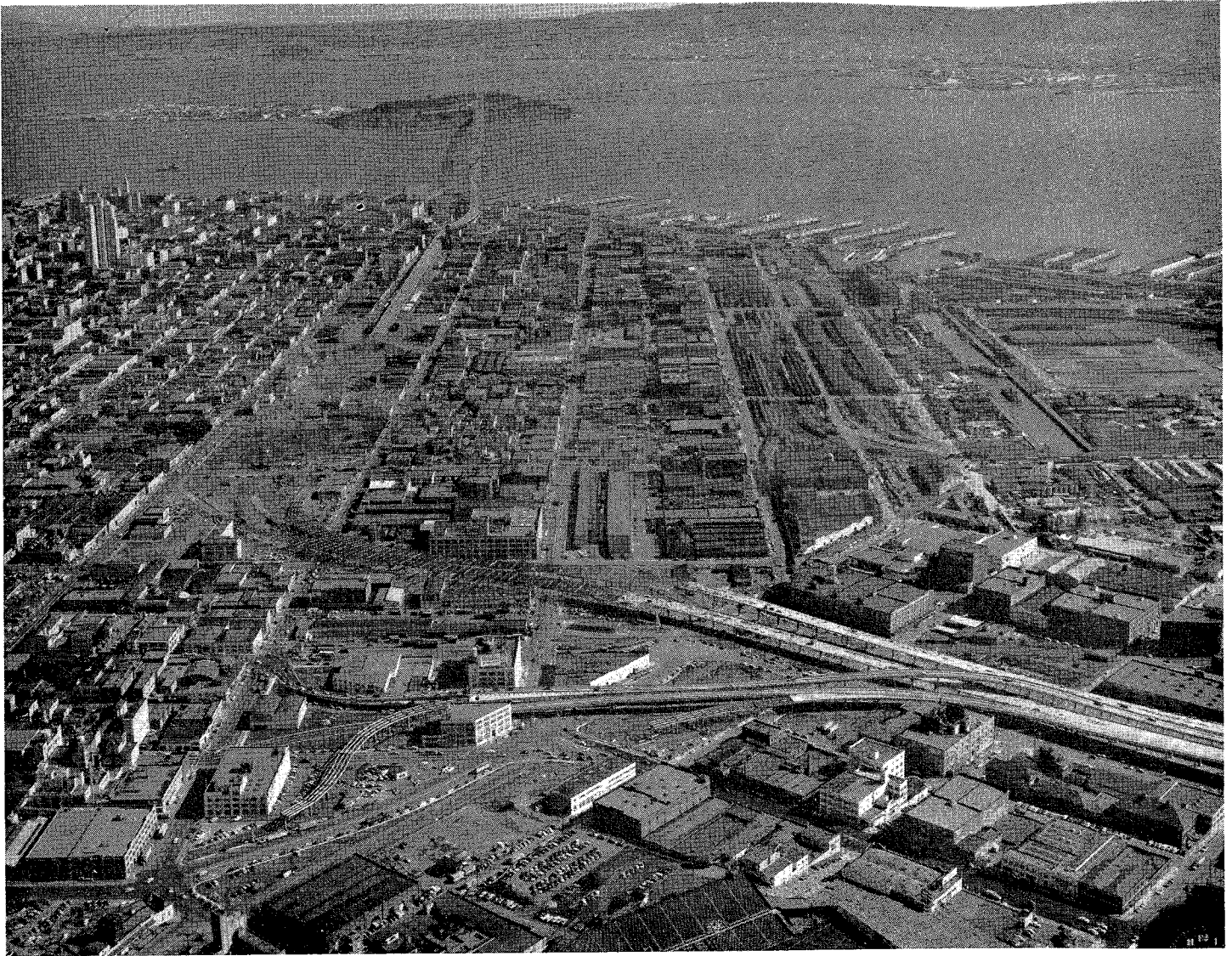
Central portion of San Francisco, showing Bayshore Freeway construction extending toward connection with Bay Bridge
