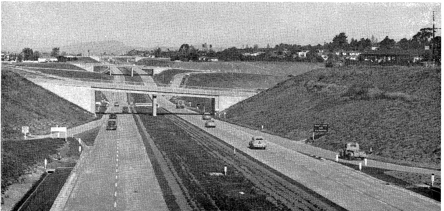
Looking north along a portion of the Oceanside Freeway, showing some of the grade separations and interchange ramps which have contributed to a sharp reduction in accidents since opening of the freeway on November 16, 1953
