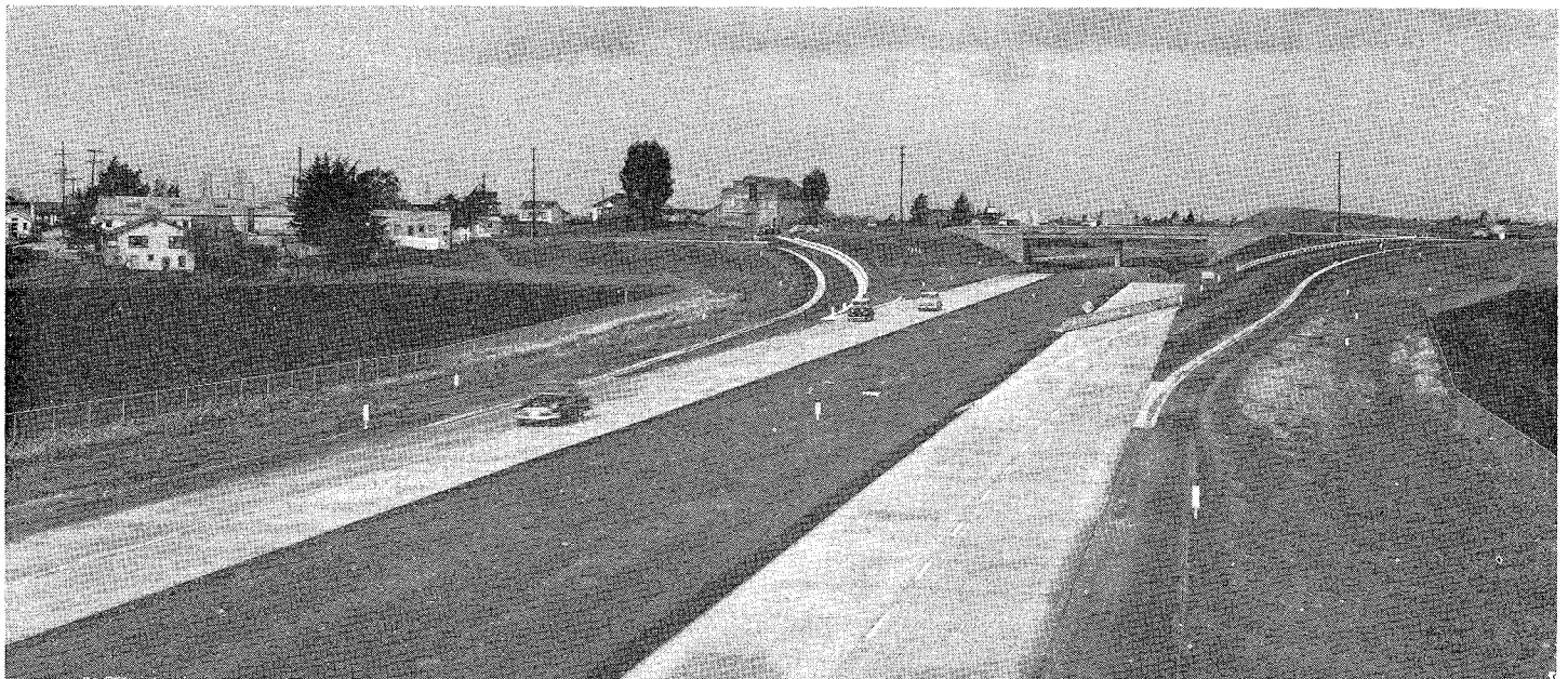
View of North Main Street interchange looking north from Sherwood Drive Undercrossing
