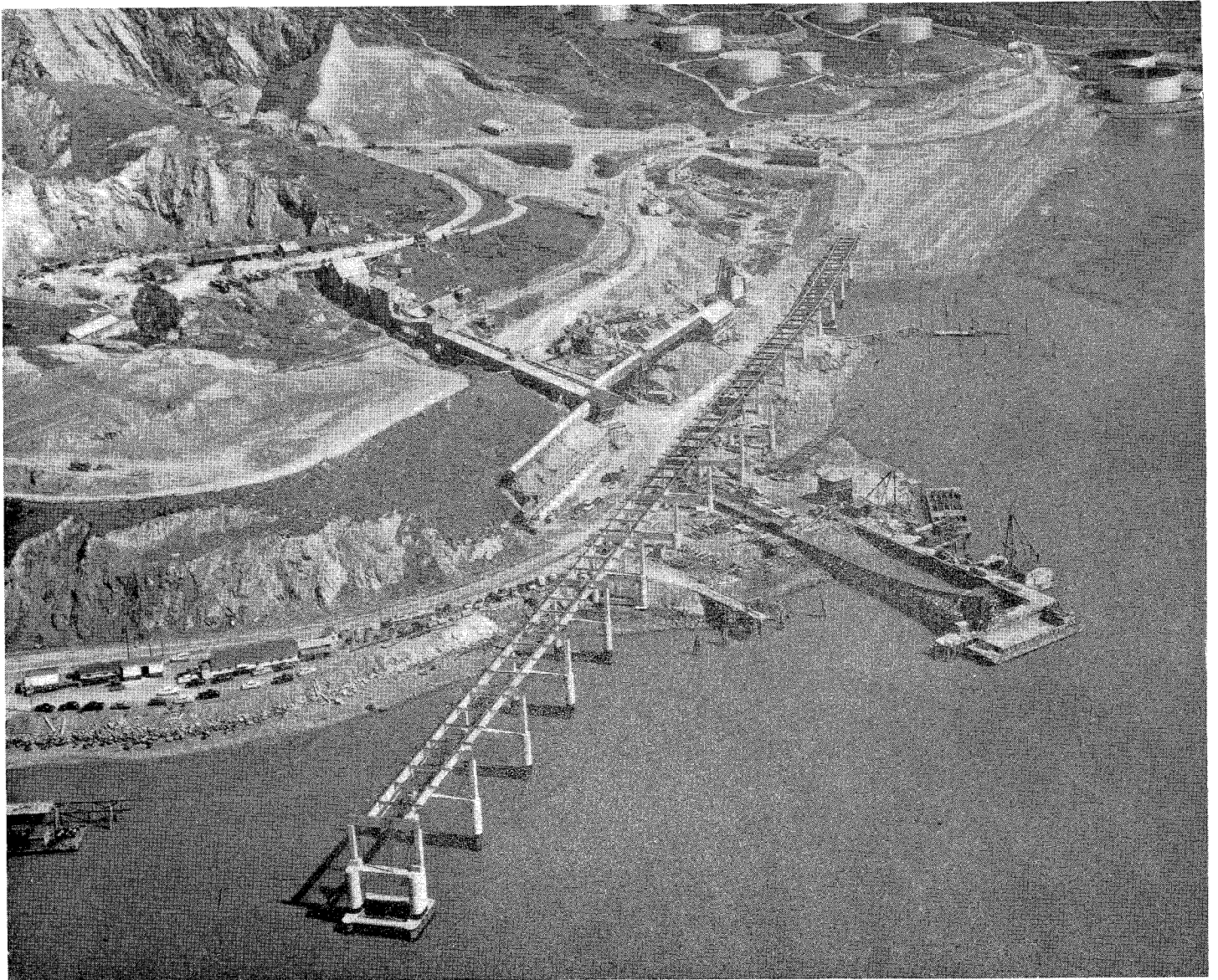
Completed piers Nos. 61-78 with start of steel construction, Contra Costa County
