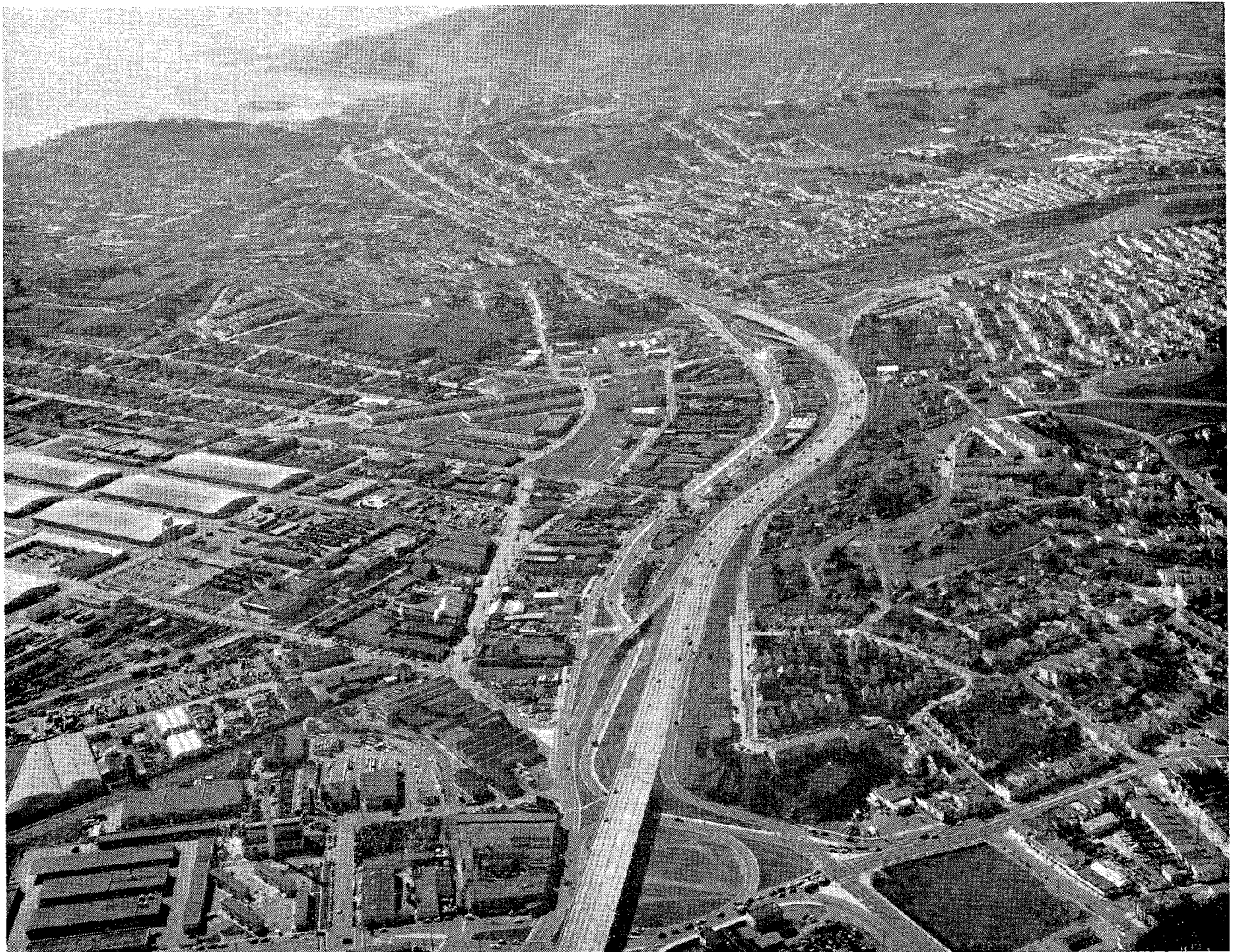
Bayshore Freeway in San Francisco; Army Street interchange at bottom; Alemany Boulevard interchange, center; with section presently under construction between Alemany Boulevard and Third Street extending to upper left
