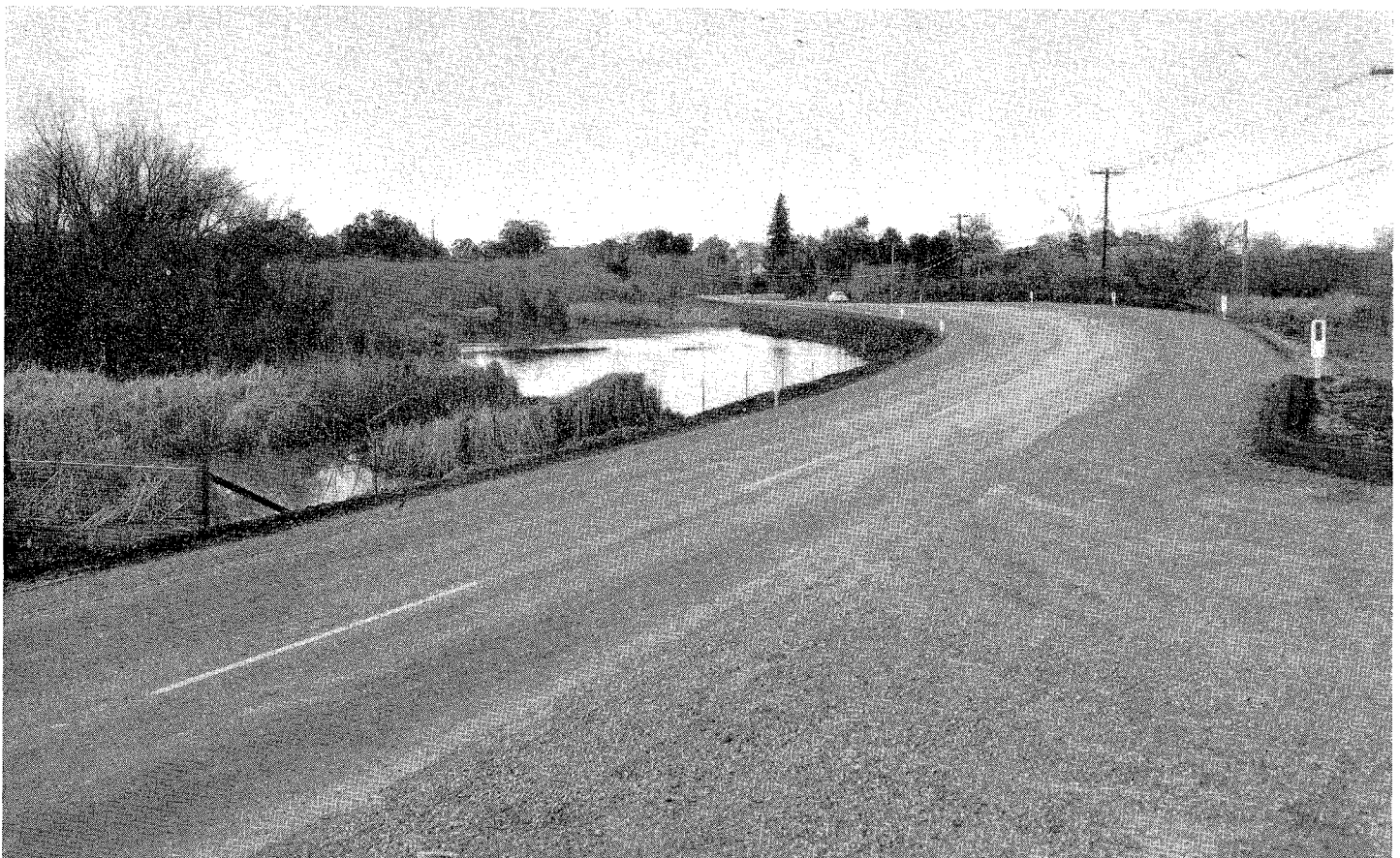
FAS Route 1048, a San Mateo County road recently reconstructed with federal, state, and county funds
