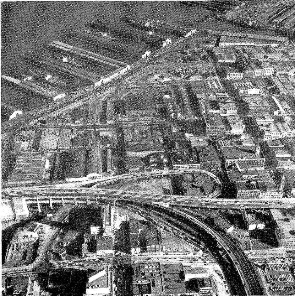
Close-up of the San Francisco ramp system looking southerly. In the center foreground, automobile traffic in the San Francisco city streets is being partially diverted to the lower deck (truck level) by the San Francisco city police. The absence of Key System buses, which normally use the lower deck, assisted materially in making it possible to divert a substantial amount of upper-deck traffic to the truck level, thereby relieving the potential bottleneck at the merging point of upper-deck ramps shown at center righthand portion of picture.
