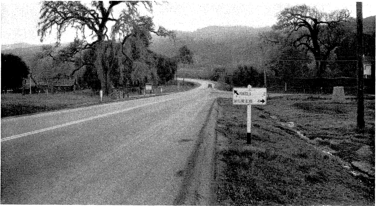
North end of Portola Road. This county road was recently reconstructed under the Federal Aid Secondary Highway Program.
