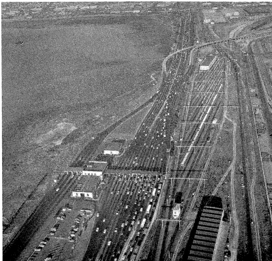
Close-up of Toll Plaza looking easterly. Note the idle railway rolling stock in storage yard adjacent to toll gates. Vehicular traffic passed through the toll gates in record numbers. The toll collection staff did a remarkable job under difficult circumstances as evidenced by the fact that collectors handled daily, during peak hours, as many as 12 cars per minute, or one car every five seconds.
