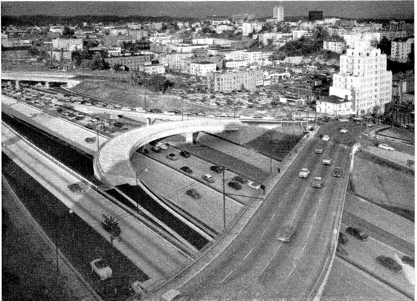
Evening peak hour traffic on the Harbor Freeway, with the Fifth Street Overcrossing in the foreground, the Fifth Street southbound on-ramp in the center and the northbound on-ramp carrying traffic in the direction of the four-level structure
