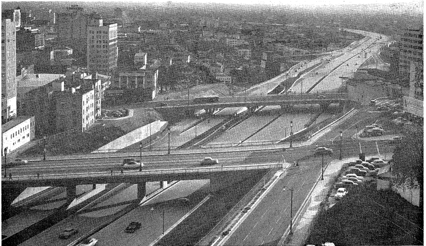
Looking south along Harbor Freeway. Wilshire Boulevard Overcrossing in foreground; Seventh Street Overcrossing in center.
