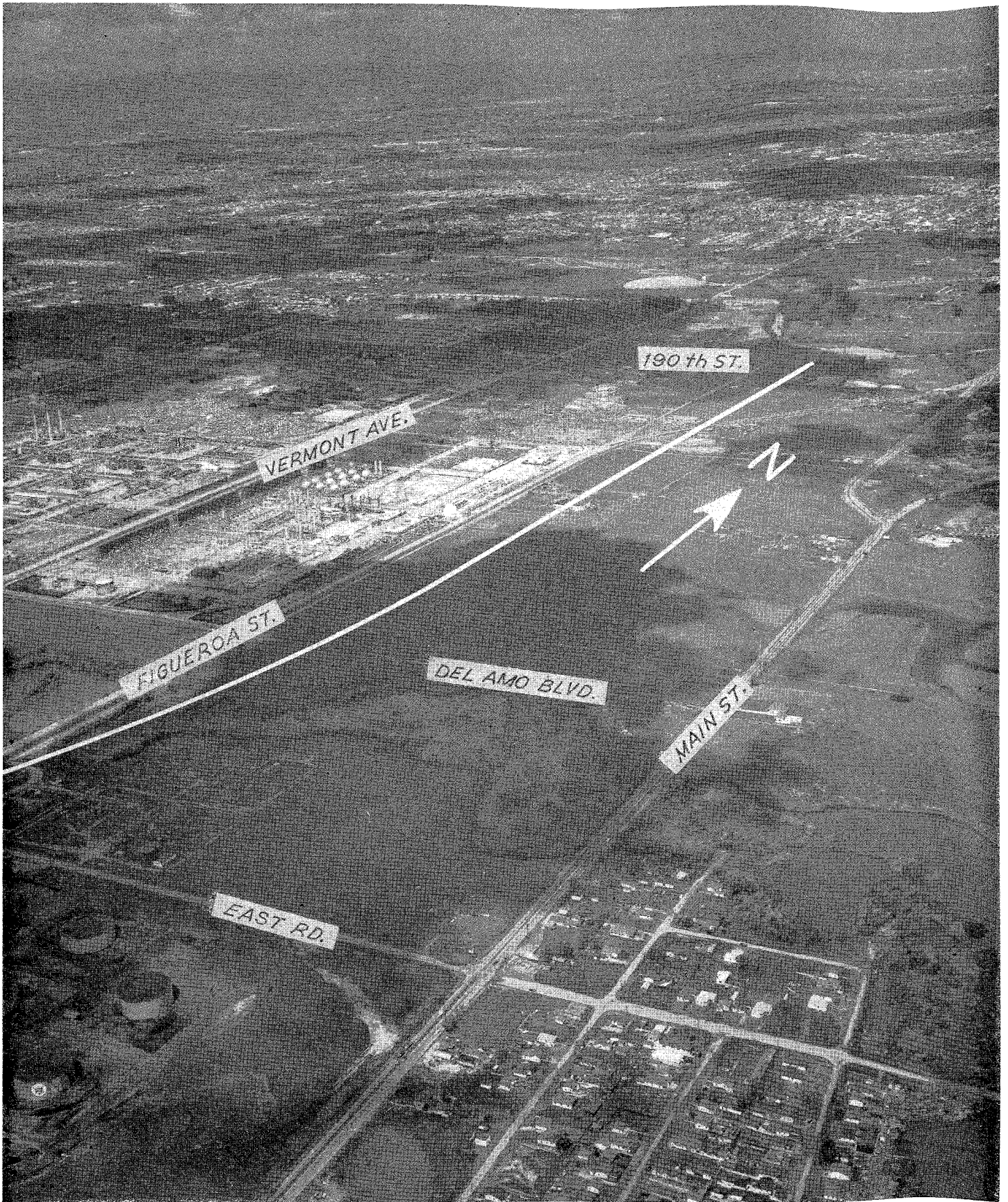
Looking northwesterly, Santa Monica mountains in background, showing Harbor Freeway in close proximity to Figueroa Street. The United States Government refinery leased to the Shell Oil Company is shown center left.
