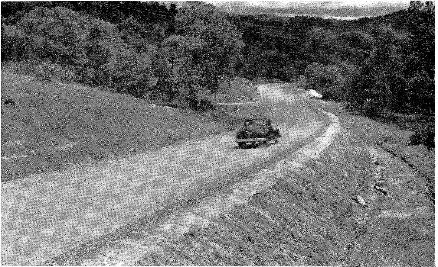
Typical alignment on new construction. Plant-mixed surfacing has not been placed.
