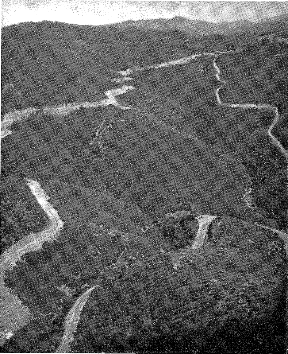
Upper portion of Priests Grade. Priests at top of picture. County road, Priests to Moccasin Creek power house on right. Widened state highway up grade on left.
