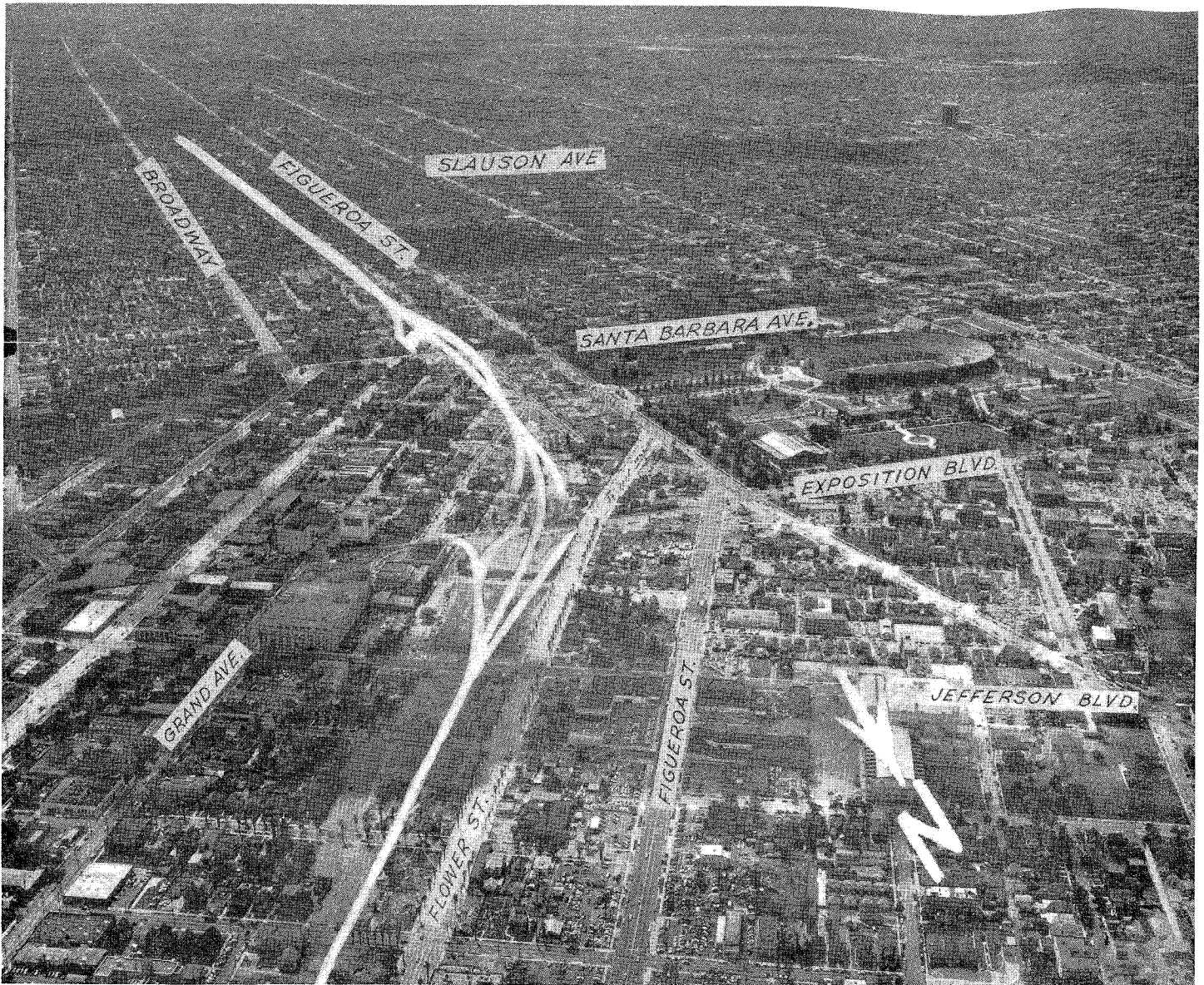
Looking southwesterly showing Harbor Freeway location close to Flower Street and Figueroa Street. Cleared right of way is in evidence foreground and center left. Los Angeles Memorial Coliseum in Exposition Park is shown center right.
