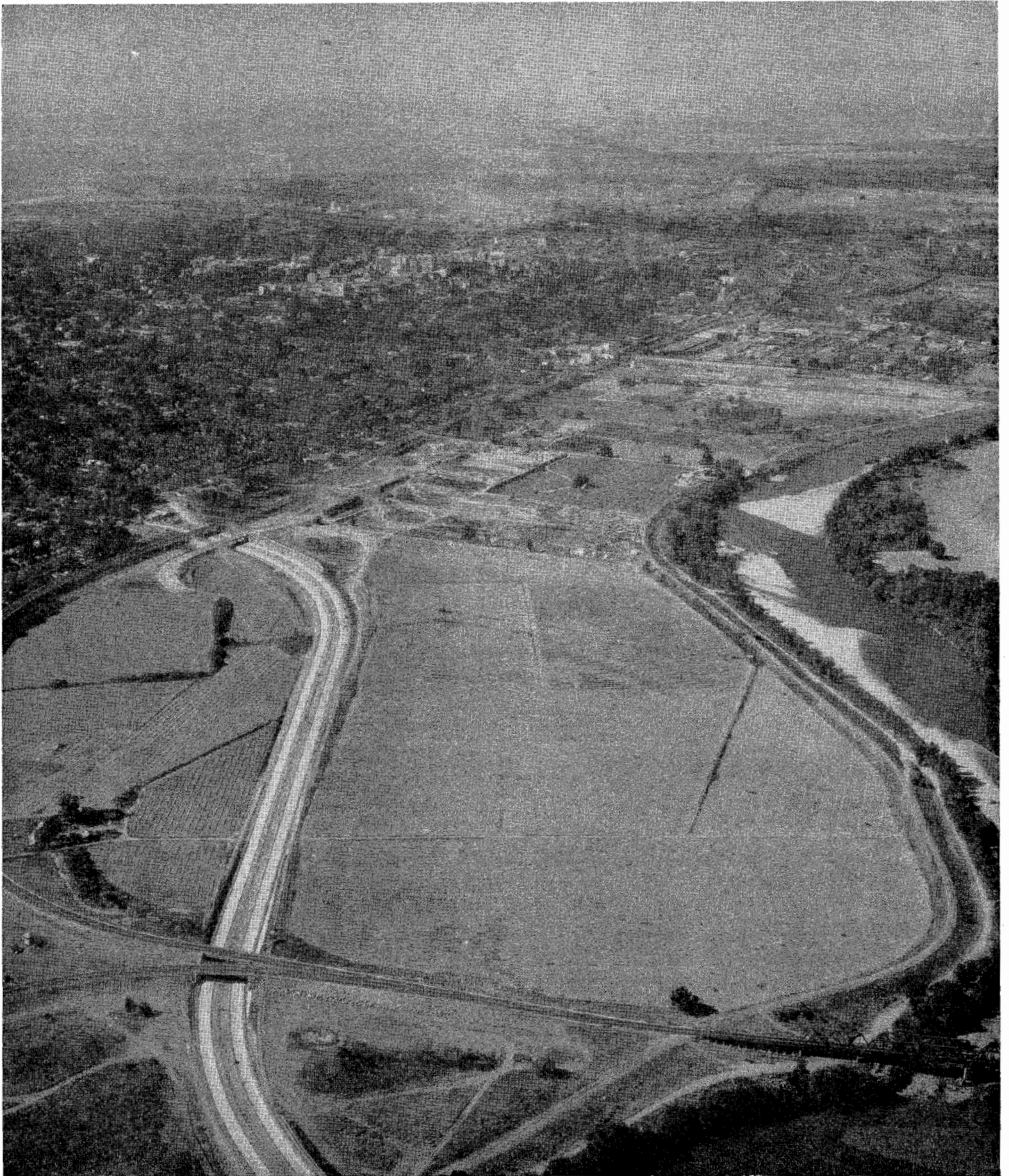
Elvas Underpass under Southern Pacific tracks in foreground. This view of the Elvas Freeway is looking south toward Sacramento.
