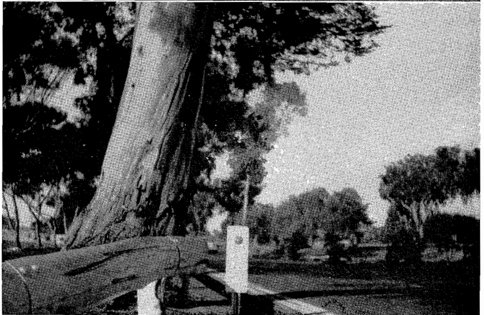
These photos show how guard rails prevented auto collisions with trees
