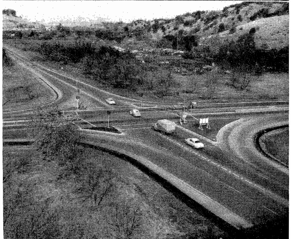
Two views of federal aid secondary county highway near Martinez. This section was constructed on a limited access freeway basis.
