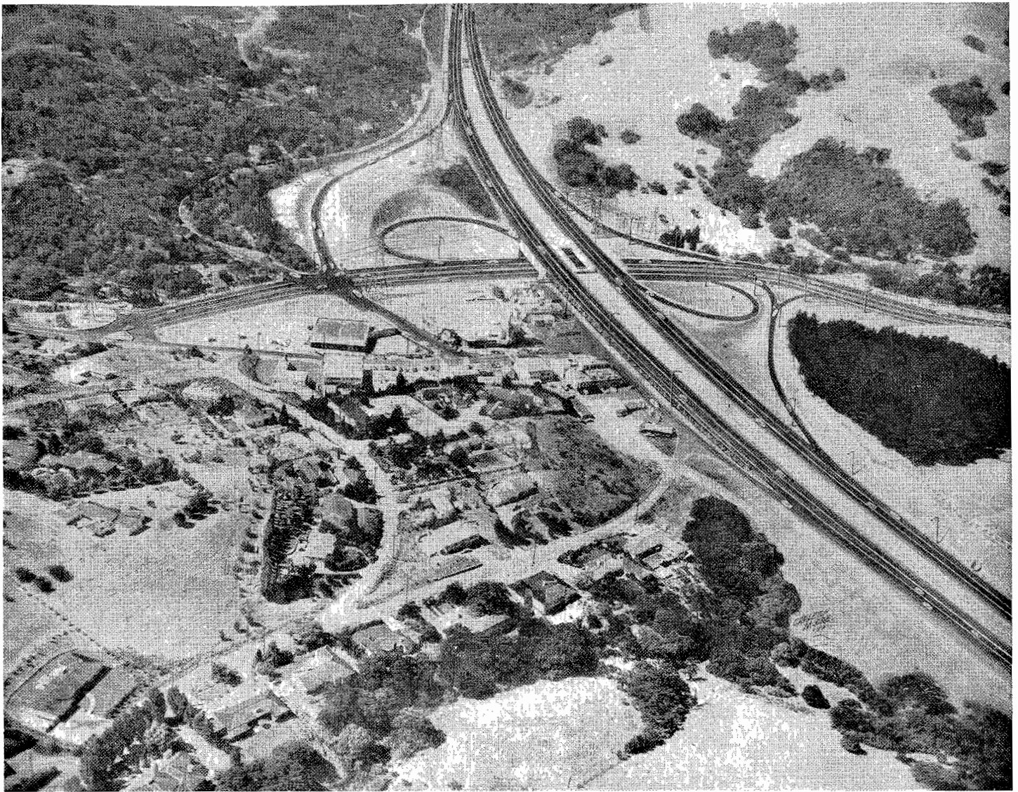
How the Orinda Cloverleaf will look when completed early in 1955. Carleton Moore, staff artist for the "Oakland Tribune," has, from careful study of construction plans, superimposed the interchange on an aerial photograph.
