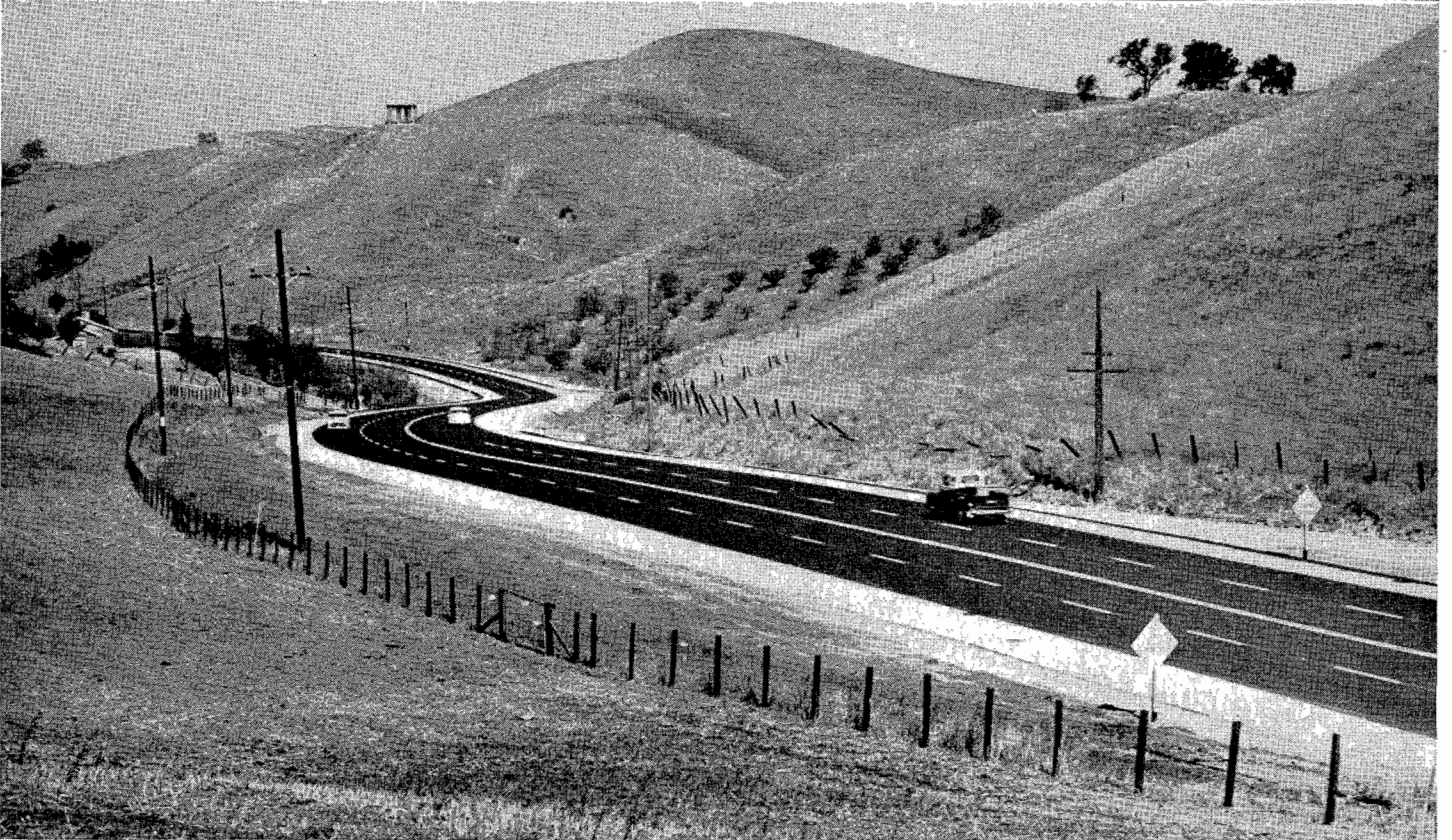
UPPER: Completed 40-foot-wide Pleasant Hill Road. Constructed by Contra Costa County as FAS and bond issue project. LOWER: Pleasant Hill Road in Contra Costa County following completion. Note four-lane passing section over summit.
