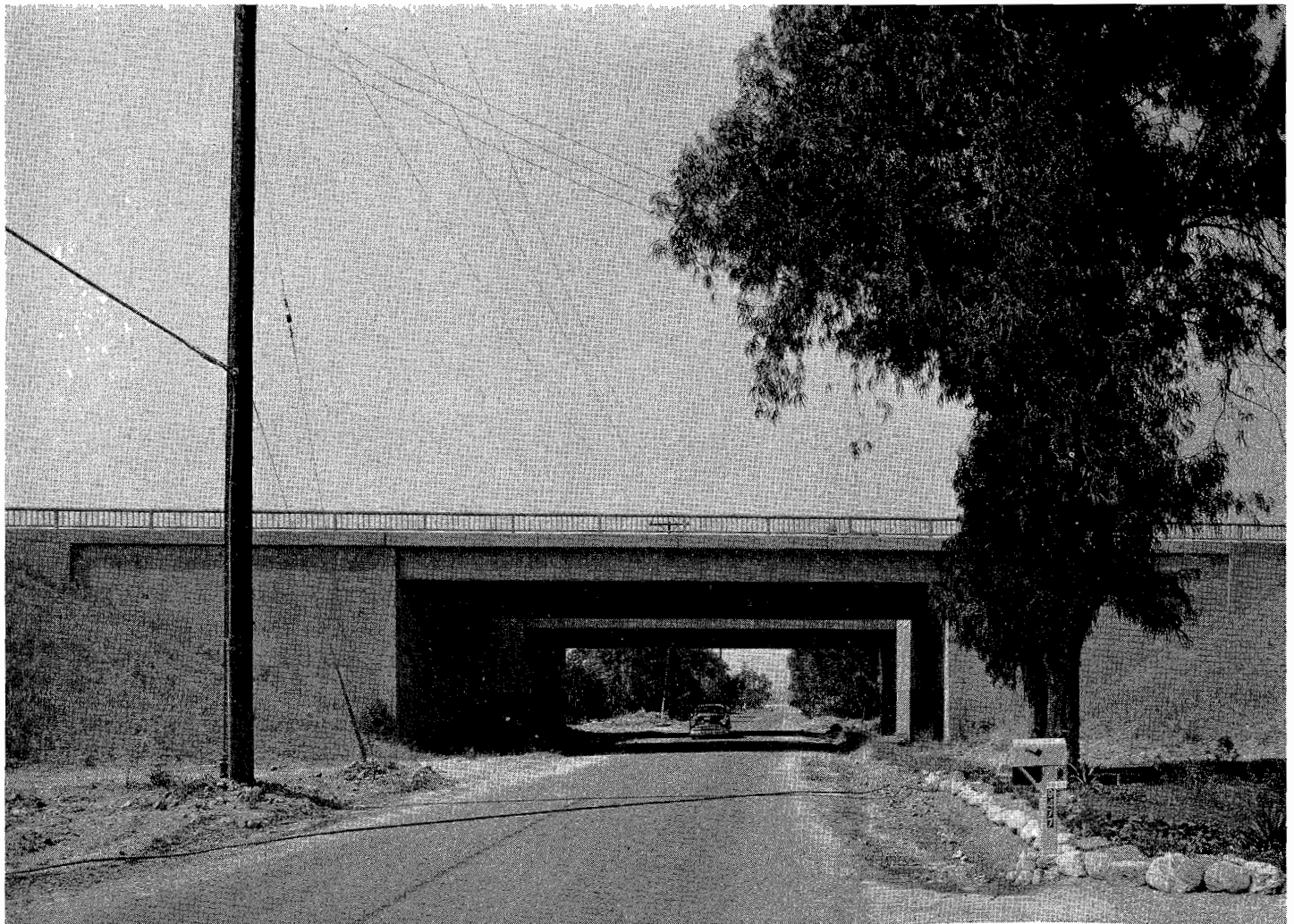
Freeway structure viewed from Monte Vista Avenue
