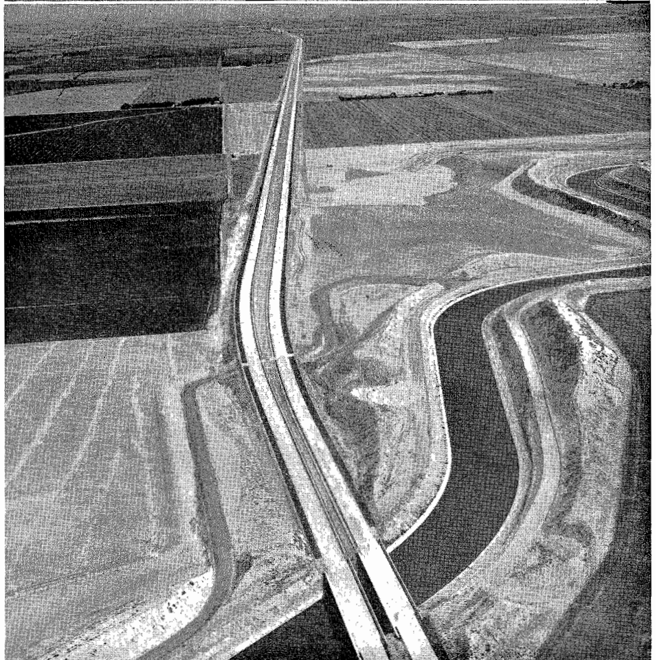
New Altamont-Tracy Expressway. UPPER: Mountain House interchange looking east. LOWER: Expressway crosses Delta-Mendota Canal, on right.
