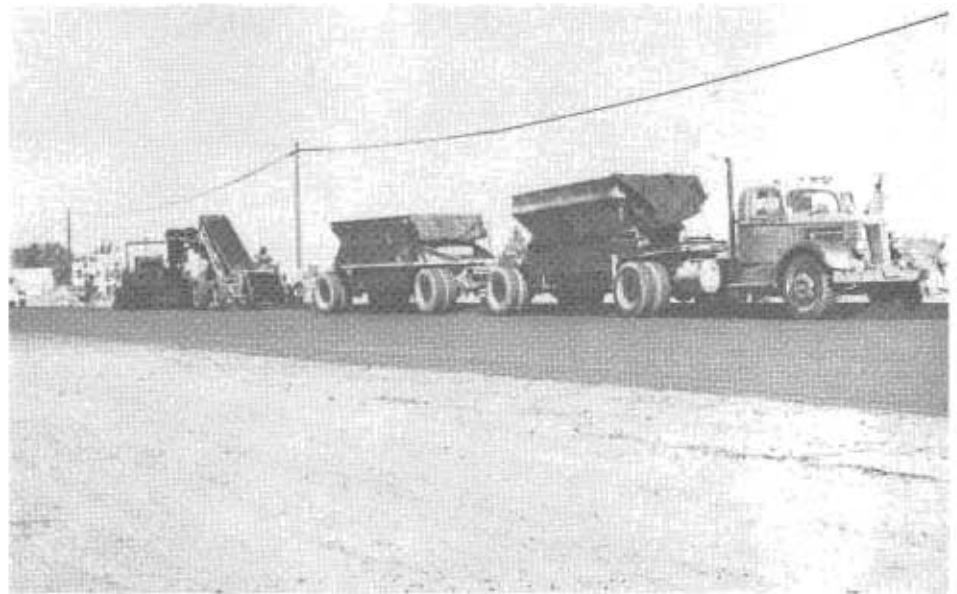
Equipment string for placing surfacing course
