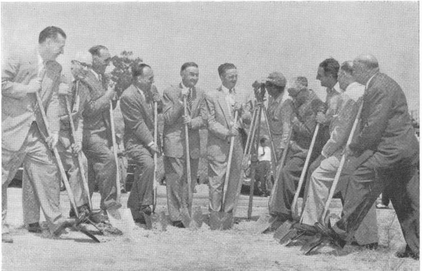
LEFT TO RIGHT: Councilman John Gibson, Assistant State Highway Engineer Paul O. Harding, Jack Yount, vice president of Vinnell Constructors, Inc., the contractors; Assemblyman Vincent Thomas; State Highway Commissioner Robert E. McClure; Howard Crandall, president of the Wilmington Chamber of Commerce; County Surveyor Burton Chace, E. R. Beck, president of the Harbor City Chamber of Commerce; Dr. E. C. Spires, president of the San Pedro Chamber of Commerce; and Harbor Manager Bernard Caughlin.
