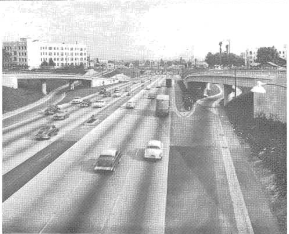
UPPER—Looking southeasterly along Hollywood Freeway from Sunset Boulevard overcrossing bridge. In center is shown the Van Ness Avenue Overcrossing. LOWER—Hollywood Freeway looking southeasterly from Hollywood Boulevard Overcrossing showing Hollywood Boulevard off-ramp overcrossing left and Hollywood Boulevard on-ramp on right.
