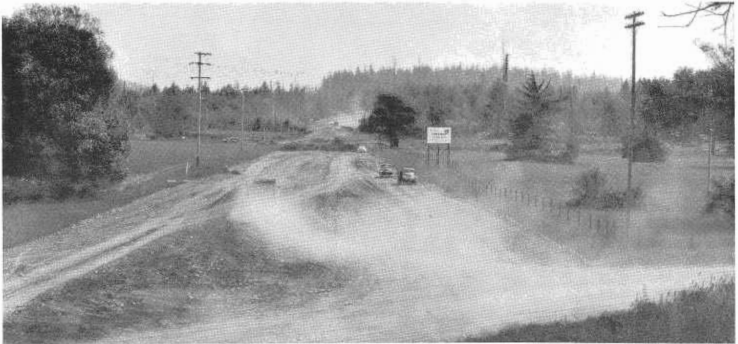
Looking south from the north end of project showing grading in progress on the only portion of alignment which was relatively clear of brush or trees. Clearing here involved only the removal of occasional stumps from approximately 3,000 feet of pasture land.
