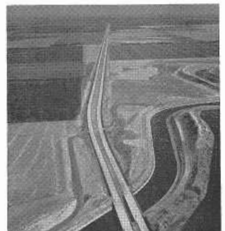
Expressway relocation of US 50 looking easterly toward Tracy, nearing completion. Delta-Mendota Canal of Central Valleys Project in foreground.
