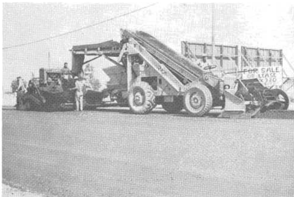
Loader and paver in operation on surfacing course
