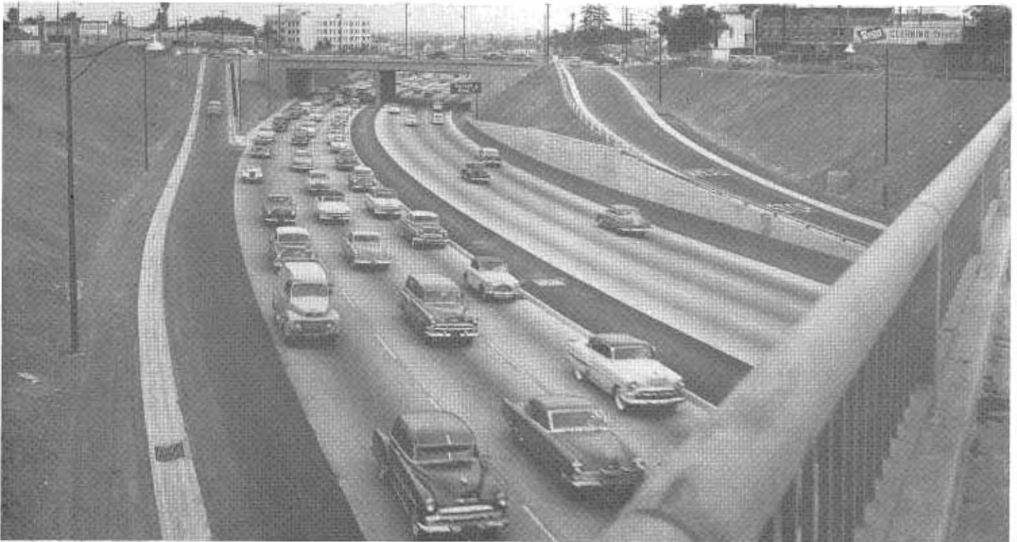
Looking southeasterly along Hollywood Freeway from Wilton Avenue Bridge showing Hollywood Boulevard Overcrossing
