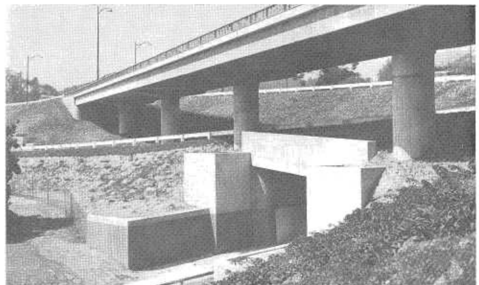
Looking northwesterly showing in foreground Ivar Street underpass with Cahuenga Boulevard eastbound on-ramp over it and with the Franklin Avenue off-ramp above. This constitutes a three-level interchange.
