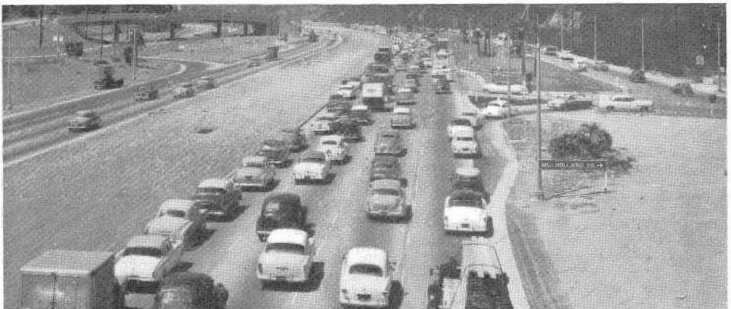
View looking northerly along Hollywood Freeway from Pilgrimage Bridge showing Highland off-ramp overcrossing center left. The cleared space between the two main freeway roadways is the strip of land 48 feet wide recently acquired from the Pacific Electric Railway after abandonment and track removal. This additional area will be available for future freeway improvement as needed.
