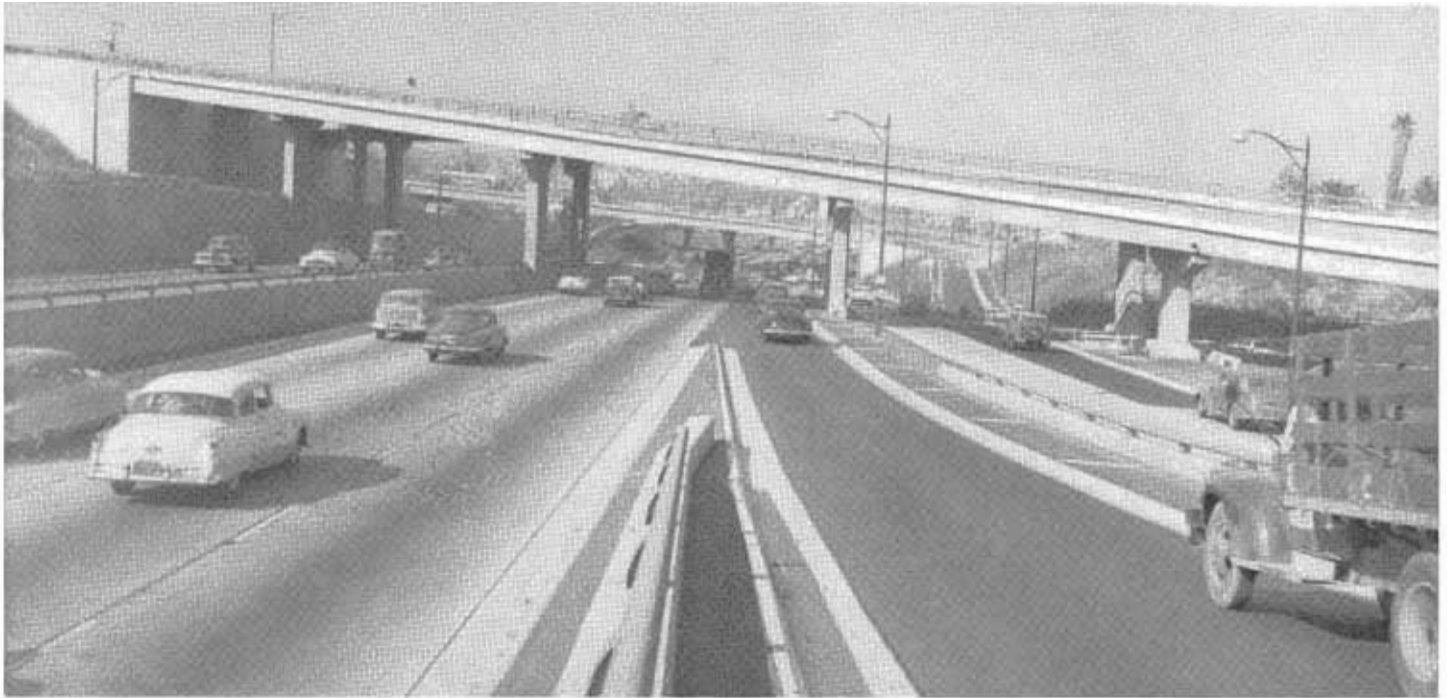
Looking northerly along completed Harbor Freeway, showing normal traffic use. The two bridges in foreground are for Fourth Street traffic. When cooperatively financed $1,400,000 construction contract now in progress has been completed for extending Fourth St. from Flower St. to Hill St., Fourth St. and Third St. will be put into operation as a pair of one-way streets similar to the one-way operation of Fifth and Sixth Sts., and Eighth and Ninth Sts.
