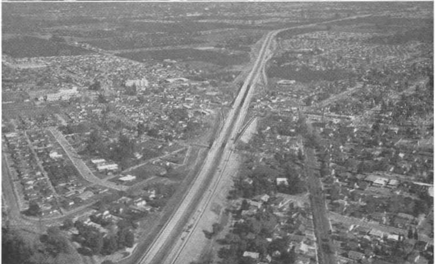
UPPER—Looking northerly, showing portion of San Bernardino Freeway with combination grade separation structure spanning over Garey Ave., State Sign Route 71, McKinley Ave. and Orange Grove Ave. LOWER—Looking easterly from above Los Angeles along San Bernardino Freeway with construction activities shown in foreground of Oberg Bros. Construction Company for widening bridge over Los Angeles River and Charles MacClusky for traffic interchange structure to take westbound motorists from San Bernardino Freeway southbound on Santa Ana Freeway.
