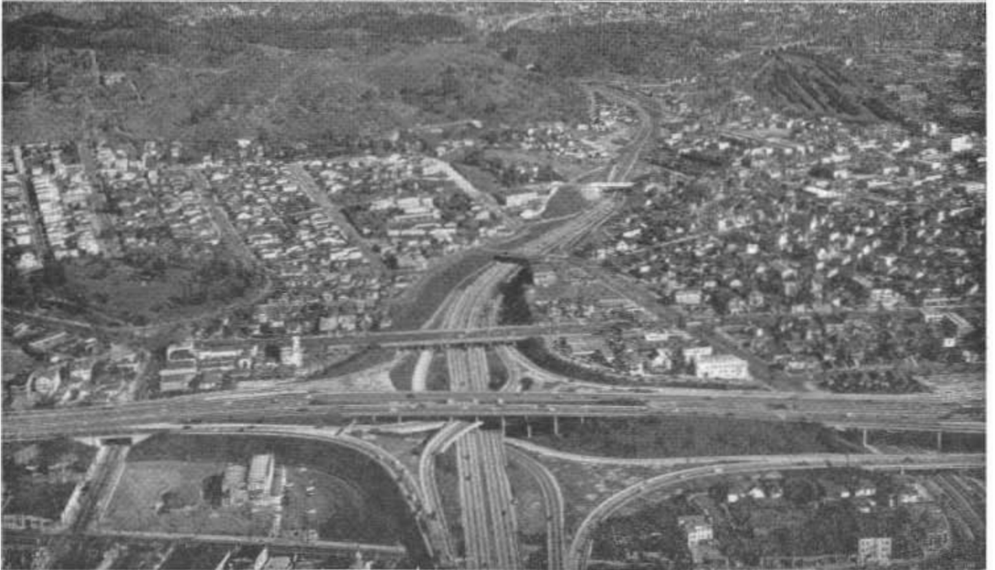
UPPER—Looking southerly from above Los Angeles along Pasadena-Harbor Freeway. Sunset Boulevard over Pasadena Freeway shown in foreground center. Four-level traffic interchange structure shown in foreground, with Hollywood Freeway extending from left to right. Portion of downtown Los Angeles business district shown above center left. LOWER—Looking northerly from above Los Angeles along Pasadena Freeway. Hollywood Freeway and four-level traffic interchange structure shown foreground, with City of Pasadena in background.
