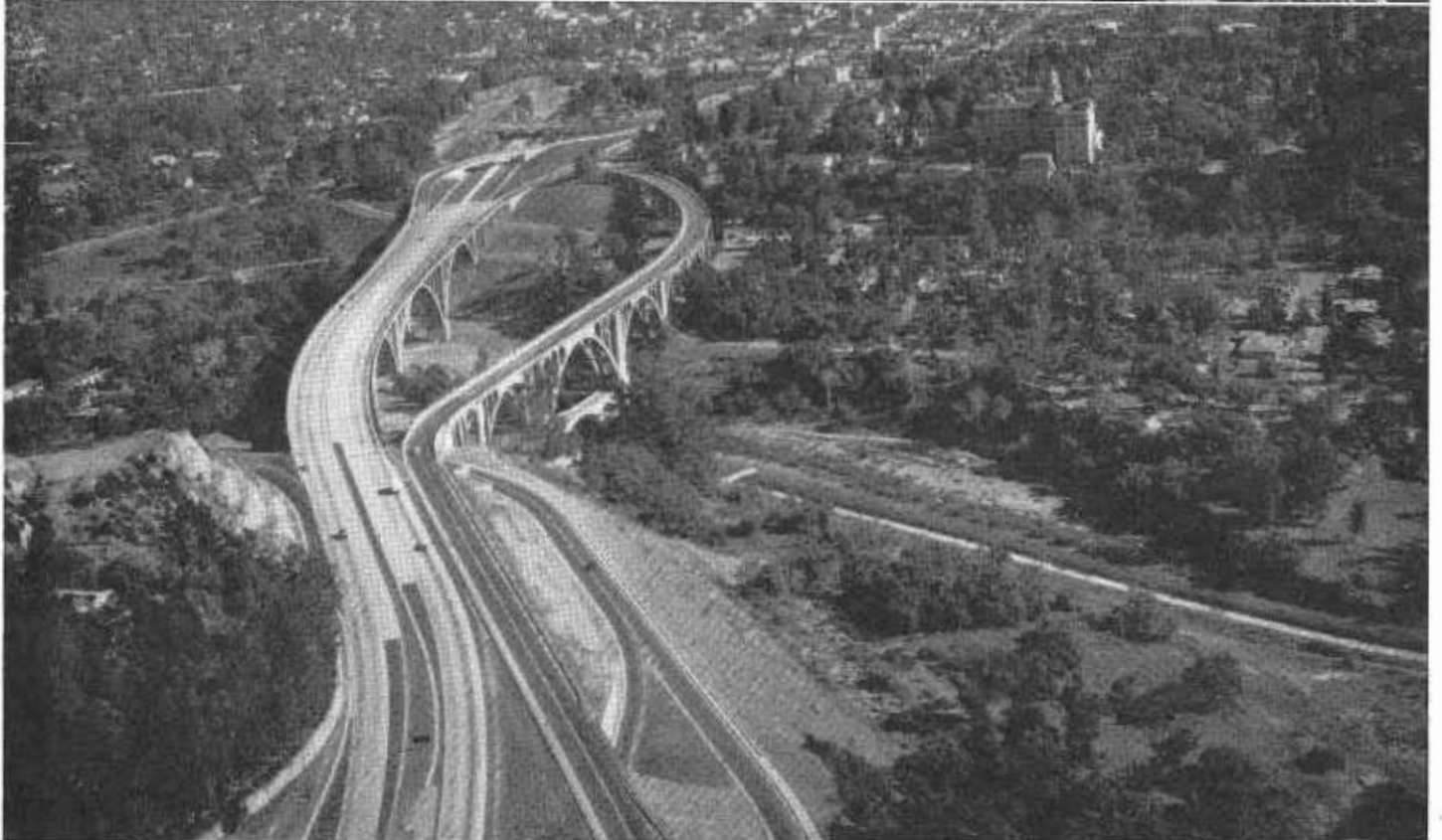
UPPER—Looking southerly along Pasadena Freeway, showing Arroyo Seco storm drain channel foreground right, bridges crossing Los Angeles River in center. In center background is Bishops Road disposal area where state contractors, at considerable saving to the State, have hauled in some 5,000,000 cubic yards of excess excavation encountered on nearby freeway projects. In the foreground is shown area that will be traversed by future Golden State Freeway that crosses the Pasadena Freeway at approximately right angles. LOWER—Looking easterly along Colorado Freeway showing "Pasadena Pioneers Bridge" over Arroyo Seco on left and Old Colorado Street Bridge on right, with Pasadena Civic Center and business district in background.
