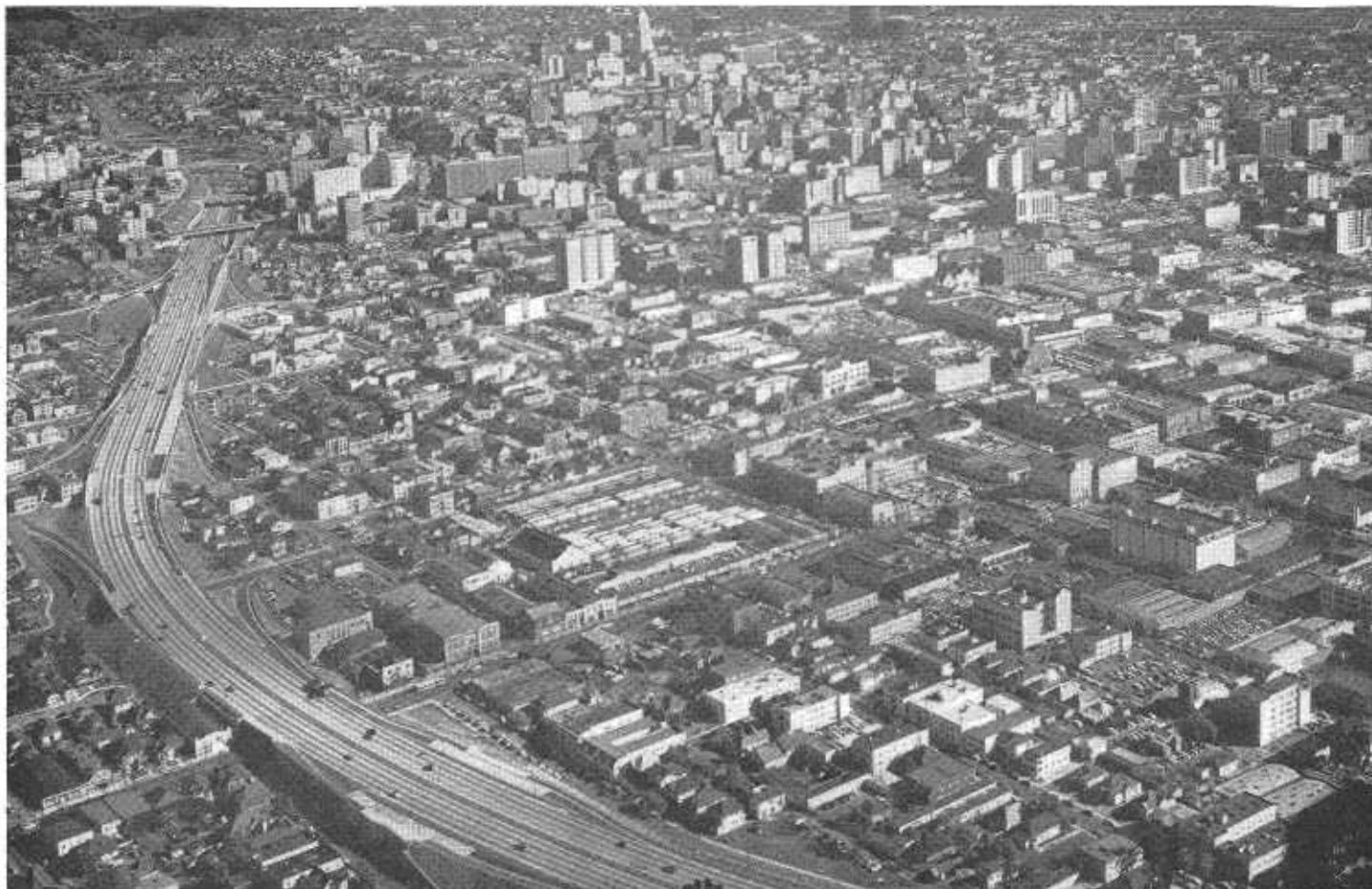
Looking northerly along completed Harbor Freeway from above Los Angeles showing downtown business buildings and Civic Center buildings in center and toward background. The grade separation bridge, foreground left, carries Pico Blvd. under the Harbor Freeway. The four-level traffic interchange structure and Hollywood Freeway are shown background left.
