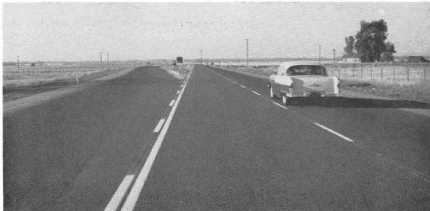
View of section of relocated portion of US 99E between Oroville Wye and Chico
