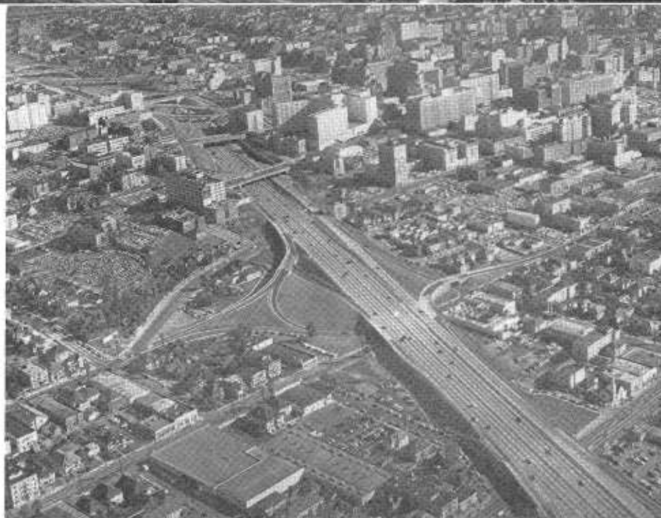
Looking northeasterly from above Los Angeles showing completed portion of the Harbor Freeway extending from foreground right to center left. Downtown business district and Civic Center shown center and right. The grade separation bridge, foreground right, carries Olympic Blvd. under the Harbor Freeway. Next above Olympic Blvd. is Ninth St. that carries one-way traffic eastbound, and above it is Eighth St. which carries one-way traffic westbound.
