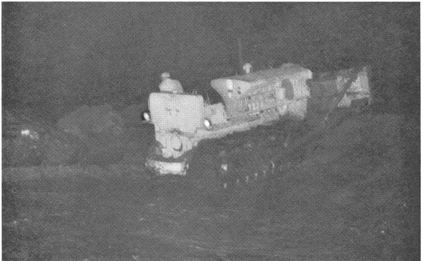
D8 dozer excavating for toe rock
