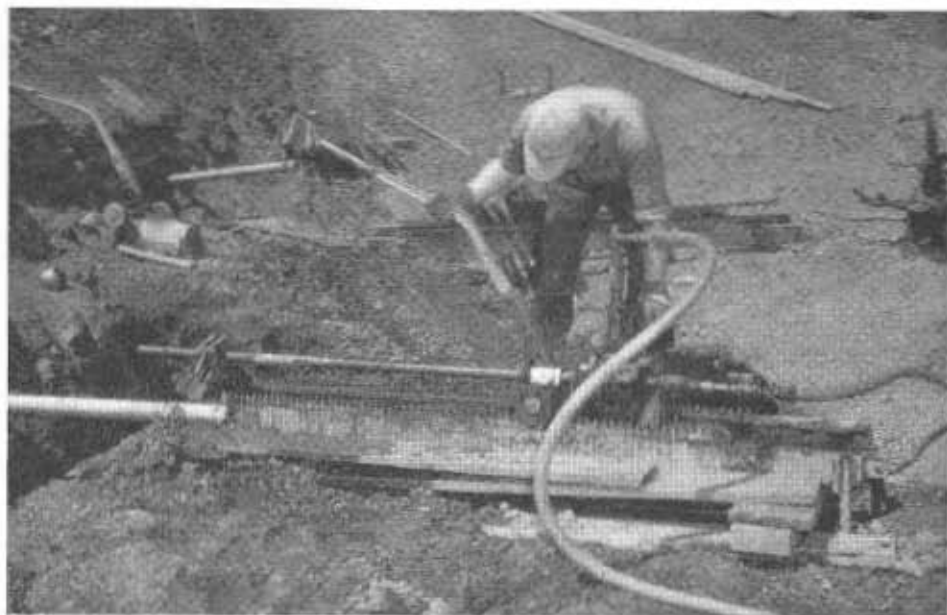
Hydrauger drill in operation
