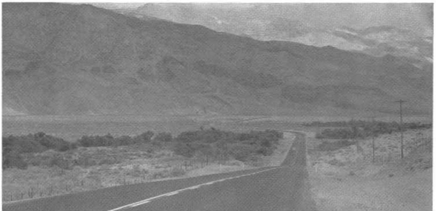
Looking easterly. Owens River Bridge in middle distance. Old road to left and new alignment to the right in background.
