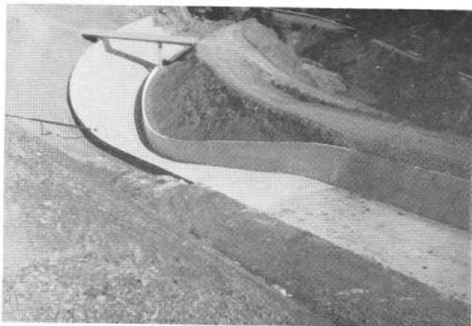
View of completed spillway extension
