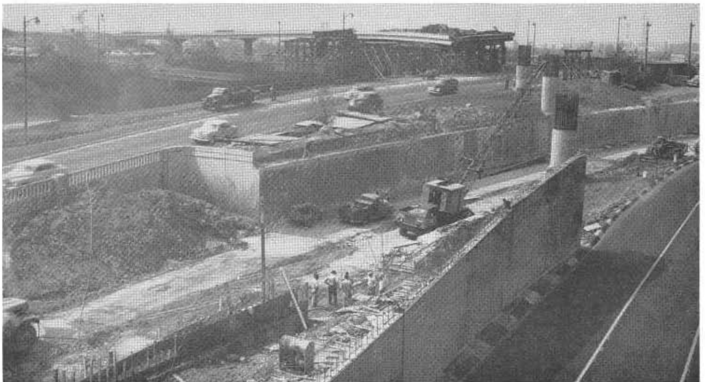
General view of the separation as seen from Macy Street Overcrossing
