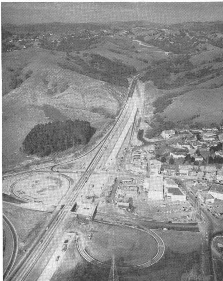
View of final stage of construction of the Orinda interchange
