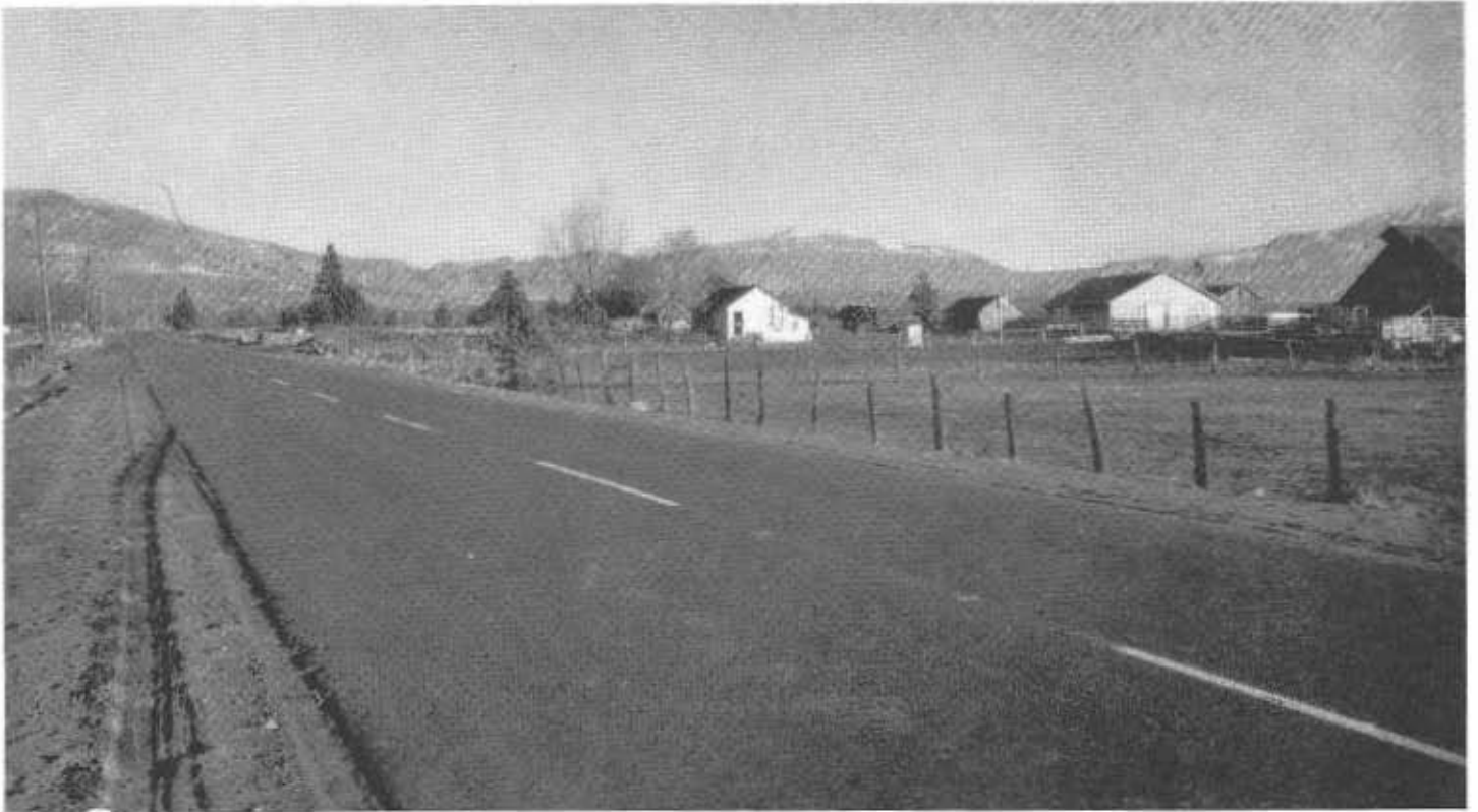
View of recently completed FAS Route 1166, in Siskiyou County, showing typical farm area served
