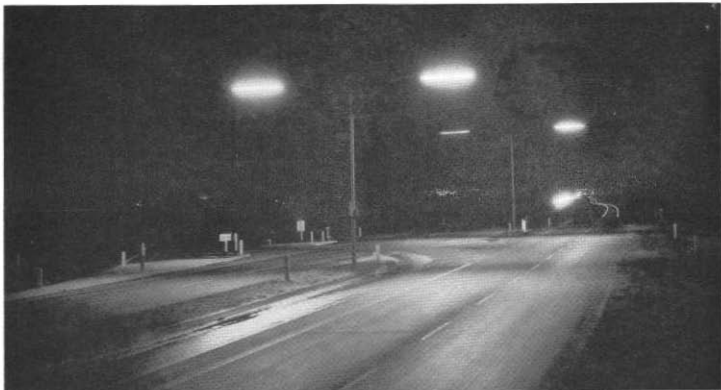
Night view on US 101 in Arcata during wet weather, showing broad band of light across intersection and its approaches provided by the new-type luminaire
