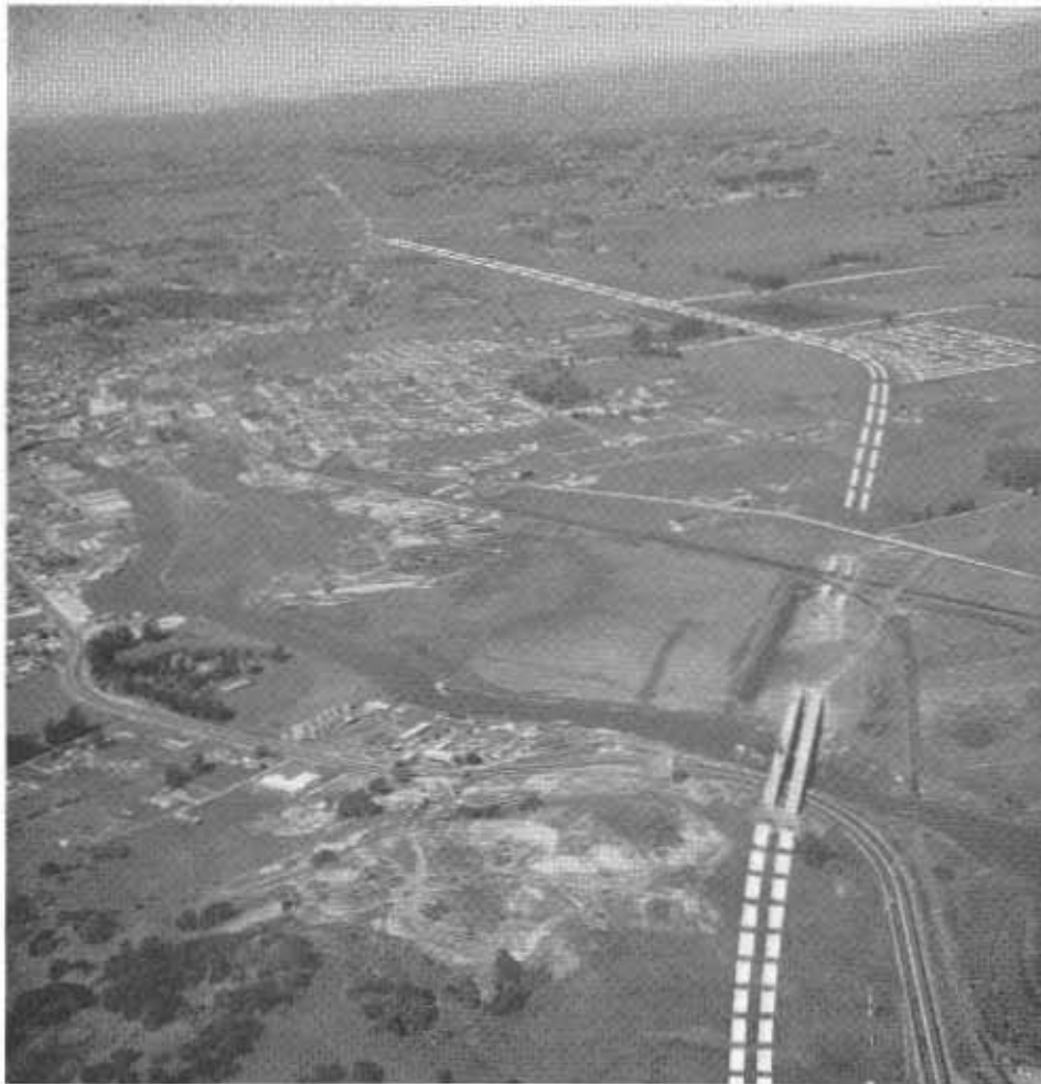
Route of the freeway bypass of Petaluma where operations are under way on two contracts for the structures and roadwork for the new facility
