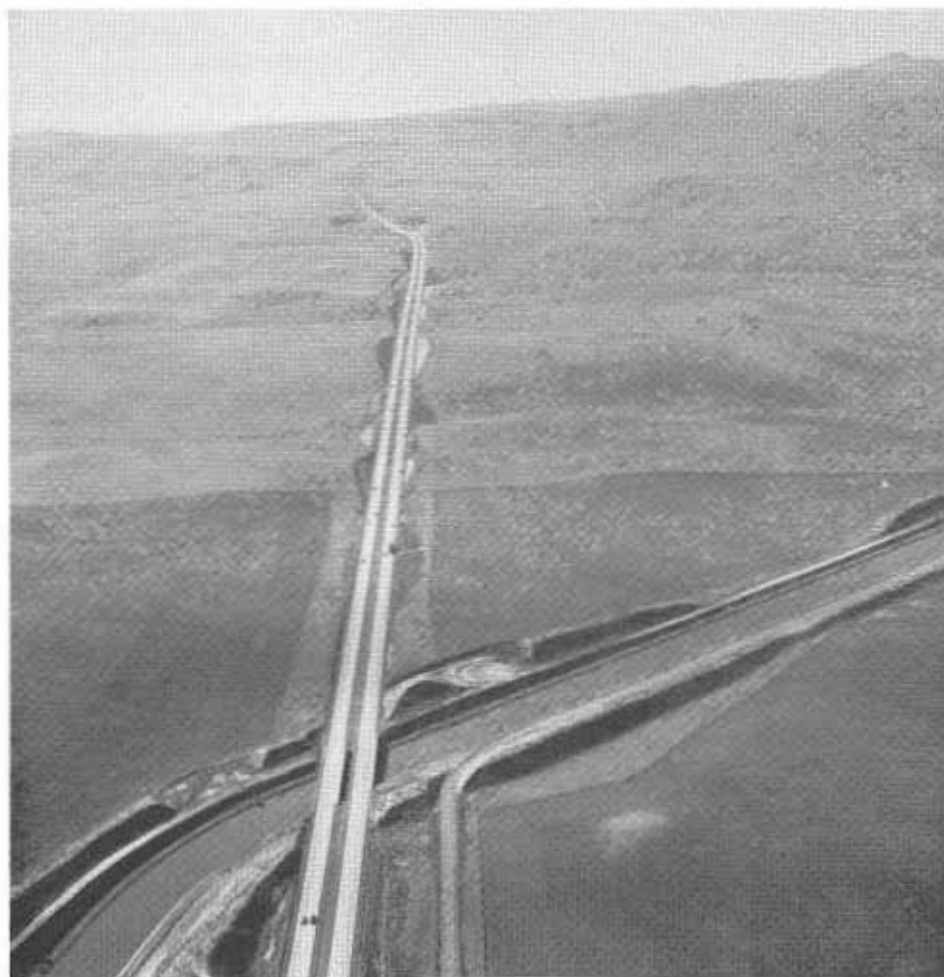
Expressway on US 50 at crossing of the Delta Mendota Canal near the Alameda-San Joaquin County line. New construction joins with the original four-lane divided facility through the Altamont Pass in the distance where the ramps of an interchange are discernible.
