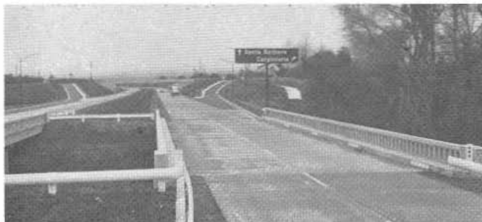
Looking west. Carpinteria Creek Bridge in foreground and on-and off-ramps for Carpinteria connecting to Casitas Pass Bridge.
