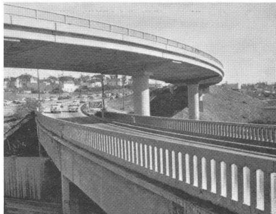
Prestressed span over the eastbound Santa Ana Freeway bridge and the on-ramp for the eastbound San Bernardino Freeway below, showing the three-level separation at this point. View also shows bottom flanges of the prestressed girders and the general shape of the girder step bearings.
