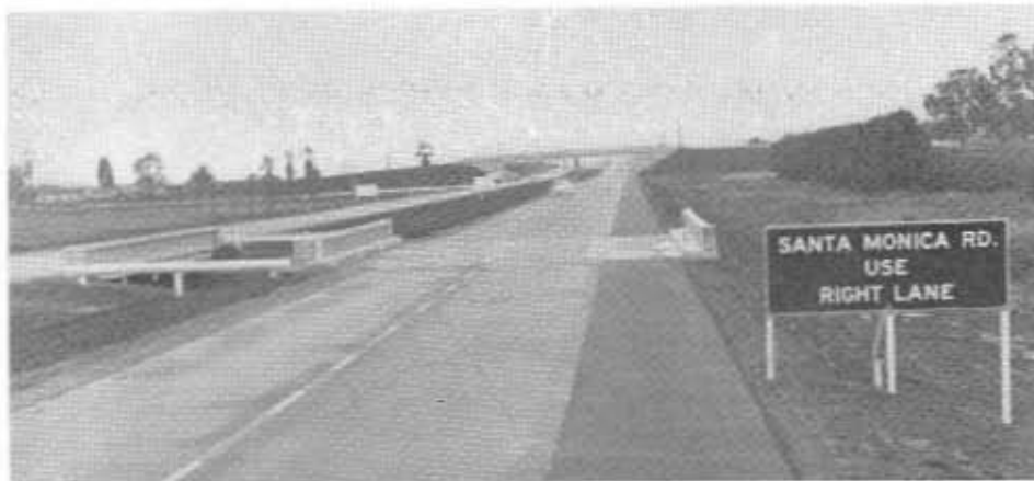
Looking west on Carpinteria Freeway. Franklin Creek Bridge in foreground and Seventh Street Overpass in background.
