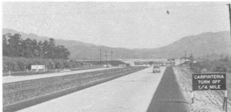
Carpinteria Expressway, looking east. Seventh Street Overpass in background.
