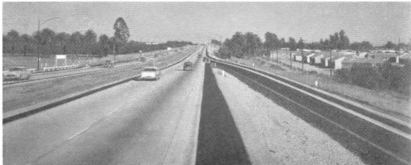
Traffic flows smoothly through the Claremont area, where the freeway is bordered by orange groves, subdivisions and palm trees. Note gentle rise and dip of freeway grade. View is east from Alexander Avenue.
