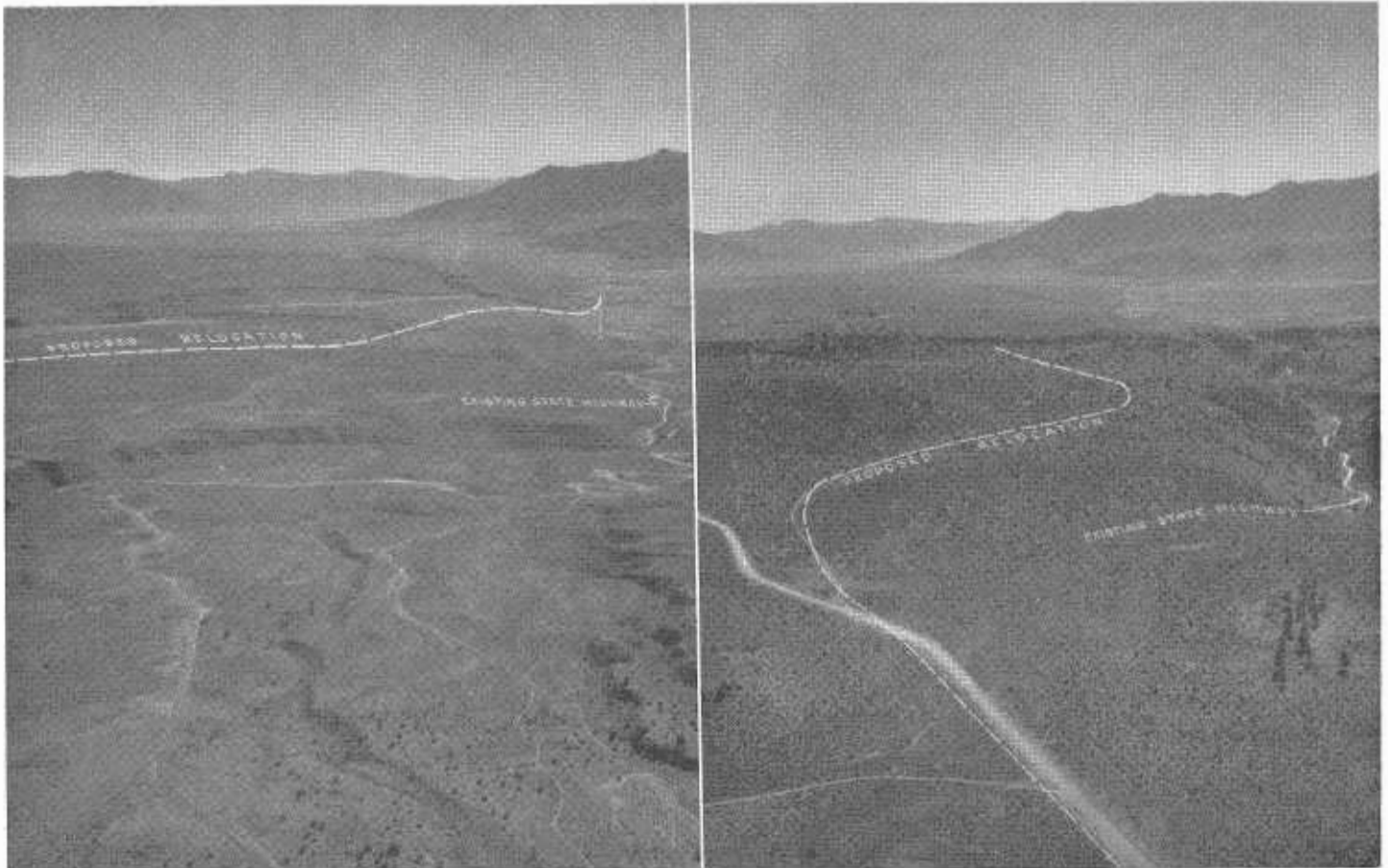
LEFT—Sherwin Grade, looking south. Dotted line shows proposed relocation. RIGHT—Upper East Mesa, looking south. Proposed relocation to the left; existing State highway on right.
