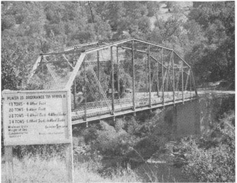
A new bridge downstream constructed by Placer County under the Federal Air Secondary Highway Program replaced this narrow steel truss bridge which served the Foresthill area between 1911 and 1955
