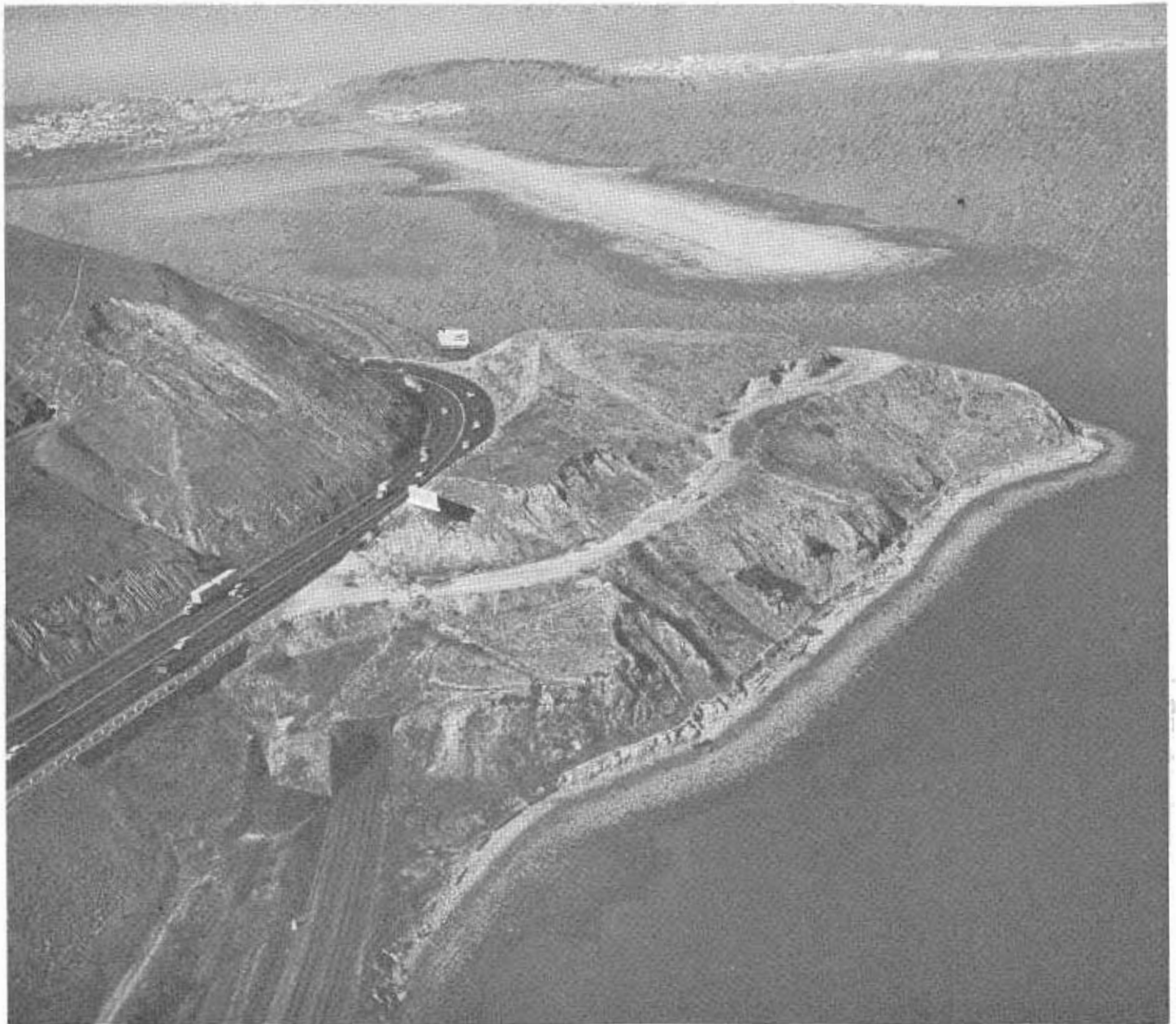
View of open water section of fill for Bayshore Freeway across Candlestick Cove, Sierra Point in foreground. Both railroad and highway will be relocated across the Point to the right of existing facilities. Purpose of railroad relocation is to provide additional tracks. Freeway will be carried over railroad on structure on solid ground at Sierra Point.
