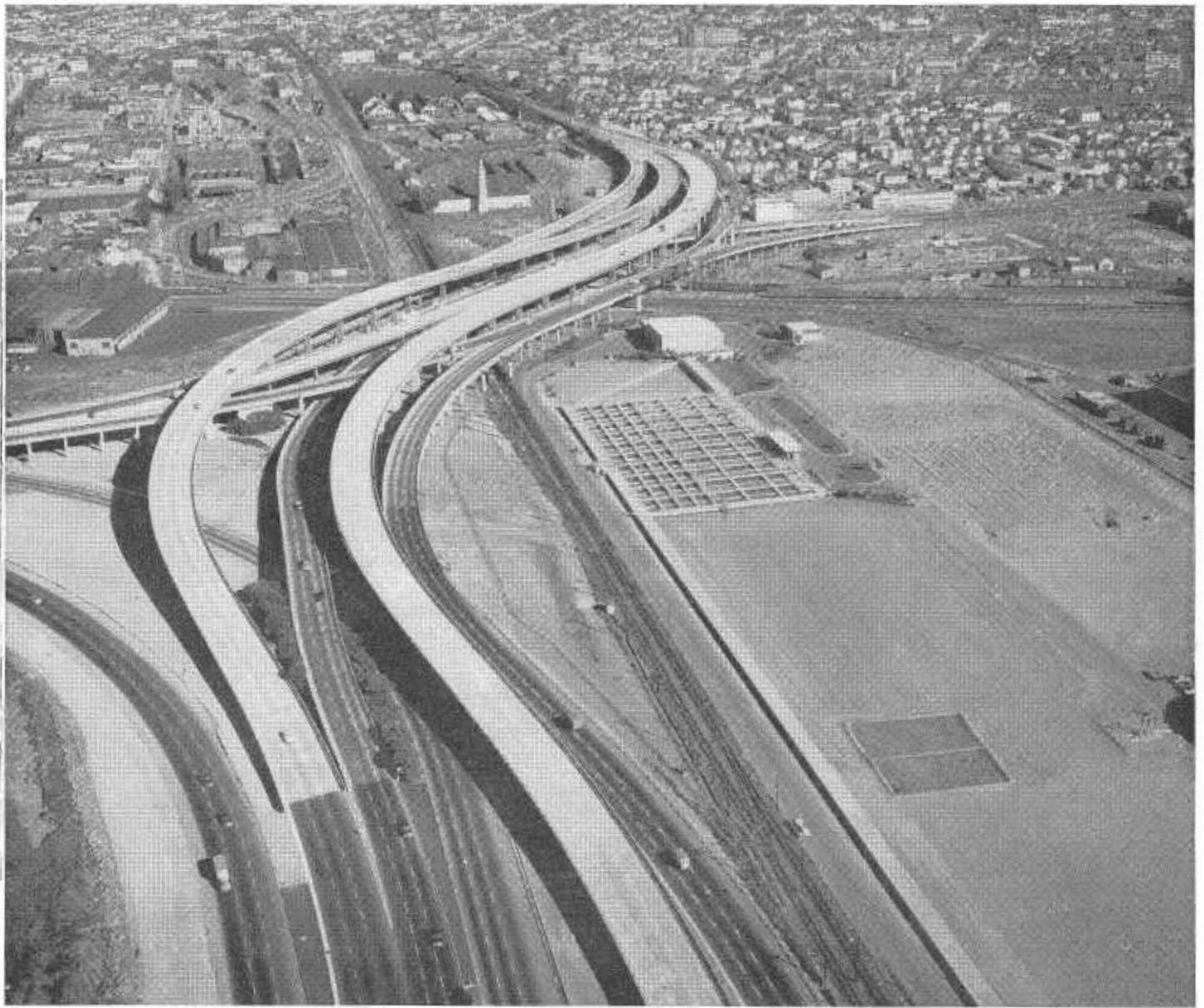
View looking easterly, showing East Bay distribution structure as reconstructed
