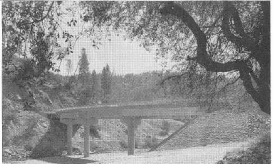
Two different views of the new bridge across the North Fork of the American River in Placer County
