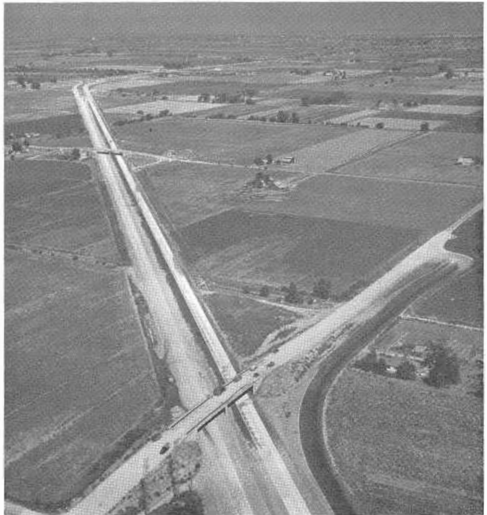
Aerial view of Manteca Freeway, looking south, showing Cottage Avenue and Louise Avenue separation structures
