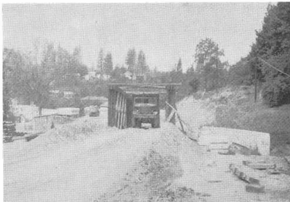
This photograph shows the Camino, Placerville and Lake Tahoe Railroad truss that was salvaged and used to span a highway grade separation structure to permit the use of over-legal loads during construction
