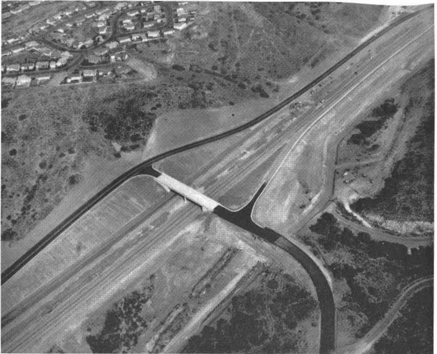
Sign Route 94, 56th Street separation near east city limits of San Diego, with new subdivision development in area.
