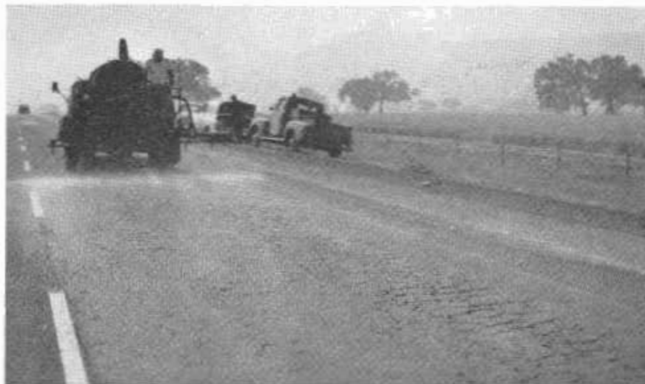
Watering the pavement
