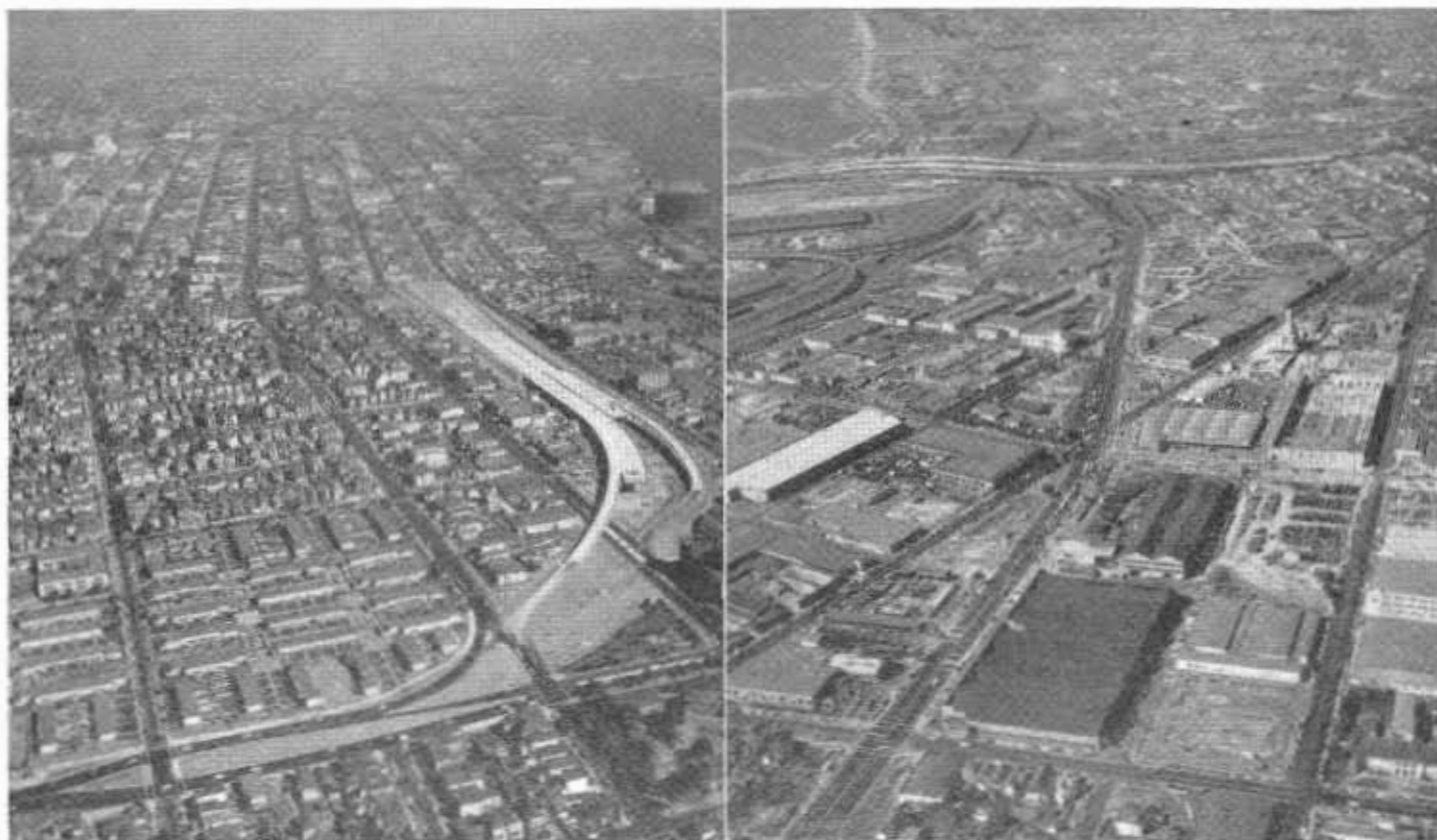
LEFT—New unit of Eastshore Freeway extending from 11th and Cypress Street to Market Street in Oakland. RIGHT—Construction has started on a major project along Cypress Street that includes a double-deck viaduct from the Distribution Structure of the Bay Bridge southerly to 16th Street.
