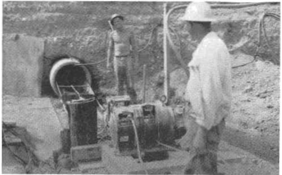
Sled and trigger winch used in removing excavated material
