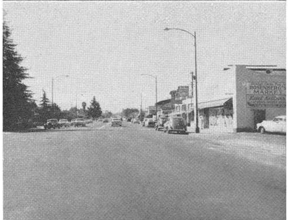
UPPER—Lincoln Avenue between Brace and Minnesota, looking south, before improvement.
