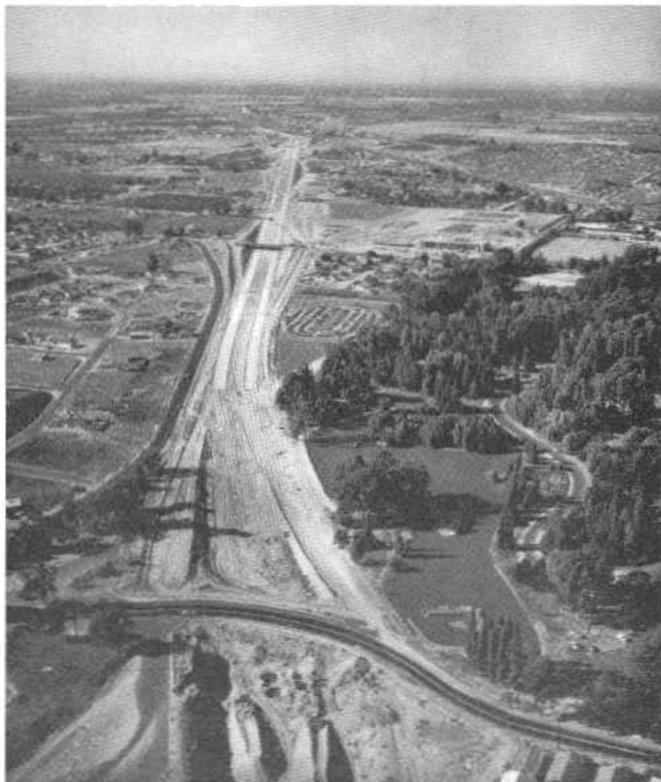
Looking north on Fresno Freeway, showing construction
