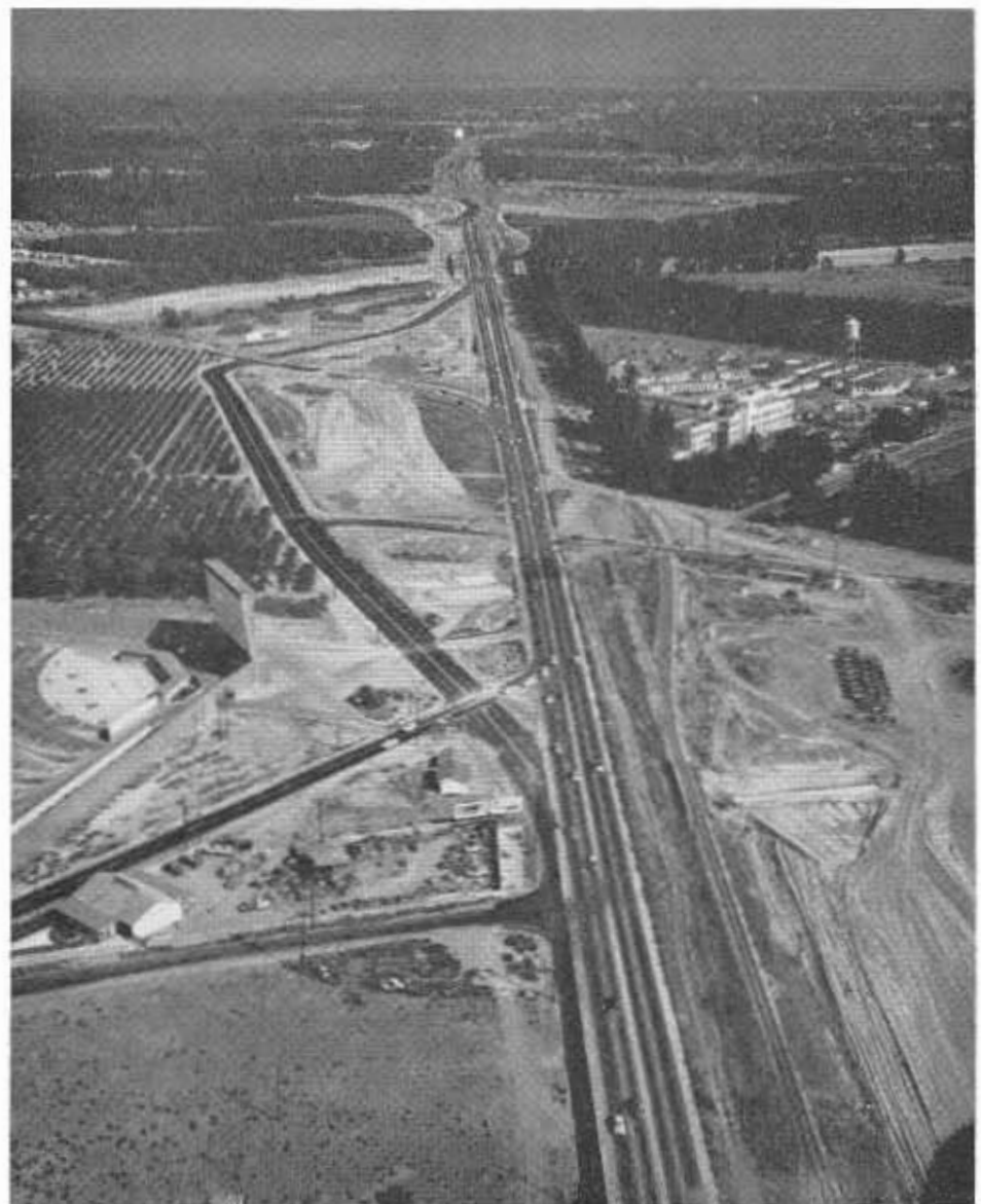
Looking southeasterly along construction in progress on Santa Ana Freeway with the site of the Chapman Avenue Traffic Interchange System shown in center. Orange County Hospital buildings are shown center right.
