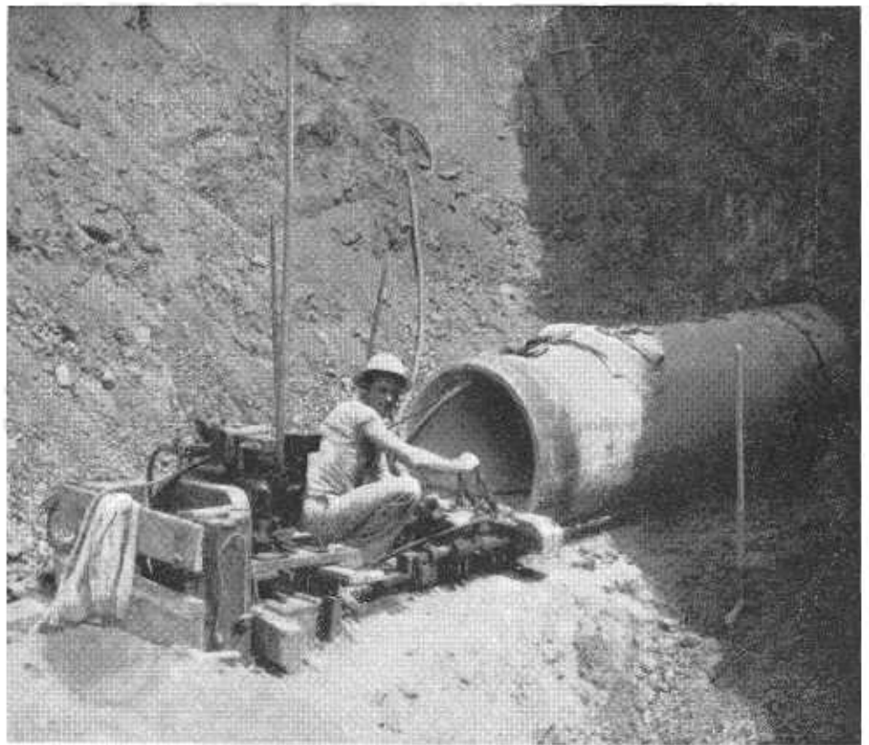
Jacking operation at Kellogg Hill
