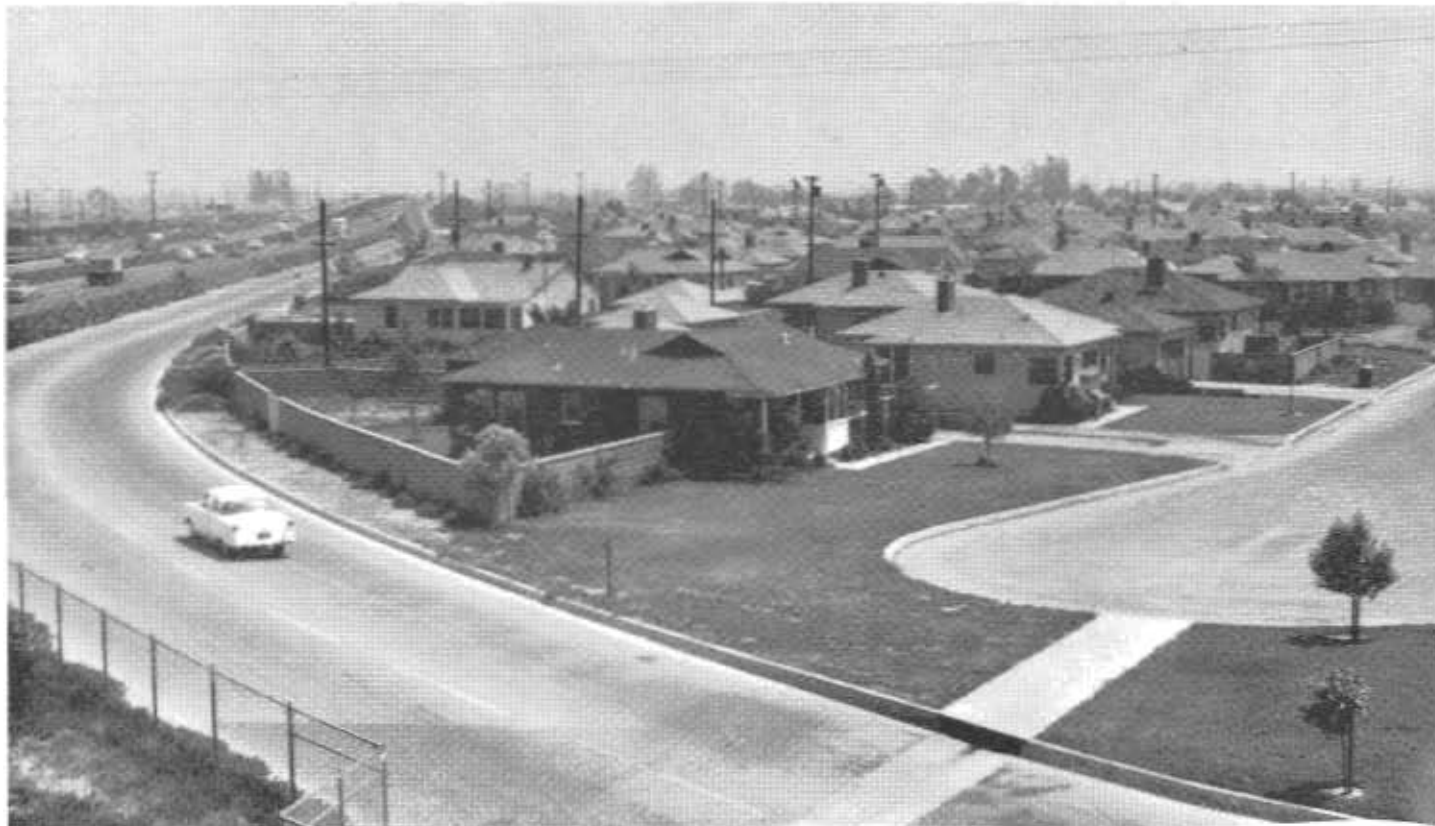
Looking southeasterly showing new homes built within last three years adjoining Dallison Drive between Florence Avenue from which this photograph was taken and the Southern Pacific Railroad over which grade separation bridge on Santa Ana Freeway is shown in background, left
