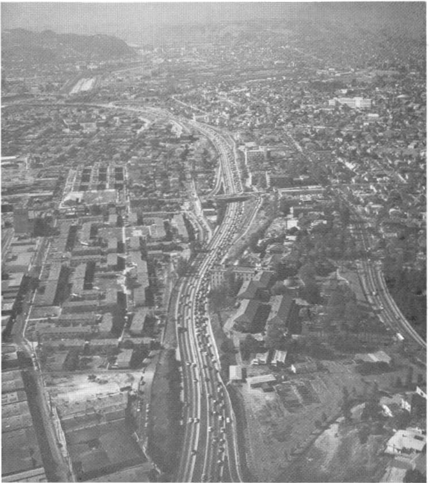
Looking northerly along Santa Ana Freeway in East Los Angeles area from above Sixth Street, showing Fourth Street Overcrossing in center
