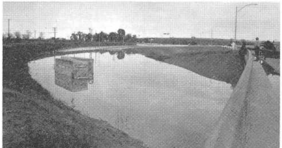
Flooded Visalia Airport Interchange, Tulare County
