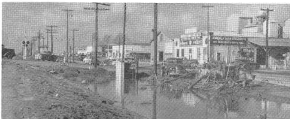
Pumping equipment set up in Chowchilla
