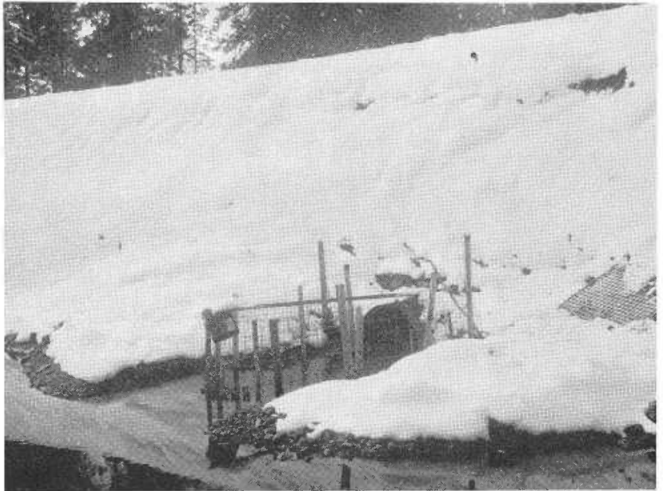
Creosote bucket still on fence. Joe had the water about two feet over the pipe.
