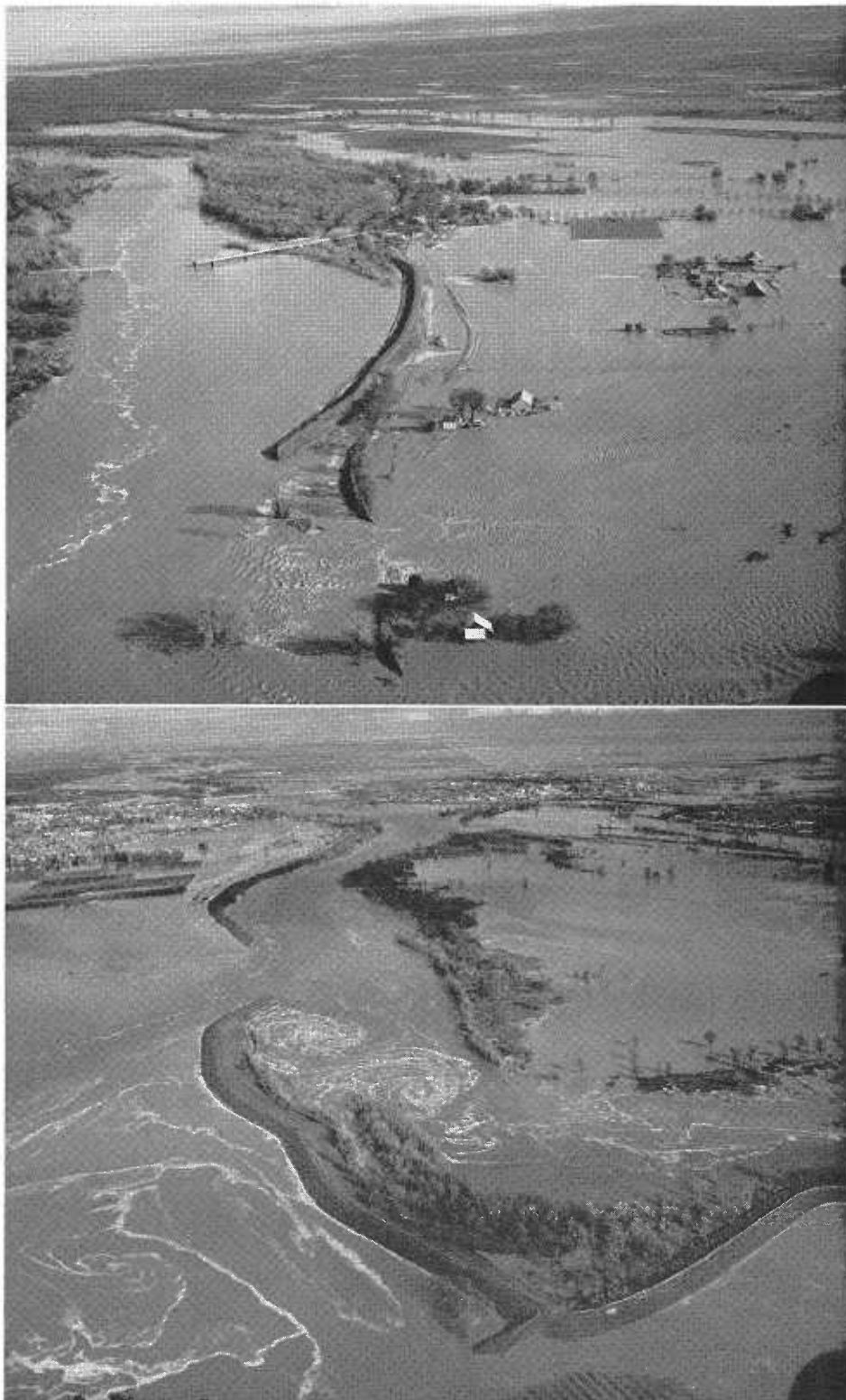
TOP—Break in Feather River levee at Nicolaus. BOTTOM—Break in Feather River levee south of Yuba City, Sutter County.
