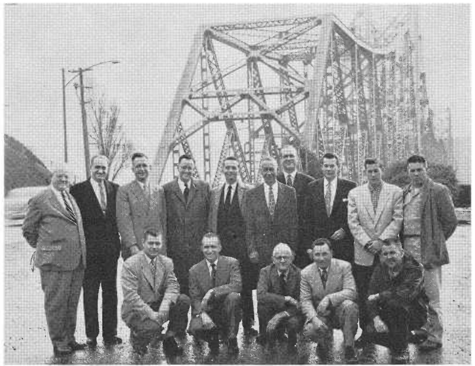
Contractors and resident engineers gathered at the site of parallel Carquinez Bridge to discuss start of project.
