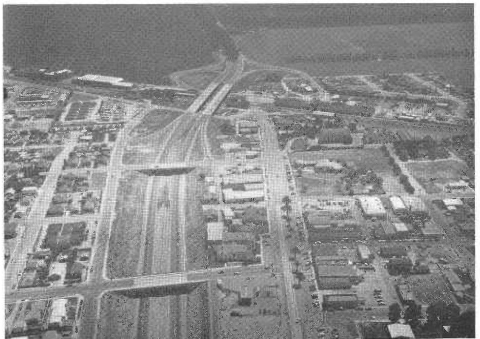
Looking east along Ventura Freeway through Camarillo
