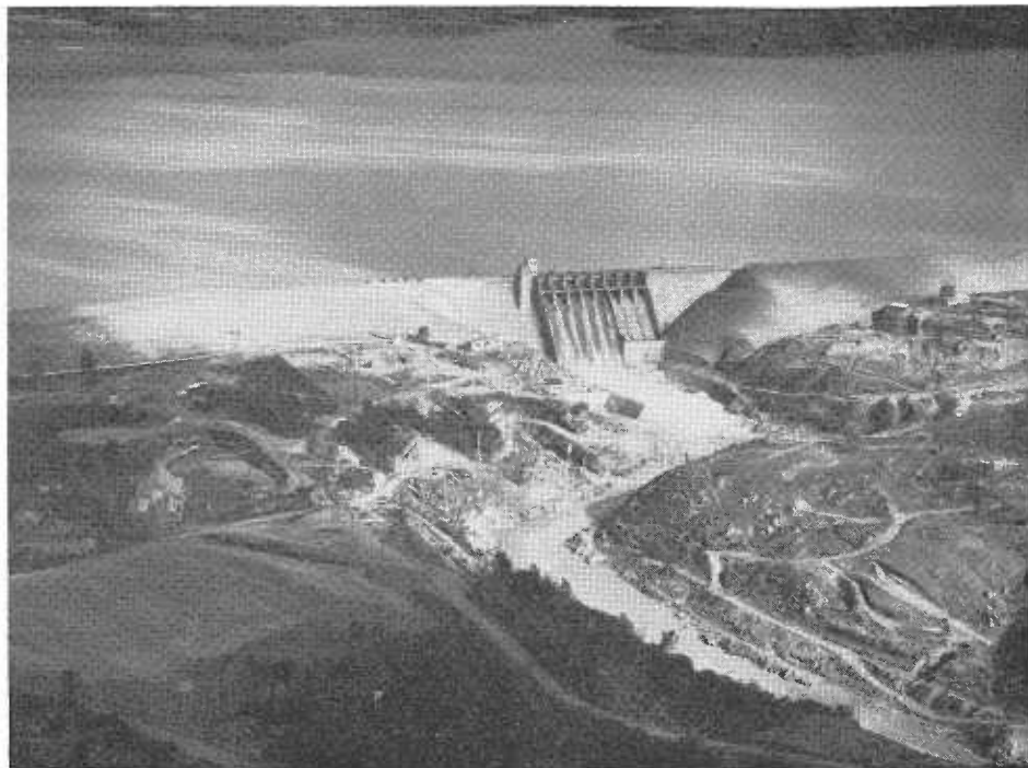
TOP—Folsom Dam and Reservoir on December 24, 1955 (Corps of Engineers Photo).
