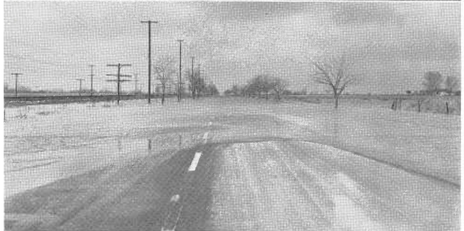
UPPER—Flooded section of US 99 through Chowchilla, Madera County. LOWER—US 99 flooded south of Chowchilla.
