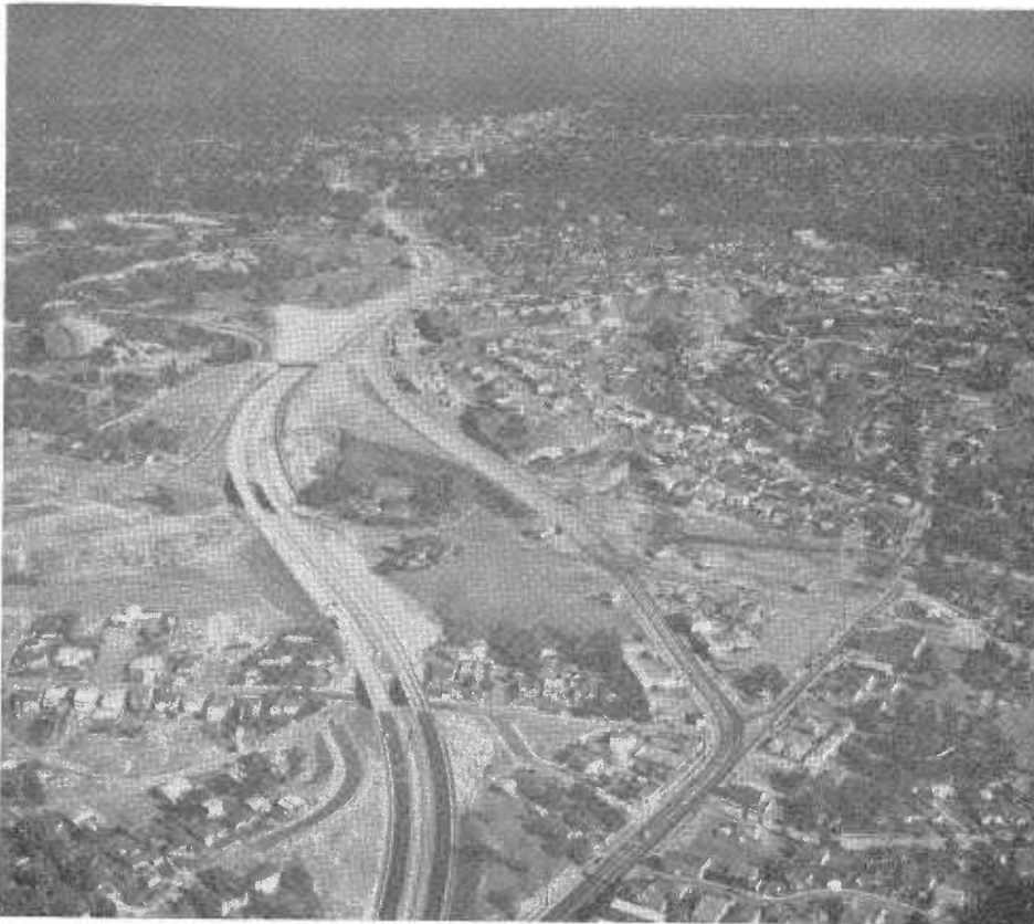
Looking east along recently completed Colorado Freeway. Eagle Rock, center left. Pasadena, center background.
