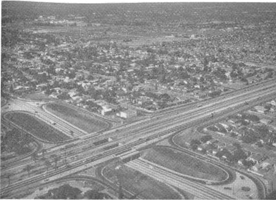
Looking northeasterly, showing completed San Bernardino Freeway over Garfield Avenue
