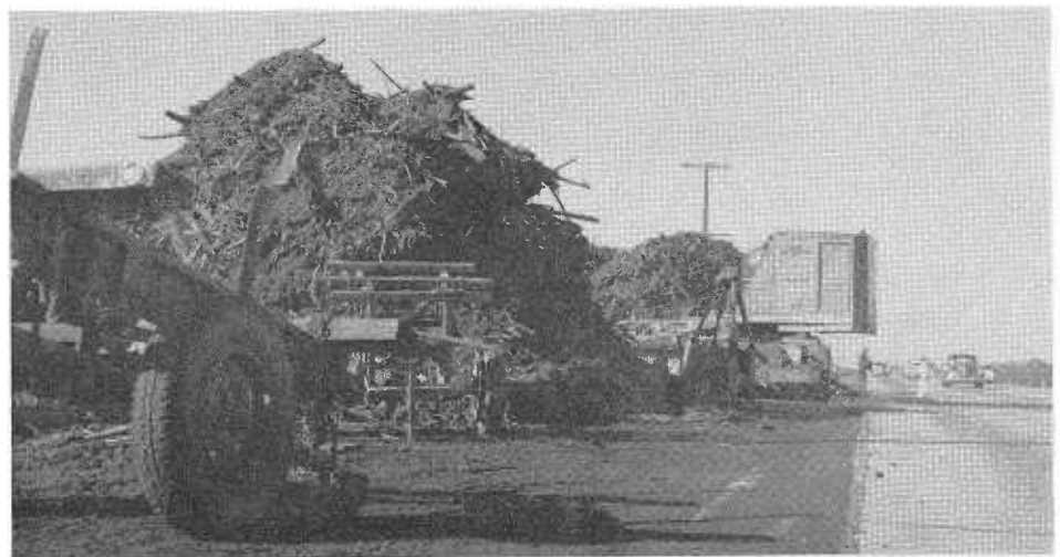
Debris removed from entrance of single span Saratoga Creek Bridge north of Santa Clara. Clogging flooded Bayshore Highway, US 101 Bypass.
