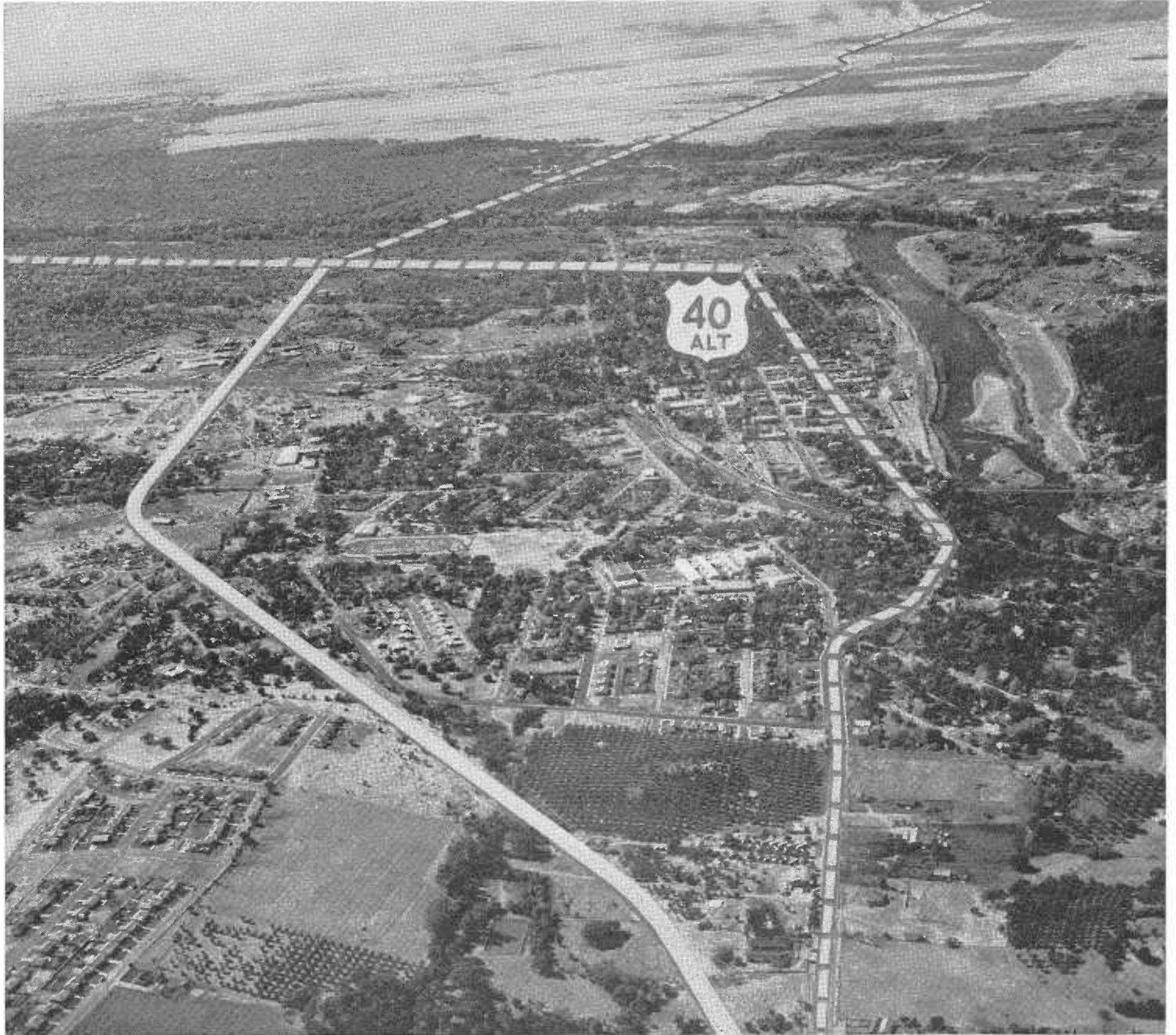
Looking westerly along FAS 1169 on the left and US 40 Alt. diverging to the right, which intersect again in background near the Feather River Bridge south of Oroville. Bridge at right center is on S. H. Route 87 to Chico.
