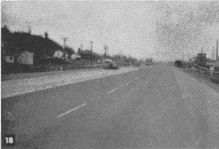
PHOTO No. 16. Showing delineation effect of O. G. PMS, also treatment of intersection areas as regards placement of O. G. PMS. PHOTO No. 17. Showing delineation effect of O. G. PMS on Highway US 101 north of Crescent City. PHOTO No. 18. Another photo showing delineation effects of O. G. PMS blanket on US 101 north of Eureka. PHOTOS Nos. 19, 20, and 21. Illustrations of the usage of open-graded PMS blankets on mountain roads where moderate winter weather conditions are experienced. Improved delineation is apparent.
