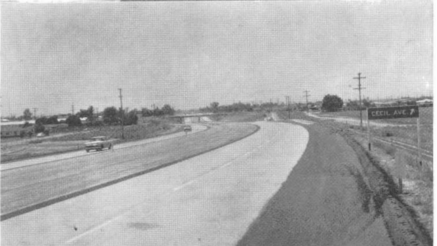
UPPER—Airport Road Overcrossing. View is looking southerly. LOWER—Cecil Avenue Overcrossing. This photo of freeway is looking southerly.
