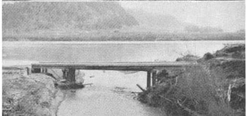
TOP—Maple Hill Bridge over South Fork of Eel River. NEXT—Temporary Bear River Bridge. NEXT—Temporary Home Creek Bridge. BOTTOM—Reconstructed Price Creek Bridge.
