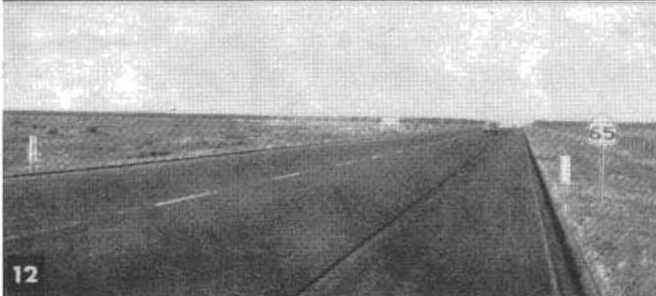
PHOTO No. 9. View of O. G. PMS blanket showing delineation characteristics—chip seal to be placed on shoulders. (No taper.) PHOTO No. 10. Question: Where are the E. P.'s? There they are! PHOTO No. 11. Here's what the O. G. looks like when carried through an intersection. PHOTO No. 12. Again the effective delineation of the open-graded PMS is clearly illustrated.
