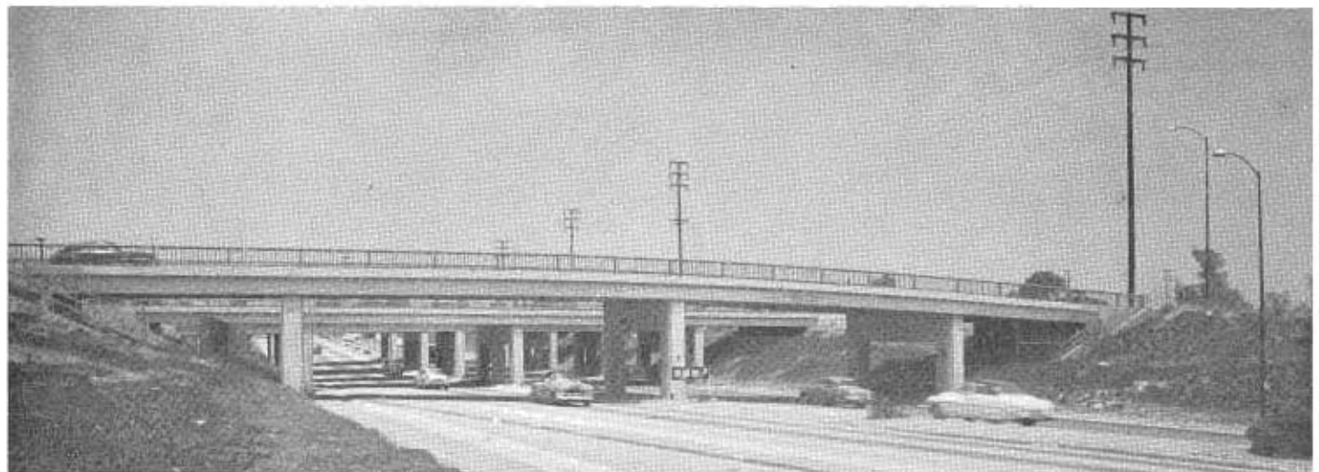
Looking northeast toward routes 158/26 separation structure on Rosemead Boulevard
