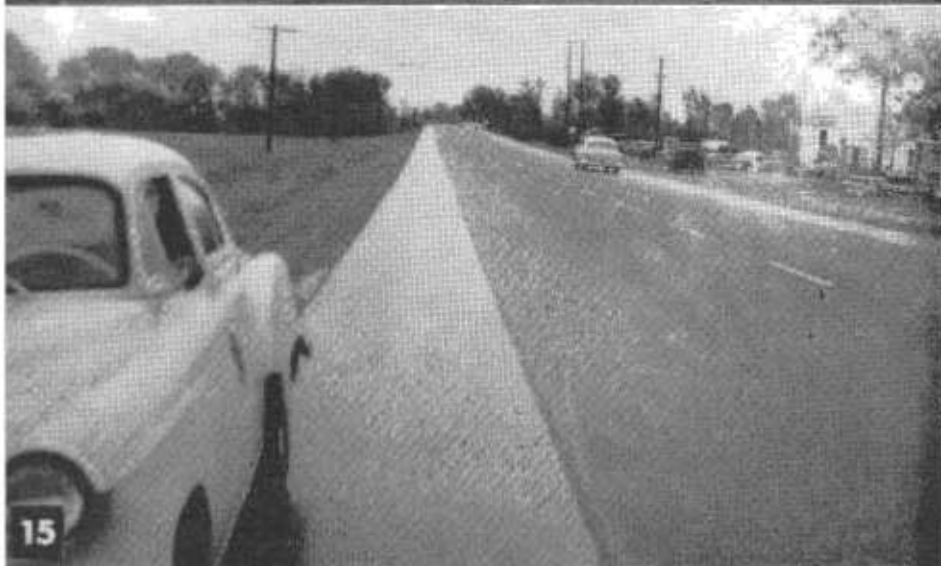
PHOTO No. 13. Another illustration of delineation characteristic of O. G. PMS. PHOTO No. 14. A section of Highway US 101 south of Klamath at the Freshwater Lagoon where recent floods inundated this section. Still in good condition. PHOTO No. 15. Delineation characteristic of O. G. PMS shown again. This pavement is one of the best in the State for smoothness and appearance.
