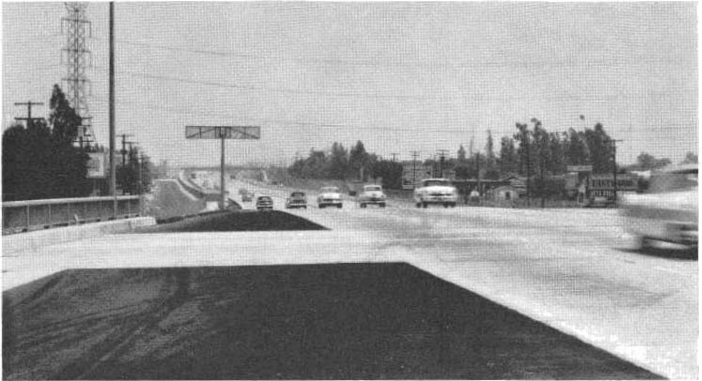
Looking easterly from River Grade Road Undercrossing
