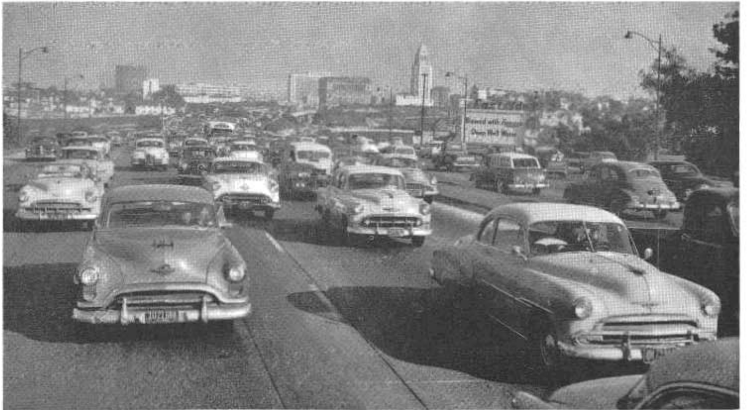
Hollywood Freeway, with traffic from the Pasadena Freeway merging. This is what a peak-hour flow of 7,800 vehicles per hour in one direction looks like.
