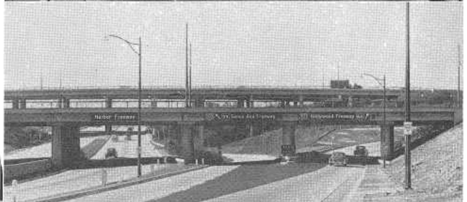
UPPER—Even slight upgrades significantly reduce capacity when truck volumes are appreciable. Note uneven distribution of traffic by lanes. LOWER—Another view of the four-level structure showing normal midday operation.
