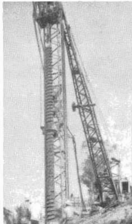
Cleaning drill rig auger
