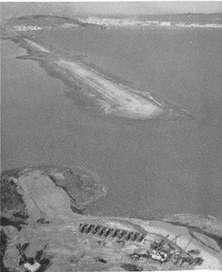
LEFT—Construction scene on Bayshore Freeway, looking south from Third and Bayshore Interchange in San Francisco toward Sierra Point. RIGHT—Open water fill for Bayshore Freeway across Candlestick Cave. Grading operations at Sierra Point in foreground.
