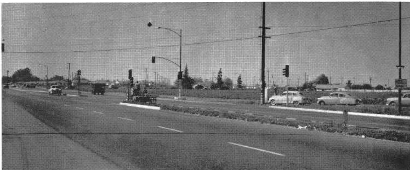
Analysis of accident reports showed clearly that in urban areas expressways with intersections at grade need to be replaced as soon as financially possible by full freeways with intersections separated by structures. UPPER—The Rosecrans-Firestone Intersection on the Santa Ana Freeway near Norwalk in 1952. LOWER—Aerial view of the same location completed to full freeway standards in 1955.
