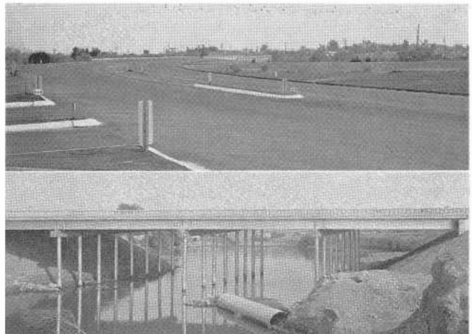
UPPER—Highway approach from existing bridge to new Yuma span. LOWER—Approach bridge to new Yuma structure.
