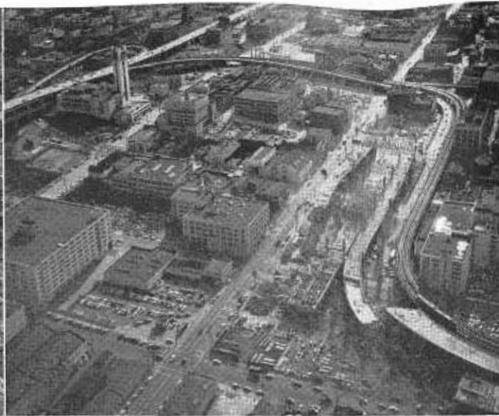
RIGHT—First stage of Embarcadero Freeway construction; Bay Bridge approaches left. LEFT—Embarcadero Freeway construction showing connection to Main and Beale Streets.
