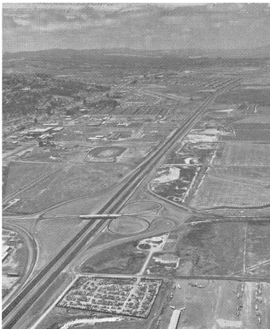
Bayshore Freeway, showing completed portion at Holly Street in San Carlos, northerly to San Mateo
