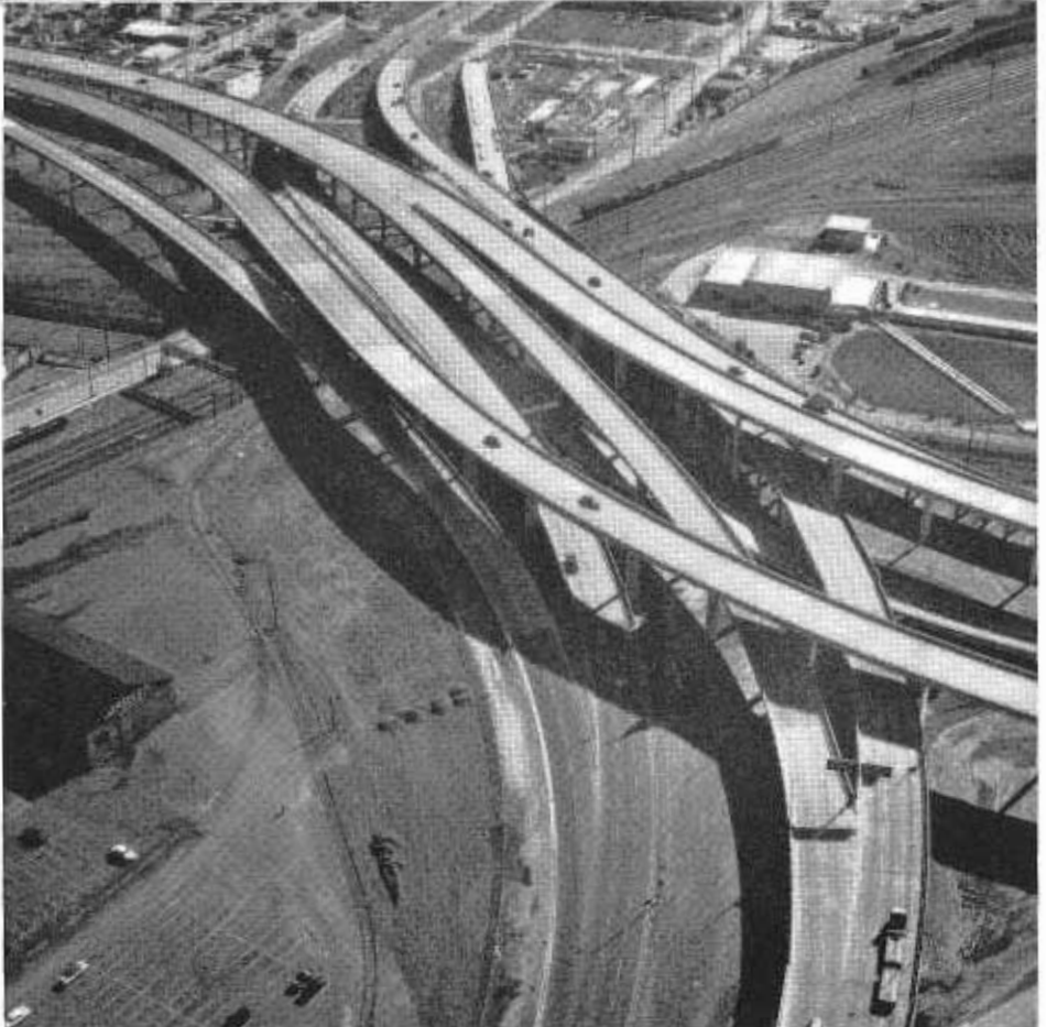
TOP—Distribution Structure from Bay Bridge toll plaza east. LOWER—Distribution Structure in Oakland looking east; three levels of highway structure over two levels of railroad.
