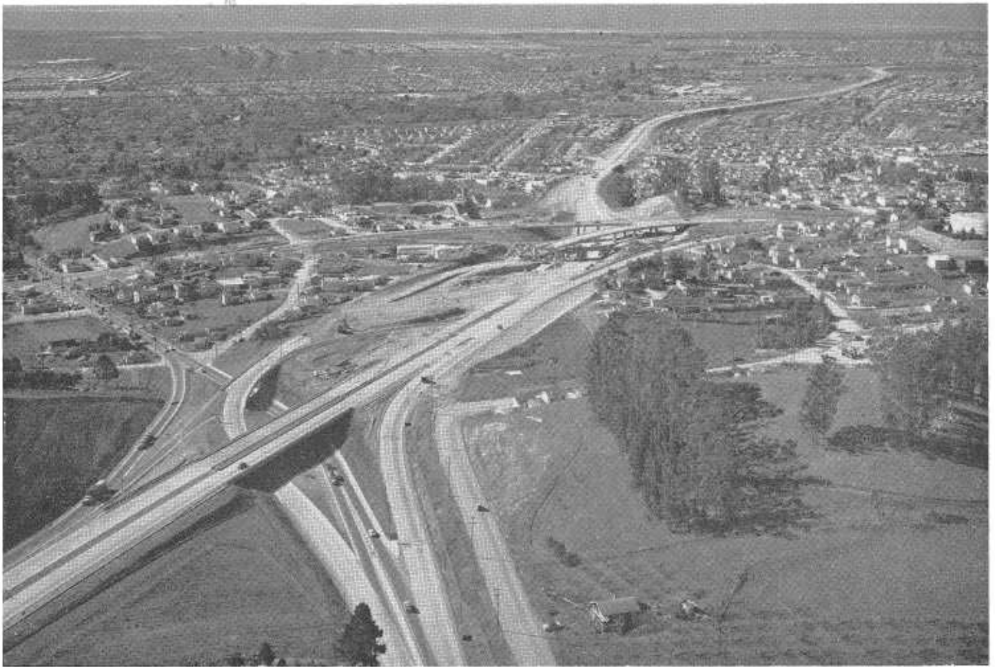
US 50 Interchange at Foothill Boulevard. Route 228 connection to Eastshore Freeway in background.
