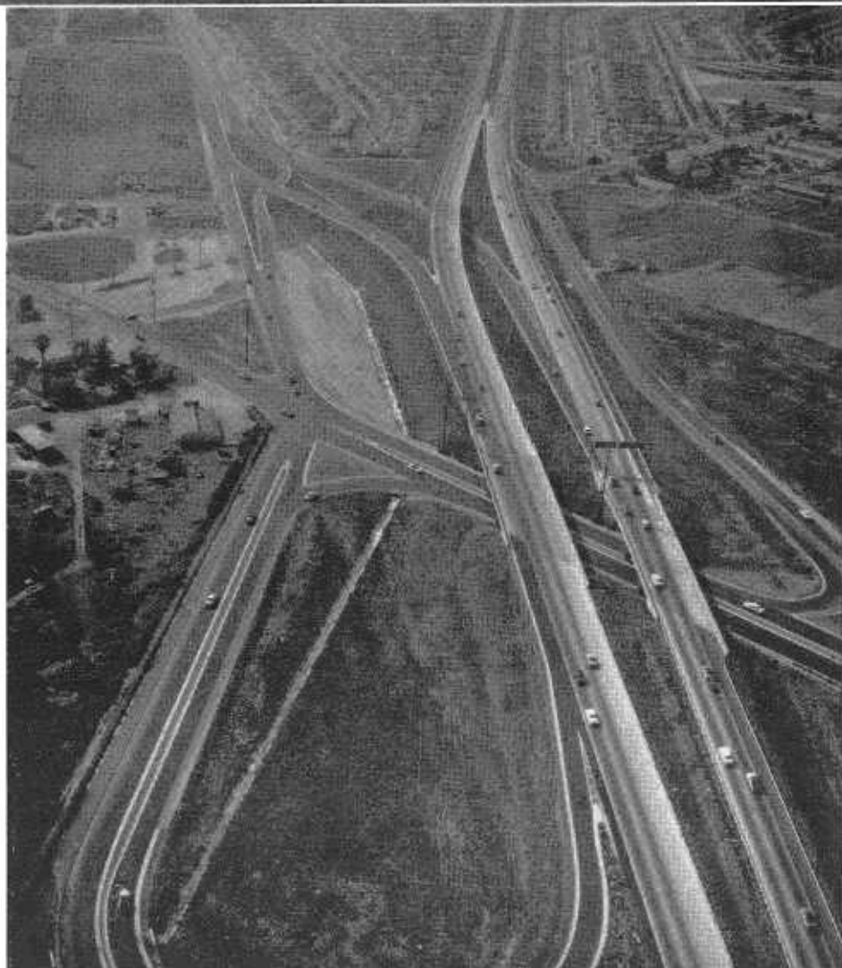
Analysis of accident reports showed clearly that in urban areas expressways with intersections at grade need to be replaced as soon as financially possible by full freeways with intersections separated by structures. UPPER—The Rosecrans-Firestone Intersection on the Santa Ana Freeway near Norwalk in 1952. LOWER—Aerial view of the same location completed to full freeway standards in 1955.
