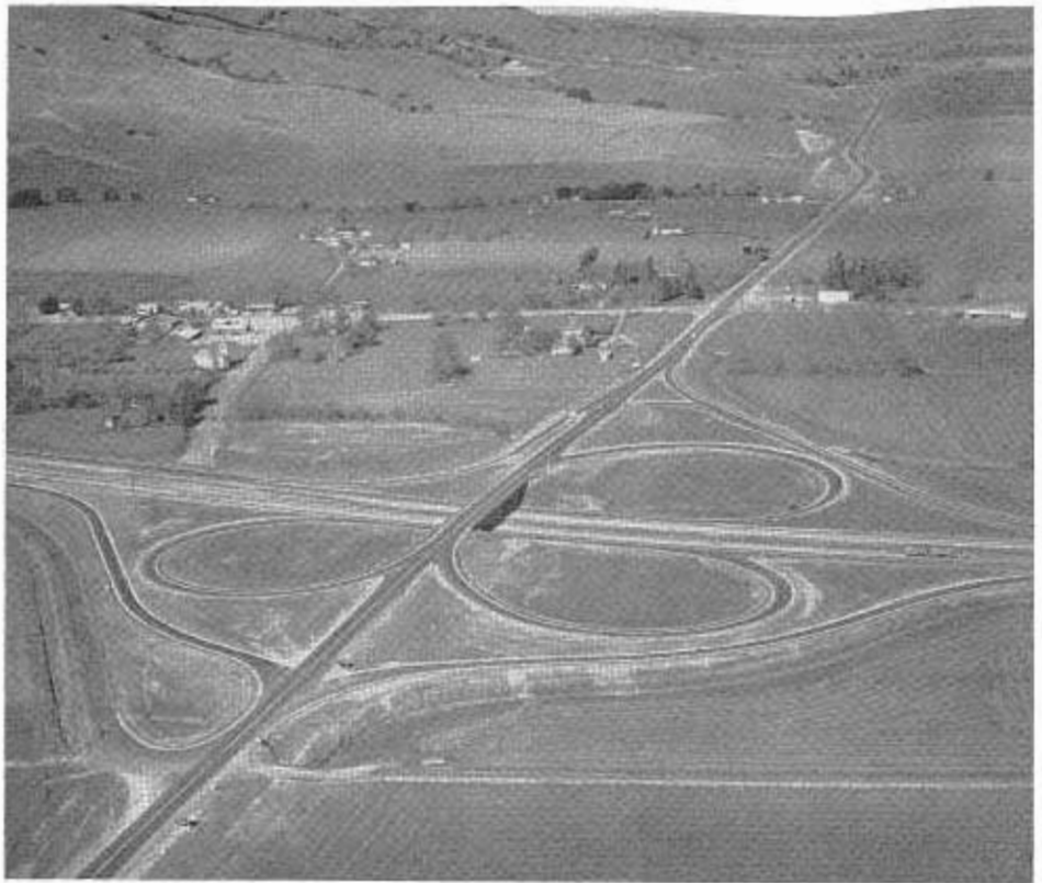
Dublin Interchange looking north; showing two-lane freeway recently constructed with provision for future four lanes northerly to Contra Costa county line
