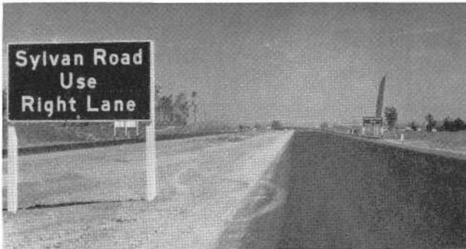
Upper and lower case letters are used in directional signs on the new Ben Ali-Roseville Freeway. The signs were installed on a test basis in an attempt to improve readability. Heretofore only overhead illuminated signs were of this type, the others all capital letters.
