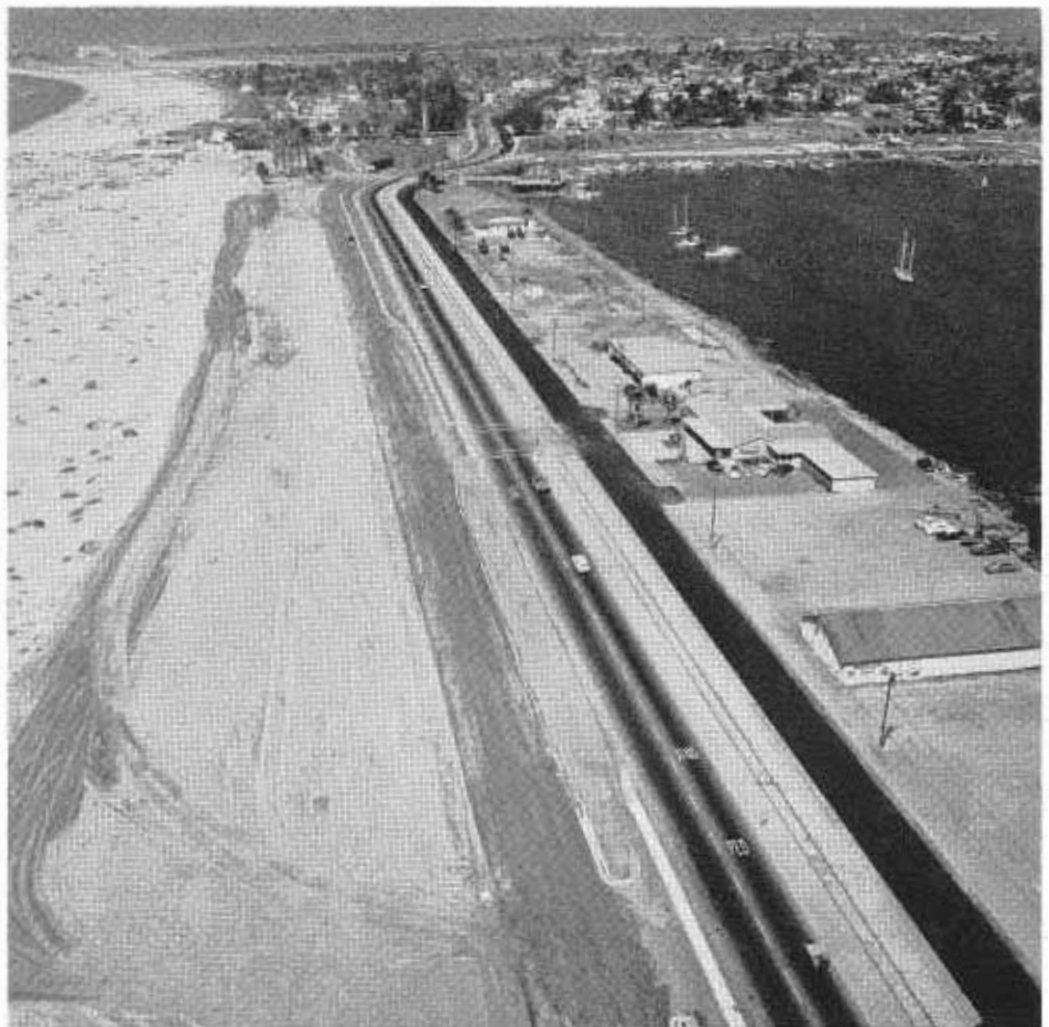
UPPER—Looking south on Silver Strand during construction. Temporary detours provide passage as pedestrian underpasses are built. Silver Strand State Park on right and left. LOWER—North end of Silver Strand at Coronado on Sign Route 74. New construction on ocean side will provide a four-lane divided highway.
