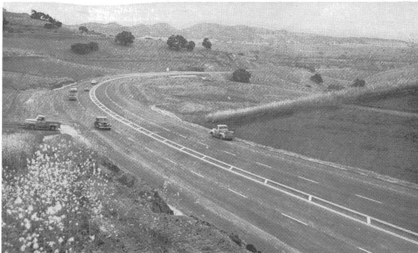
A view of the recently completed Ygnacio Valley Road Extension constructed by Contra Costa County as a limited access expressway under the Federal Aid Secondary Highway Program and the County Road Bond Issue Program
