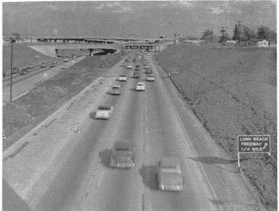
This photo shows extent of widening operations
