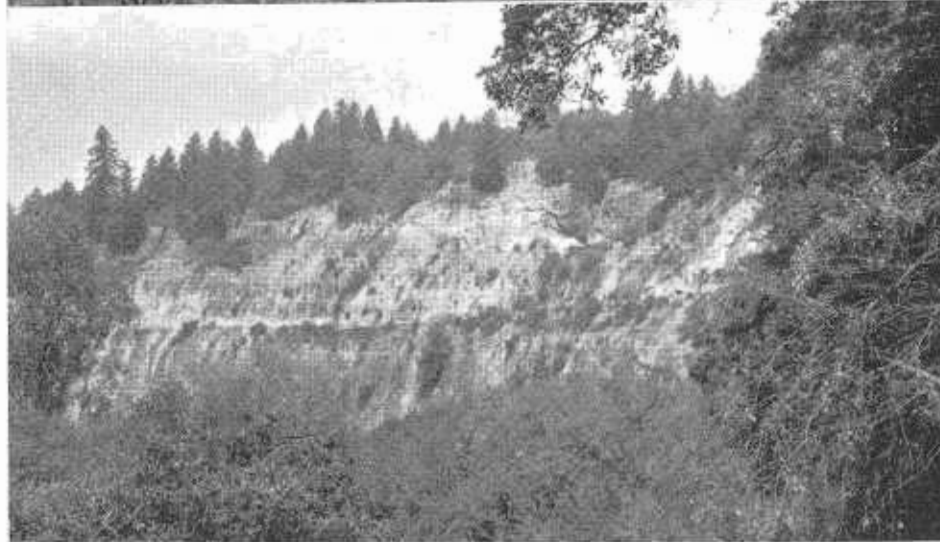
UPPER—Looking northerly down South Fork of Eel River, Phillipsville and Redwood Highway at right of picture. Typical of the terrain to be traversed by the Redwood Freeway. LOWER—Existing Redwood Highway just north of Garberville is benched into Garberville Bluffs along South Fork of Eel River. New location of proposed Redwood Freeway will supersede this portion of Redwood Highway.
