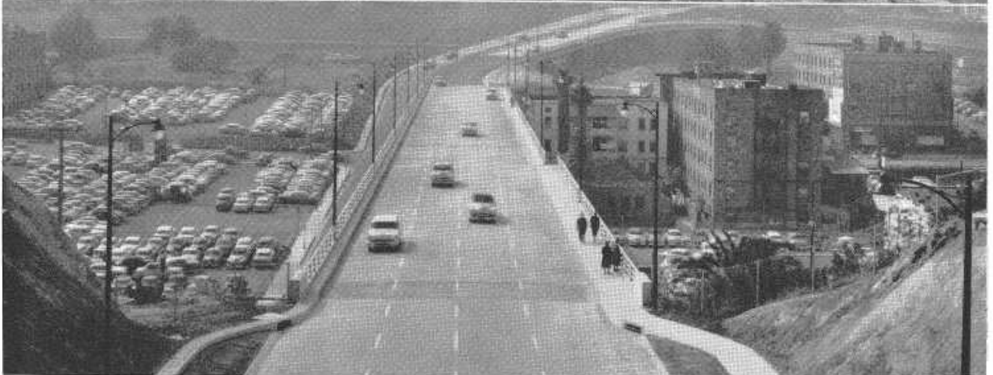
These three photographs were taken at same location as shown on opposite page after completion of project construction. (Note stairways for pedestrians to left of bridge carrying Grand Avenue over Fourth Street.)
