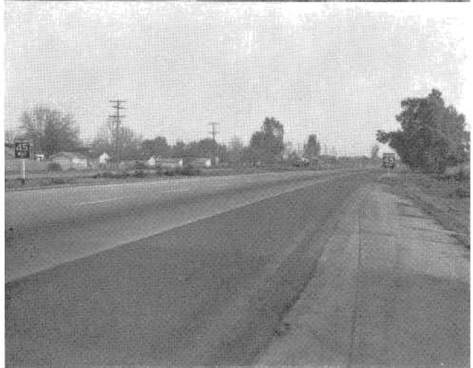
UPPER—Diamond-shaped yellow sign indicates a warning; reflectorized arrow specifically warns of curve to right ahead. LOWER—Speed limit signs are most familiar examples of regulatory type sign.
