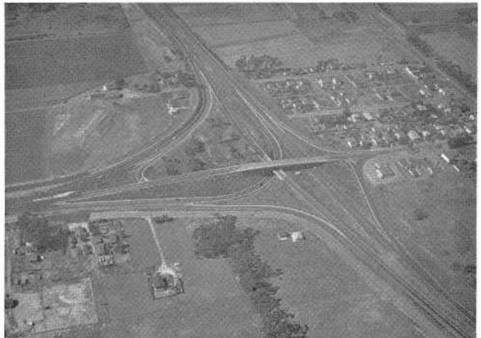
State Sign Route 75 joins US 101 at three-level structure in Palm City. Left center marks beginning of completed first unit of Route 75.
