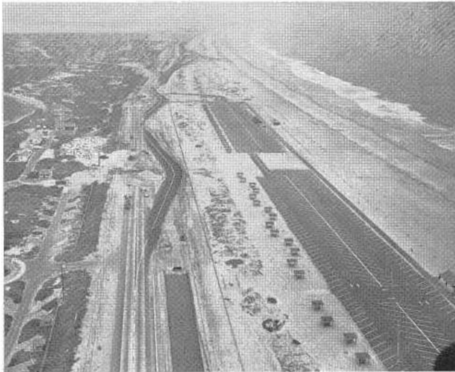
UPPER—Looking south on Silver Strand during construction. Temporary detours provide passage as pedestrian underpasses are built. Silver Strand State Park on right and left. LOWER—North end of Silver Strand at Coronado on Sign Route 74. New construction on ocean side will provide a four-lane divided highway.
