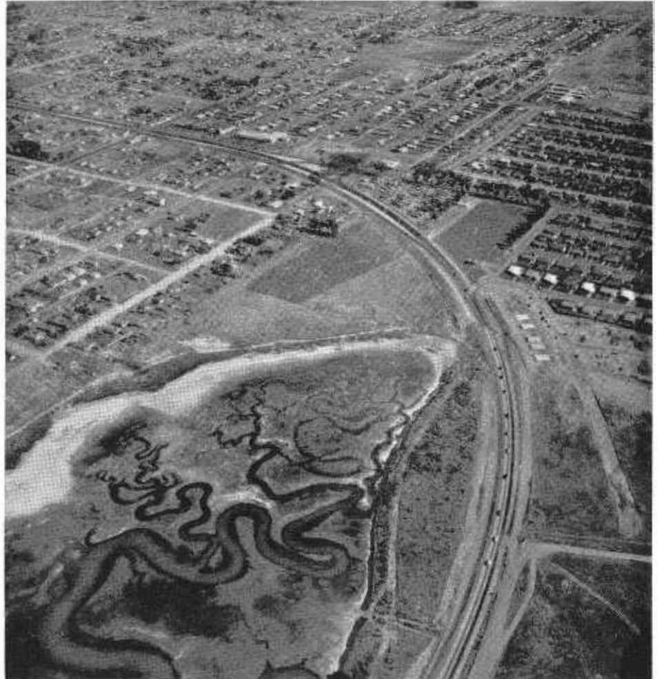
Southern end of Strand on Palm Avenue prior to construction. Divided highway in background marks completed portion of first unit.
