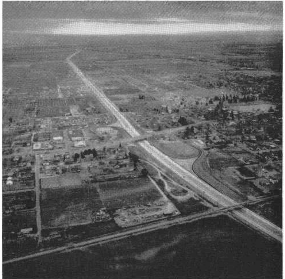
Aerial view showing freeway bypass of Tulare. Old highway can be identified by row of trees across upper right portion of photo. Interchange in center of picture shows Lindsay highway left of freeway and Tulare street on the right. This street extends west to intersection with old highway in vicinity of central business district, right of photo.
