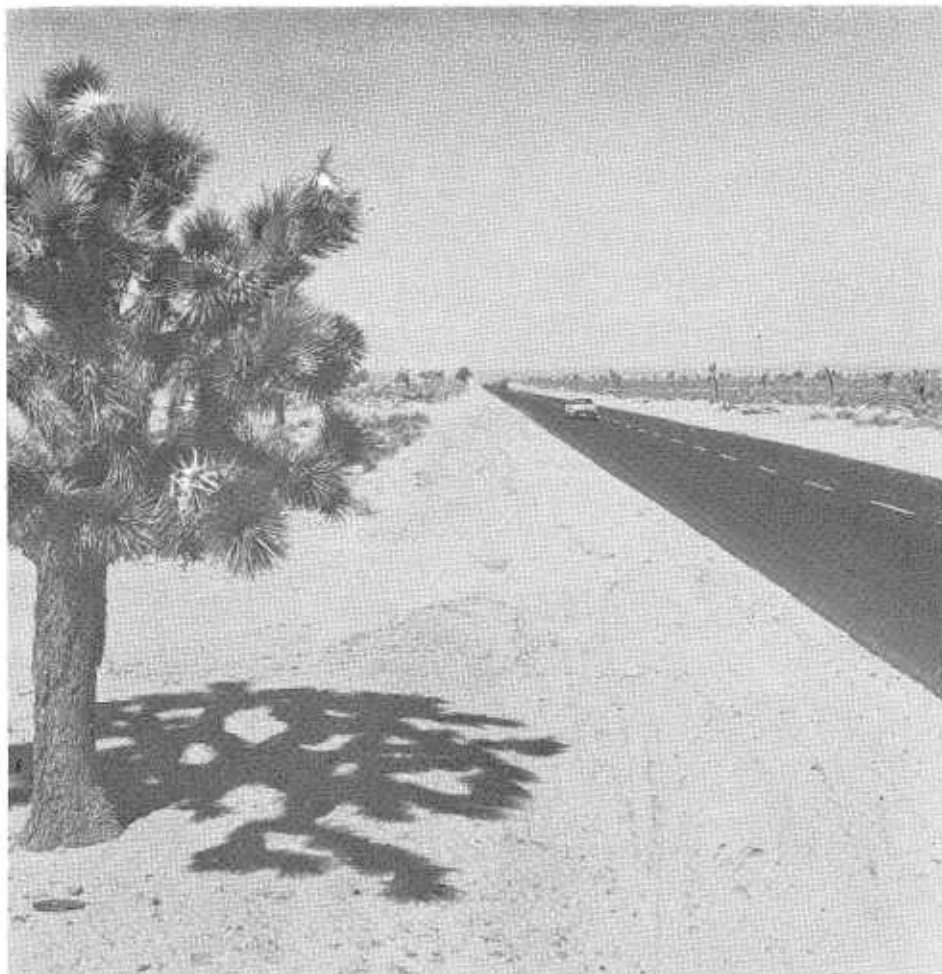
Desert scene showing section of new highway between Mojave and Boron
