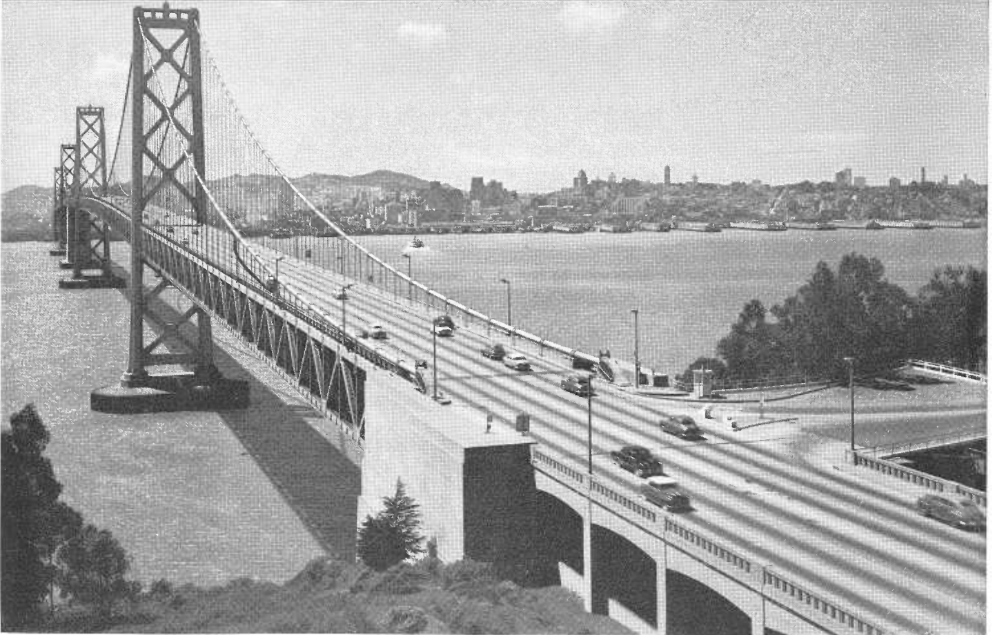
UPPER—Night scene of Bay Bridge during spinning of gigantic cables for the suspension section. LOWER—View of Bay Bridge just after its opening to traffic.
