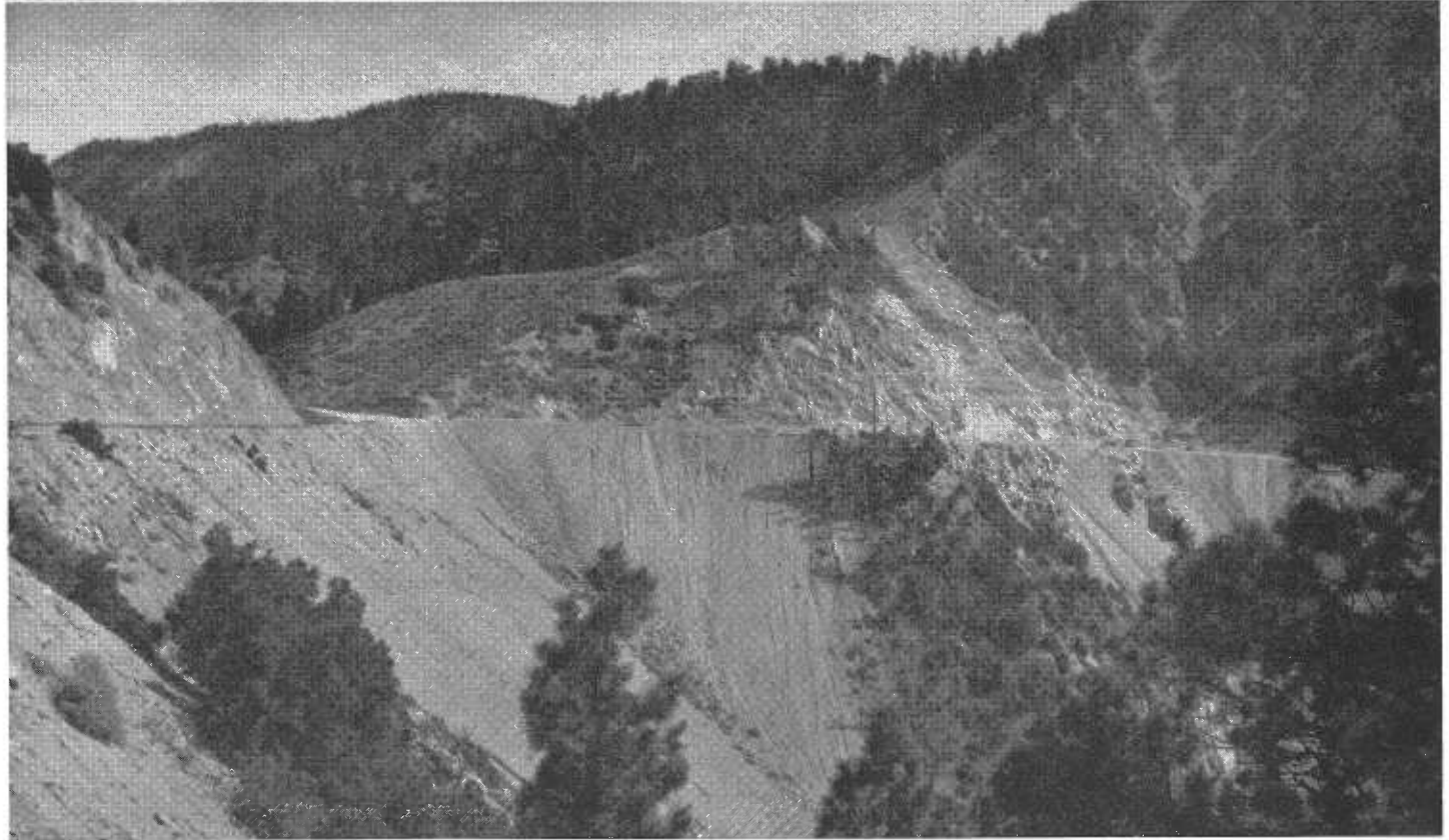
UPPER—Completed Angeles Crest Highway at entrance to Upper Chilao recreational area in the Angeles National Forest. LOWER—Looking easterly showing long embankment slopes where junction occurs between Crystal Lake Highway and Angeles Crest Highway. Completed Angeles Highway to left. Crystal Lake Road under construction, to right.
