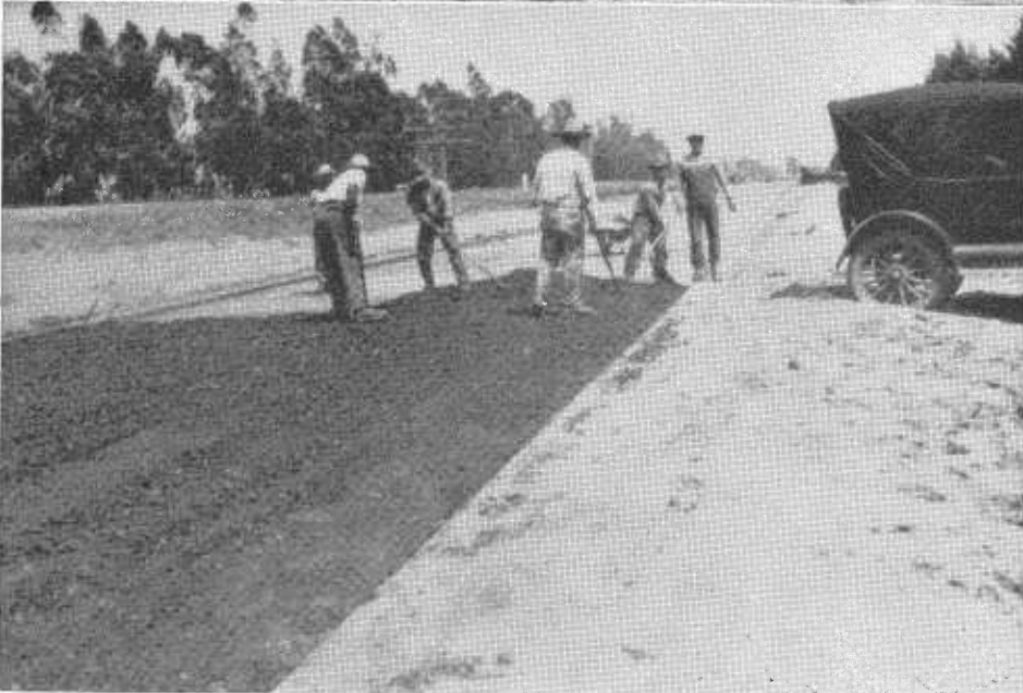
UPPER—Old sand subgrade, looking east. Raking old base course.
