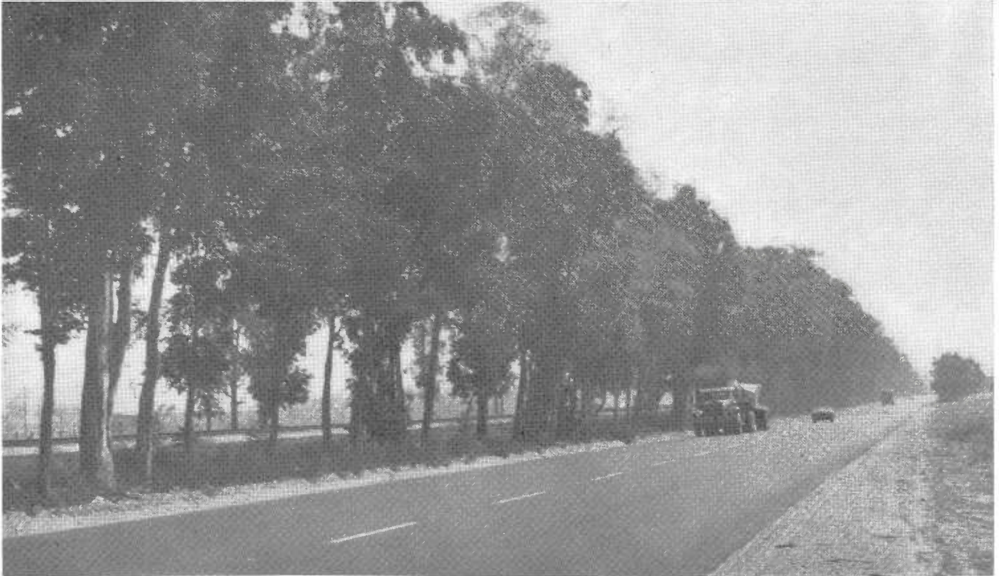
UPPER—View of road just before resurfacing. Note new eastbound roadway on right. LOWER—View of new road as it looks today.
