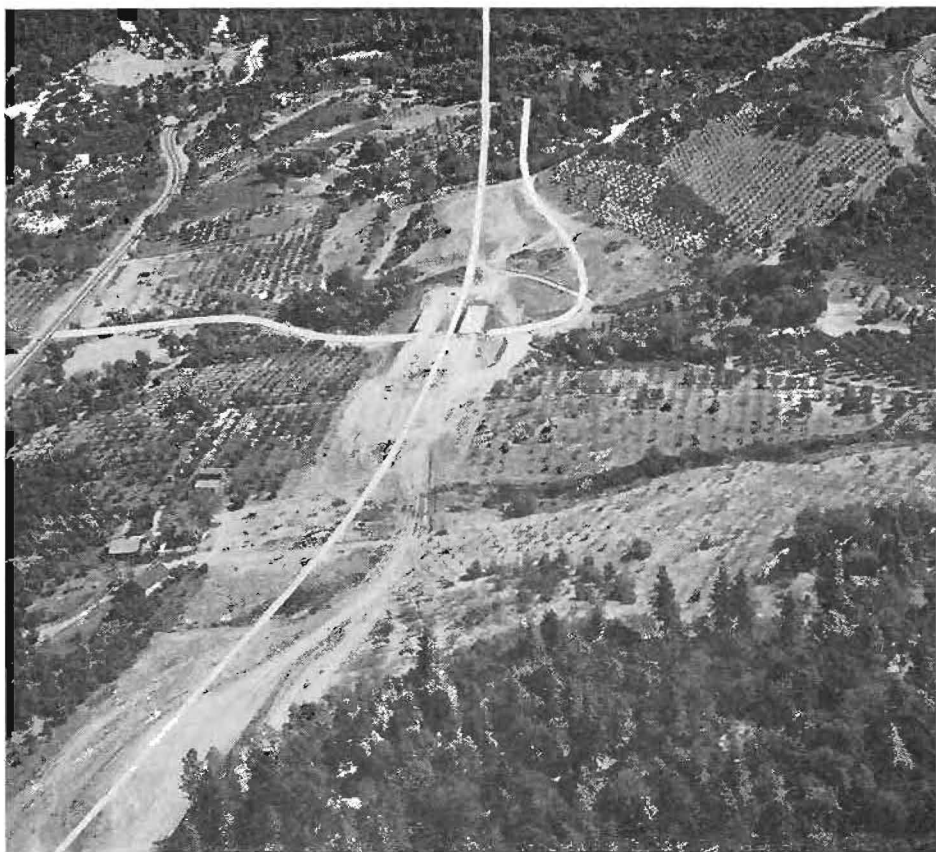
Looking easterly—Hallbom Road Undercrossing under construction
