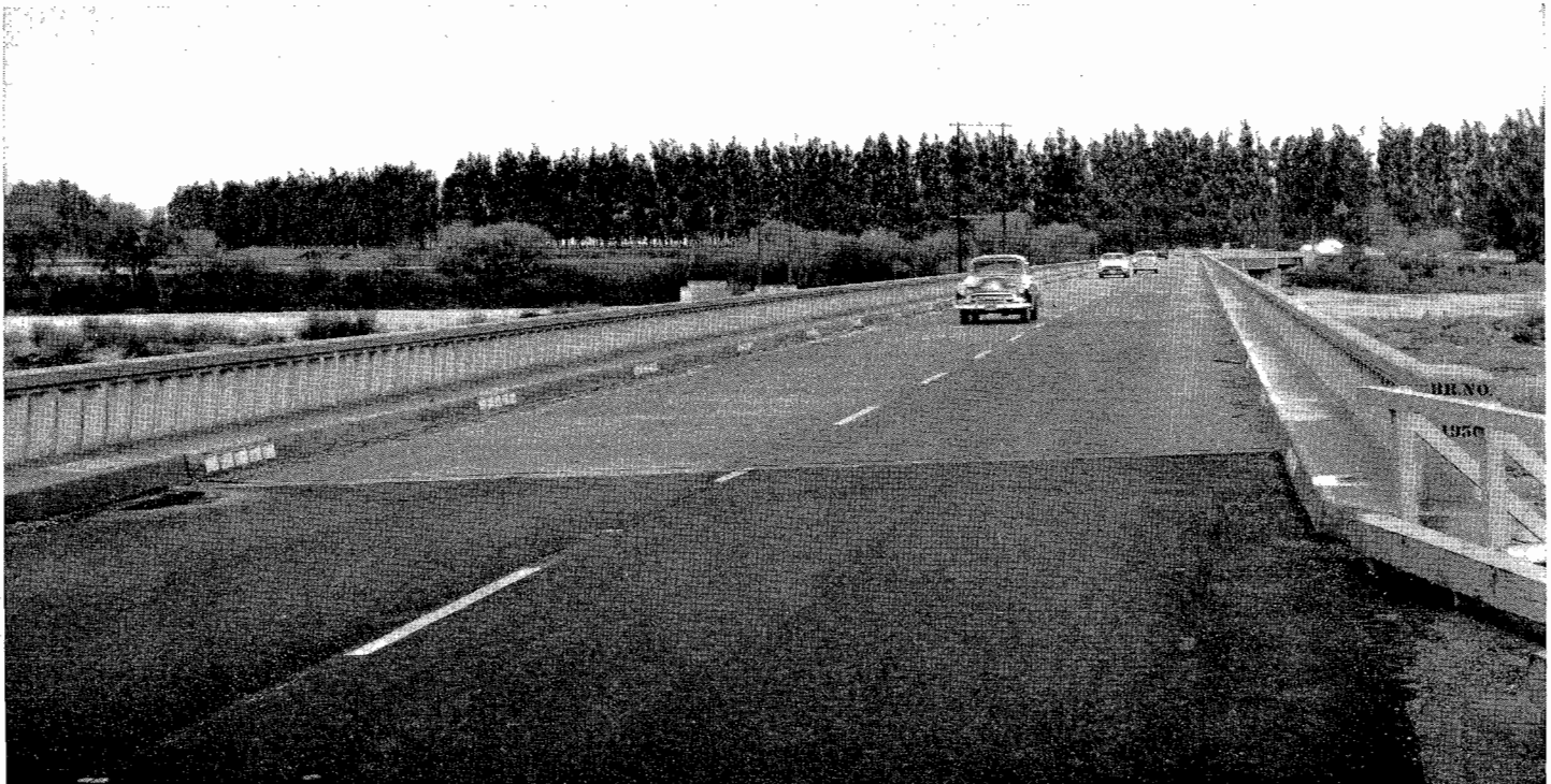
Traffic begins using new span across Salinas River
