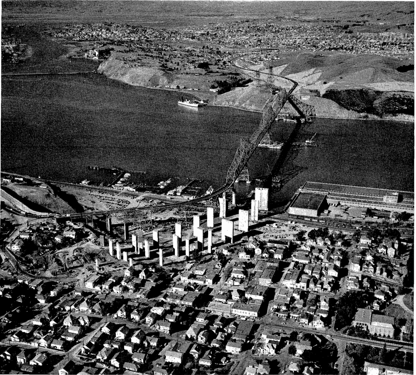
Work is in progress on the Vallejo side of Carquinez Strait in this picture. Contractor's derricks and barges can be seen at each of the main channel piers. The Crockett Interchange piers are being constructed in this picture. These interchange piers will be completed in January and steel erection will start in February, 1957.
