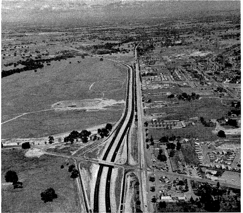
This photo shows completed section of Roseville Freeway in Sacramento County
