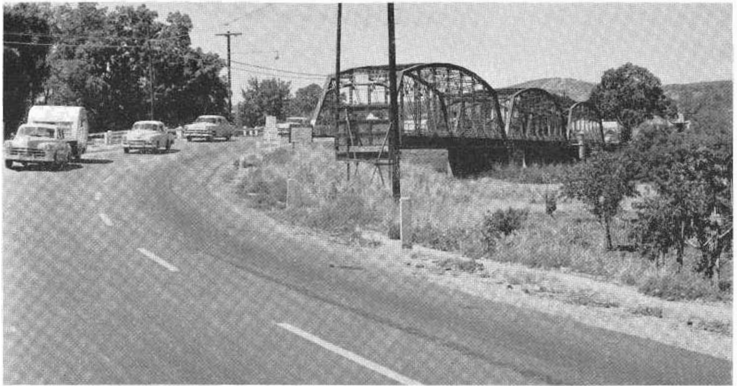
Present steel pratt truss bridge across Salinas River looking westerly toward Paso Robles
