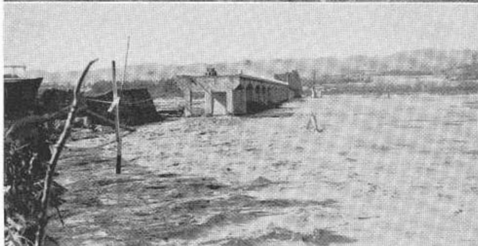
UPPER—Floodwaters washed out detour bridge and detour during reconstruction work on the Santa Clara River bridge in 1939. LOWER—Southwest approach to the Santa Clara River bridge washed out during flood of February, 1944.
