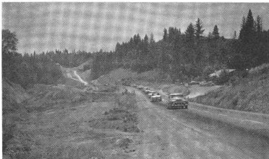
On US 40 about one mile west of Colfax, looking easterly
