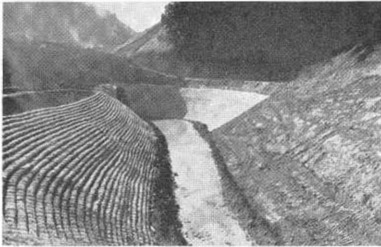
LEFT—Looking westerly down riprap section of channel approaching 20-foot arch culvert, one of three on project. RIGHT—Showing 84-inch reinforced concrete pipe installation's relative position to existing traveled way—new alignment.
