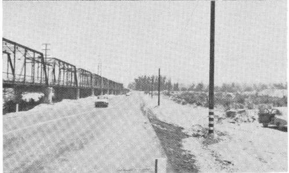
UPPER—Prestressed girders at casting bed. LOWER—View along detour and existing bridge.
