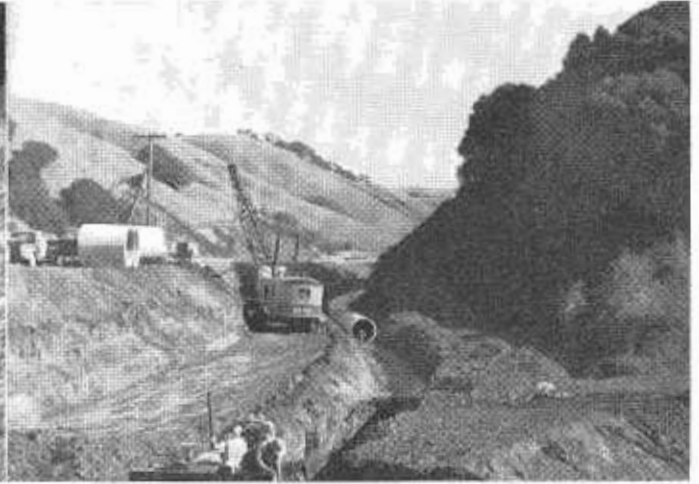
LEFT—Looking westerly down riprap section of channel approaching 20-foot arch culvert, one of three on project. RIGHT—Showing 84-inch reinforced concrete pipe installation's relative position to existing traveled way—new alignment.
