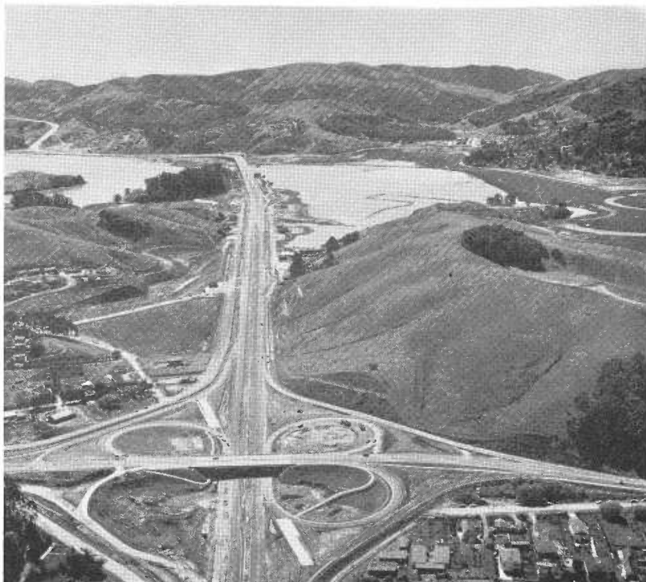
Alto interchange looking south toward the new bridge at Richardson Bay on US 101
