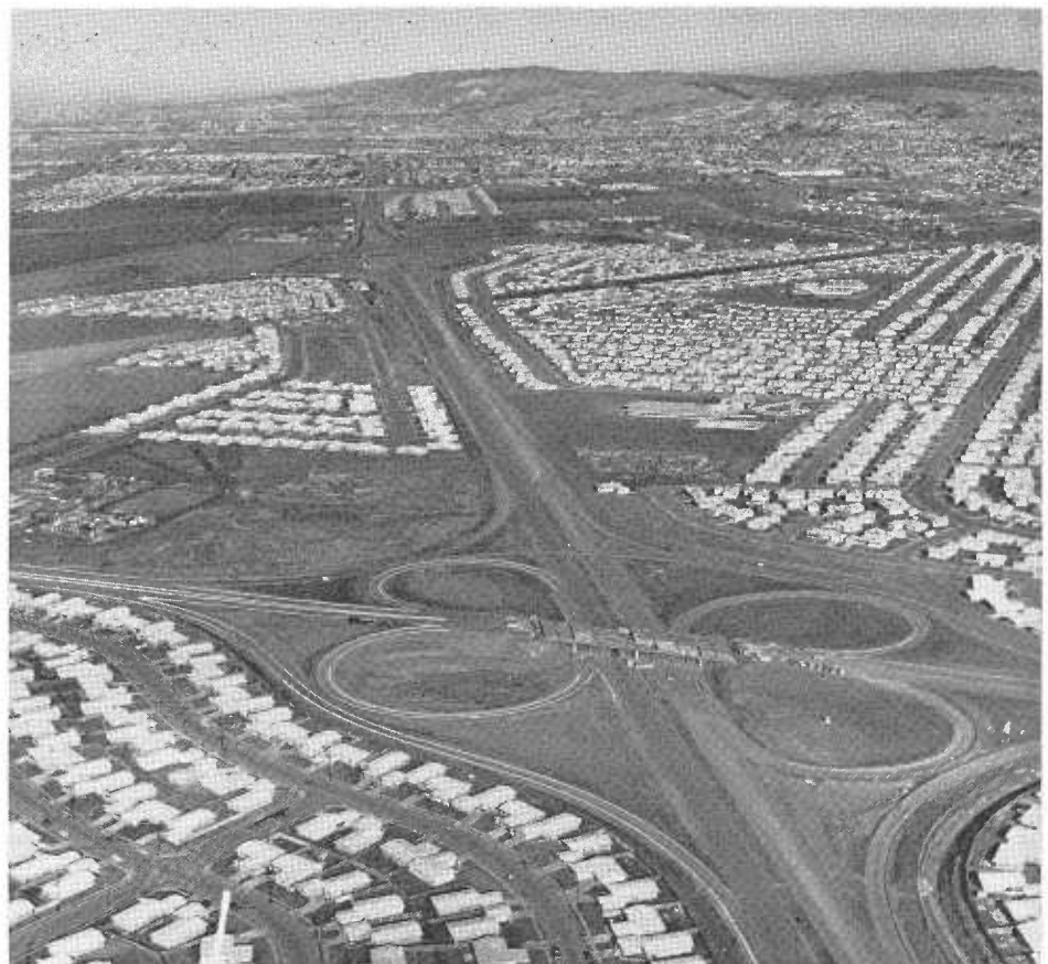
Eastshore Freeway construction between Beard Road and Jackson Street in Hayward. Note desirability of locating residential areas near ready access and also result of advance planning.
