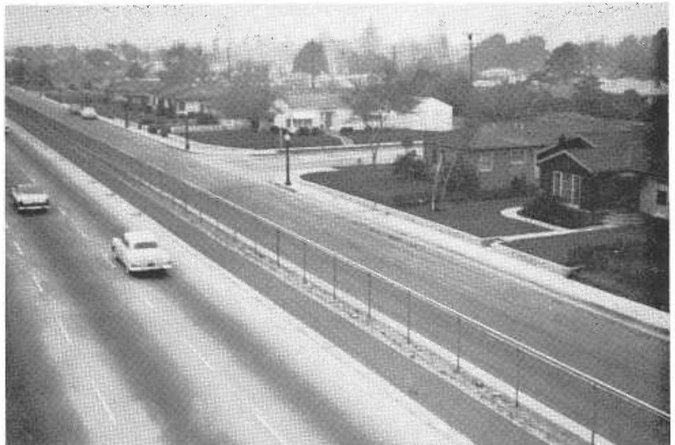
Residences on frontage road alongside San Bernardino Freeway. The chain-link fence through center of photo separates freeway traffic lanes from frontage road.
