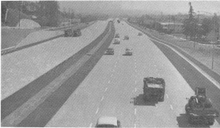
Looking south at completed section of San Diego Freeway from Sunset Boulevard overcrossing
