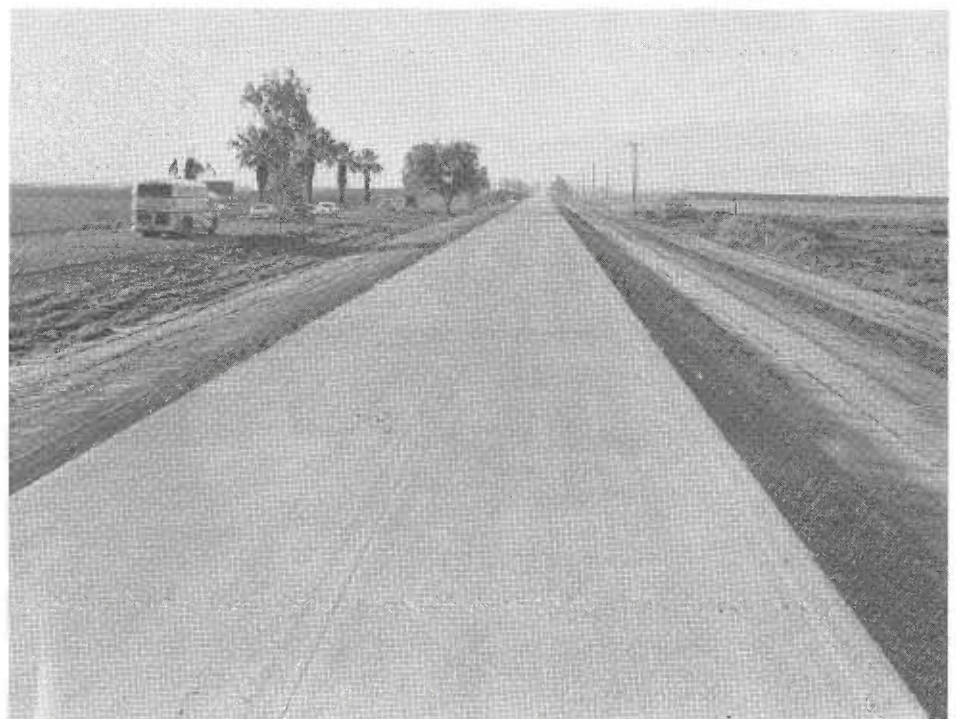
View looking southerly, showing long stretch of second-story concrete paving
