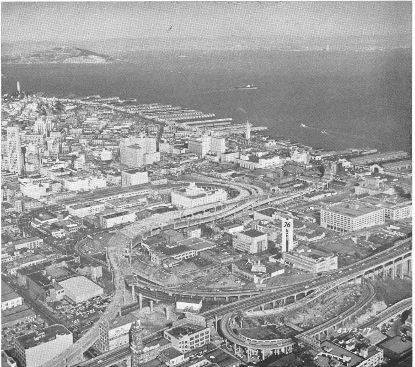
Embarcadero Freeway construction in progress on single and double decked structures. West approach to the Bay Bridge at bottom. Main and Beale Street connections in center.
