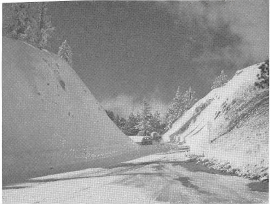
Merritt Ridge near Newcombs ski lift on Angeles Crest Highway
