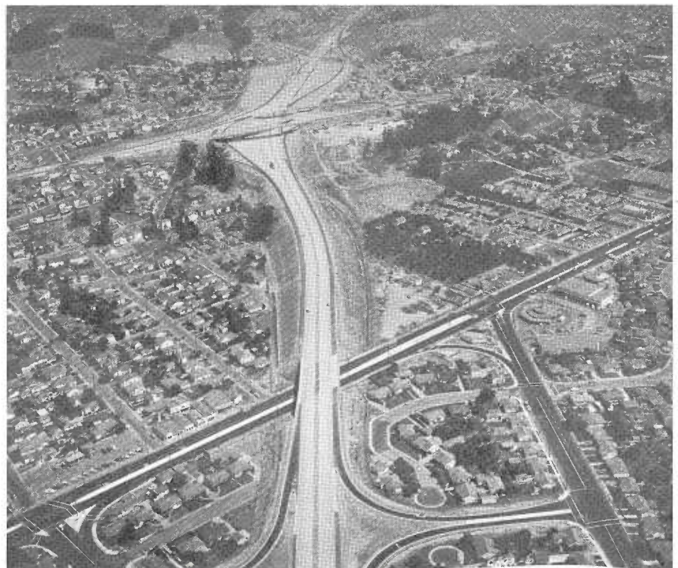
Looking easterly along connection from Eastshore Freeway to US 50 between San Lorenzo and Castro Valley. East 14th Street interchange in foreground. Foothill Boulevard interchange top center.
