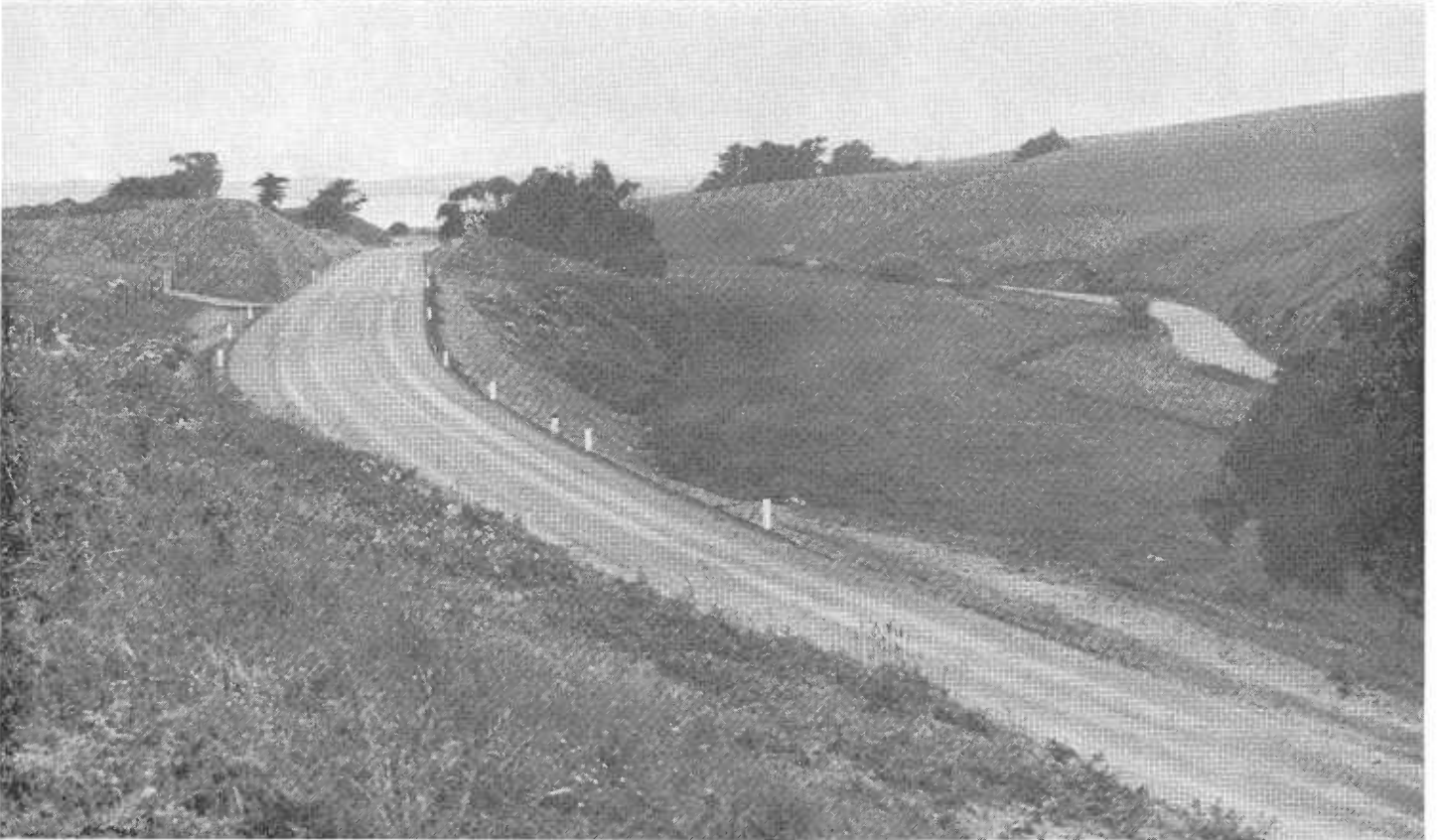
UPPER—Newly completed highway. Note contrast with old road at left. LOWER—This is another view of new highway, showing old winding road on right.
