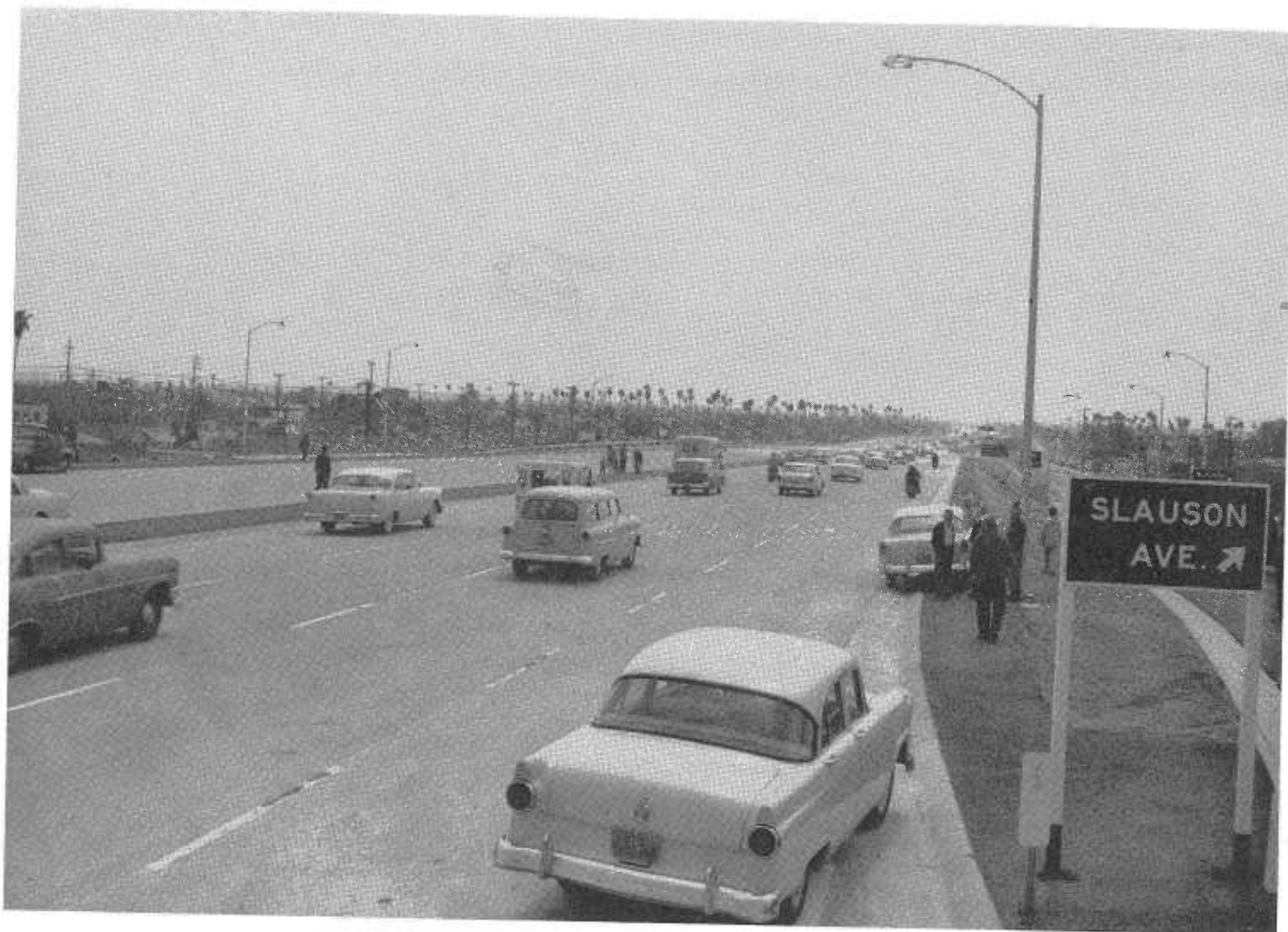
Following ribbon cutting auto caravan traveled over new section of Harbor Freeway
