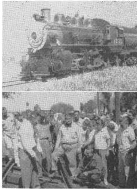
Driving golden spike. In foreground Frank Pucci with hammer; center, Stuart Waite, and kneeling, Leonard Payne.
