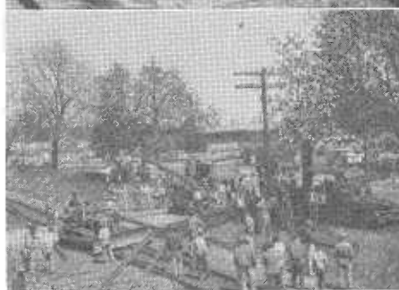
Setting up sections of rail across main line of railroad tracks
