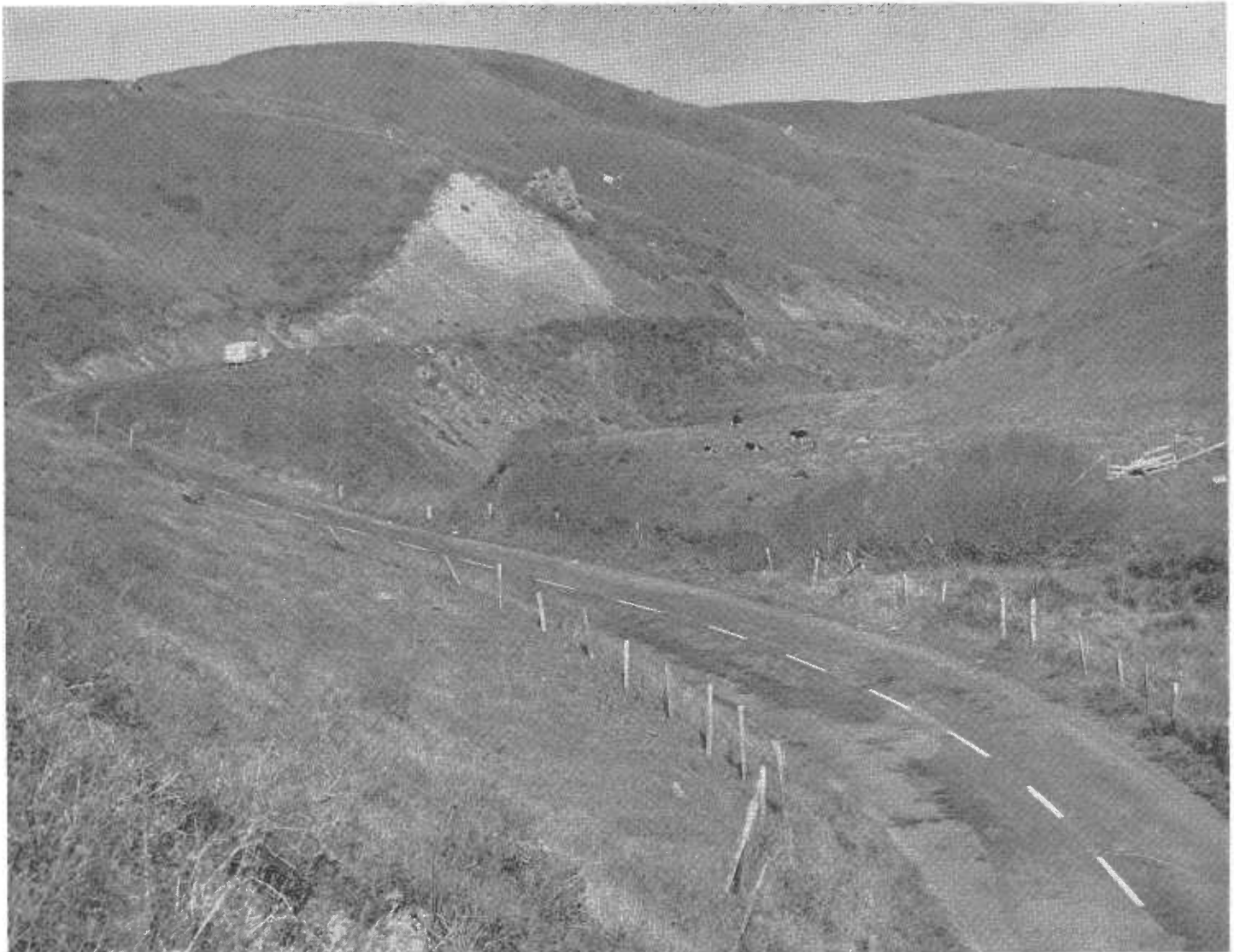
This photo shows section of old Valley Ford-Bodega Bay highway prior to recent improvement
