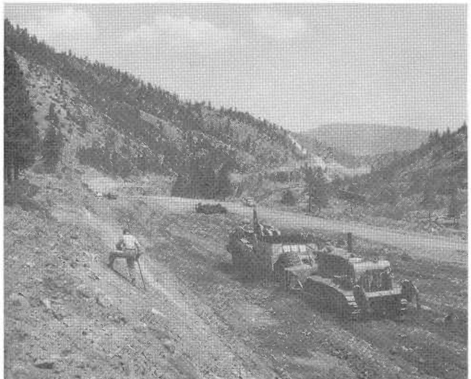
Start of construction in Truckee River Canyon
