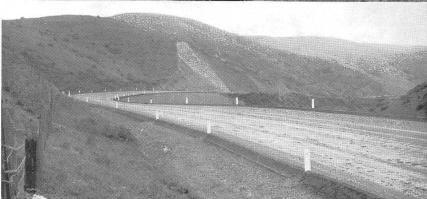
UPPER—Section of the Valley Ford-Bodega Bay highway recently completed by Sonoma County. LOWER—This photo shows improved section of highway shown in picture on page 5.
