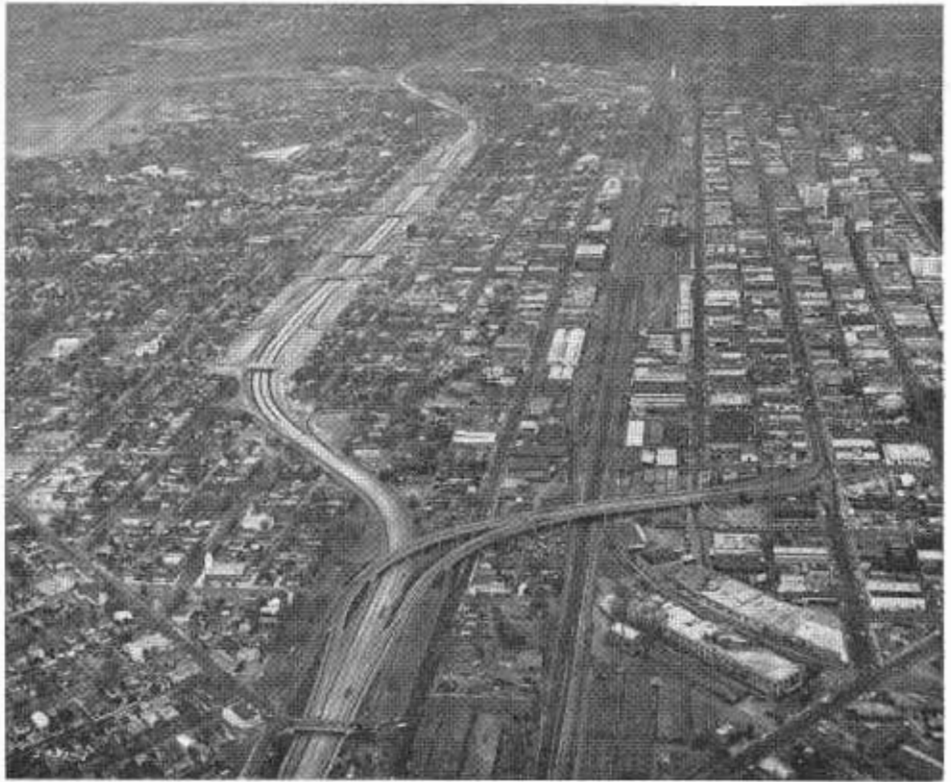
The fresh whiteness of the newly completed Fresno Freeway makes it prominent at the left of this aerial photograph looking north over the city. Bypassed area downtown is to the right.
