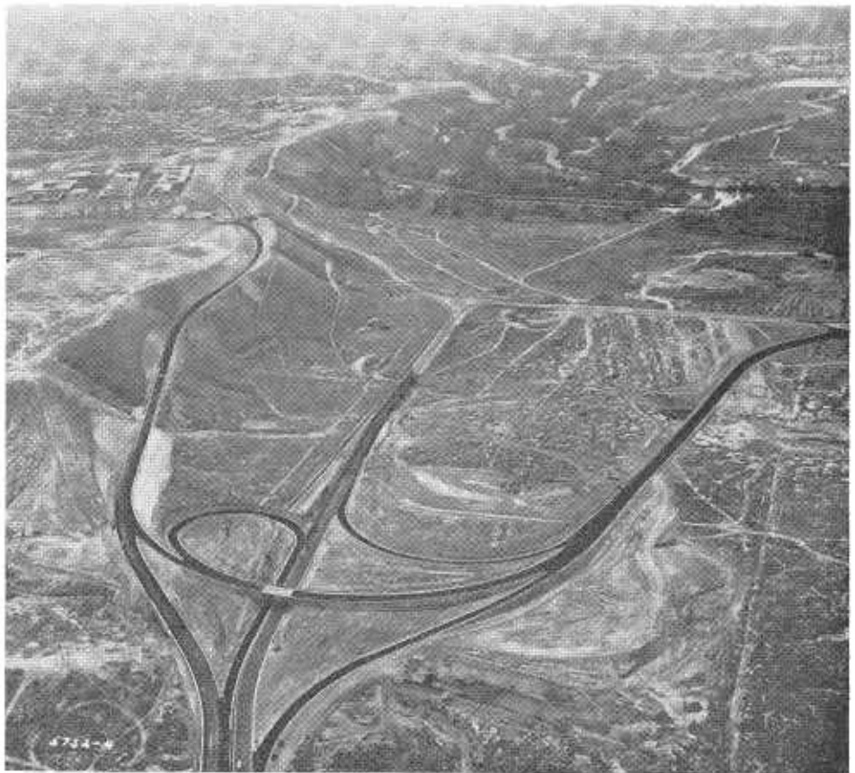
Interchange constructed with federal, state and county funds, seen from above the Alfred Harrell Highway with Bakersfield in distant left, Panorama Drive and Bakersfield College at left
