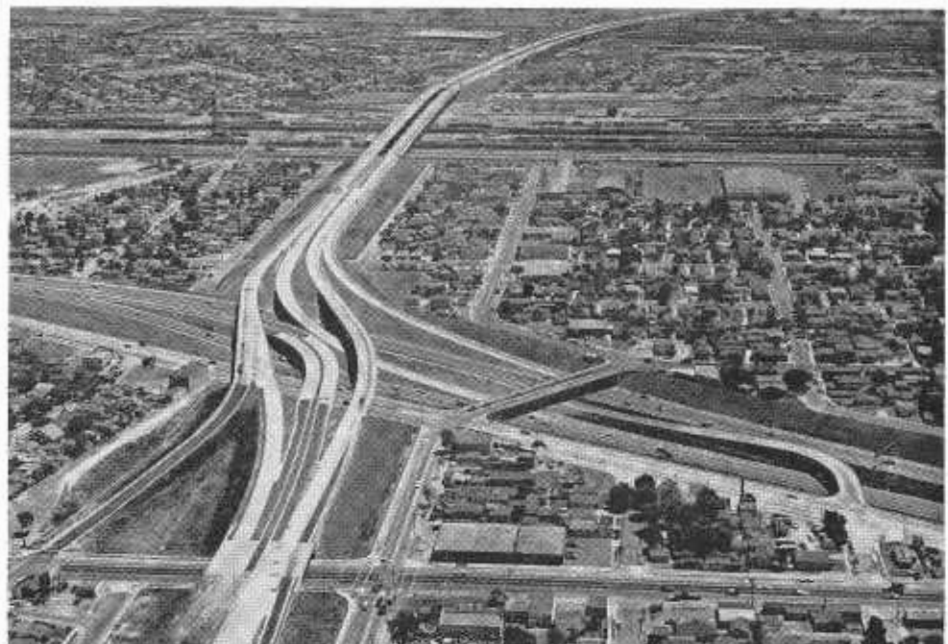
Here is a view looking southerly along Long Beach Freeway showing the interchange with Santa Ana Freeway and in the background the crossing over freight classification yard of Union Pacific Railroad.
