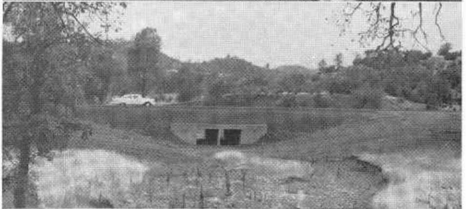
Eleven fords like this one (UPPER) on State Sign Route 36 west of Red Bluff were replaced by culverts (LOWER) in a highway improvement program which was celebrated by a log barrier cutting ceremony attended by (CENTER, left to right): District II Highway Engineer H. S. Miles, Assistant State Highway Engineer J. W. Trask, Chairman Lynn Raymond of the Tehama County Board of Supervisors, State Senator Louis G. Sutton, Miss Judy Adams (Miss Tehama County), Pioneer Erle Gans operating the power saw, Deputy Public Works Director C. M. (Max) Gilliss, Master of Ceremonies James Froome, Jr., Thomas McGlynn, Red Bluff Chamber of Commerce leader; Lumberman A. B. Hood, and Sheriff Albert Nichols of Humboldt County. Other leaders of both Tehama and Humboldt Counties were at the opening festivities.
