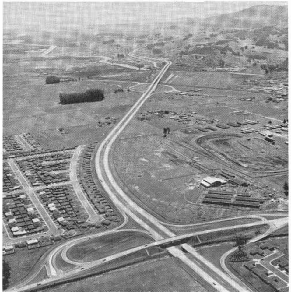
Various aspects of sound zoning and subdivision planning are illustrated in this view of the East Washington Street Interchange area on US 101 near Petaluma. Not only do the homes nearest the freeway back onto it, but the subdivider has also enhanced the residential-access feature of his streets by providing turnaround areas. The author also points out that the freeway serves as a buffer between residential and industrial zones while permitting safe, free-flowing circulation between them by means of the overcrossing structure and interchange ramps.
