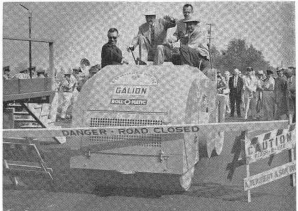
Lieutenant Governor Harold J. Powers operates the control that drives a lumbering roller against a road barrier as he participates in the ceremonies opening widened US Highway 50
