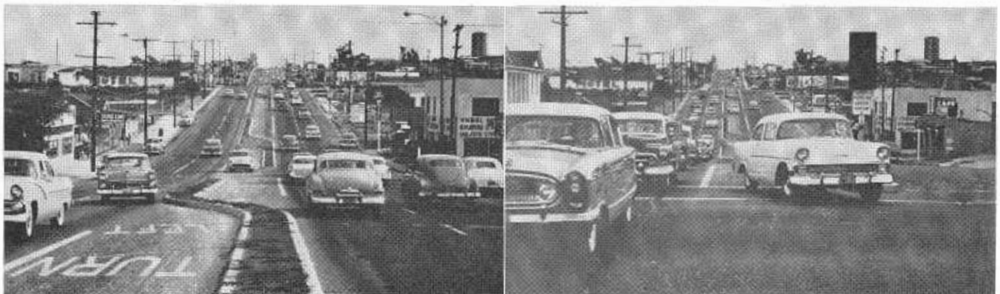
LEFT—Looking south on Sepulveda Boulevard from Manhattan Beach Boulevard, showing conditions of roadway after completed improvement. Note sampling detectors in right foreground. RIGHT—Looking south from Manhattan Beach Boulevard, showing vehicles moving during A minor phase.
