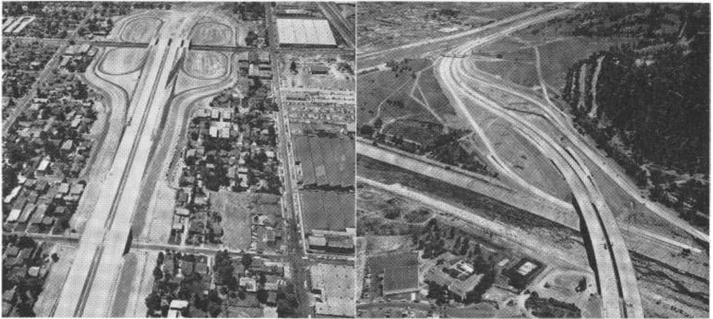
LEFT—Looking northerly along Golden State Freeway showing construction nearing completion with Allen Avenue Undercrossing in foreground and Alameda Avenue Undercrossing in background. RIGHT—Looking southerly along Golden State Freeway construction nearing completion in Griffith Park with Los Angeles River and Riverside Drive Bridge in foreground. Traffic interchange facilities with future Ventura Freeway shown in center.
