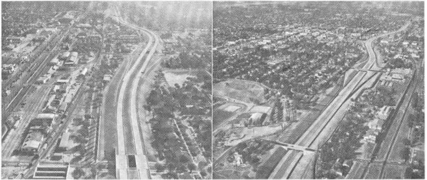
LEFT—Looking south along recently completed Riverside Freeway from above Third Street. Seventh Street and Eighth Street crossing near middle of photo. RIGHT—Looking north along Riverside Freeway through center of Riverside. Fourteenth Street Overcrossing in middle of photo.
