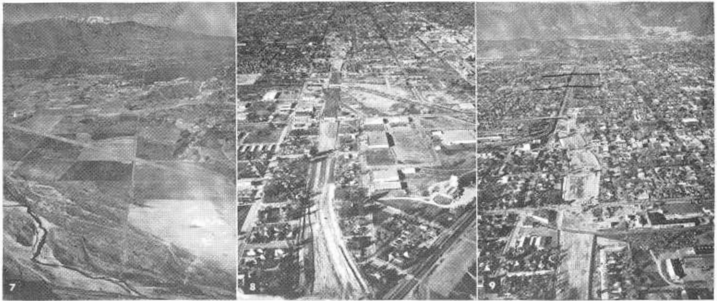
PHOTO No. 7—Looking east toward the Grand Terrace area. The north end of the future Riverside Freeway shows in the fill construction near the grain bins at the extreme left center of the picture. A future freeway contract for which plans are now in the design stage will traverse the farmland east of the Santa Ana River in the foreground. PHOTO No. 8—Looking north along the San Bernardino Freeway from a point above the Colton Avenue interchange. The Mill Street Undercrossing and the Lytle Creek Bridge are under construction in the center of the picture. I Street lies parallel to and just west of the freeway. The portion from Mill Street to Sixth Street in San Bernardino is now under construction by E. L. Yeager Company, the completion estimated in January, 1958. PHOTO No. 9—Looking north along the San Bernardino Freeway from above Rialto Avenue. The Santa Fe railroad yards and the Fifth Street Viaduct show in the center of the photo. Construction of the northbound freeway lanes across Fifth Street (US 66 Business) required the closing of Fifth Street for approximately six months. This structure was completed and Fifth Street reopened to traffic on June 15, 1957. Future extension of the freeway to the north, with two contracts expected to be advertised for bids this summer, is indicated by the line on the photo.
