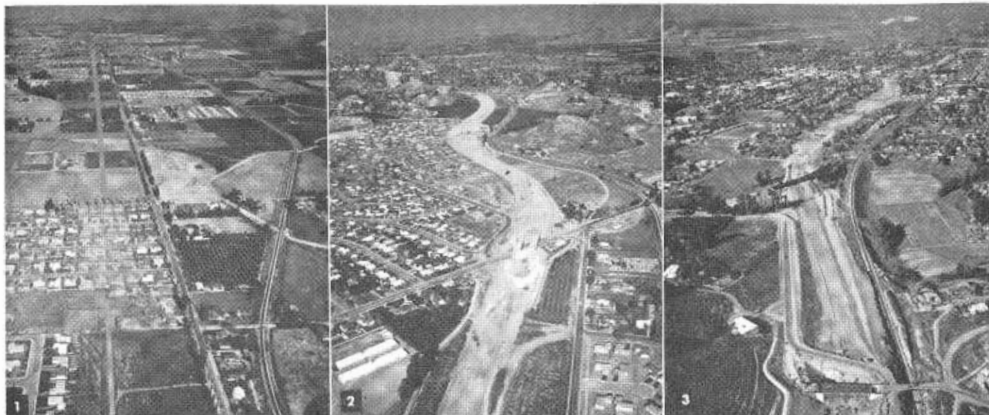
PHOTO No. 1—Looking north along route of the third unit of Riverside Freeway, which soon will be under construction. Freeway will lie to the left of Indiana Avenue, where housemoving operations can be seen underway. Jackson Street crosses through the center of the picture. This third unit will extend from Polk Avenue to the end of the second unit at Arlington Avenue, which can be seen in the background. PHOTO No. 2—Looking north from the south end of the second unit of the Riverside Freeway, which is now under construction by Griffith Company. Arlington Avenue Undercrossing and interchange ramps are in the foreground; Pachappa Hill is in the left center. This $2,000,000 contract extends from Arlington Avenue to 14th Street, with estimated completion in September, 1957. PHOTO No. 3—Looking north from the Ivy Street Overcrossing, showing construction underway through the City of Riverside. Pachappa Underpass of the Union Pacific Railroad is in the center.
