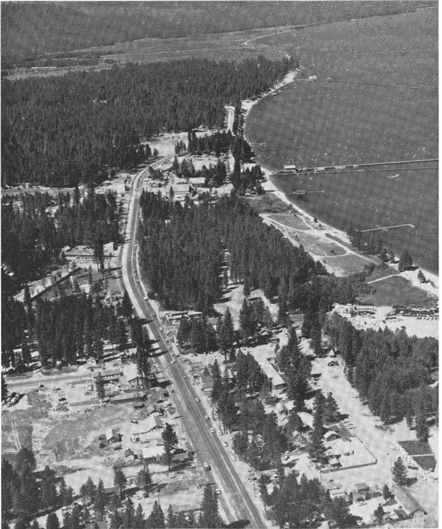
View of widened section of U. S. 50 looking westerly from Bijou on Lake Tahoe
