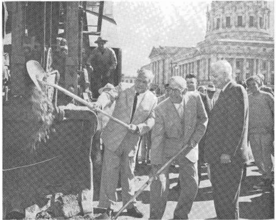
Scene at ground breaking. Left to right—Governor Goodwin J. Knight, Contractor J. F. Barrett, and Director of Public Works Frank B. Durkee.
