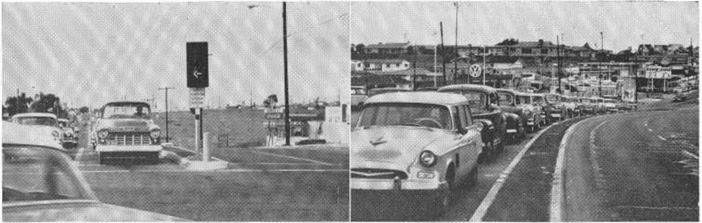
LEFT—Looking north from Manhattan Beach Boulevard, showing 12-inch left-turn green arrow during A minor phase. RIGHT—Looking north on Sepulveda Boulevard from Gould Lane showing 780 vehicles per hour left-turn movement.
