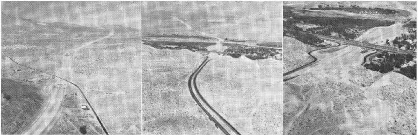
LEFT—Grading under way at south end of Fredericksen & Kasler contract. Bridge piers under construction for the first crossing of Stoddard-Wells Road, a county road. CENTER—North end of completed Victorville bypass showing construction under way by Gordon H. Ball, contractor on Victorville Overhead and Mojave River Bridge. RIGHT—Closer view of construction at Victorville Overhead and Mojave River Bridge. First crossing of Stoddard-Wells Road in right background.
