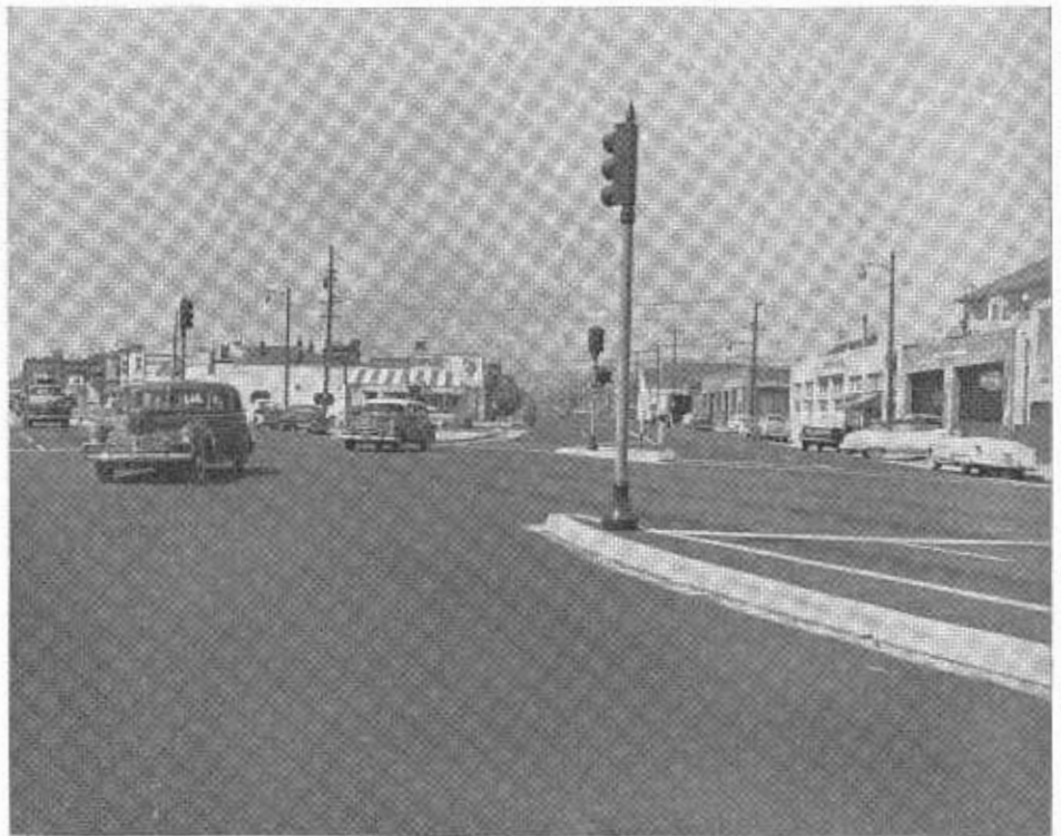
Channelization at San Pablo Avenue and West Street, looking northerly up West Street
