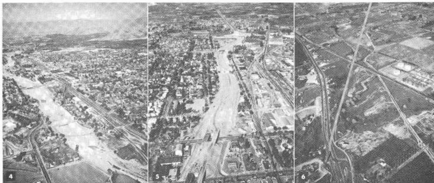
PHOTO No. 4—Looking north along the Riverside Freeway, showing Cridge Street Overcrossing in the foreground, and 14th Street Overcrossing in the center. The first unit of the Riverside Freeway is under contract with Griffith Company, and extends from 14th Street to Russell Street in the background. PHOTO No. 5—Looking north along the Riverside Freeway from above Eighth Street. The existing expressway along La Cadena Drive shows at top of photo, and the Third Street Undercrossing near the center. This unit, a $1,900,000 contract, is estimated to be completed in July, 1957. PHOTO No. 6—Future extension of the Riverside Freeway is indicated by the line running northeast from a point north of the present junction of Iowa Avenue and La Cadena Drive at lower edge of photo. Barton Road, a major county highway, extends across through the Grand Terrace area at the top of the picture.
