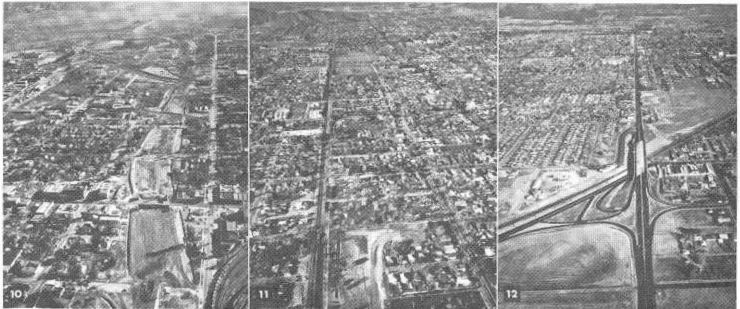
PHOTO No. 10—This is a photo looking southward along the San Bernardino Freeway from a point above Fifth Street. The large fills under construction for the US 70-99-91-395 interchange are visible in the far background. PHOTO No. 11—A view looking north along I Street from above Fifth Street, showing right-of-way clearance operations underway immediately east of I Street. PHOTO No. 12—Looking east along Highland Avenue, State Sign Route 30. The large graded area in the lower left will be the location of additional interchange ramps to be constructed in conjunction with the US 91 freeway project.
