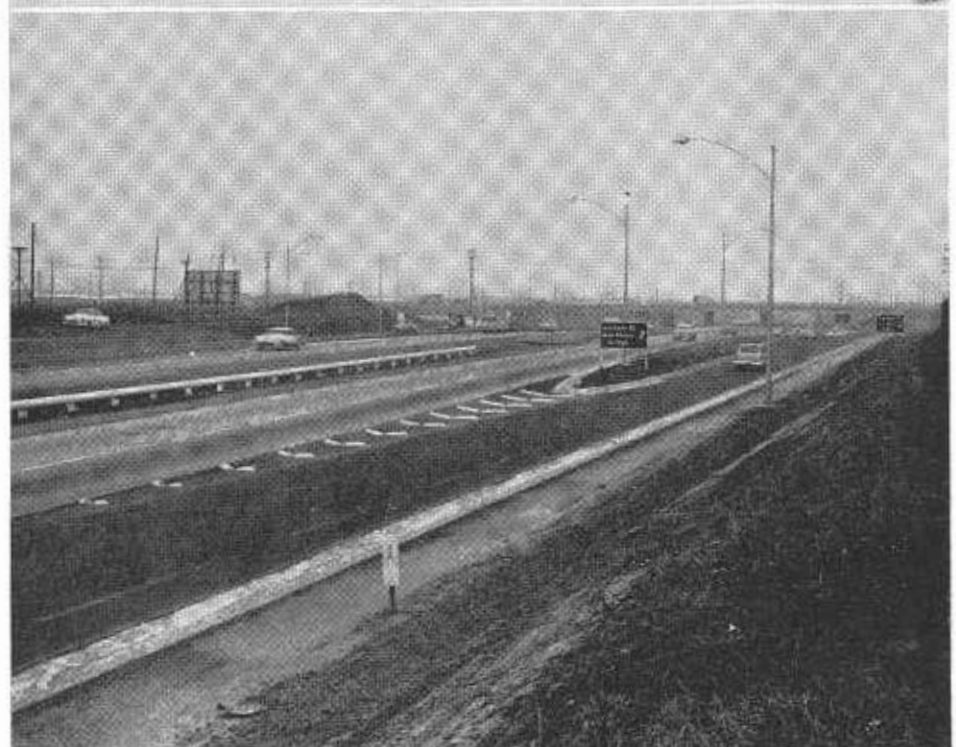
UPPER—Giant scissors cut a ribbon and open to traffic the most recently completed section of the Eastshore Freeway. LOWER—The Jackson Street separation shortly after the freeway was opened to traffic.
