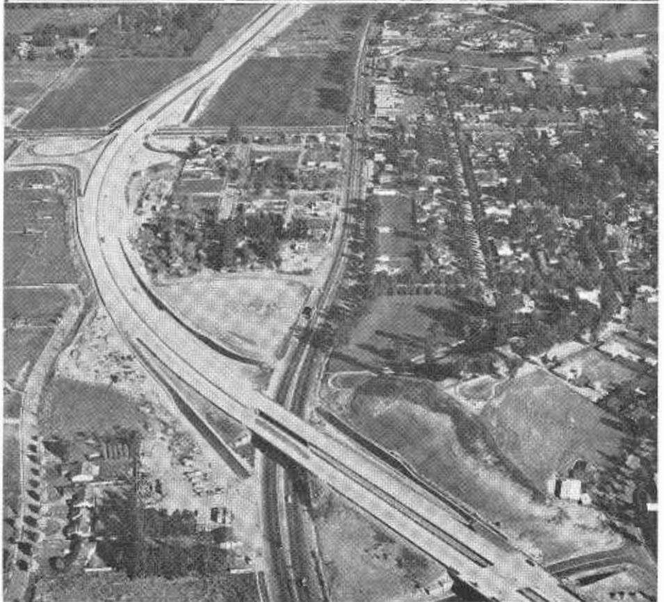
UPPER—Looking east along Ventura Freeway construction near Calabasas showing Mulholland Drive Bridge in foreground. LOWER—Looking east along Ventura Freeway construction in the Woodland Hills area.
