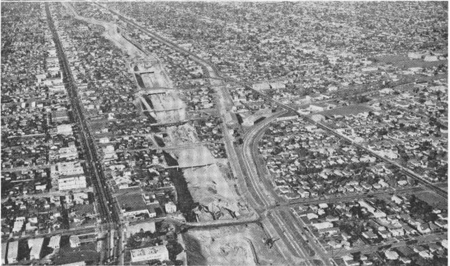
UPPER—Looking north along the Harbor Freeway in the City of Los Angeles showing the Wilshire Boulevard Bridge crossing the freeway in the foreground and the Four-level Traffic Interchange, hub of four major freeways, in the background. LOWER—Looking north along construction in progress on the Harbor Freeway from above 124th Street. Figueroa Street is to the left, Broadway to the right.
