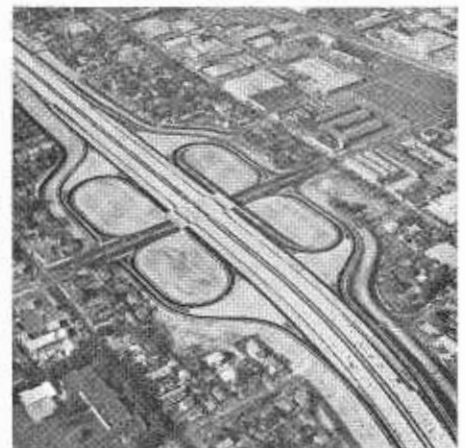
Looking north showing cloverleaf interchange for Golden State Freeway and Western Avenue in Glendale
