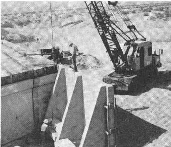
LEFT—Workers place heel planks on wingwall units of a bridge. RIGHT—Tensioning the transverse reinforcement on an abutment.
