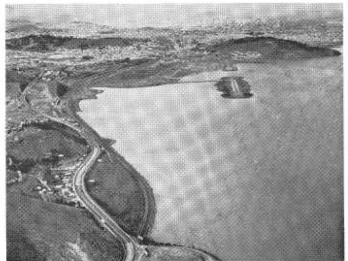
The Bayshore Freeway link between Candlestick Point in San Francisco and Sierra Point in San Mateo County was placed in operation in 1957. The new freeway section (left) is built on an earth fill across open water at the edge of San Francisco Bay. Below is a photograph taken in 1954 during an early stage of the project.
