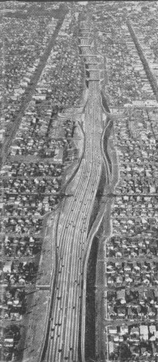
Aerial photo looking north along a completed section of the Harbor Freeway from above Manchester Avenue
