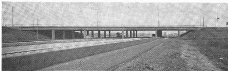
Separation structures such as this on the Eastshore Freeway are typical of the State's freeway construction program
