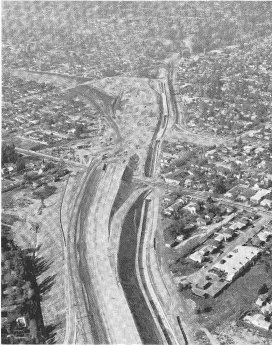
Looking northwest along Hollywood Freeway Extension. Traffic artery in center is Moorpark Street.
