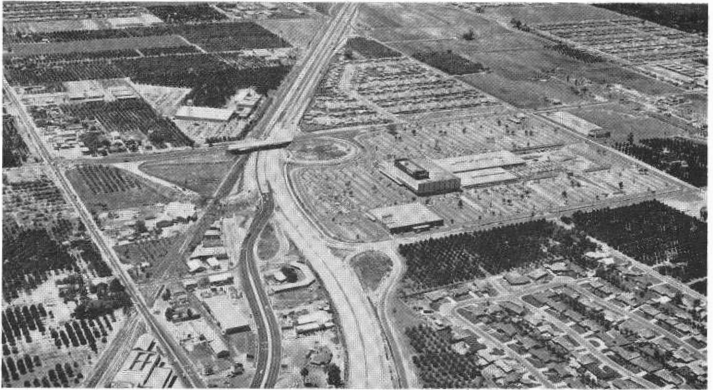
Looking northwest along Santa Ana Freeway under construction between City of Anaheim in foreground and City of Buena Park in background. In center is Broadway-Anaheim shopping center.
