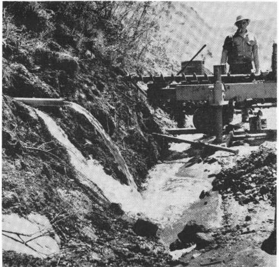
Completed horizontal drain in foreground and boring being made for another drain on a recently completed horizontal drain installation in San Luis Obispo County
