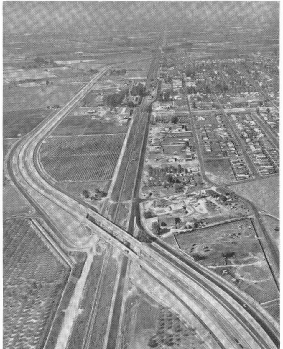
An aerial view looking northwest along the new US 99 Bypass of Atwater. In the foreground is the East Atwater overhead and the Broadway frontage road. The dark road in the center of the picture extending from foreground to background and paralleling the railroad tracks is old US 99.
