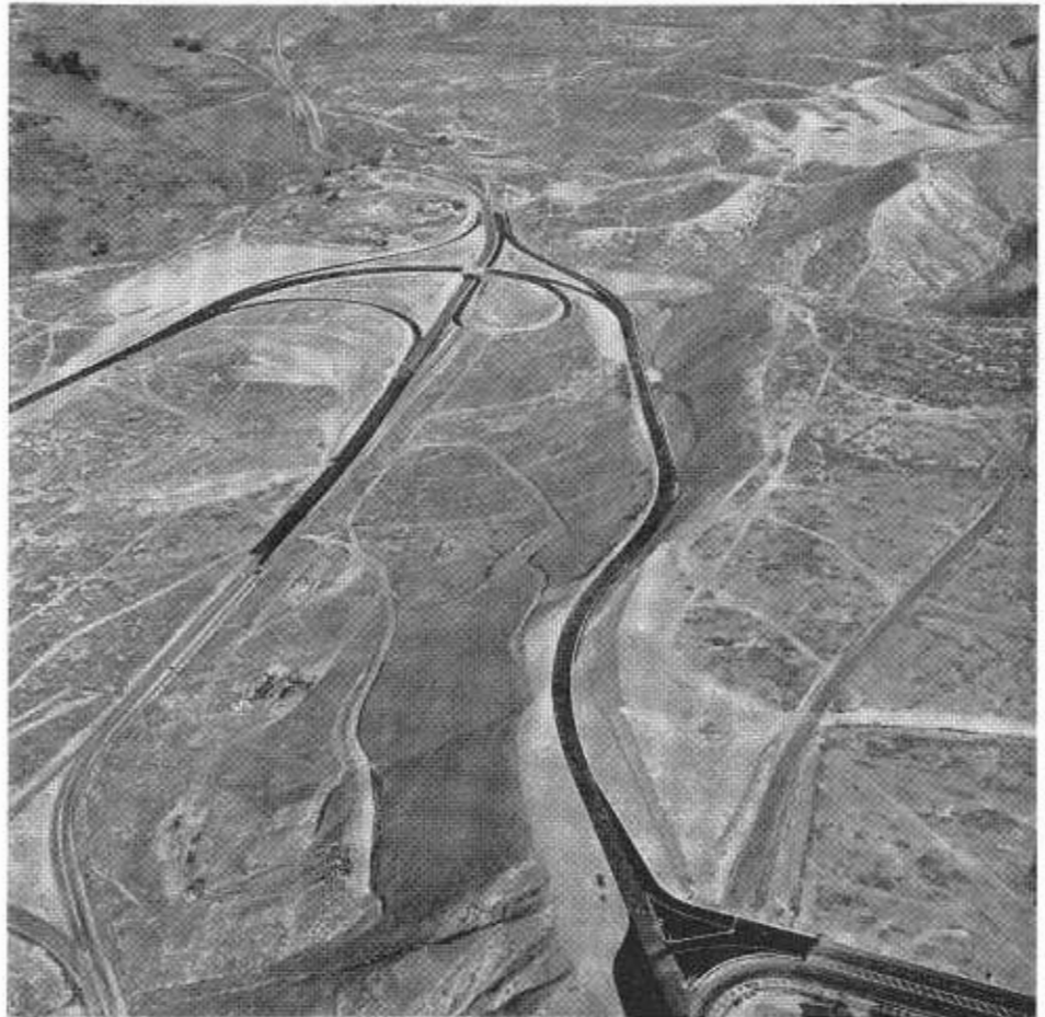
Federal aid secondary county road projects are planned by the county and in most instances constructed with county supervision following review and approval by the Division of Highways. One large-scale 1957 FAS project was this improvement and interchange on the Alfred Harrell Highway near Bakersfield, Kern County.
