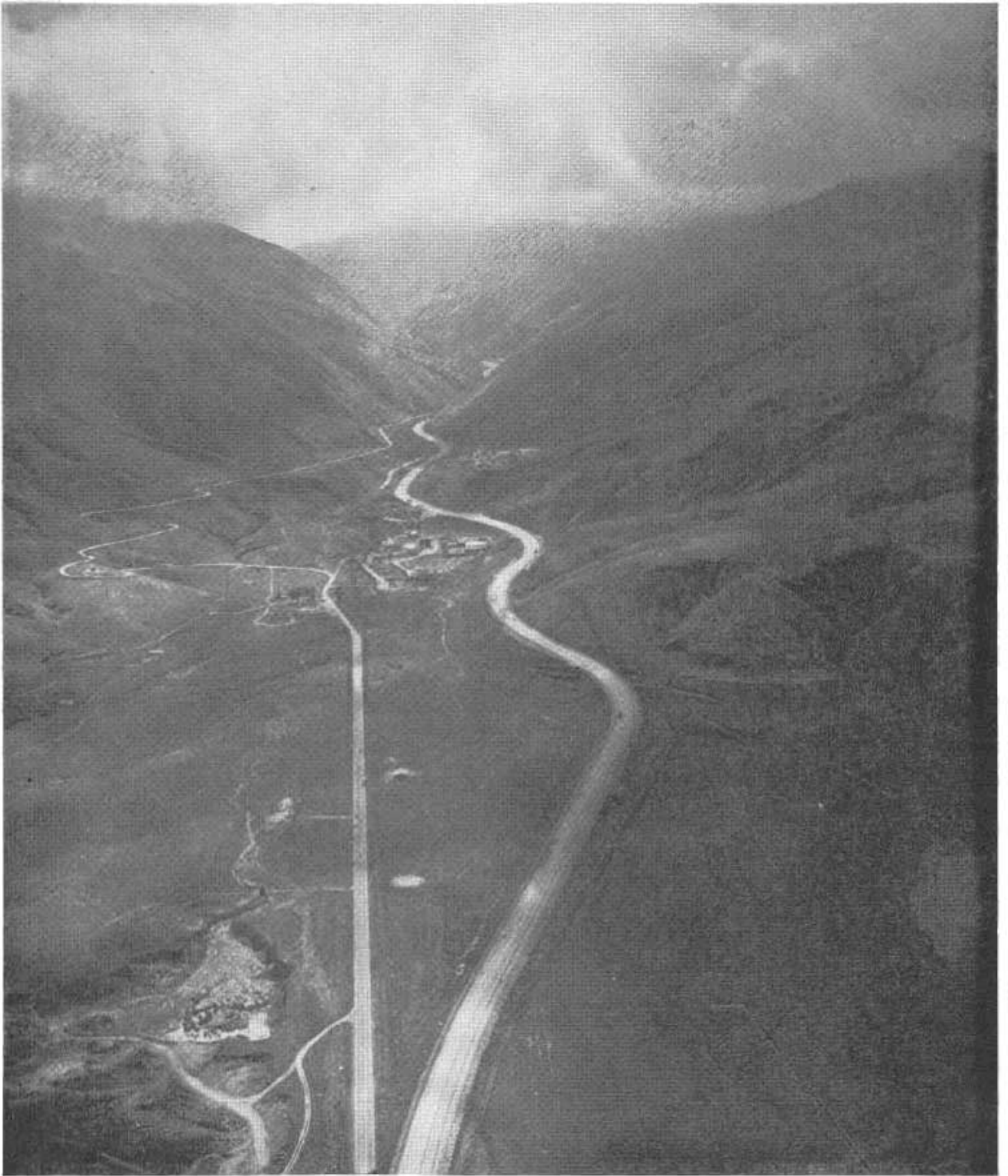
A dramatic shot of the Grapevine Grade showing the present highway (right) heading southward up into the canyon and the old 1914 highway twisting its way up the grade on the left. The present highway is seven miles shorter than the old 1914 road.
