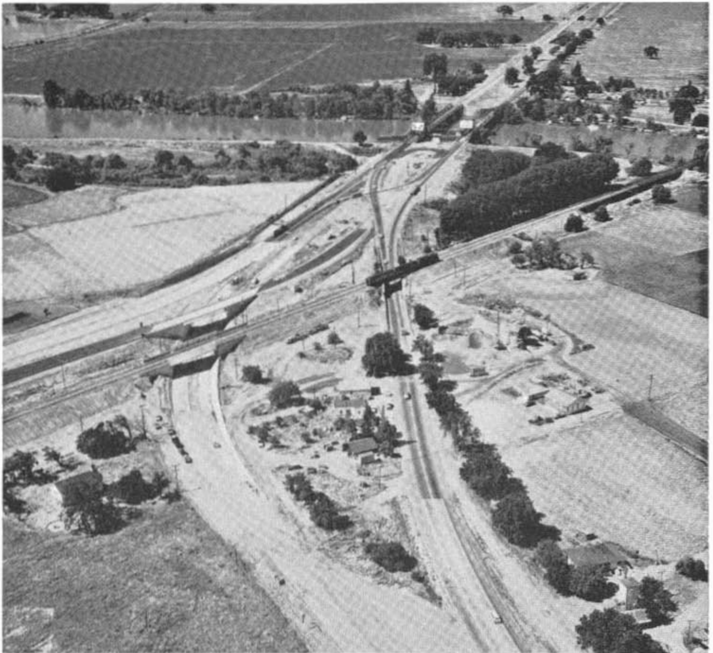
The US 50-Sign Route 120 interchange at Mossdale is nearing completion. The river in the background is the San Joaquin.
