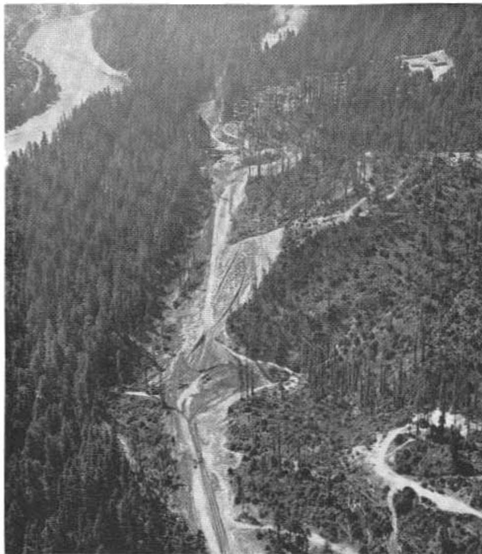
Heavy grading operations on the first unit of the Redwood Freeway. This aerial view southward was taken over High Rock Hill. The river in the upper left is the Eel.
