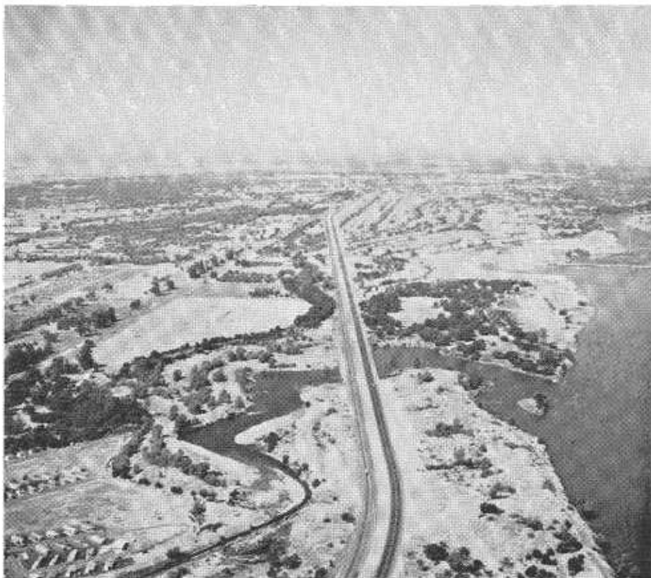
This view eastward shows the four-lane interim improvement on US 50 between Sacramento and Alder Creek. Nimbus Dam and Reservoir is to the right.
