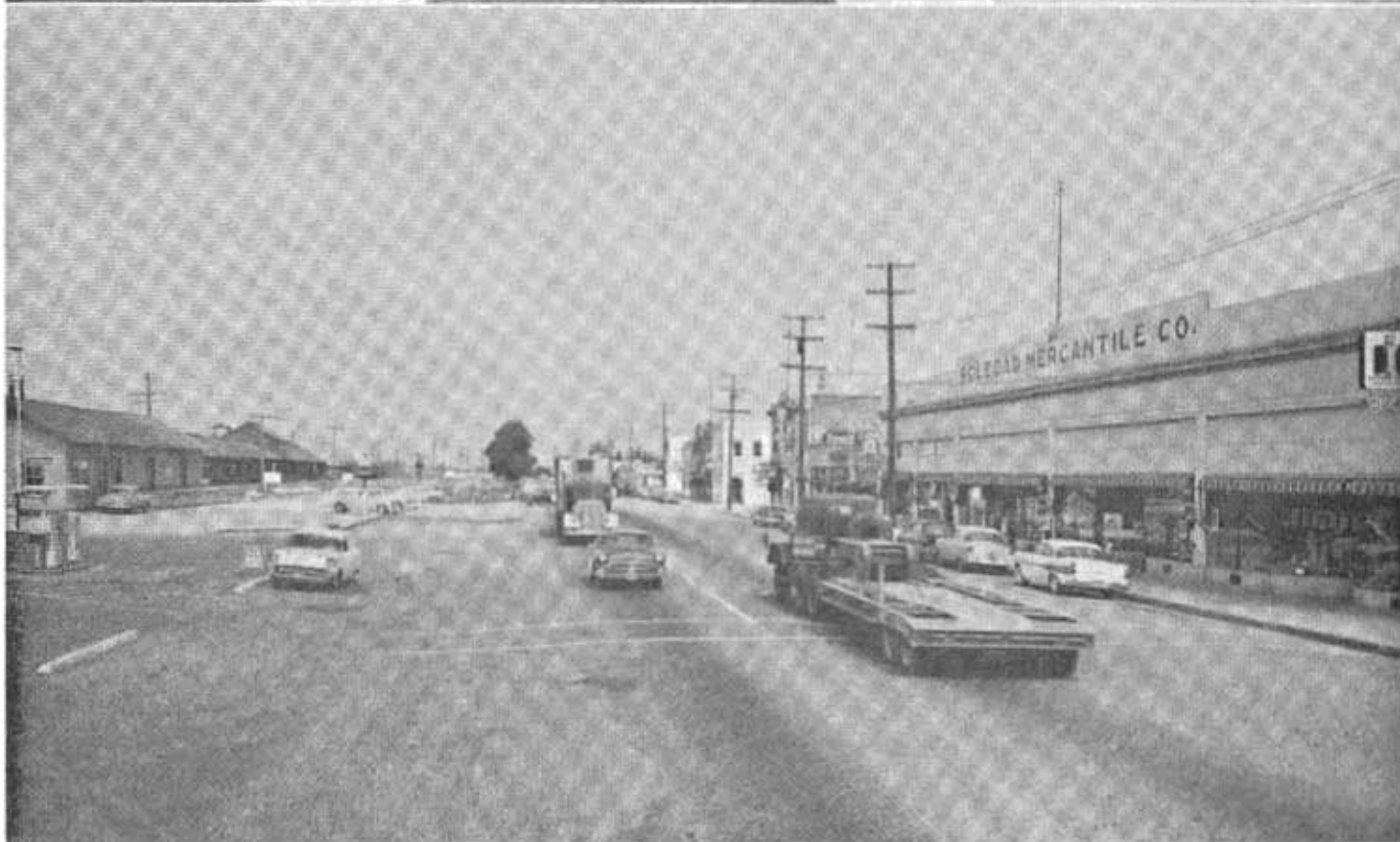
The section of US 101 expressway between Soledad and Greenfield (upper) showing the Arroyo Seco overhead and frontage roads left and right is typical of the new divided, multilane construction replacing such sections as the existing highway through Soledad (lower) with its slow-moving traffic
