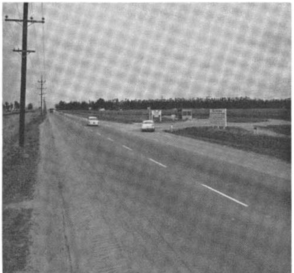
This is US 101 north of Soledad at the entrance to Soledad State Prison as it looked before the contractor began operations in June. New highway lanes will be constructed on the right, parallel to the existing roadway.
