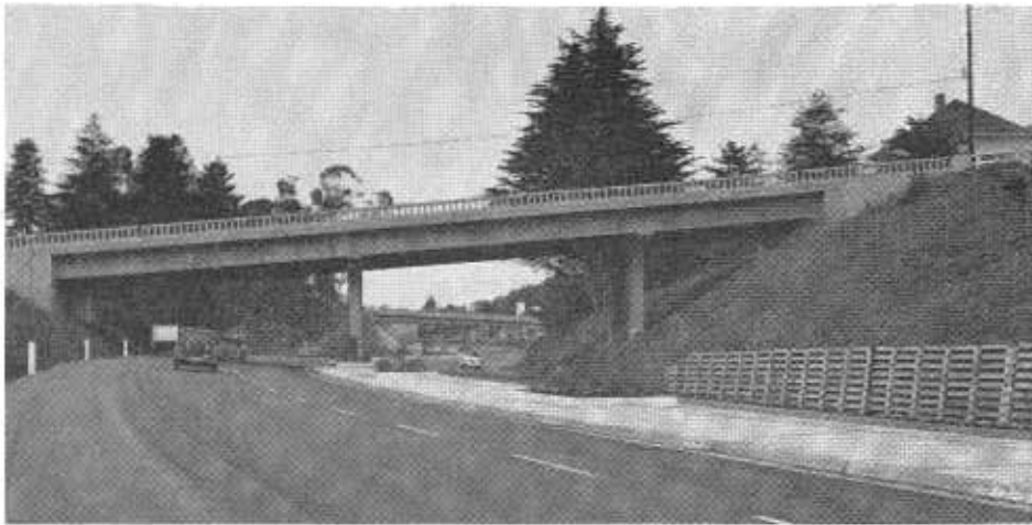
US 101 in Arcata was reconstructed on a new routing east of the central business area. This view northward shows the Ninth and 14th Street overcrossings.
