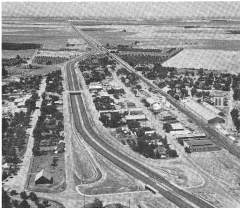
An aerial view of the freeway through the Town of Arbuckle on US 99W. The separation structure in the center of the picture is the Hall Street Overcrossing.
