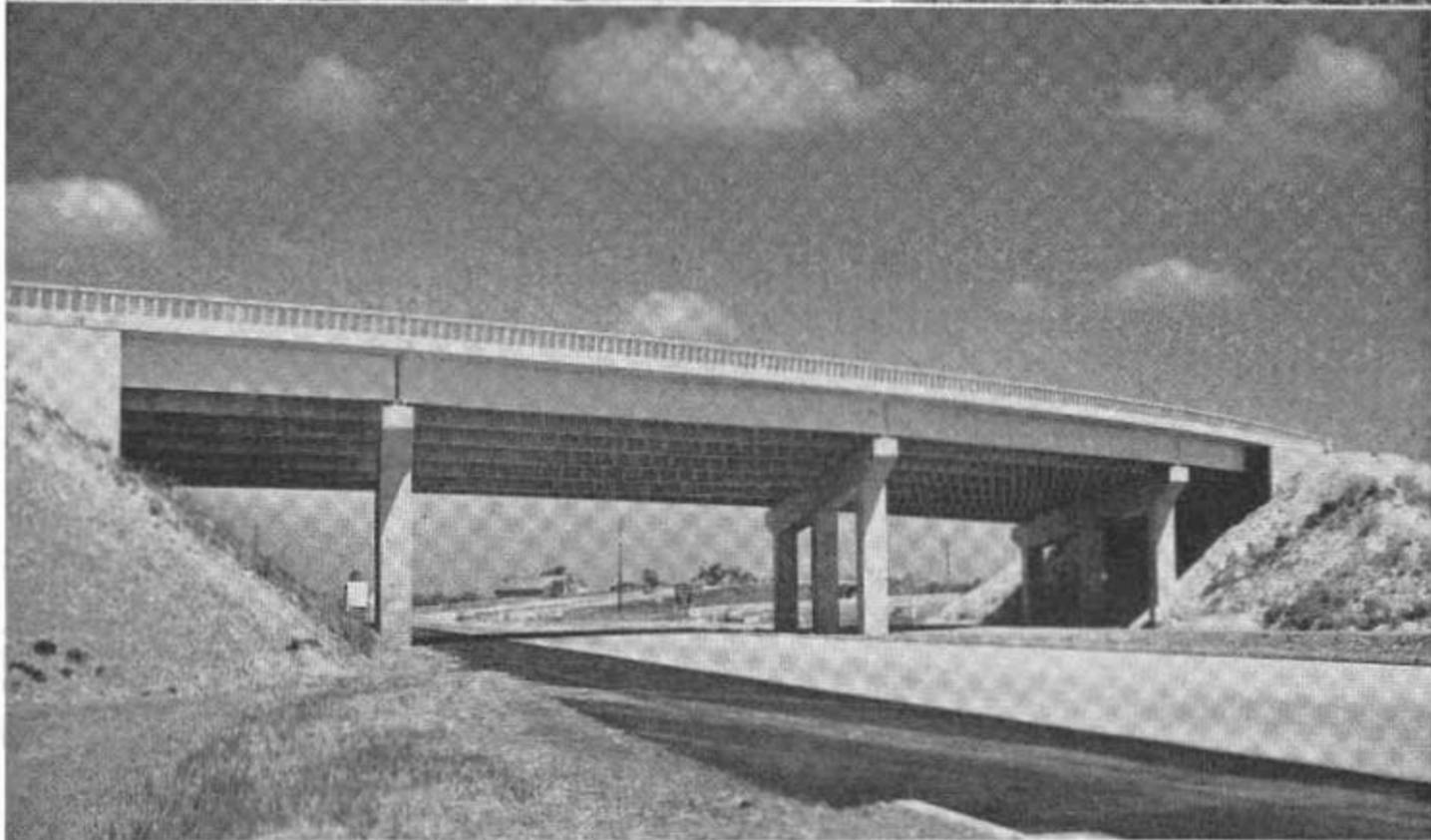
UPPER —This photo, taken from the new Laguna Canyon Road traffic separation structure, shows the new section of the Santa Ana Freeway looking south toward San Juan Capistrano. LOWER —The new traffic separation connecting Laguna Canyon Road with the Santa Ana Freeway. (Story on previous page.)
