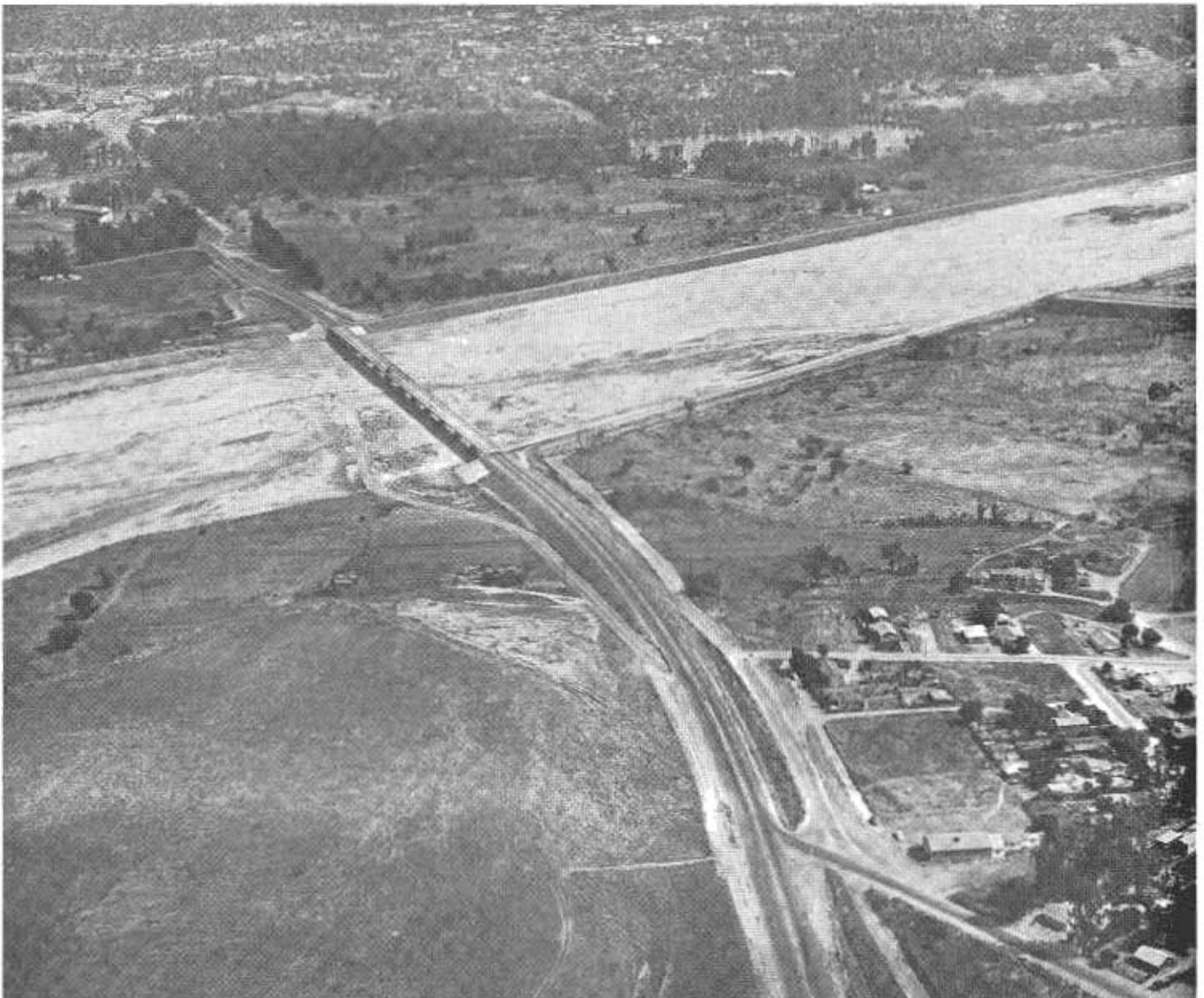
An aerial view of the new Crestmore Road and Bridge with the City of Riverside in the distance. The bridge was lengthened by Riverside County under the Federal-aid Secondary program. The river is the Santa Ana.
