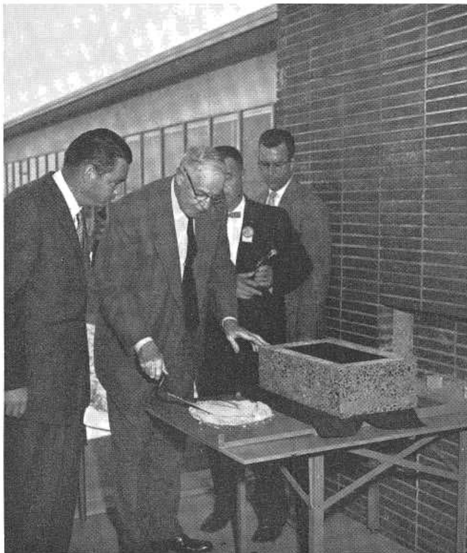
Commissioner Chester H. Warlow trowels mortar while Director of Public Works C. M. Gilliss (left) and members of the Highway Laboratory staff look on
