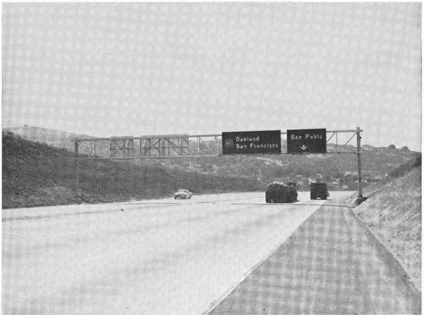
This is a sign bridge. In this type the Standard Plans cover structures up to 10 feet high by 130-foot span. Although walkways and safety railing are on this structure, they are hardly perceptible to the motorist.
