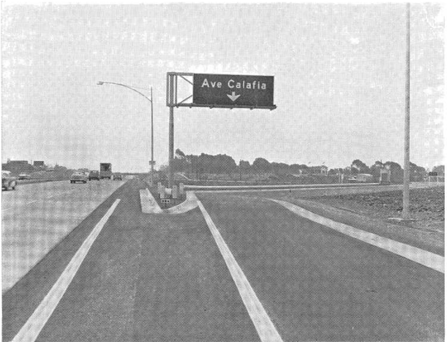
Pictured here is a cantilever type sign structure. This type of sign reaches maximum proportions of 10 feet by 30 feet.
