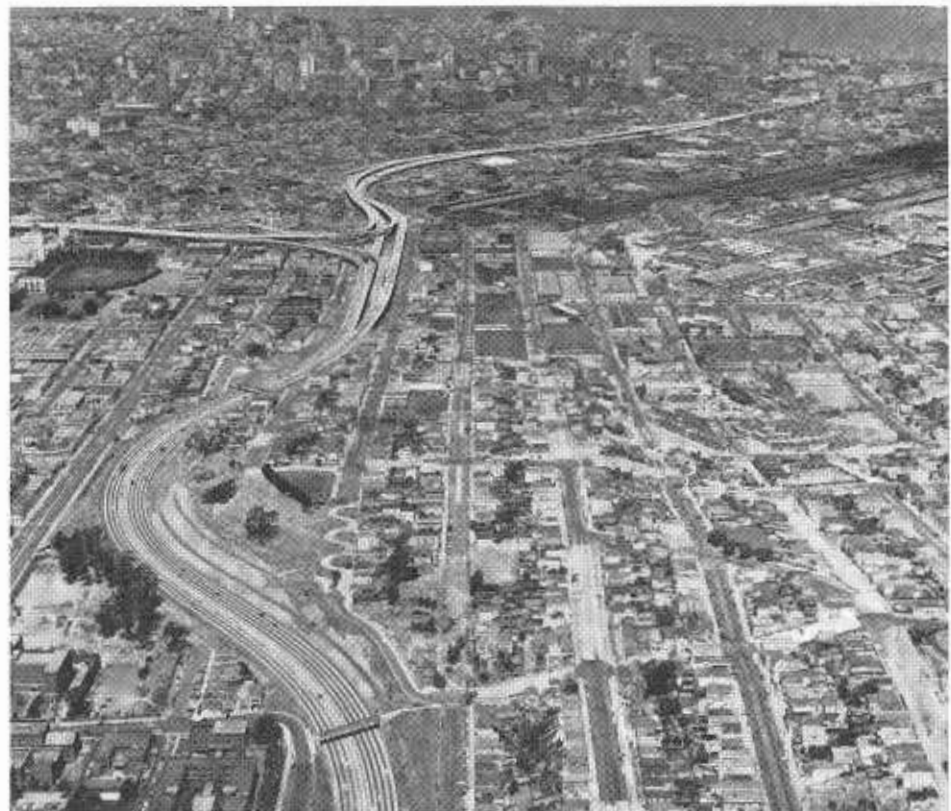
“ * * * The State has assumed full responsibility for the costs of constructing and maintaining state highways in cities * * * California has probably gone further than any other state in this direction, and the more impressive freeways for which we are known are actually state highways in urban areas.” UPPER—Aerial view along Blackstone Avenue in Fresno (State Sign Route 41), a major city arterial recently widened by the State. LOWER—Typical state-built freeway development, in San Francisco.
