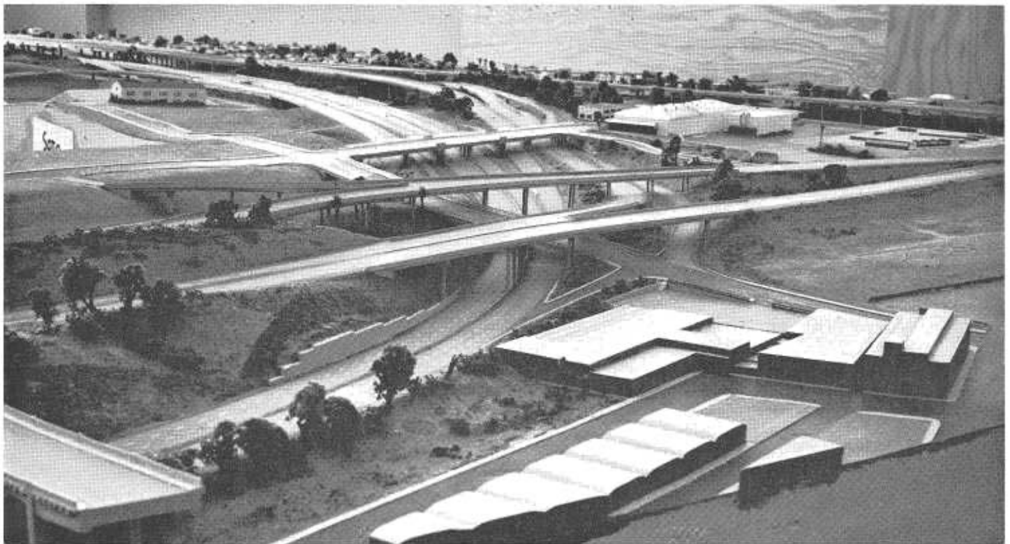
A photo of the model near completion stage. In the foreground is the three-level structure which will carry the Golden State Freeway across Seventh Street and the Santa Ana Freeway.
