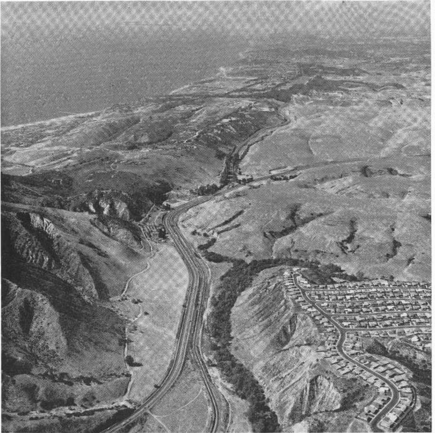
This aerial view northward was taken above US 101 in Rose Canyon two miles north of Balboa Avenue
