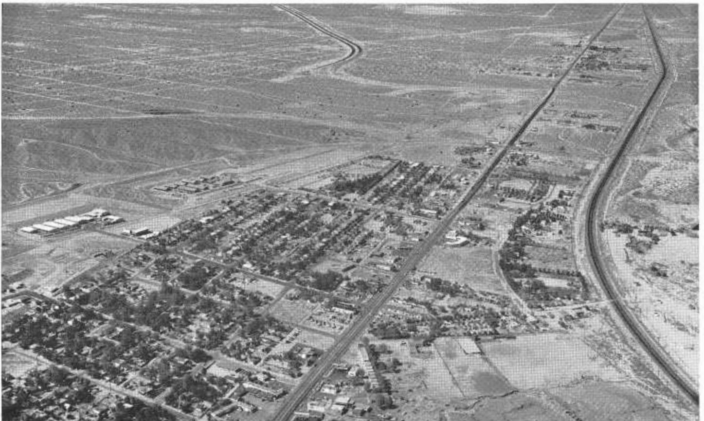
UPPER—The State Street interchange on US 66-91-395 under construction near the north entrance to San Bernardino from Cajon Pass. LOWER—An aerial taken over Barstow showing the construction on the northern end of the Victorville-Barstow Freeway in the distance.
