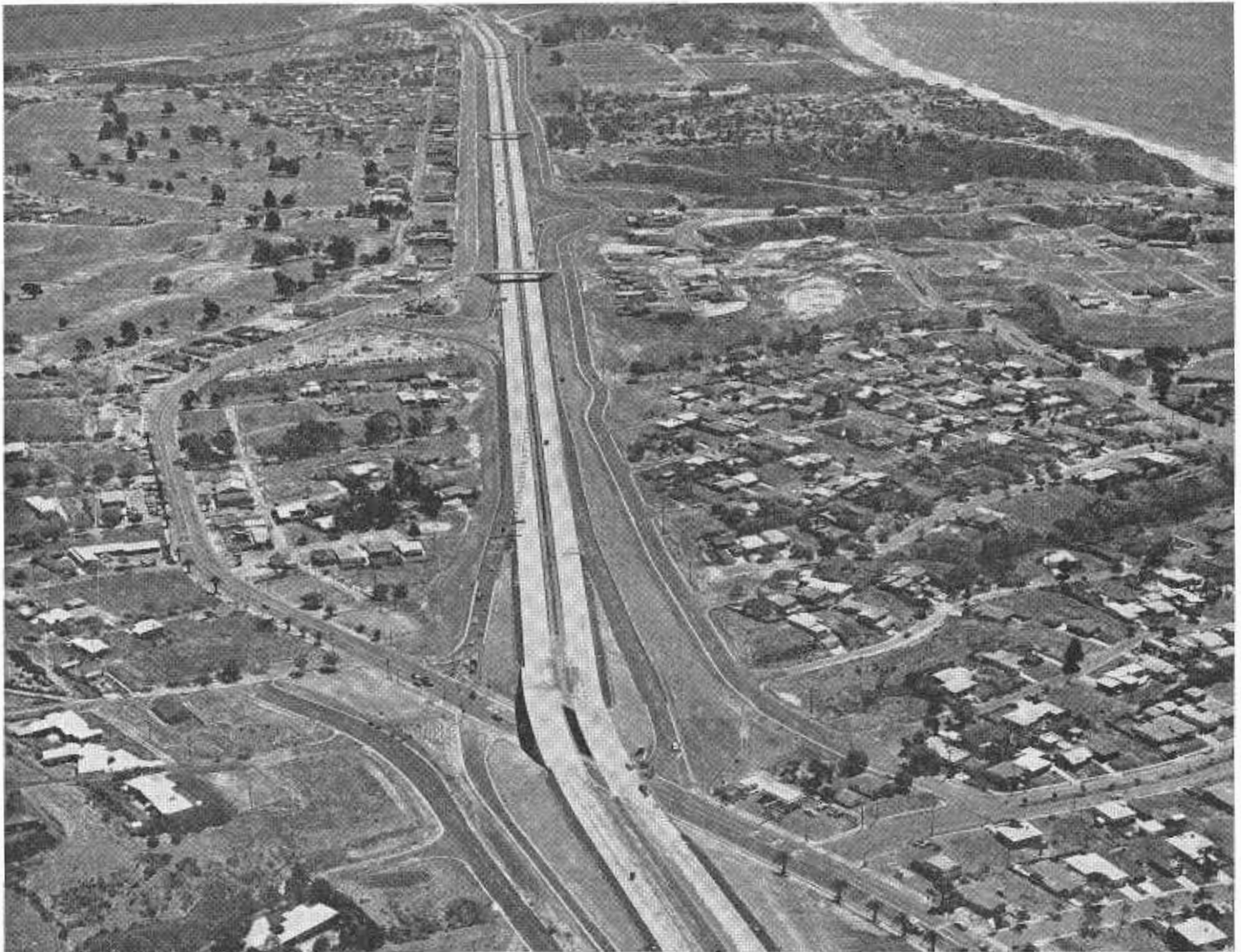
Looking south along the new freeway through San Clemente. The north connection with present US 101, which passes under the freeway, can be seen in the foreground.
