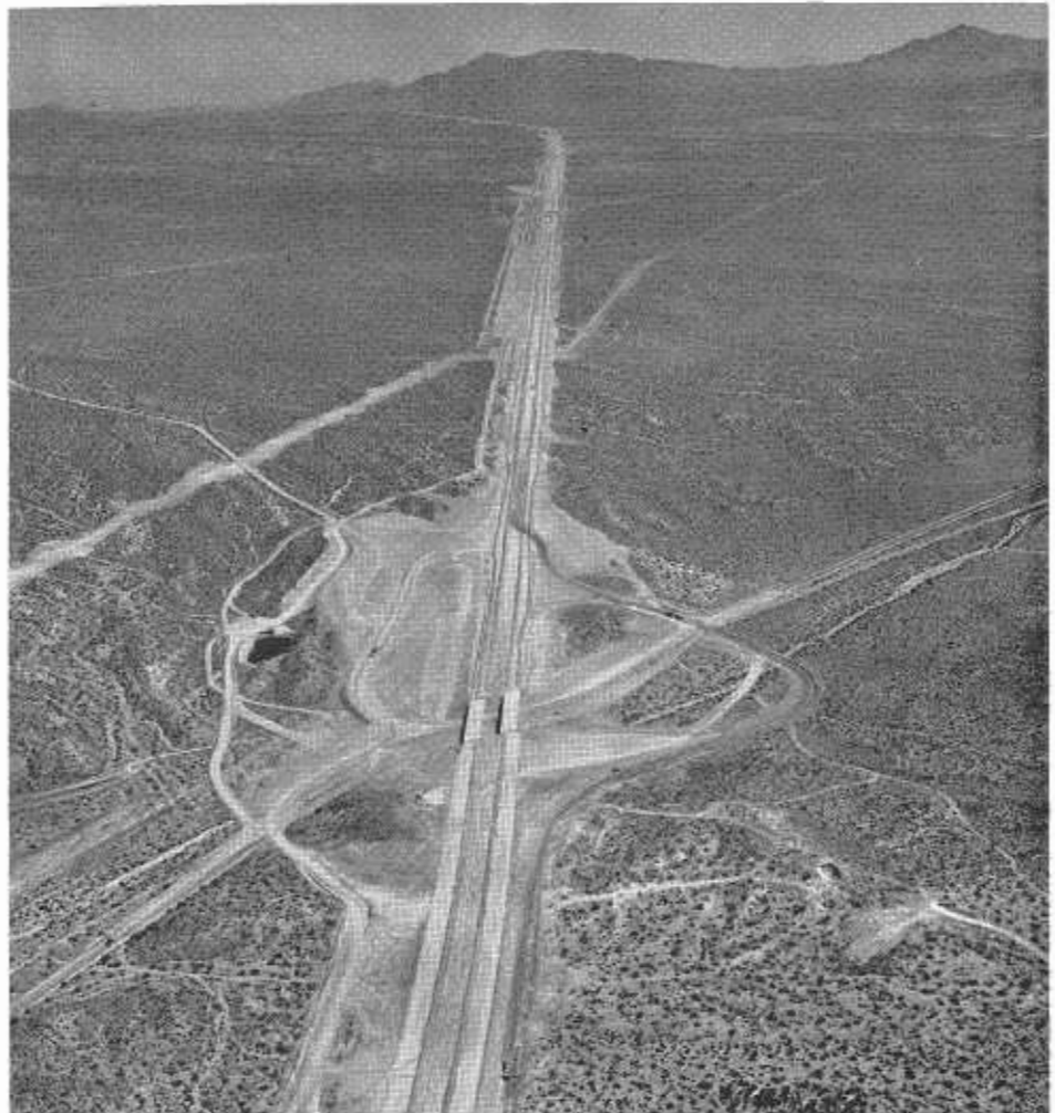
California highway construction is performed under contracts awarded on the basis of competitive bidding. The longest freeway ever built in California under one contract was opened in December, 1958. A portion of this 29-mile stretch of freeway on US Highway 91-66 between Victorville and Barstow is shown above during construction.
