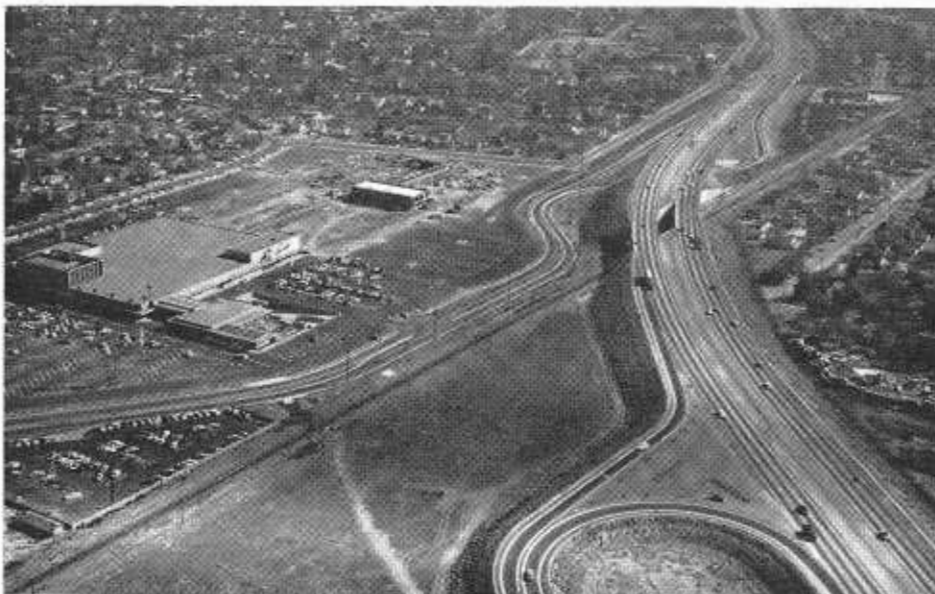
An aerial view of the San Bernardino Freeway through the City of El Monte. Peck Road interchange is in the foreground.
