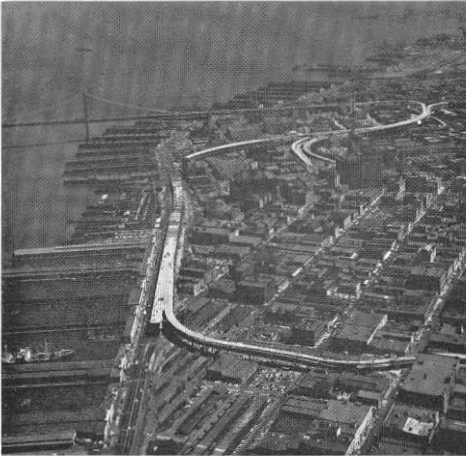
At the end of 1958 work was nearly completed on this section of the double-deck Embarcadero Freeway in San Francisco. In the background is a portion of the San Francisco-Oakland Bay Bridge.
