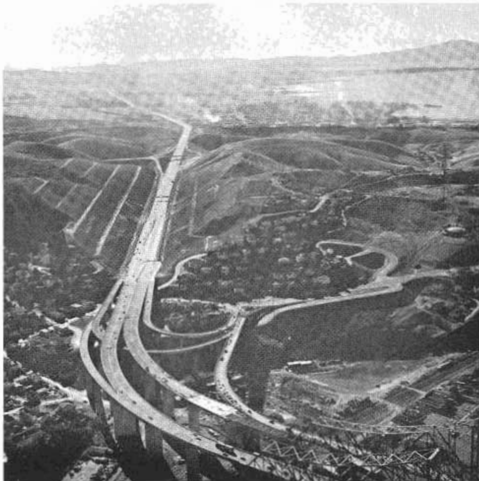
Motorists on the new US Highway 40 freeway approaches to the Carquinez Bridges in Contra Costa County travel through a manmade canyon believed to be the largest cut in the history of road building. The "Big Cut" is a quarter-mile wide at the top and up to 350 feet deep.
