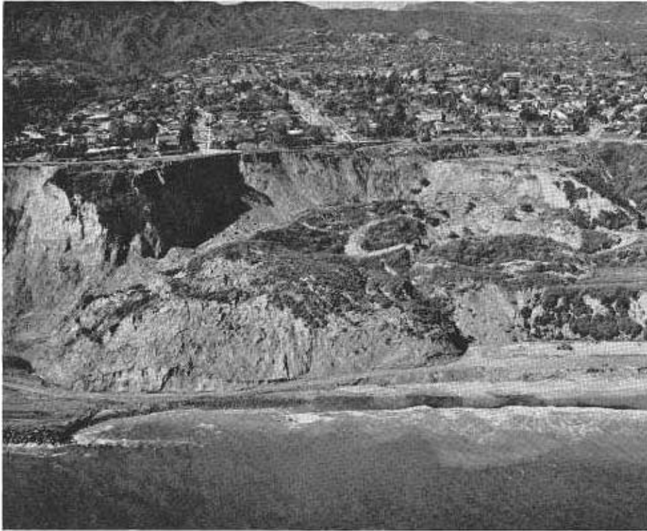
This huge landslide along the Pacific Palisades closed US Highway 101 Alternate near Santa Monica and took the life of a Division of Highways maintenance superintendent. A temporary detour was constructed to reopen the highway, and at the end of the year work was being pushed on rerouting the highway around the slide.
