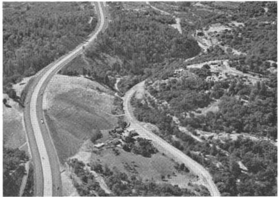
This new stretch of freeway west of Auburn was one of four freeway sections completed during 1958 on US Highway 40 east of Sacramento. Completion of other current and budgeted projects on this route will leave only one 11-mile gap in continuous freeway and expressway between the state capital and Nevada. (Note old highway winding through Auburn Ravine at right.)
