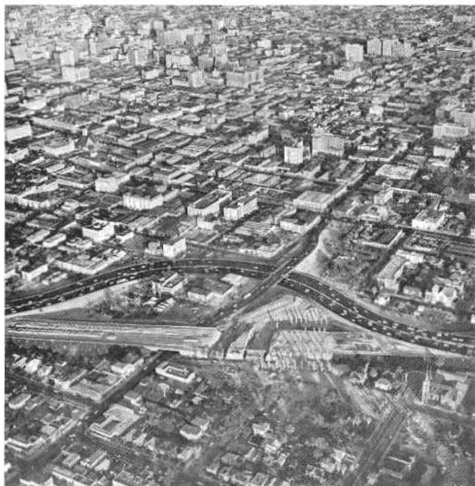
This view northeast toward downtown Los Angeles shows the detour now in operation on the Harbor Freeway while bridges for the future interchange with the Santa Monica Freeway are being constructed.
