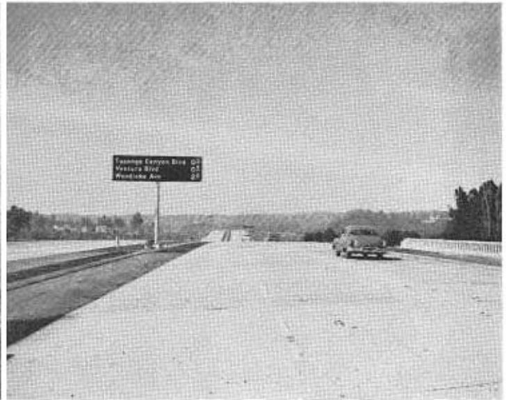
Constant improvements are being made in the design and placement of directional signs on freeways to make it easier for motorists to find their destinations. At left is an overhead illuminated sign bridge typical of those now used extensively on freeways. At right is a sign showing distances to the next three turnoffs. Standard plans and specifications for freeway sign structures have been developed and are included in major freeway construction contracts.
