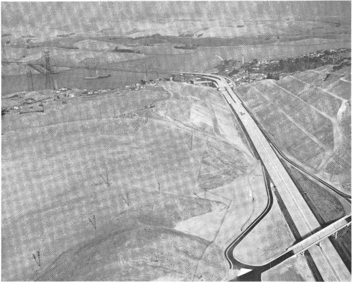
Picture showing the "Big Cut" completed with the Carquinez Bridge in the background. To the right can be seen the 30-foot benches spaced every 60 feet in elevation going up the side of the cut. Slope of cut between benches is 2:1; that is one foot up for every two feet horizontal.
