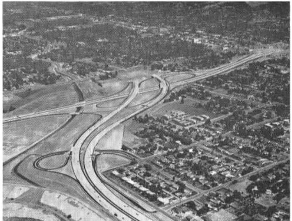
This view to the northeast along the Ventura Freeway shows the interchange with the San Diego Freeway.
