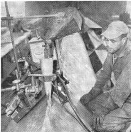
One of the heavy box section compression members being welded by the submerged arc process at one of the American Bridge fabricating plants.
