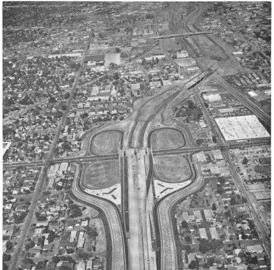
Looking north along a section of the Golden State Freeway showing construction through the City of Burbank. The cloverleaf in the foreground is the Alameda Avenue interchange.
