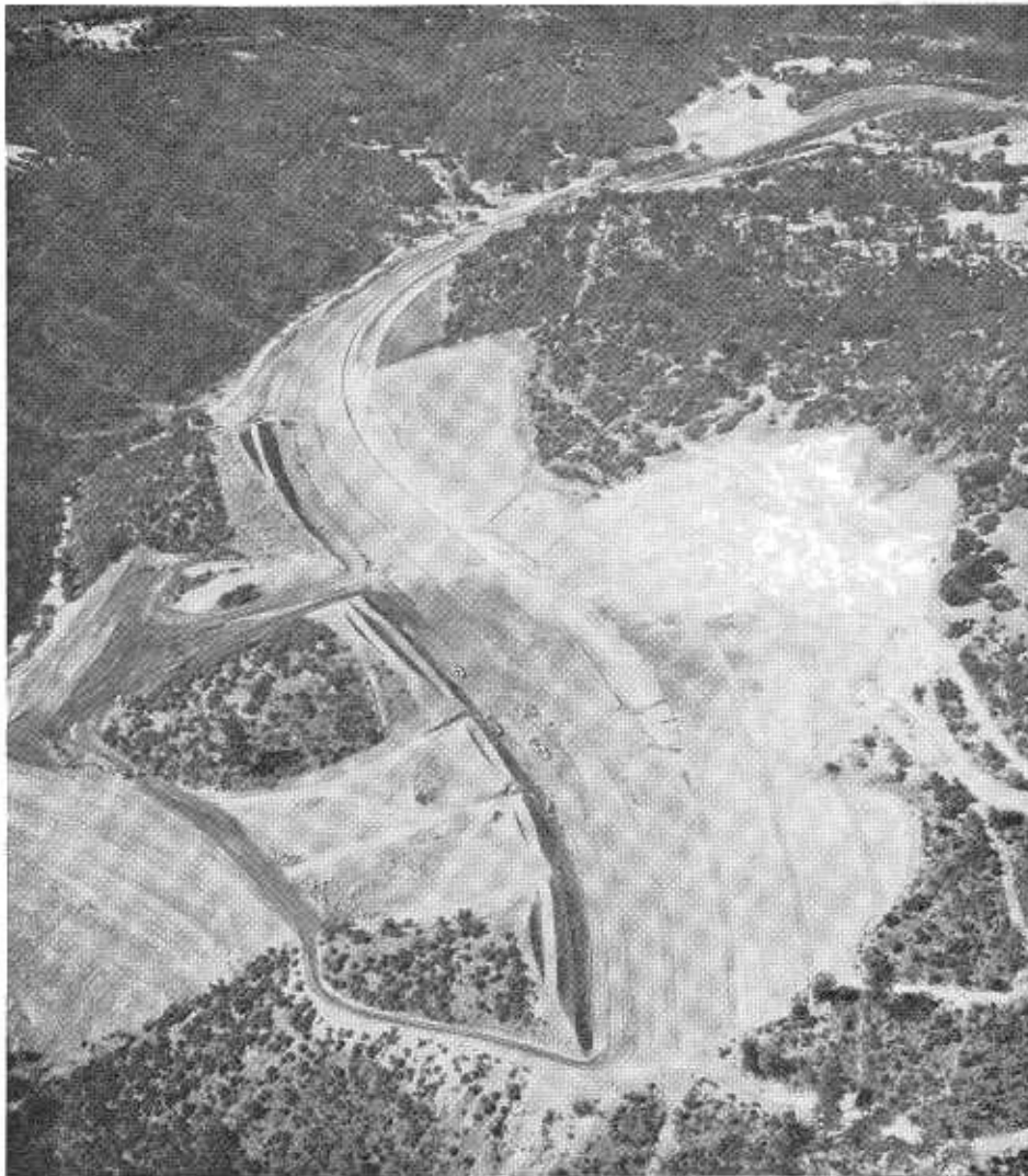
This large benched cut on US 40 Alternate in Butte County is located just south of the future location of the new West Branch Bridge.
