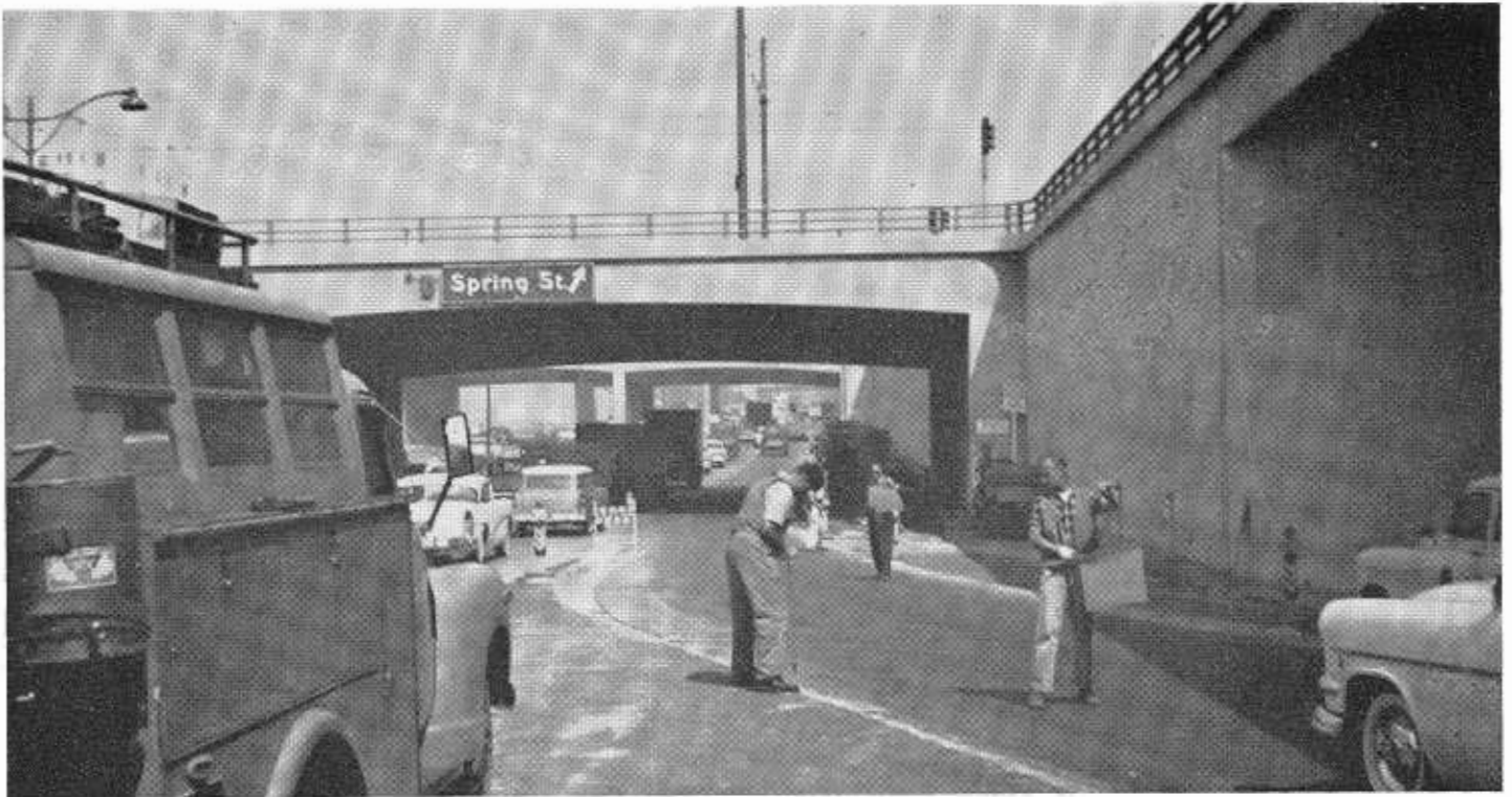
Traffic on a freeway inlet is temporarily stopped while surveying operations are in progress.
