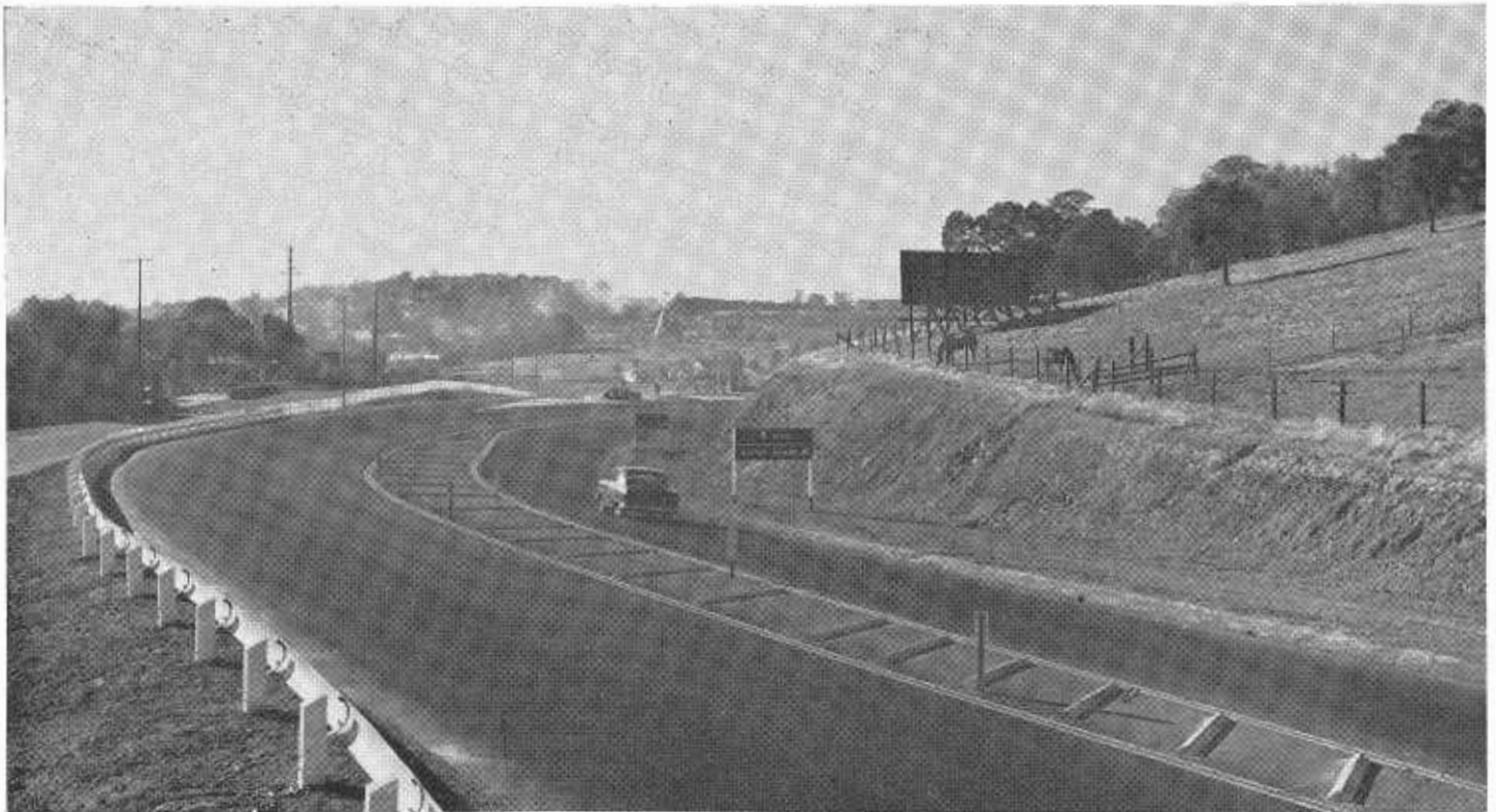
The Martell Junction looking northwest. The highway in the foreground is combined Sign Route 88-49 with Sign Route 88 to lone bearing left and Sign Route 49 North bearing to the right.
