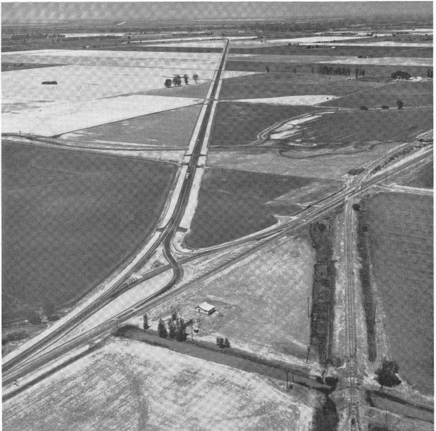
This new section of Drescher Boulevard in Sutter County is the final link in 41 miles of improved highway between Yuba City and Sacramento. From a connection with State Sign Route 24, the recently completed FAS road (center) extends northwest toward Nicolaus, where a new bridge carries traffic across the Feather River.
