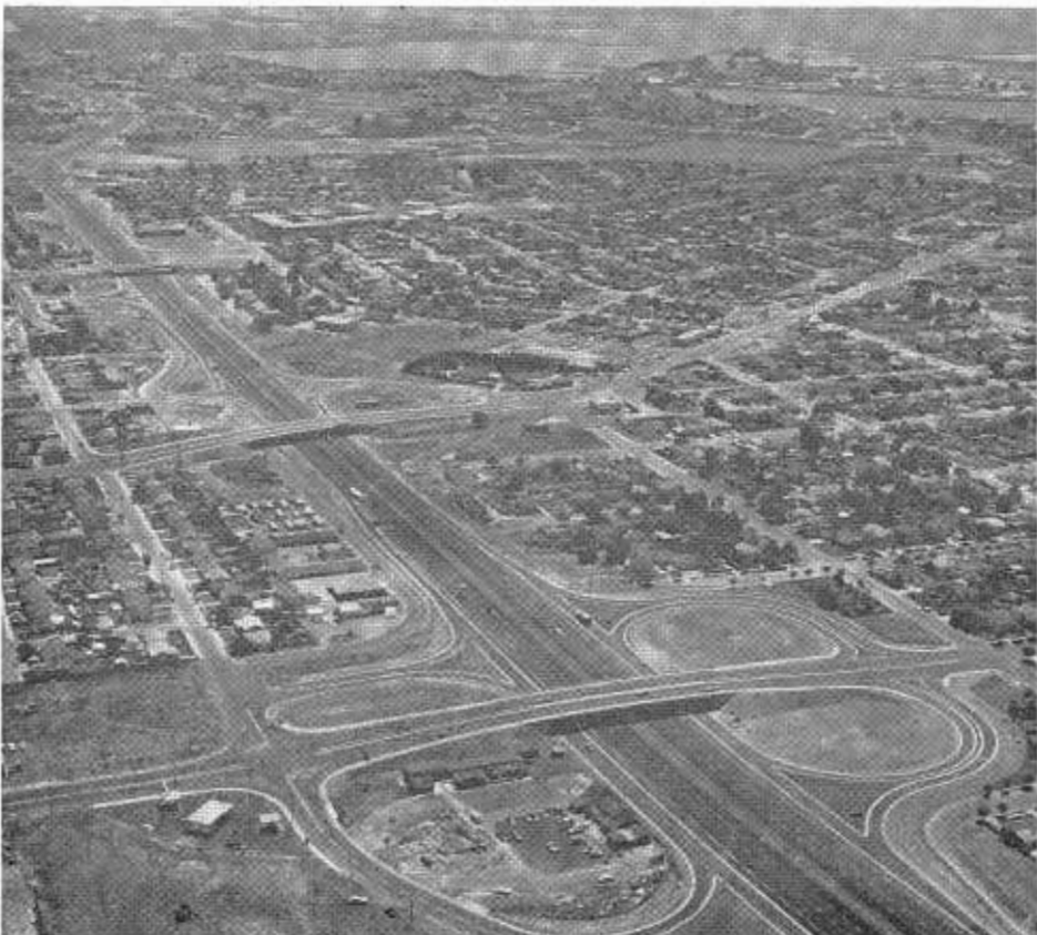
UPPER—The Mariposa Road (foreground) and Farmington Road Interchange on US 99 in San Joaquin County, a step in the conversion of the Stockton Bypass from expressway to full freeway. LOWER—The new US 40 freeway through Vallejo. In the foreground is the Tennessee Street Interchange.
