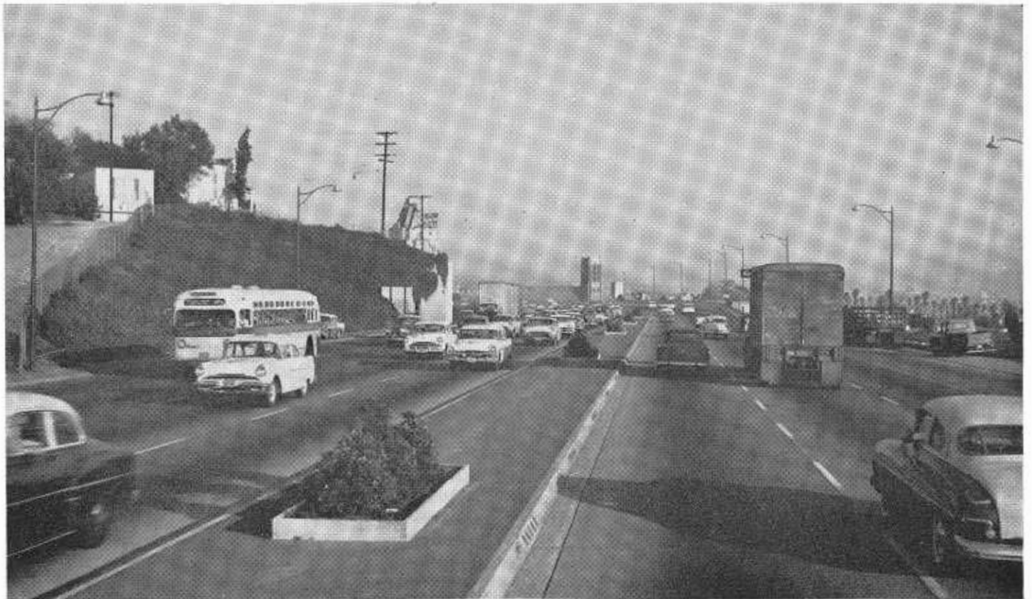
UPPER—The effectiveness of various median designs was evaluated in a recent Division of Highways safety study. Medians with barriers, such as this one on the James Lick Freeway in San Francisco, were among those classified as nontraversable. LOWER—This type of curbed center strip on the Hollywood Freeway in Los Angeles was one of the deterring median designs included in a recent Division of Highways freeway safety study.
