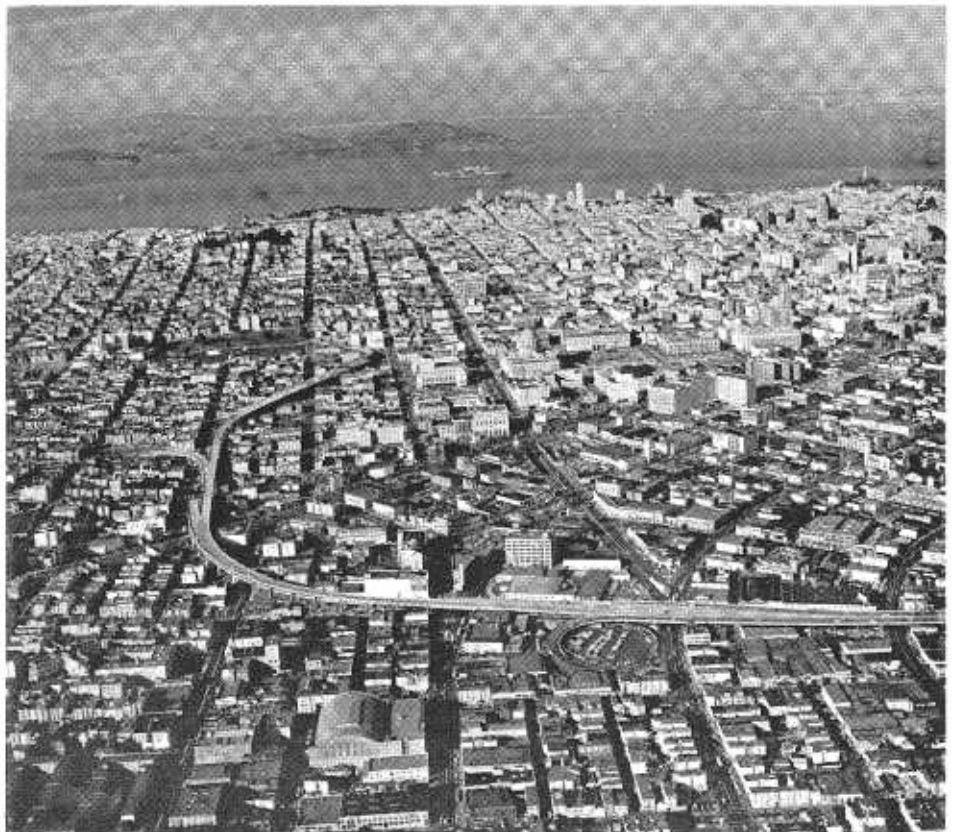
UPPER The new Embarcadero Freeway in San Francisco connects traffic with Main, Beale, Mission, Fremont and Folsom Streets and north of Market Street with Broadway, Sansome and Battery Streets. LOWER—The Central Freeway Extension from South Van Ness Avenue (lower right) to Turk Street (center left). Civic Center in right middleground.
