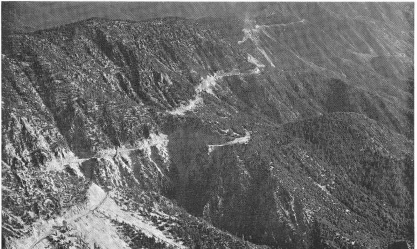
UPPER—Another view of the rugged terrain through which the road is being constructed. LOWER—An aerial showing the alignment of the road. Note the dust cloud in the background where the construction is going on.
