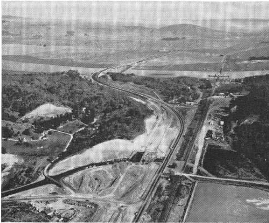
Expressway construction on the Black Point Cutoff (Sign Route 37) with the new bridge across Petaluma Creek in the upper center and the Atherton Avenue interchange in the foreground.
